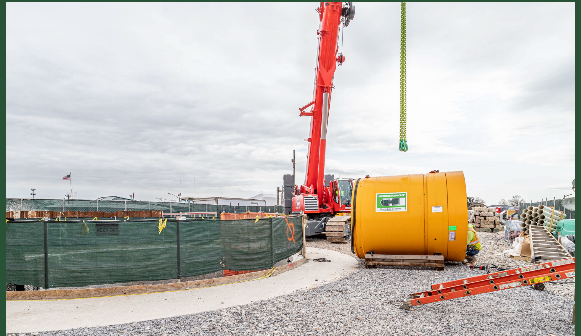
Construction Site at BP2 (April 2022)
