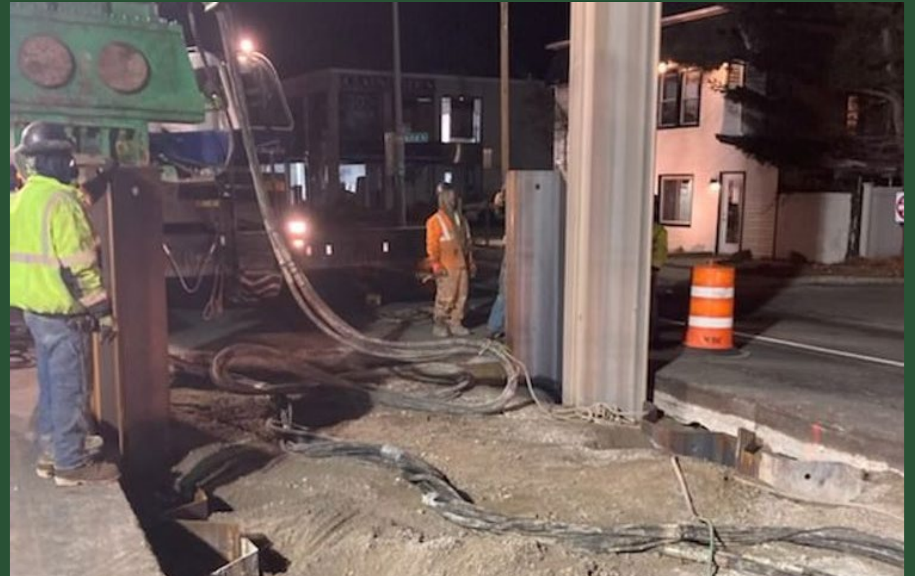
Sheeting Installation at Pit R (January 2022)
