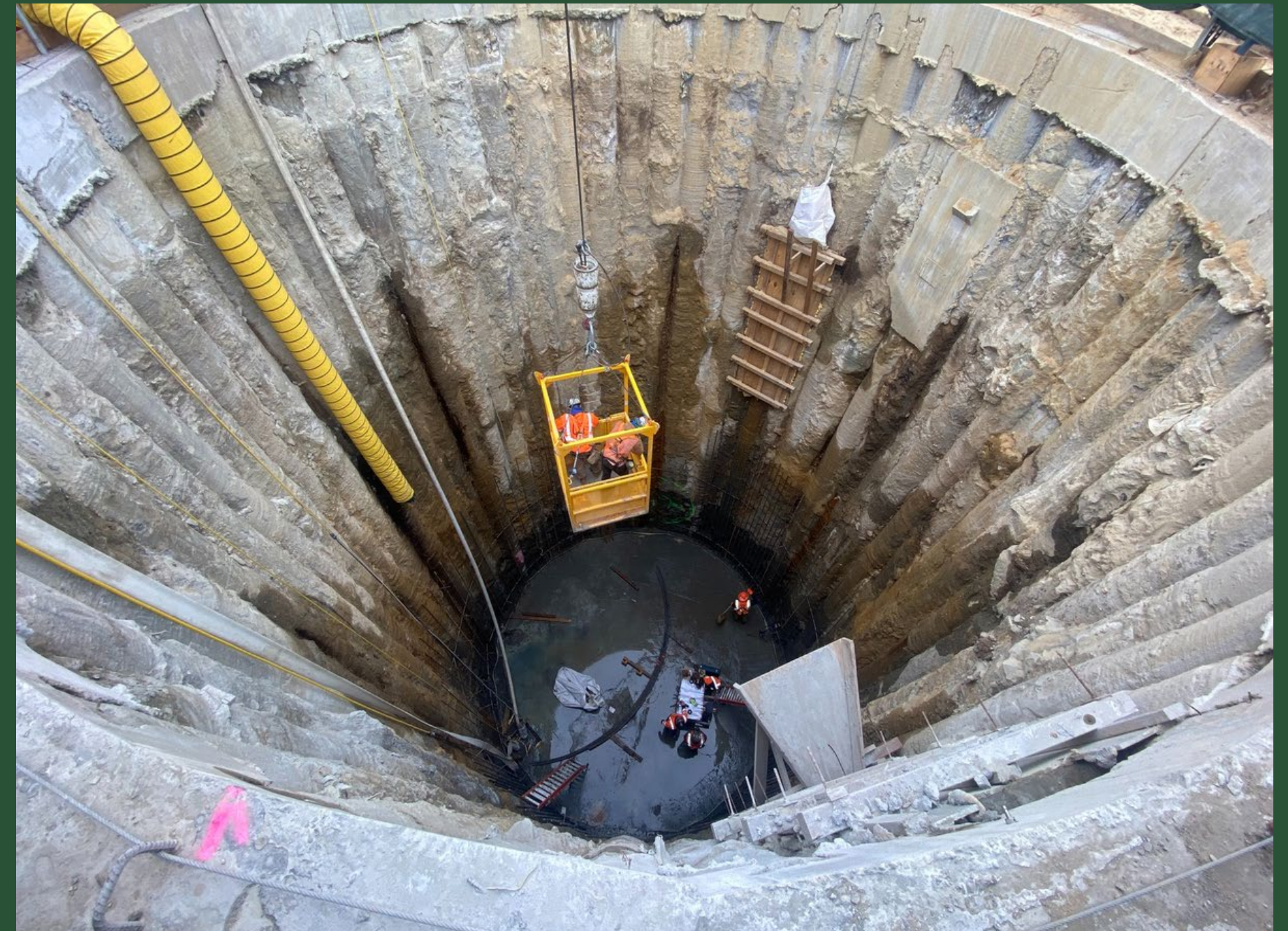
Shaft Liner Installation at CC2 (March 2022)
