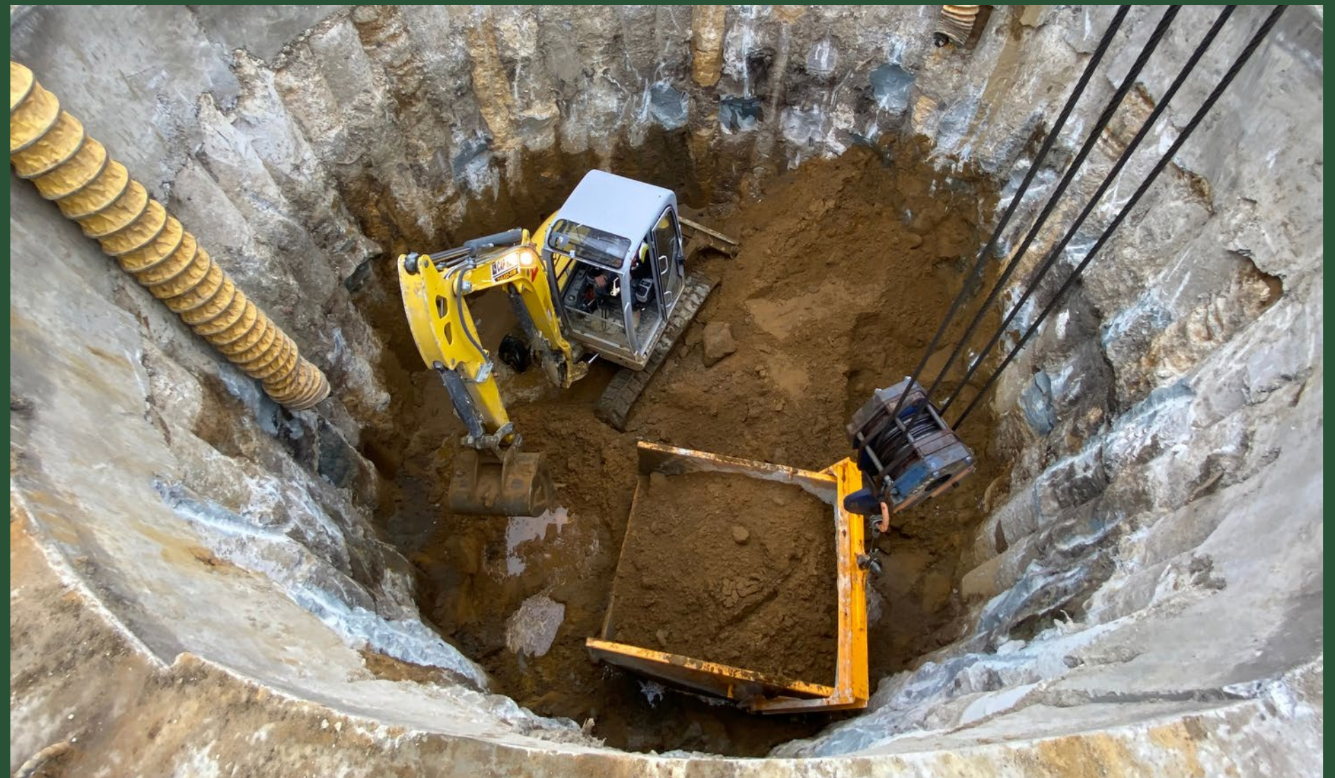
Shaft Excavation at BP4 (April 2022)
