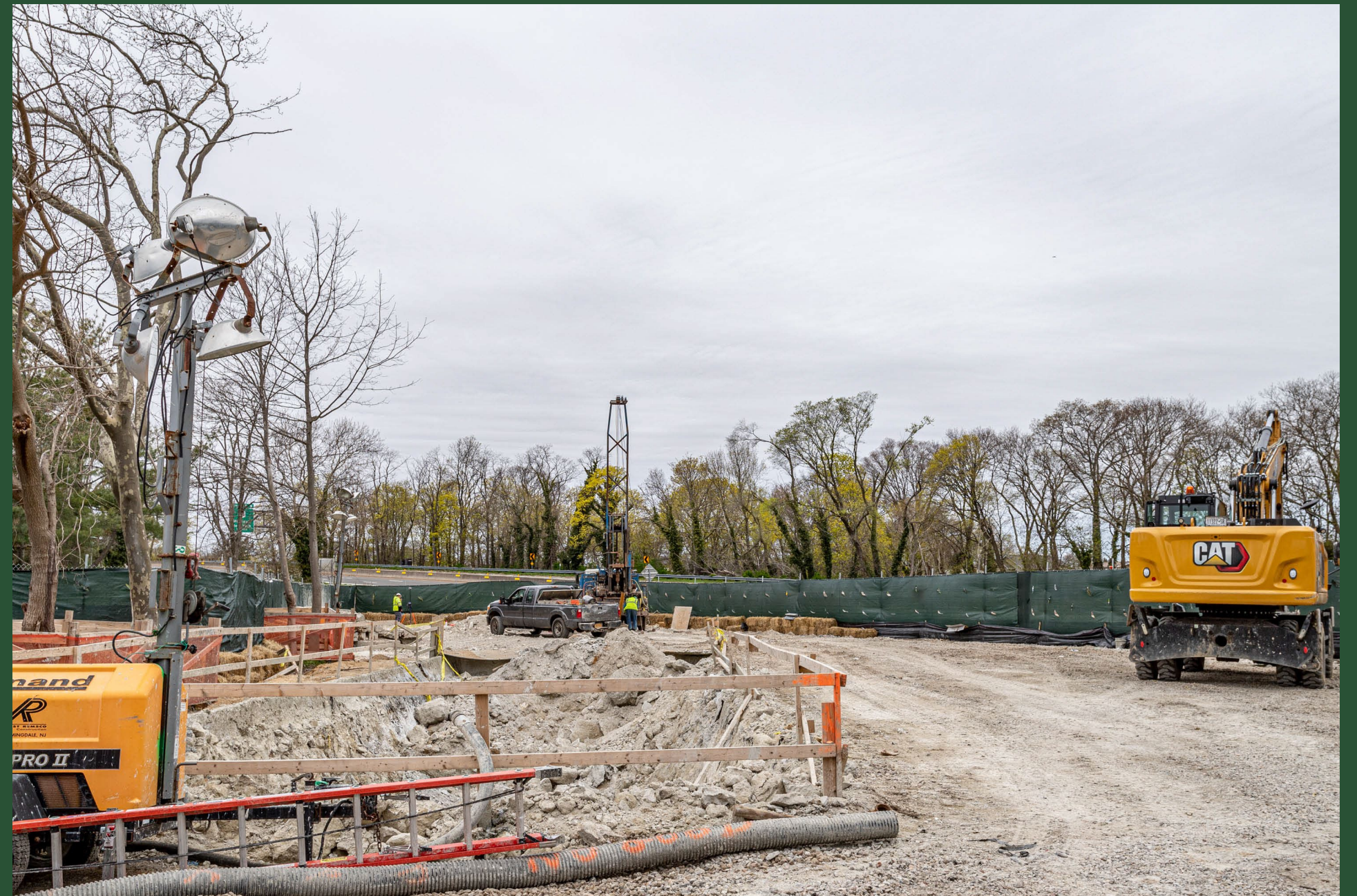
Construction Site at CC4 (April 2022)
