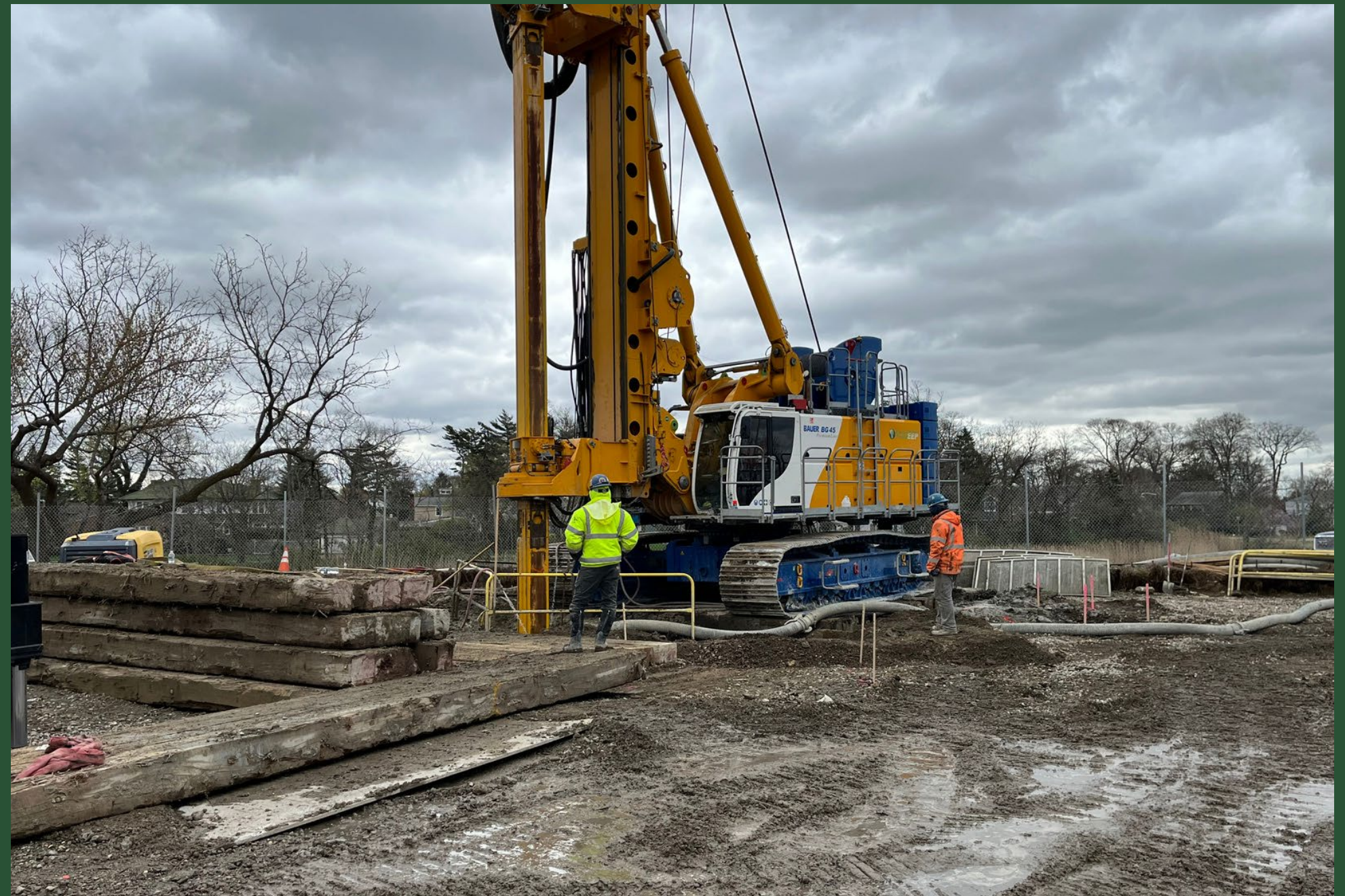
SOE Installation at BP7 (April 2022)
