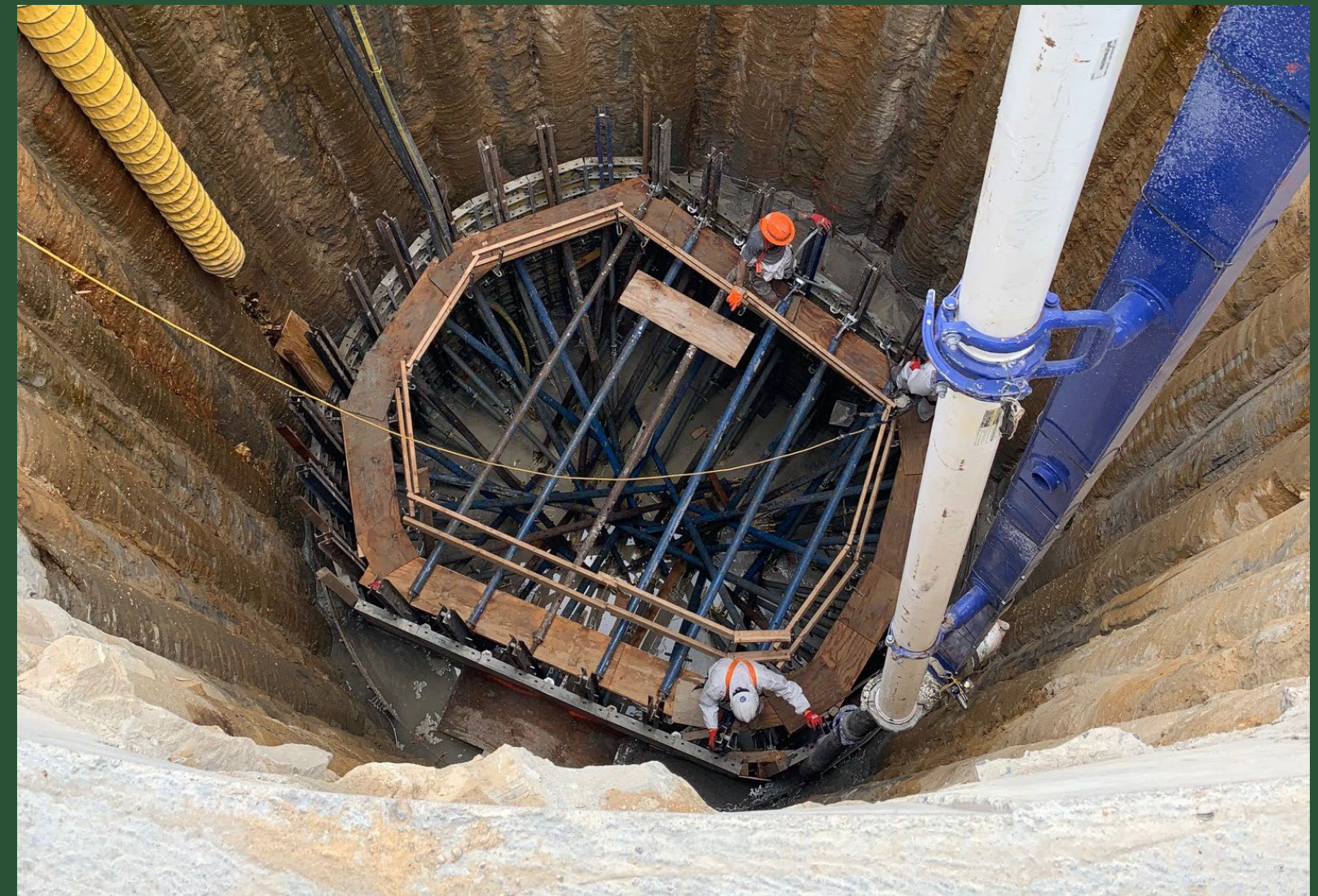
Rebar Installation at CC3 (May 2022)
