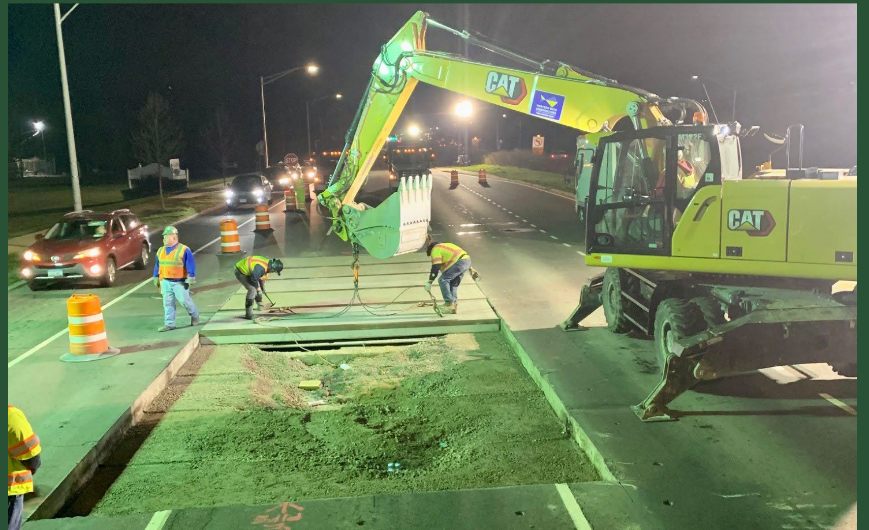
SOE installation at Pit T (April 2022)
