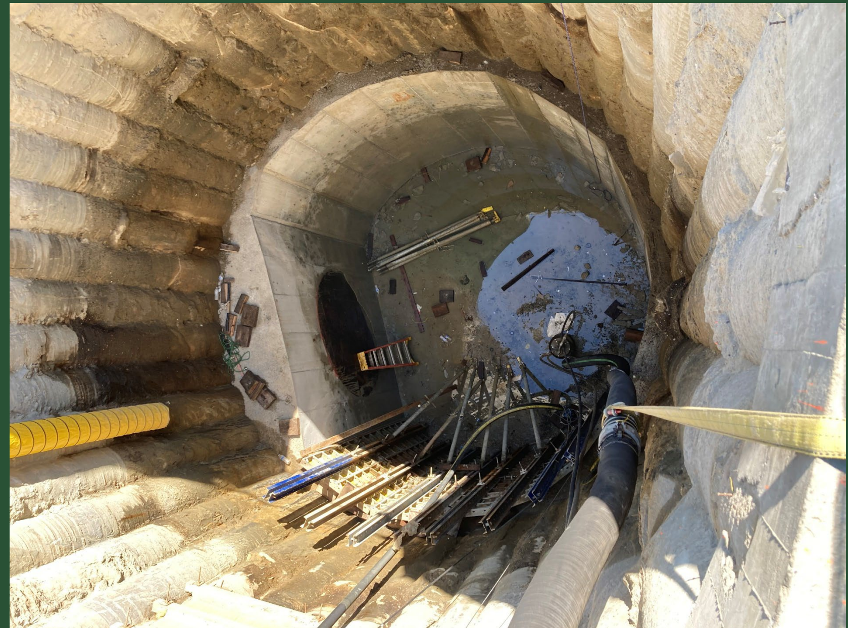
Shaft Construction at CC1 (May 2022)
