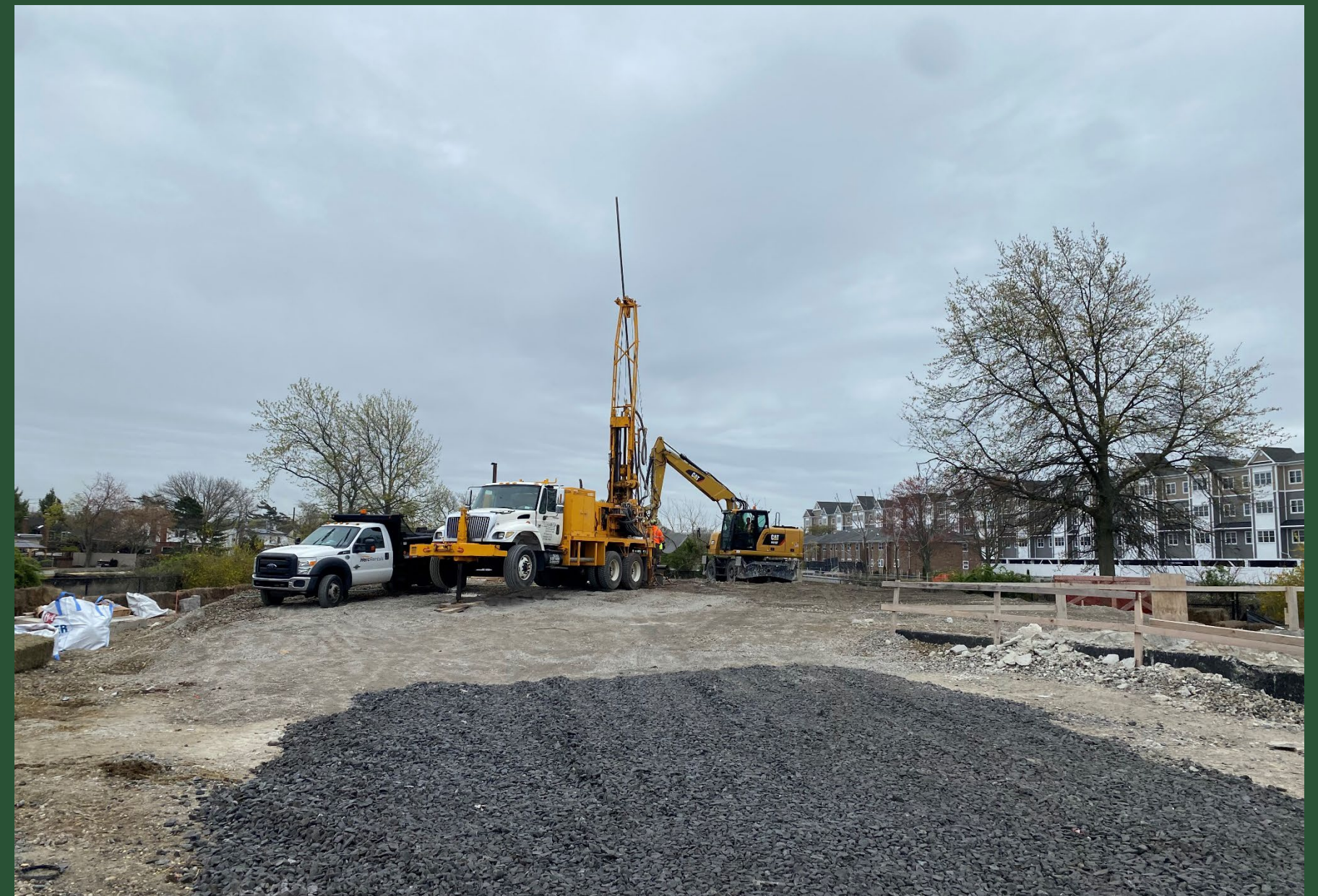
SOE Installation at BP5 (April 2022)
