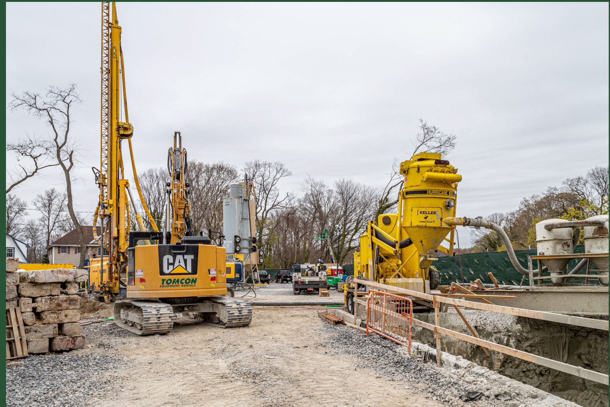
Construction Site at CC5 (April 2022)
