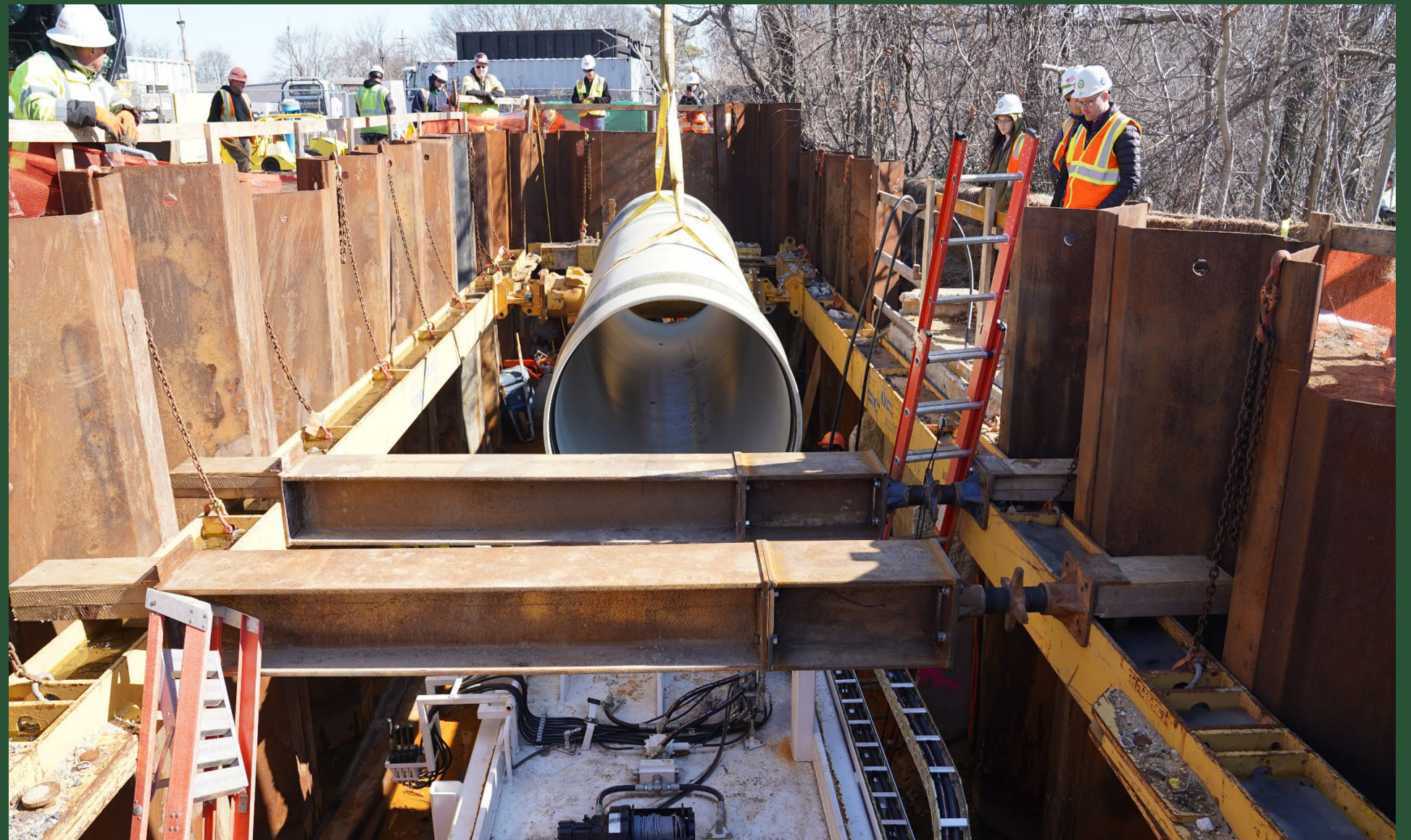
Start of Sliplining at Pit O (March 2022)
