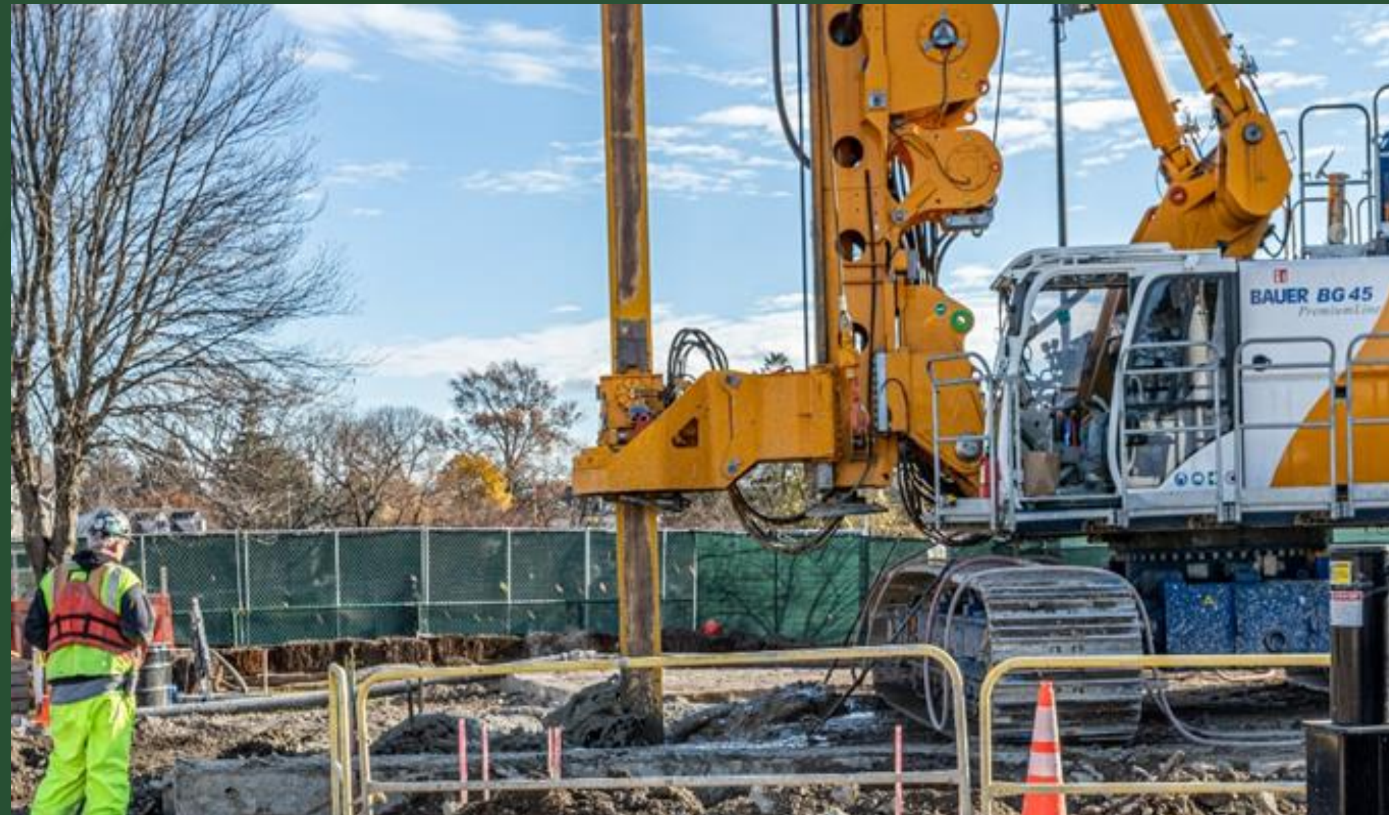
SOE Installation at BP8, December 2021
