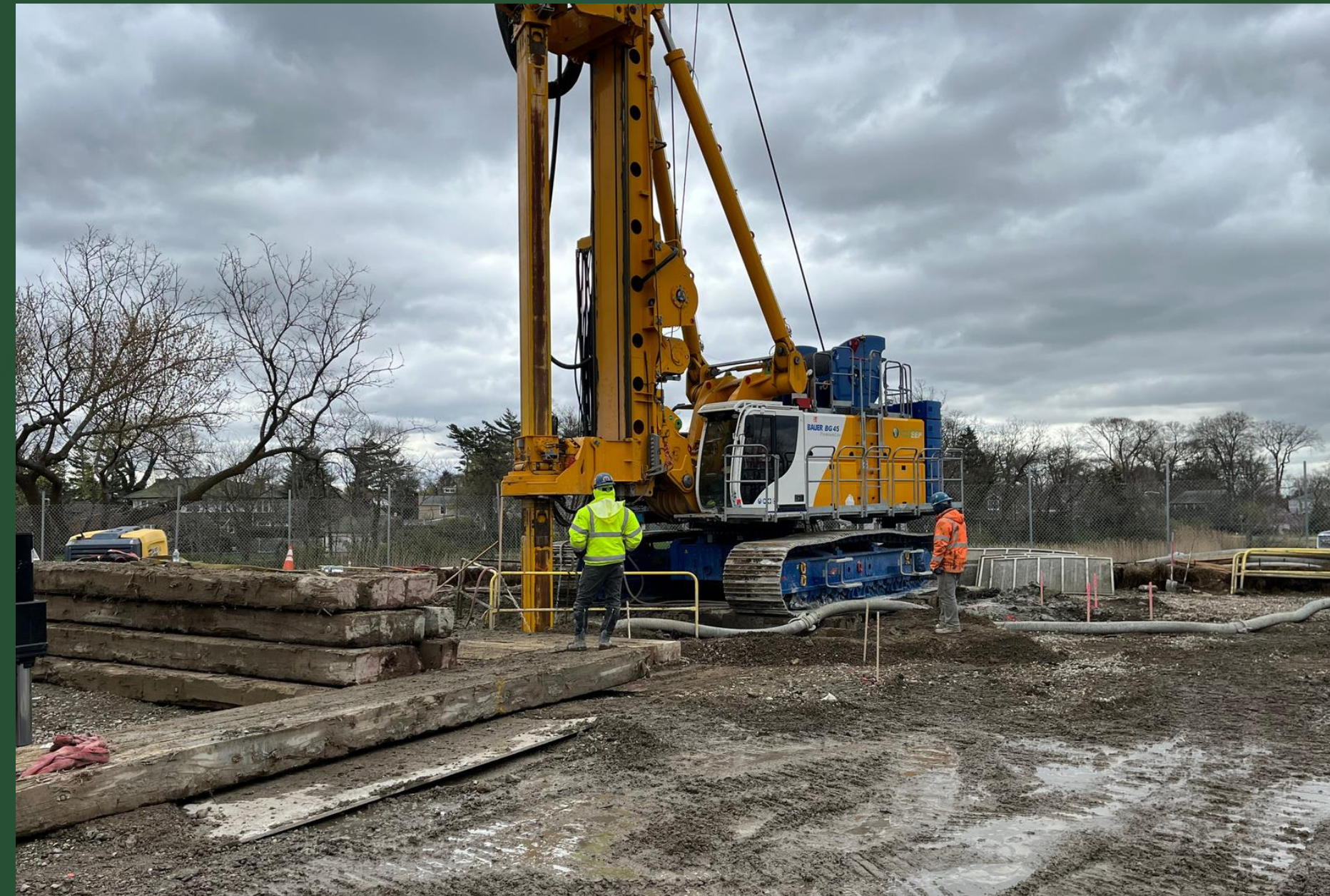
SOE Installation at BP7, April 2022
