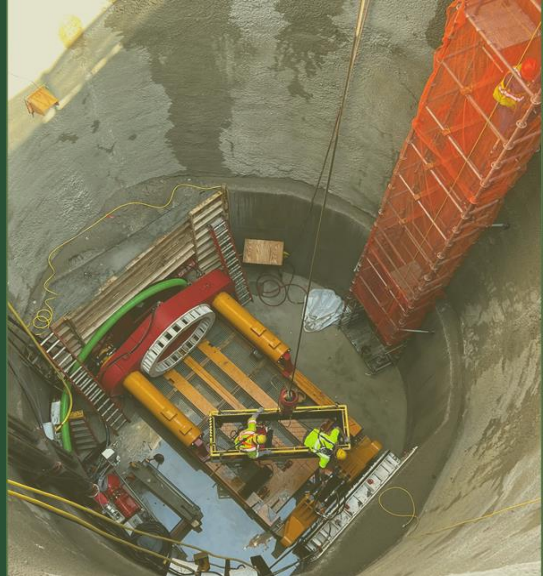
Jacking Station for Microtunnel Boring Machine (MTBM) named MARSH-MELLOW at Bay Park Shaft 2, March 2022
