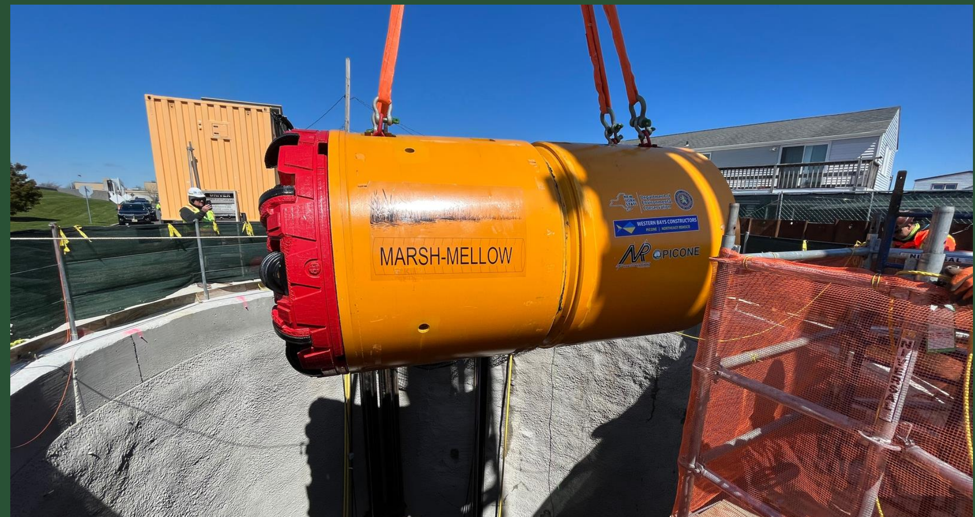
MTBM "MARSH-MELLOW" Lowered into BP2, April 2022
