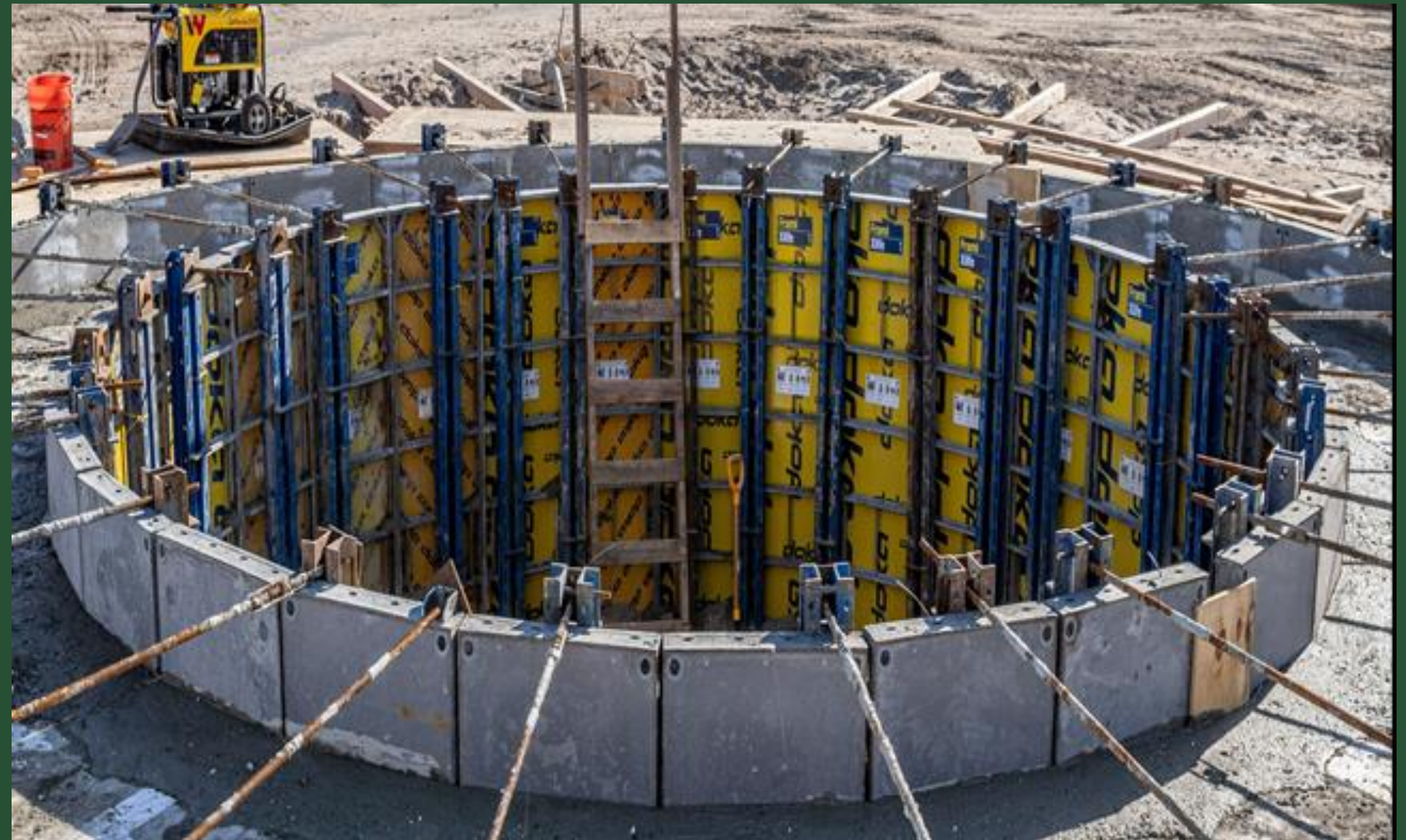
Guide Wall Installation at CC3, January 2022
