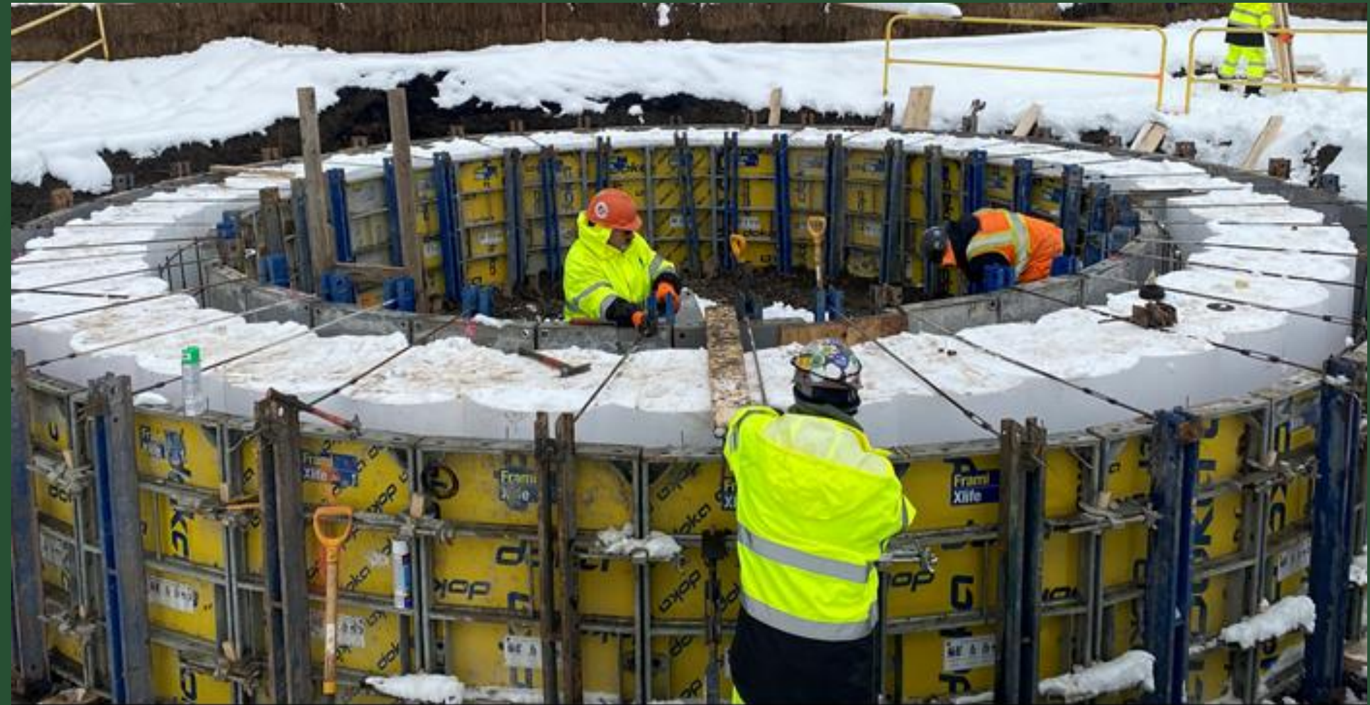
Guide Wall Construction at BP4, January 2022
