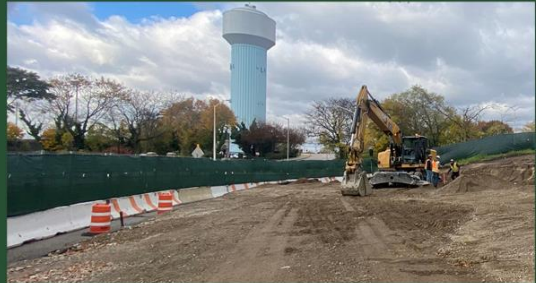
BP9 Site Preparation, January 2022
