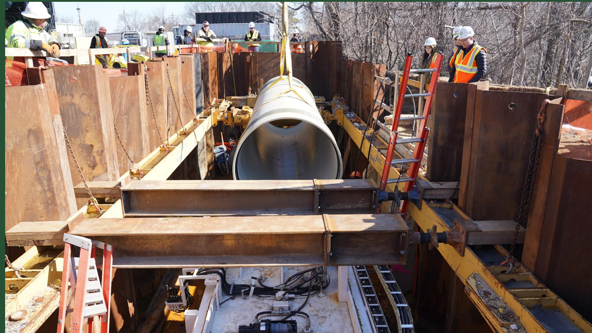
Start of Sliplining at Pit O, March 2022
