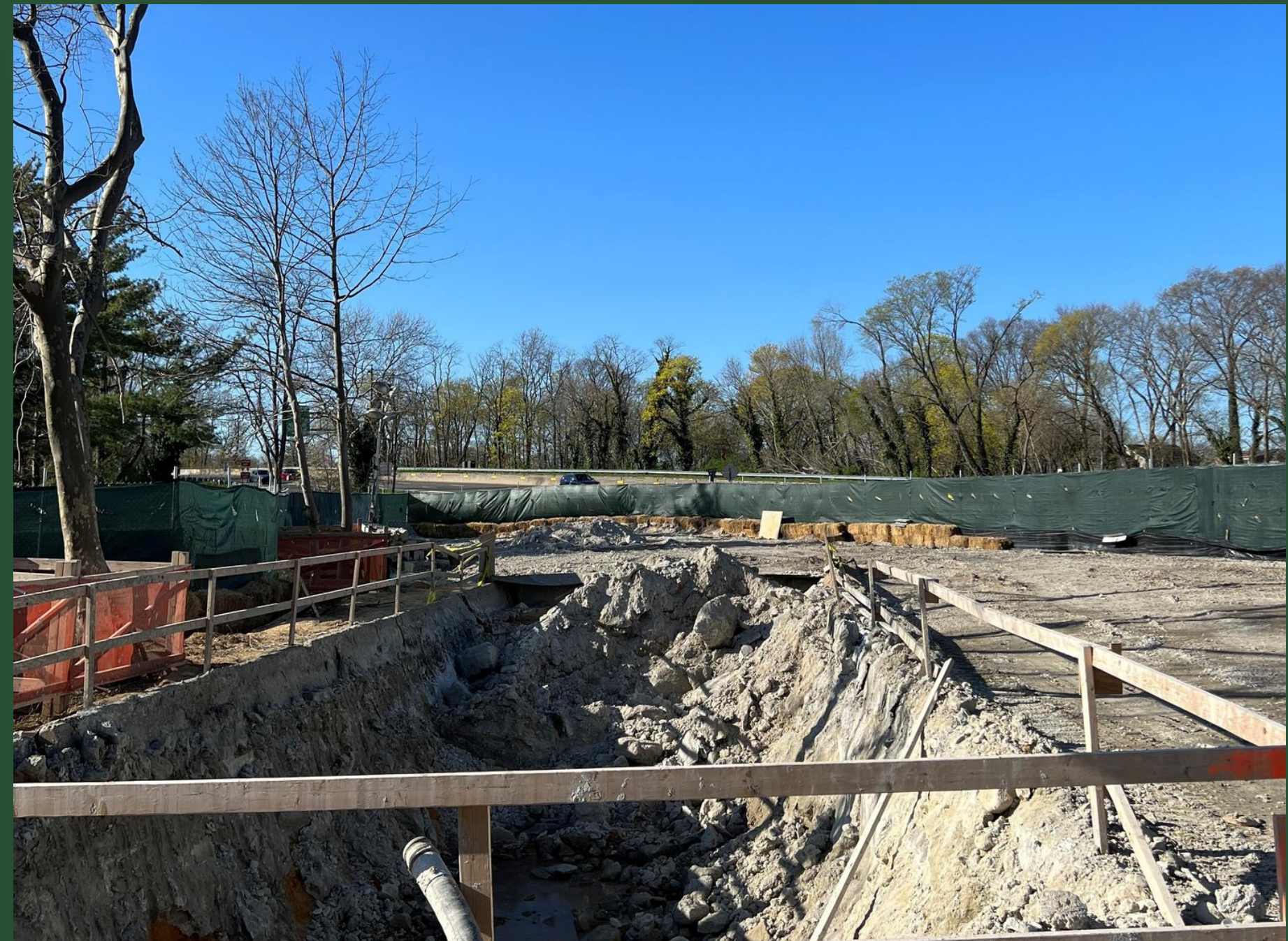
Construction site at CC4, April 2022
