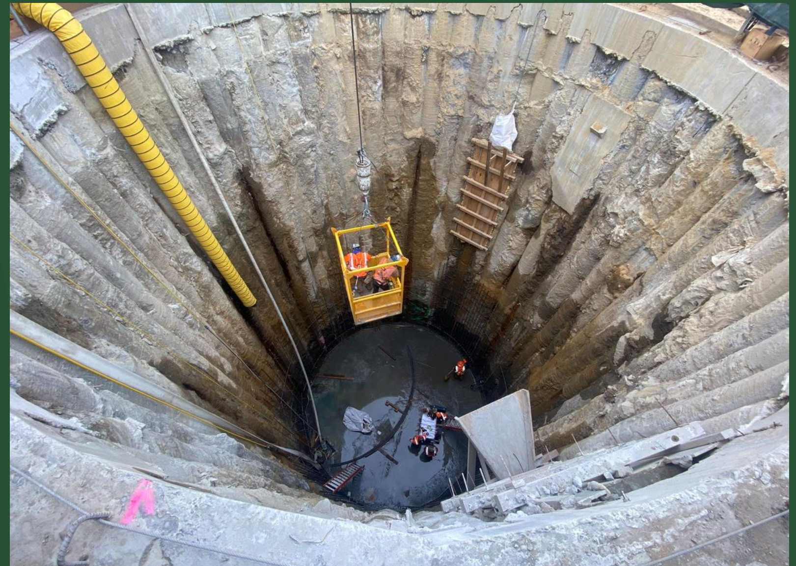
Shaft at CC2, March 2022
