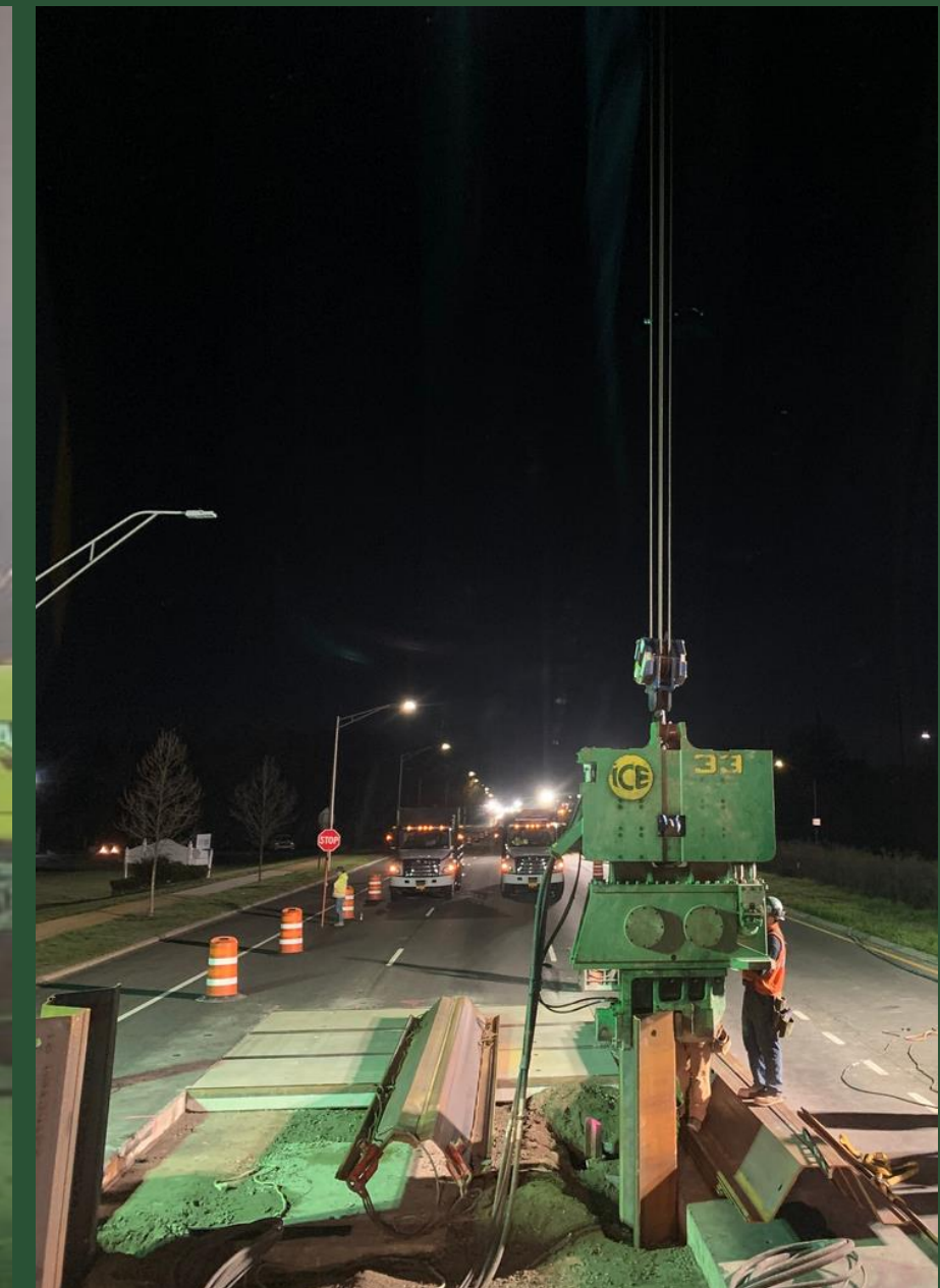
SOE installation at Pit T, April 2022
