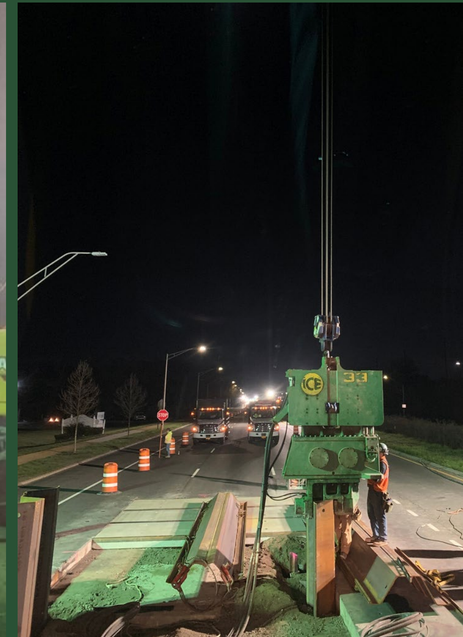
SOE installation at Pit T, April 2022
