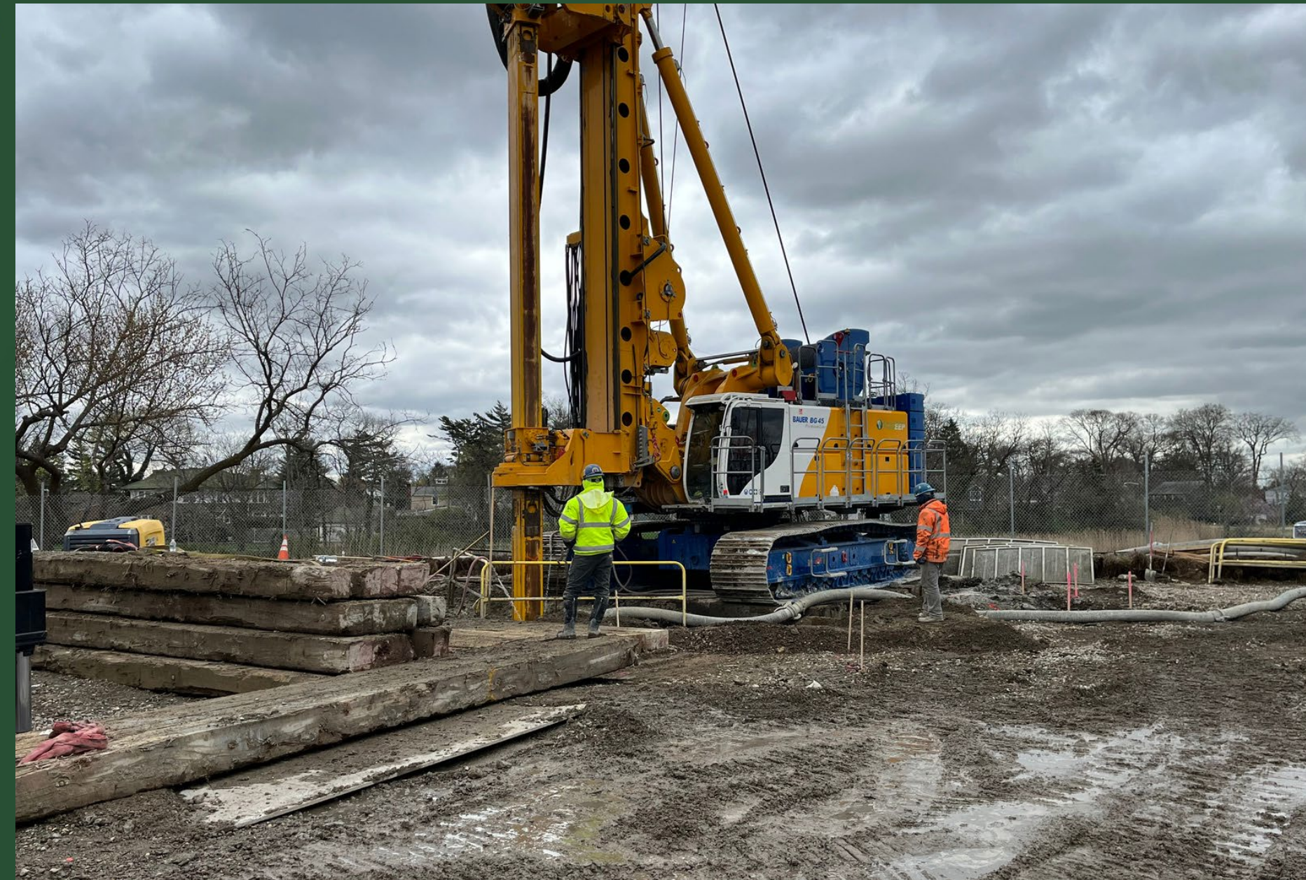
SOE Installation at BP7, April 2022
