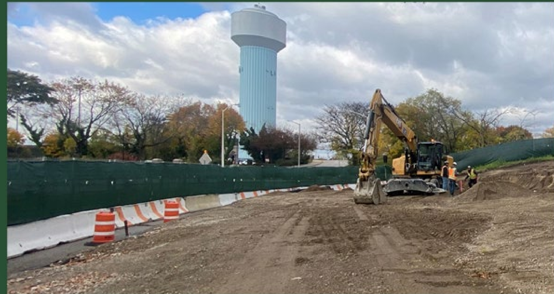
BP9 Site Preparation, January 2022
