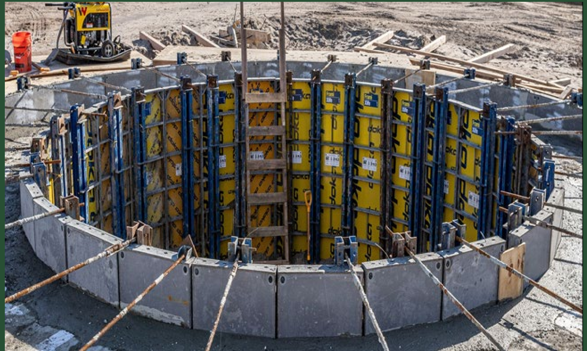
Guide Wall Installation at CC3, January 2022
