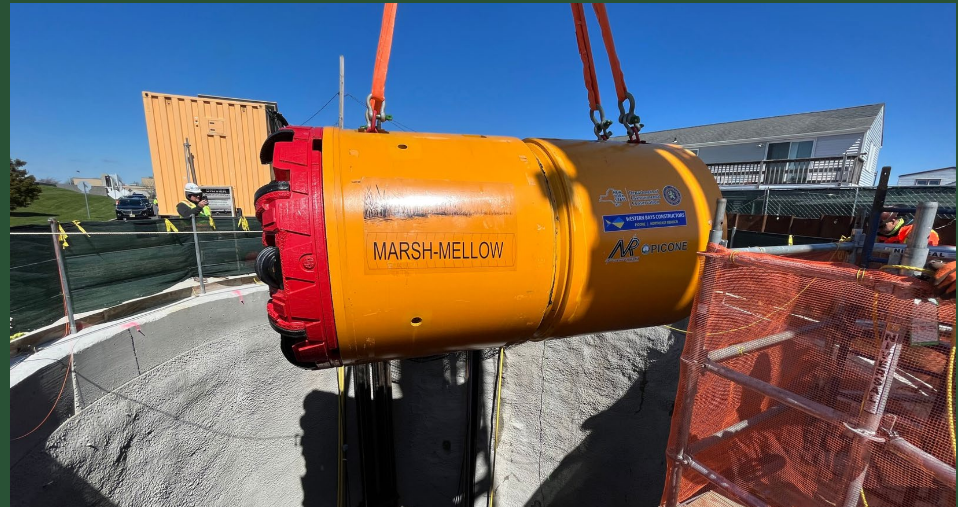
MTBM "MARSH-MELLOW" Lowered into BP2, April 2022
