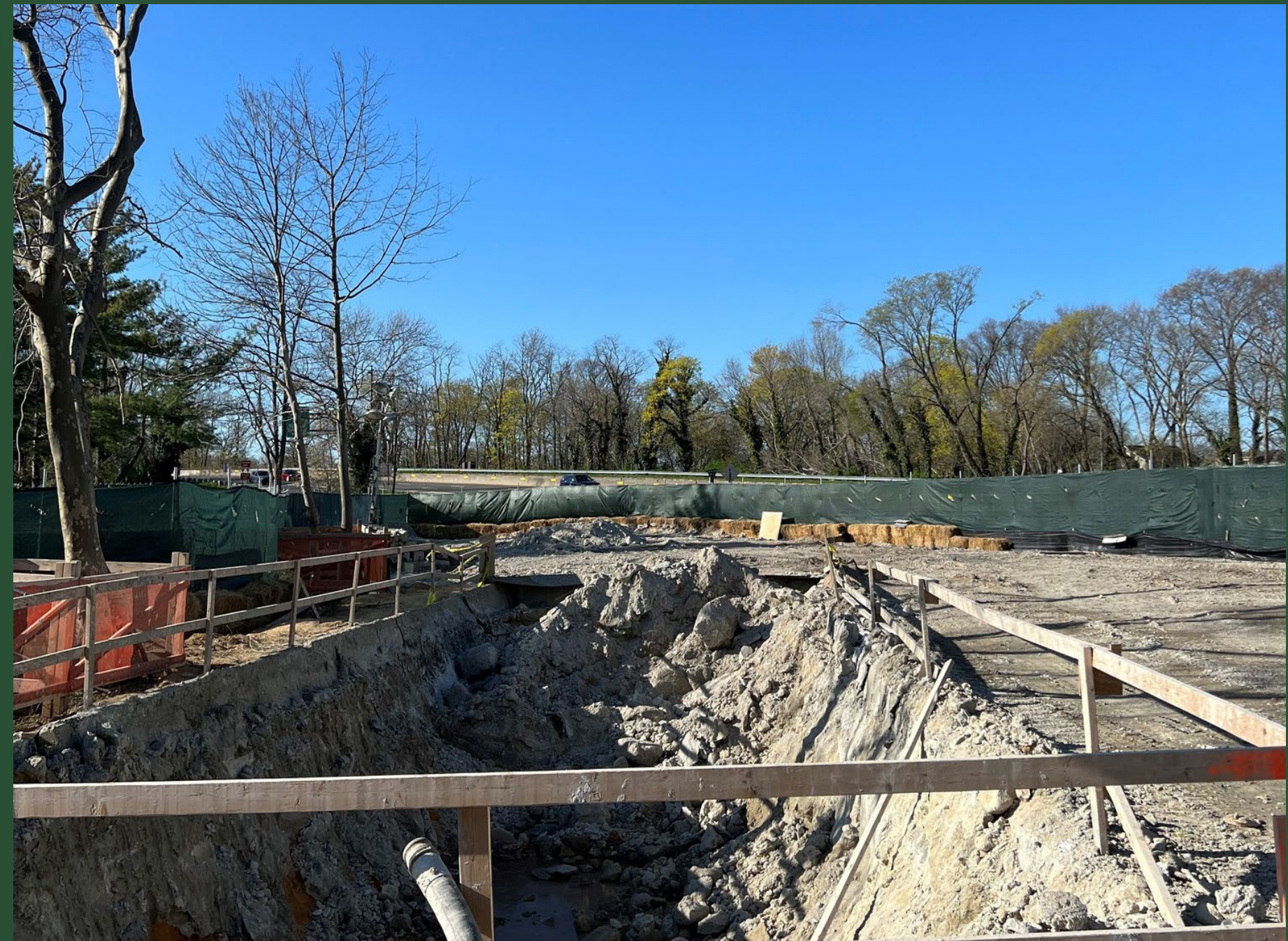
Construction site at CC4, April 2022
