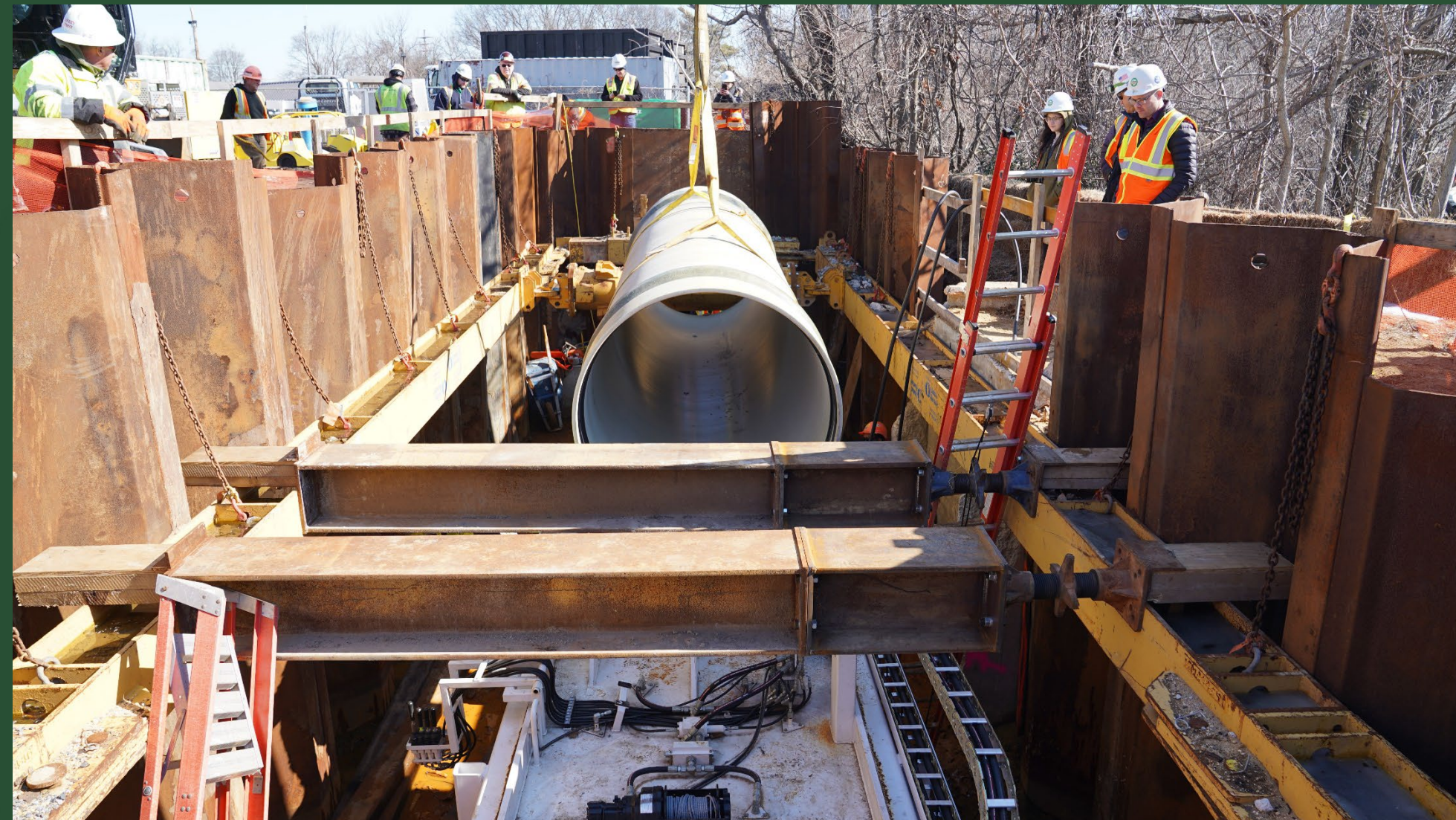
Start of Sliplining at Pit O, March 2022
