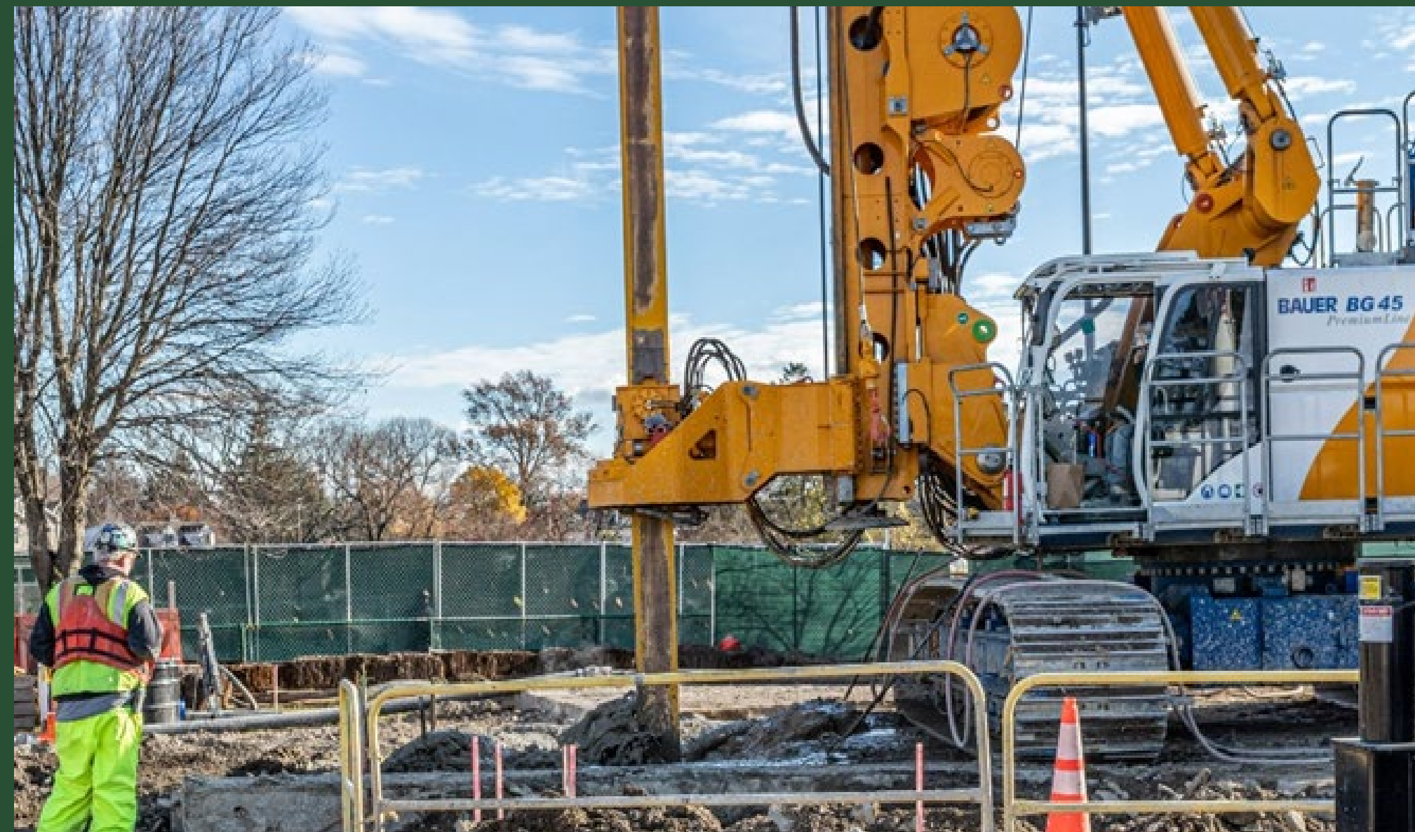
SOE Installation at BP8, December 2021
