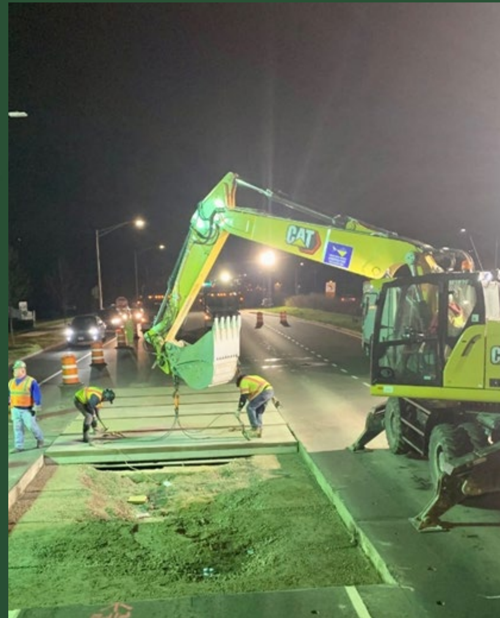
SOE installation at Pit T, April 2022
