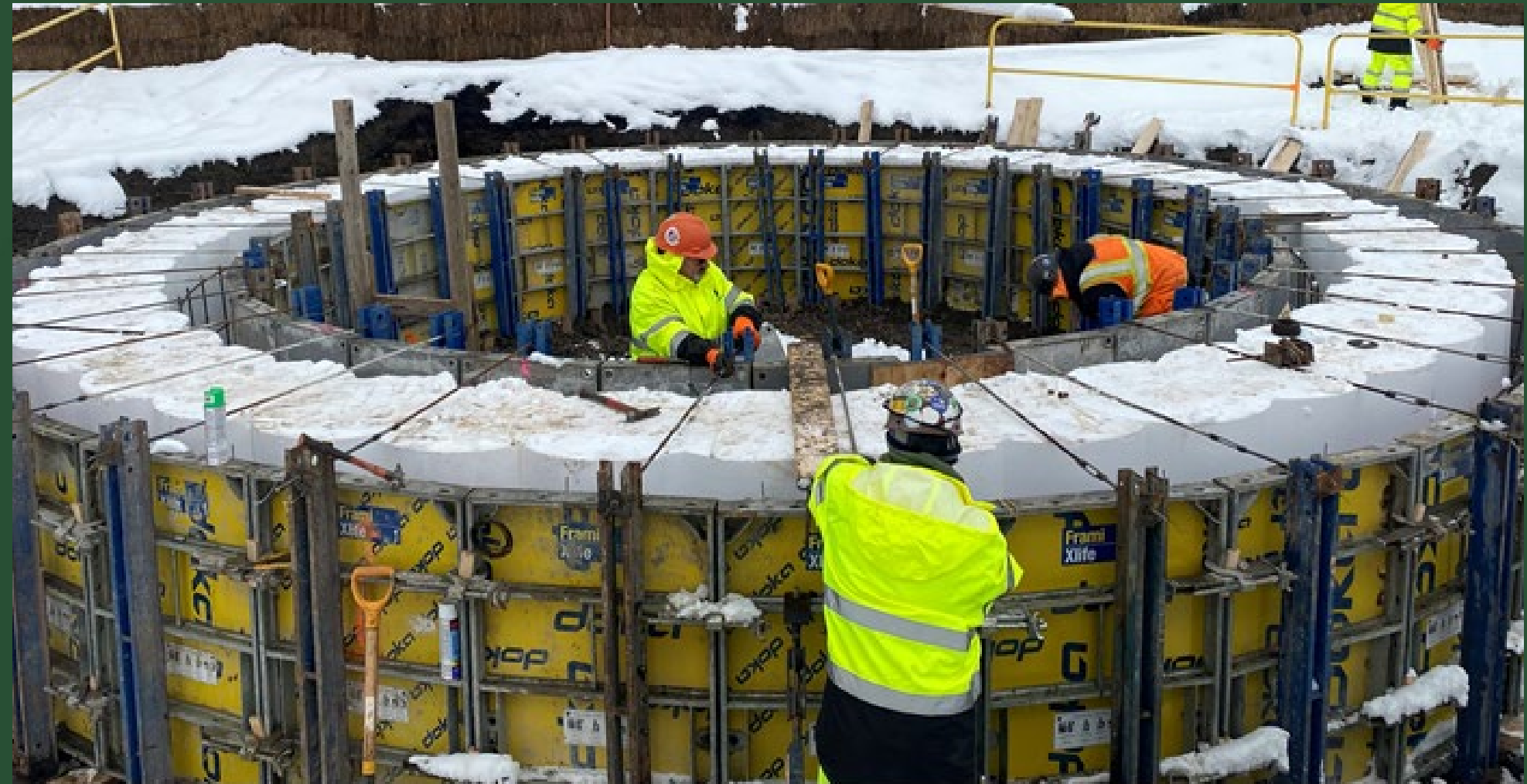
Guide Wall Construction at BP4, January 2022
