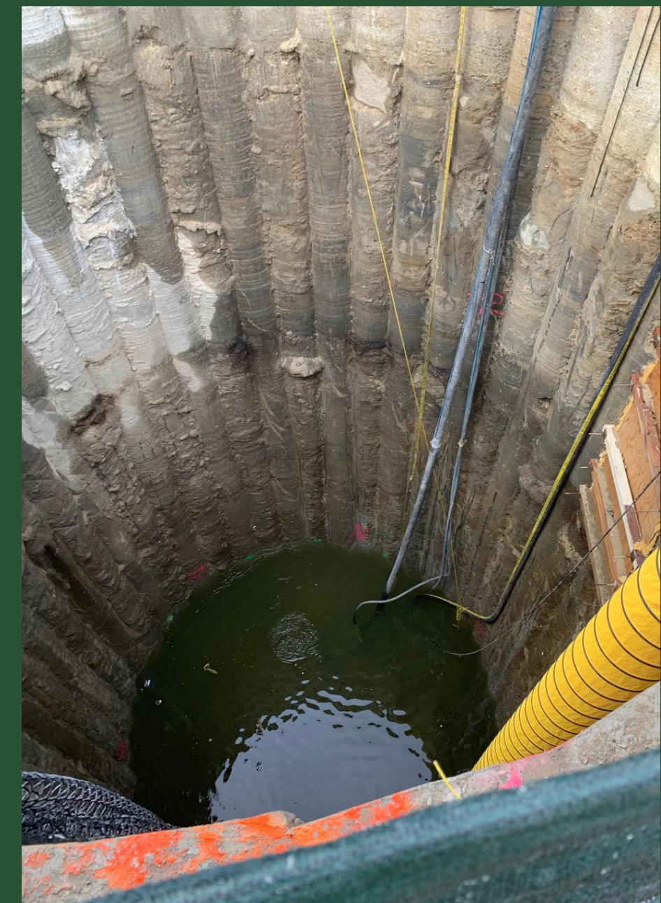
Shaft excavation at CC1, April 2022
