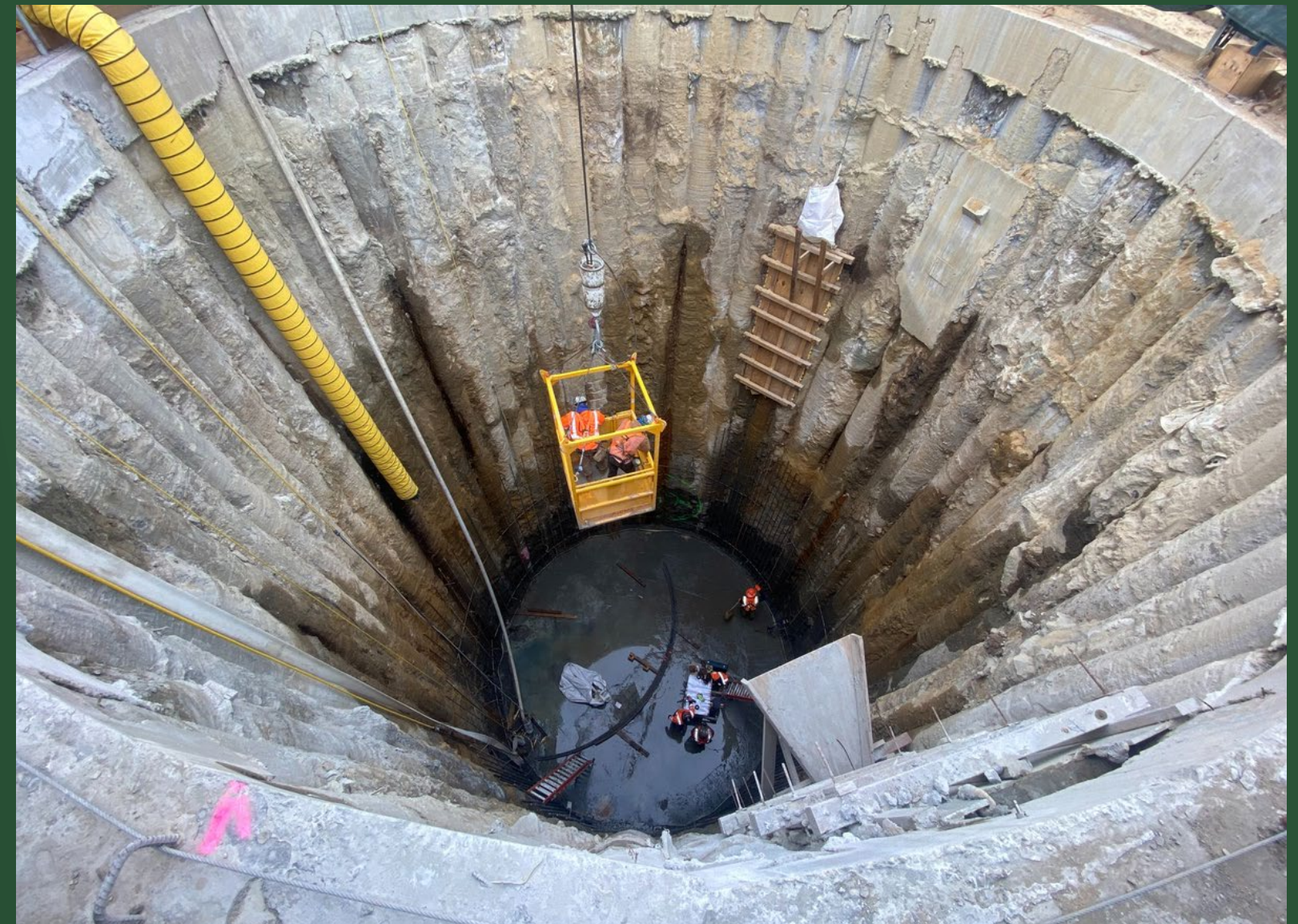
Shaft at CC2, March 2022
