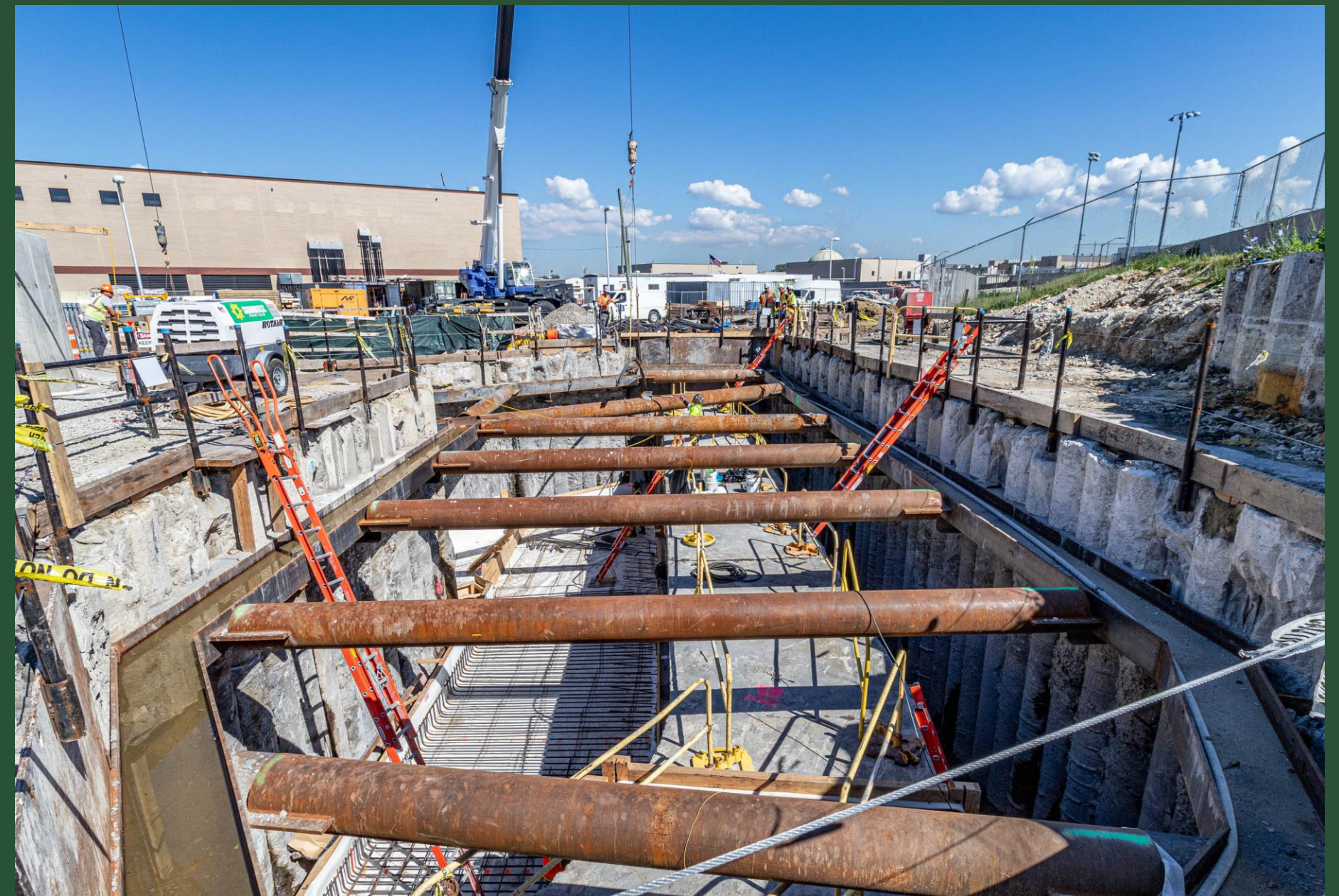
Diversion Structure at BP1 (June 2022)
