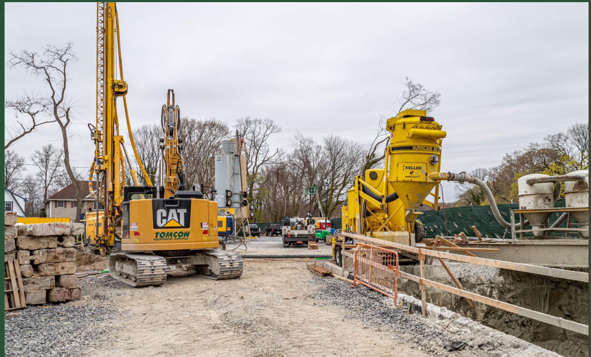
Construction Site at CC5 (April 2022)
