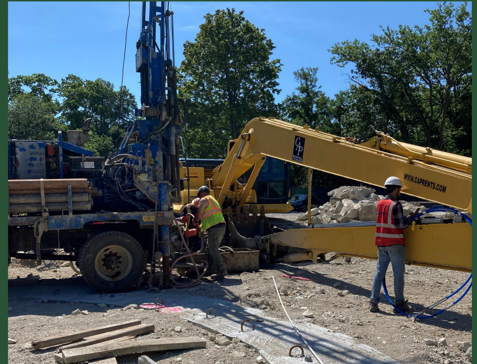
Core Drilling at CC4 (June 2022)
