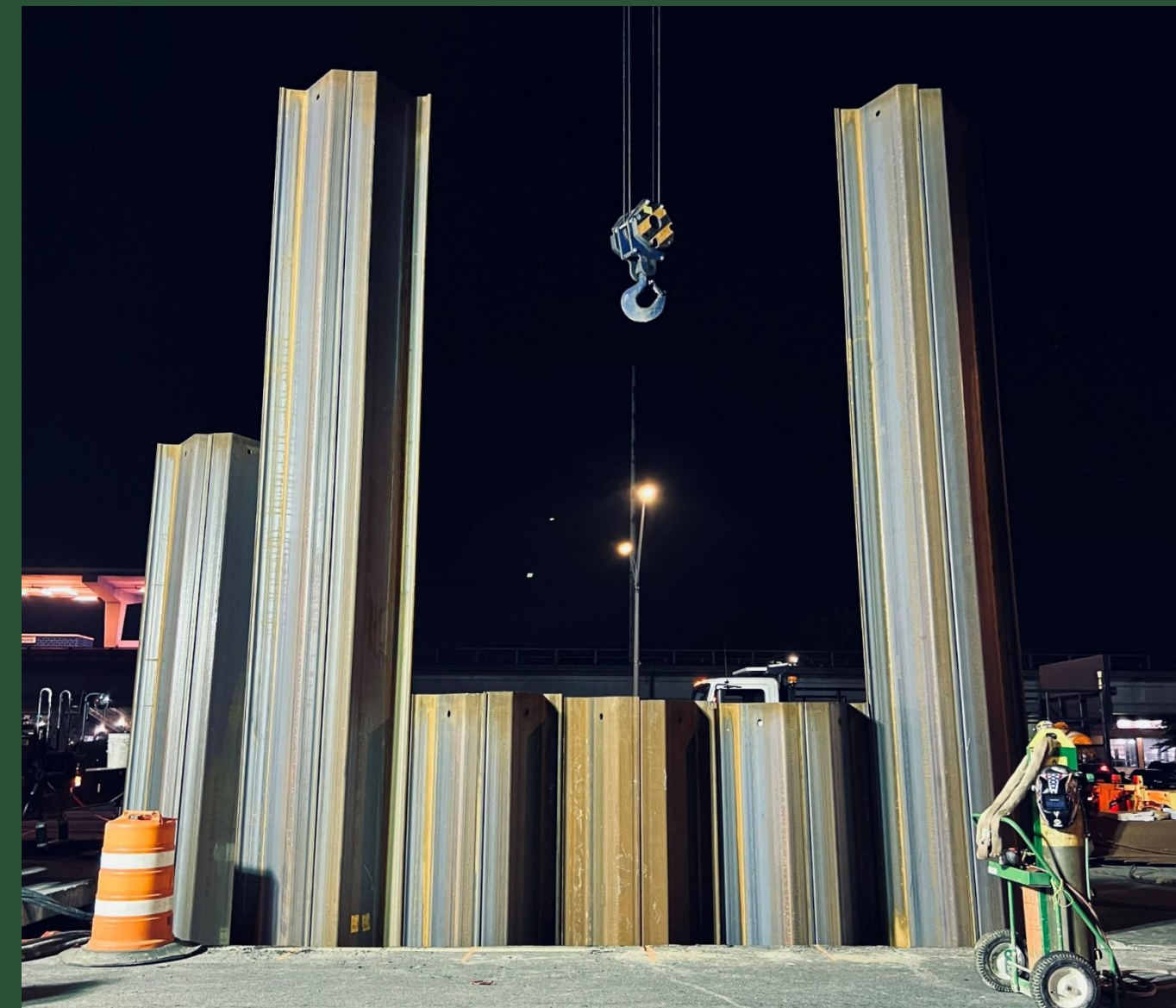
SOE installation at Pit V (June 2022)
