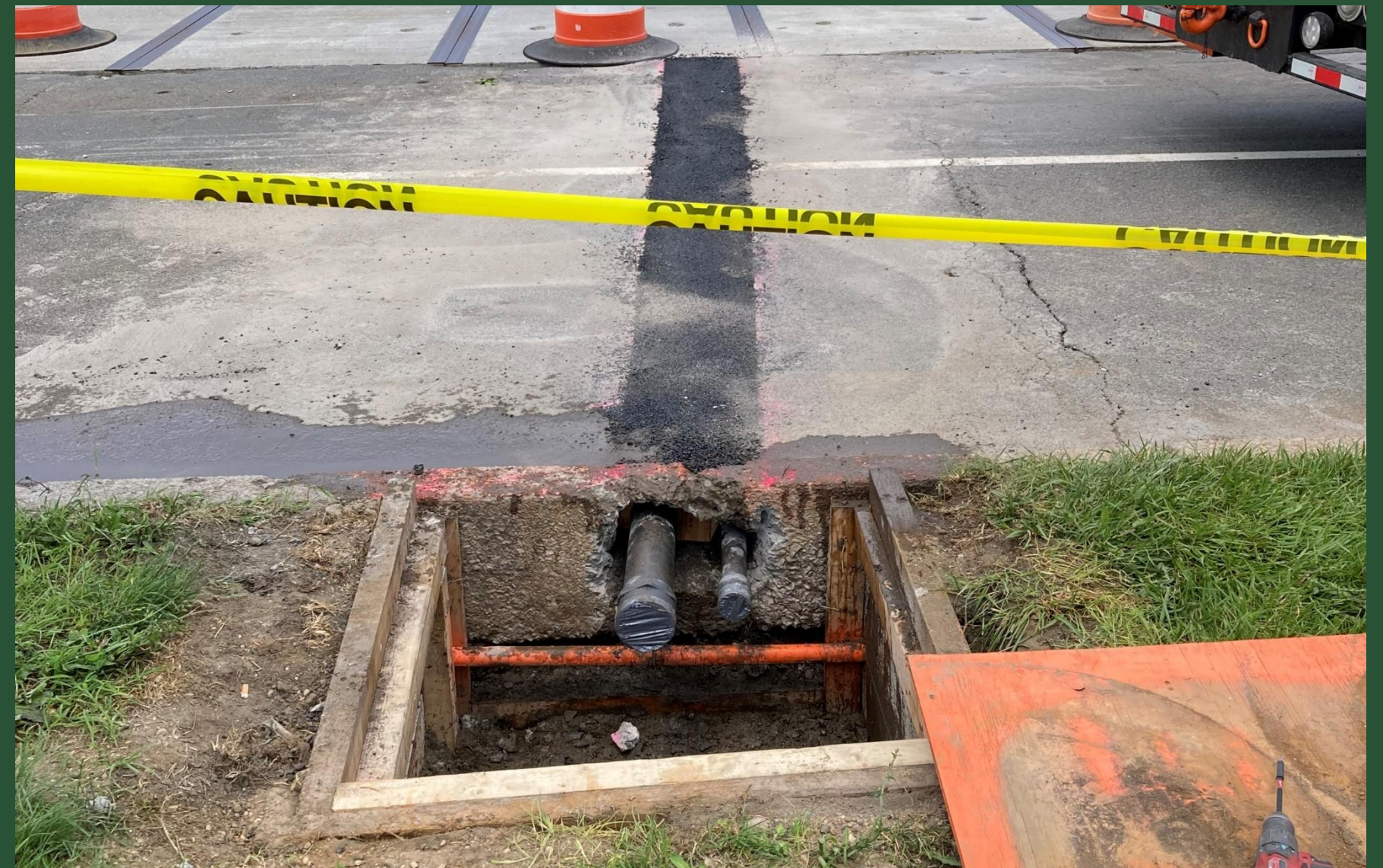
Pipe Installation at Pit S (June 2022)
