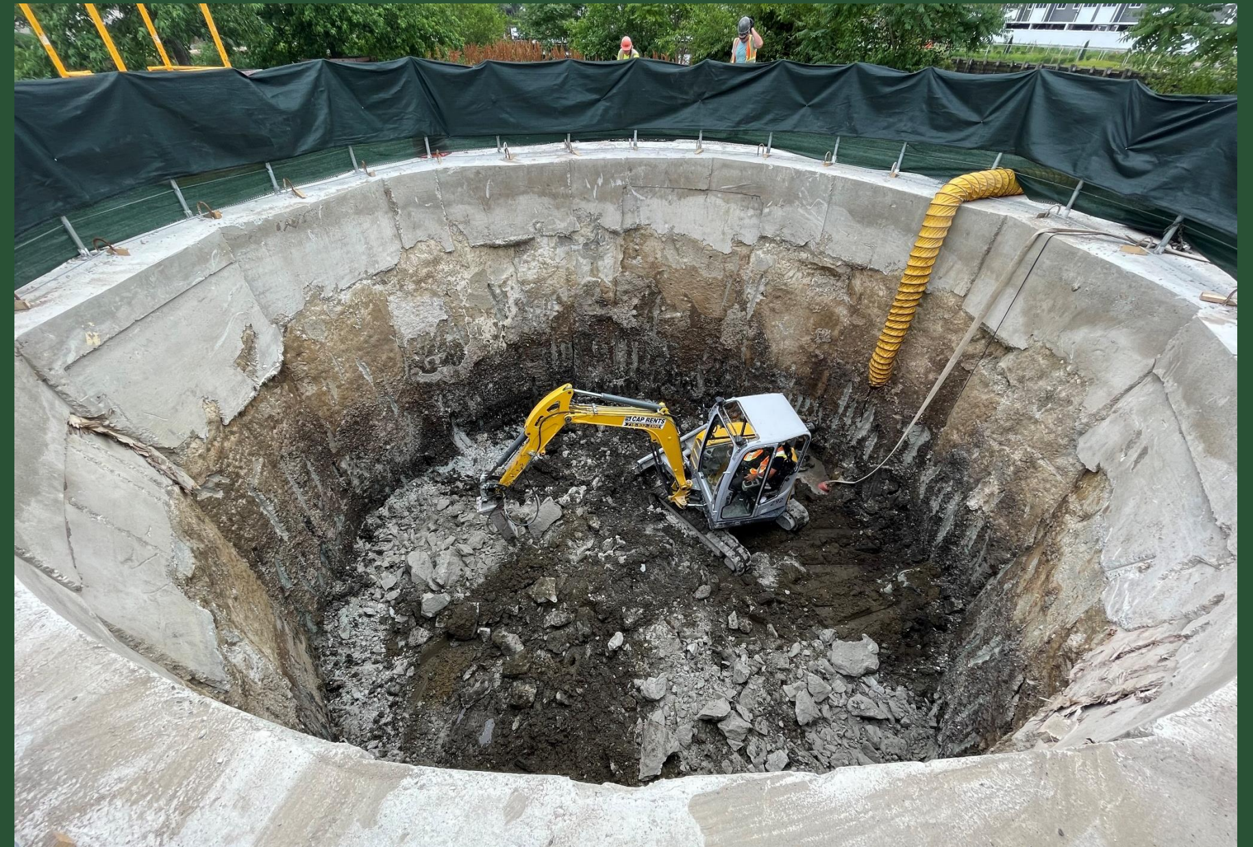
Excavation at BP5 (June 2022)
