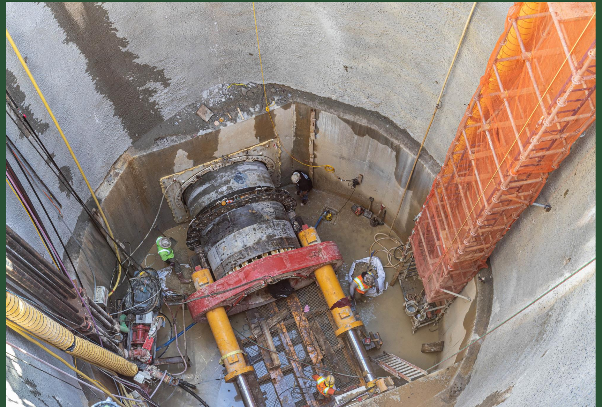
Microtunnel Operations at BP2 (June 2022)
