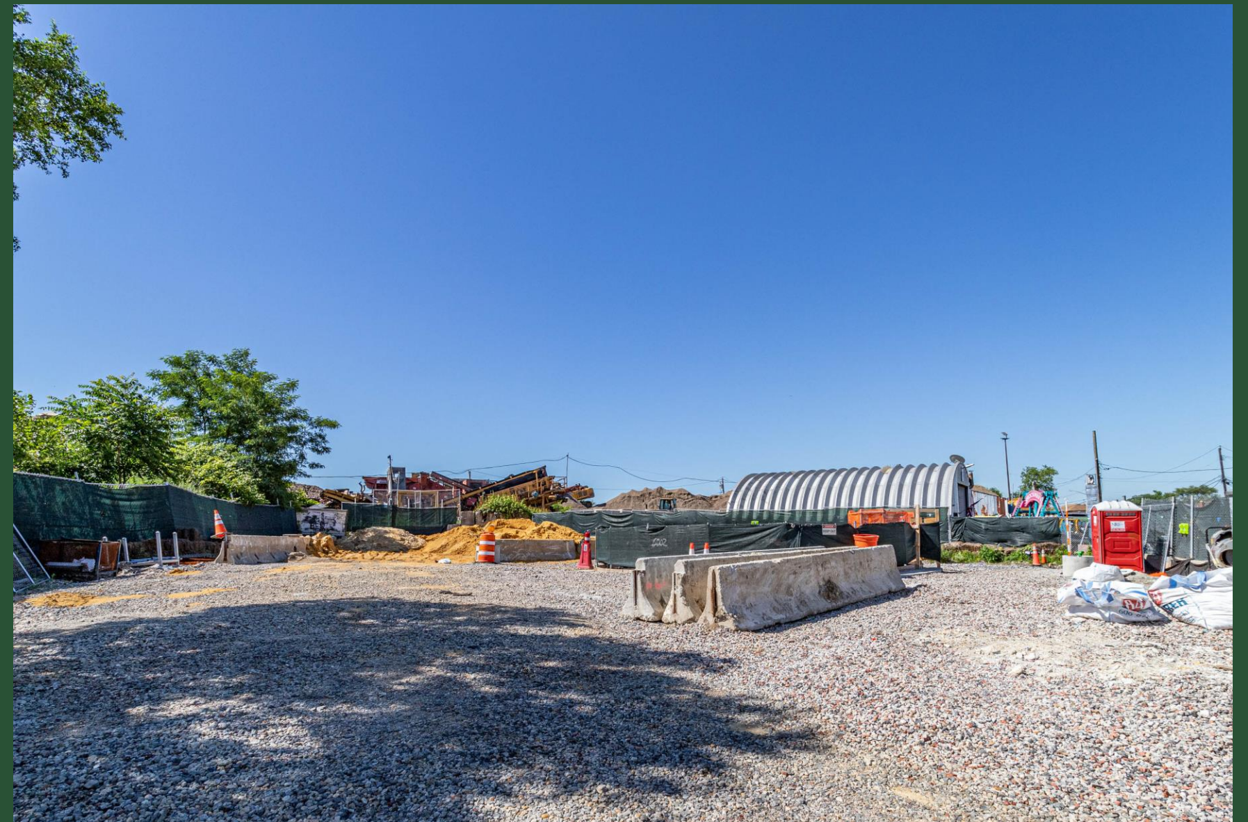
Construction Site at BP3 (June 2022)
