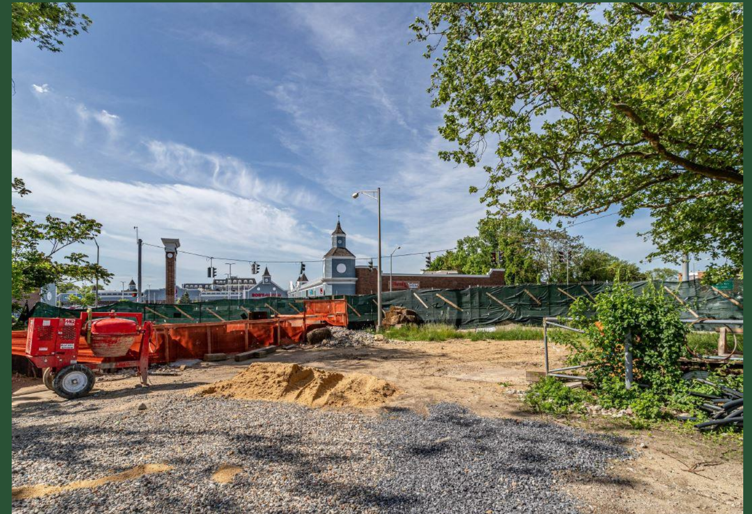
Pit O Construction Site (May 2022)
