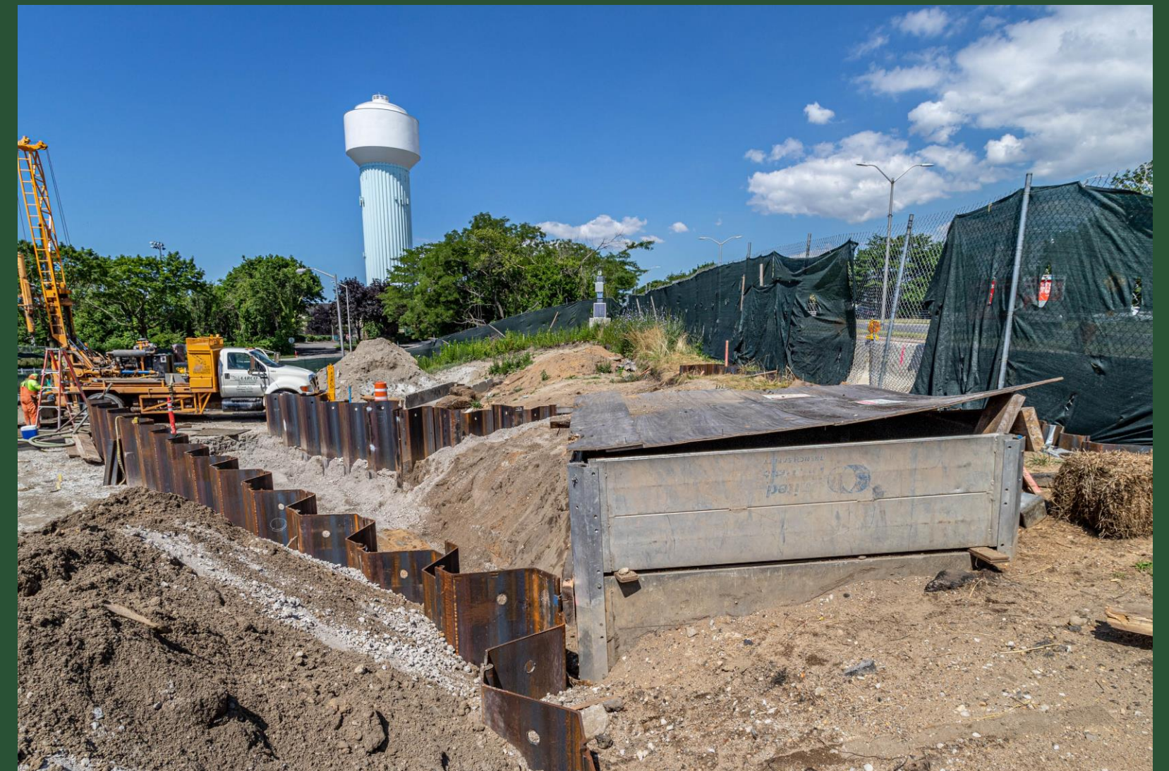
Sheet Installation at Pit A (June 2022)
