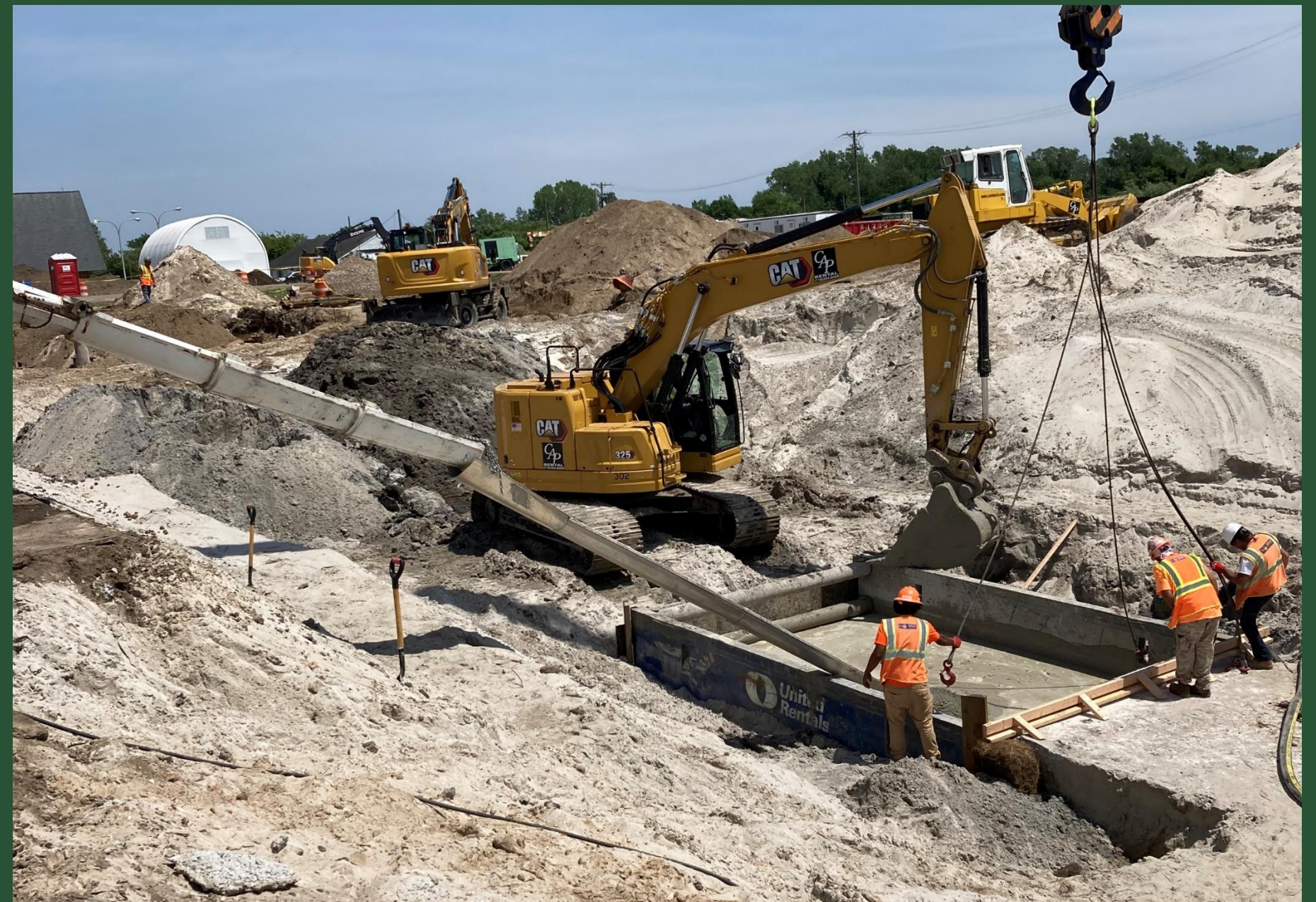
Shaft Construction at CC1 (May 2022)
