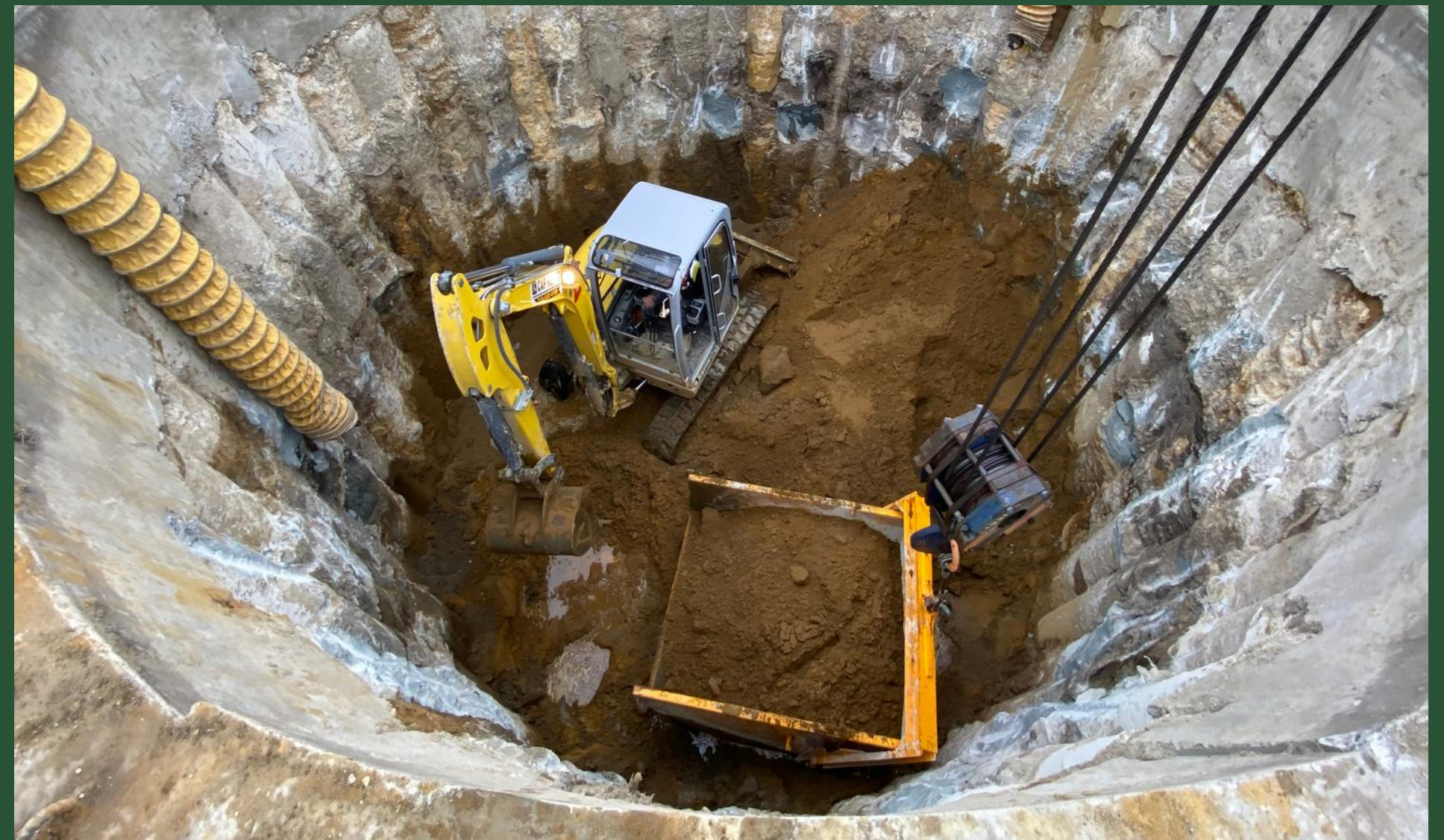
Shaft Excavation at BP4 (April 2022)
