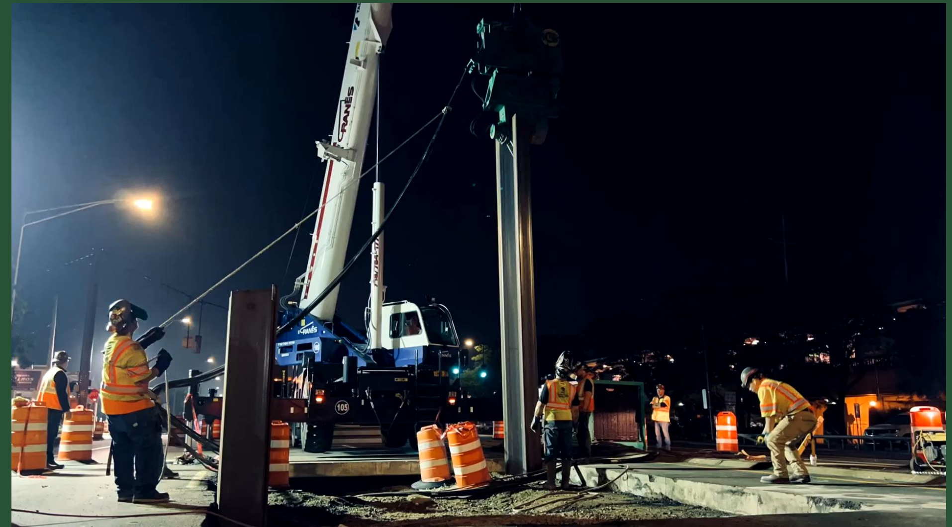
SOE installation at Pit V (June 2022)
