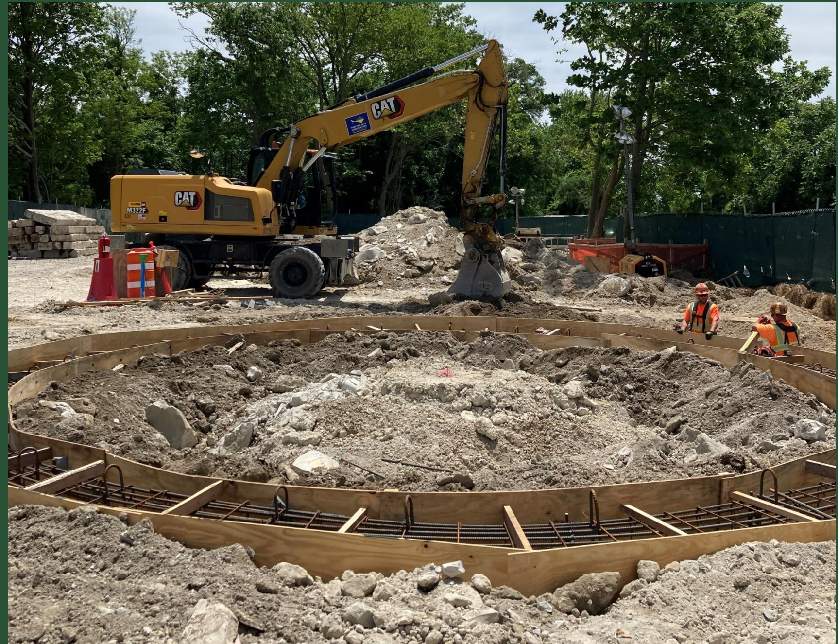
Ring Beam Installation at CC4 (June 2022)
