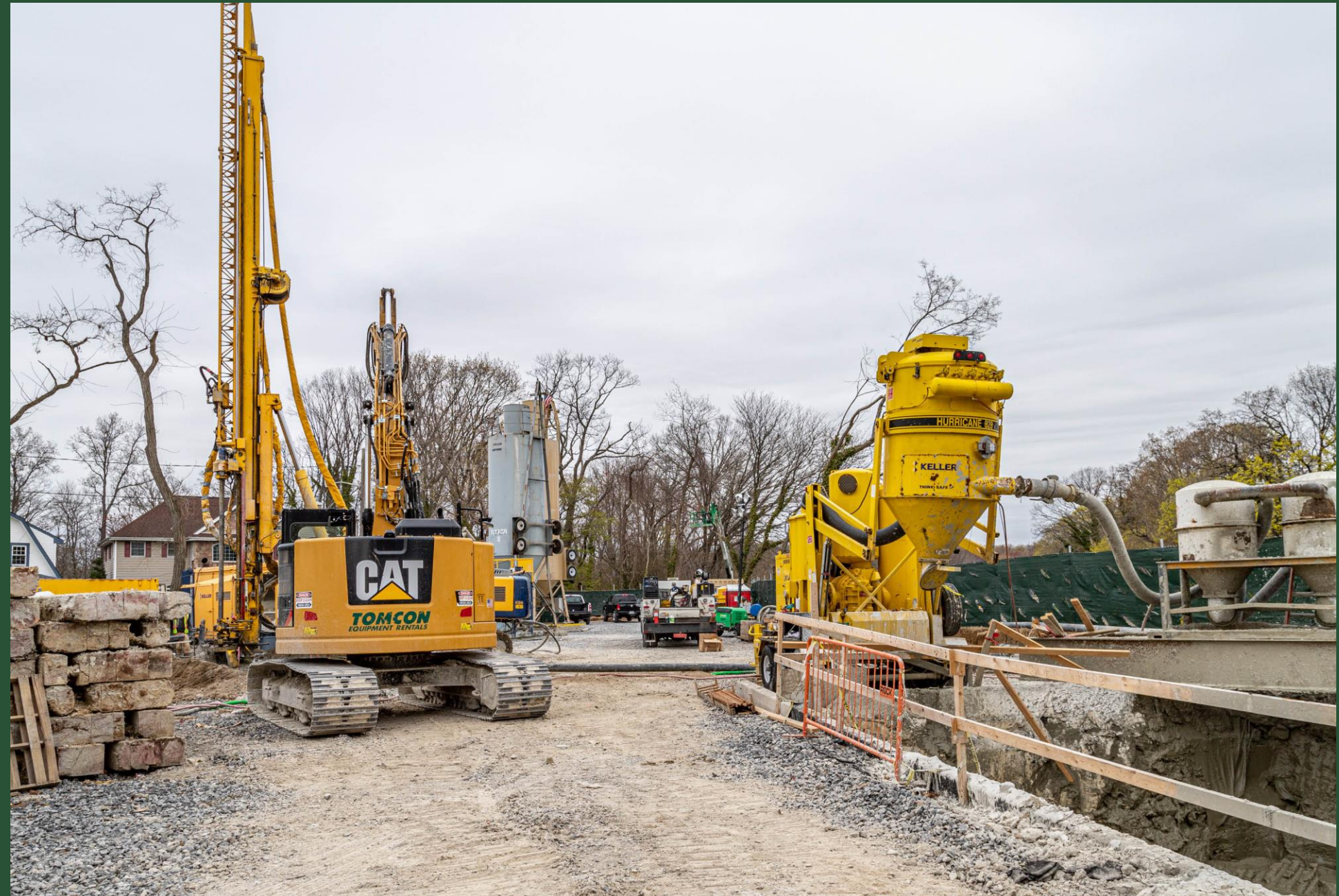
Construction Site at CC5 (April 2022)
