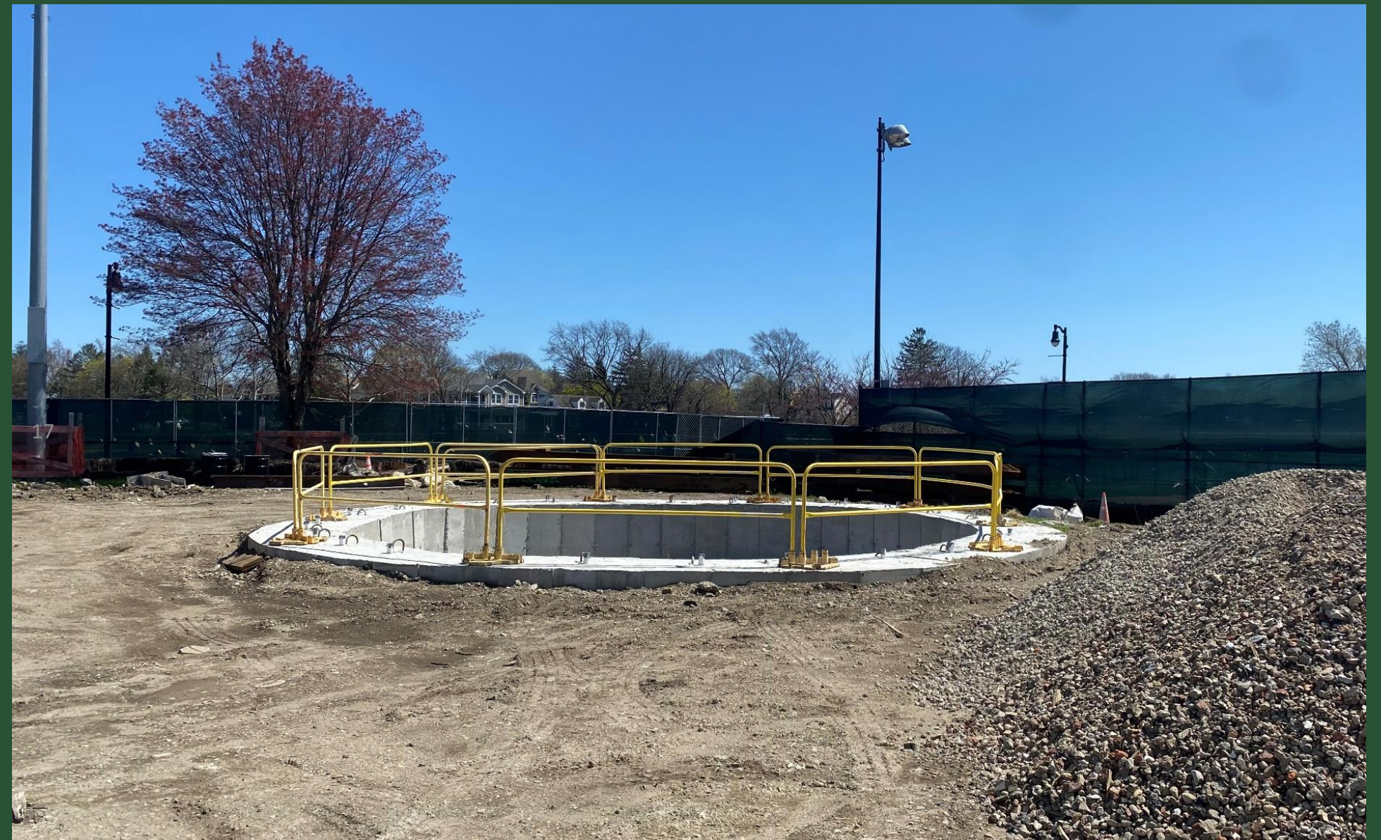
Shaft Site at BP8 (April 2022)
