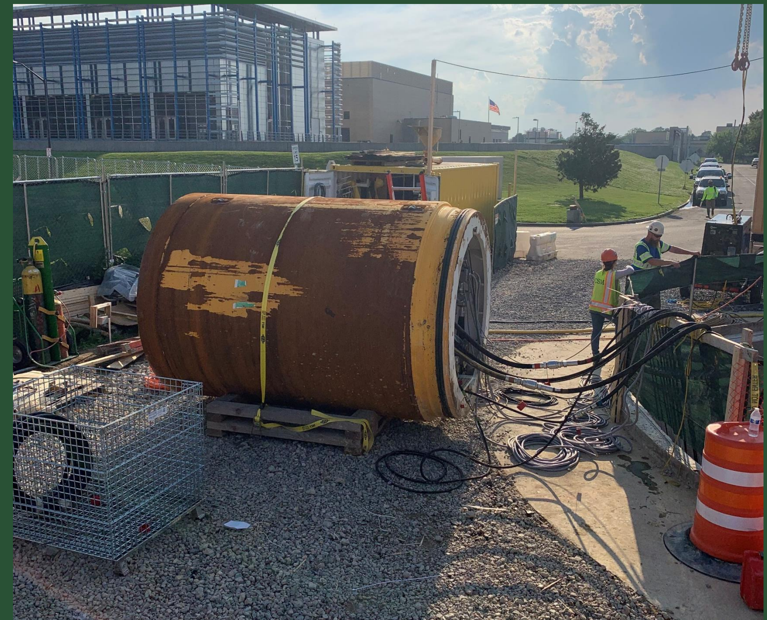
Microtunnel Preparations at BP2 (June 2022)
