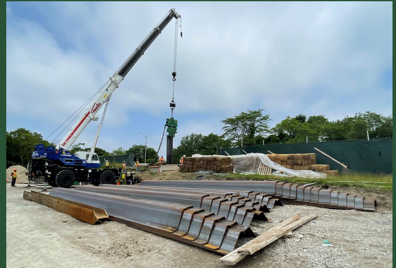
Sheet Installation at Pit A (June 2022)
