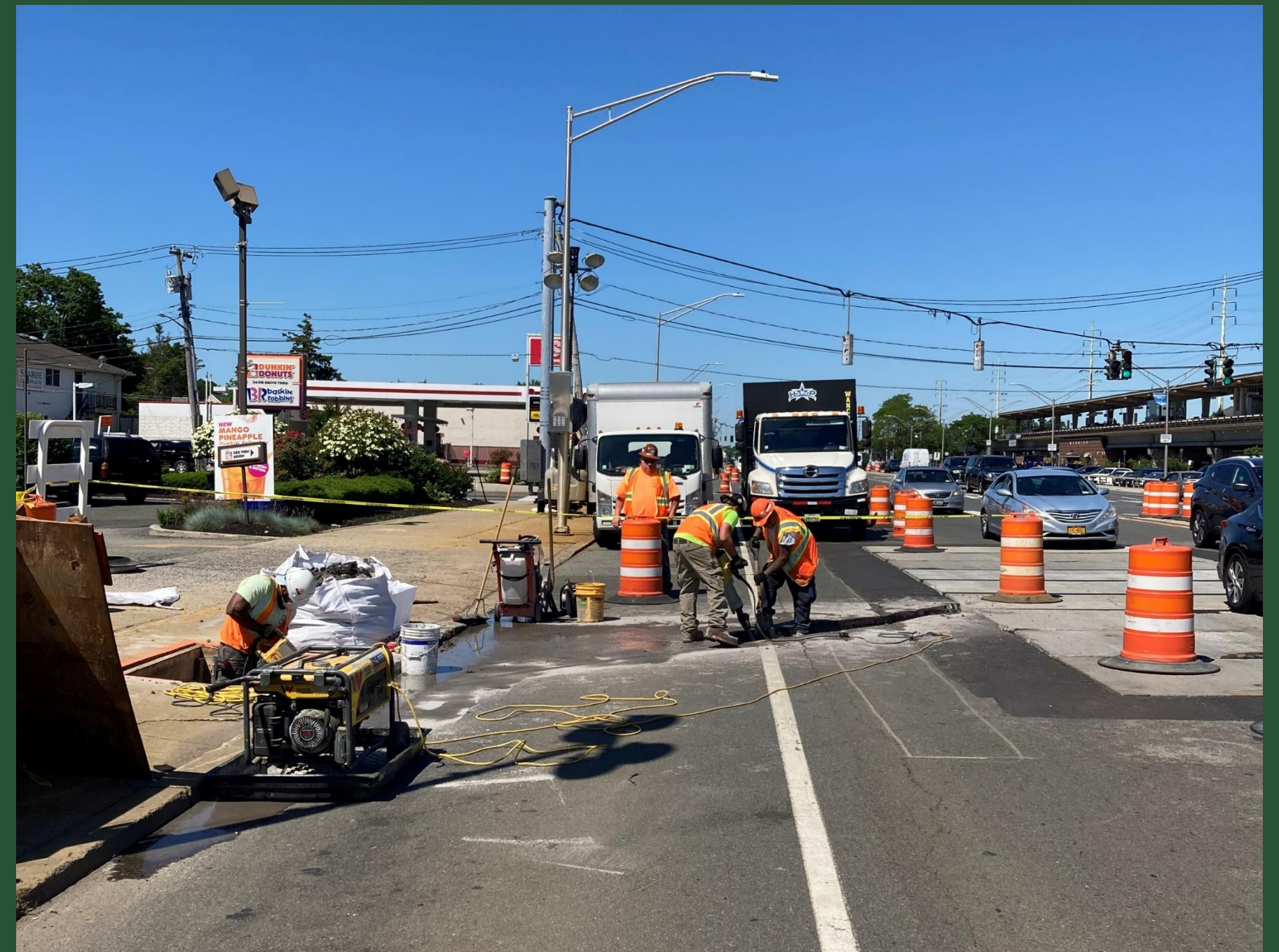
Pipe Installation at Pit S (June 2022)
