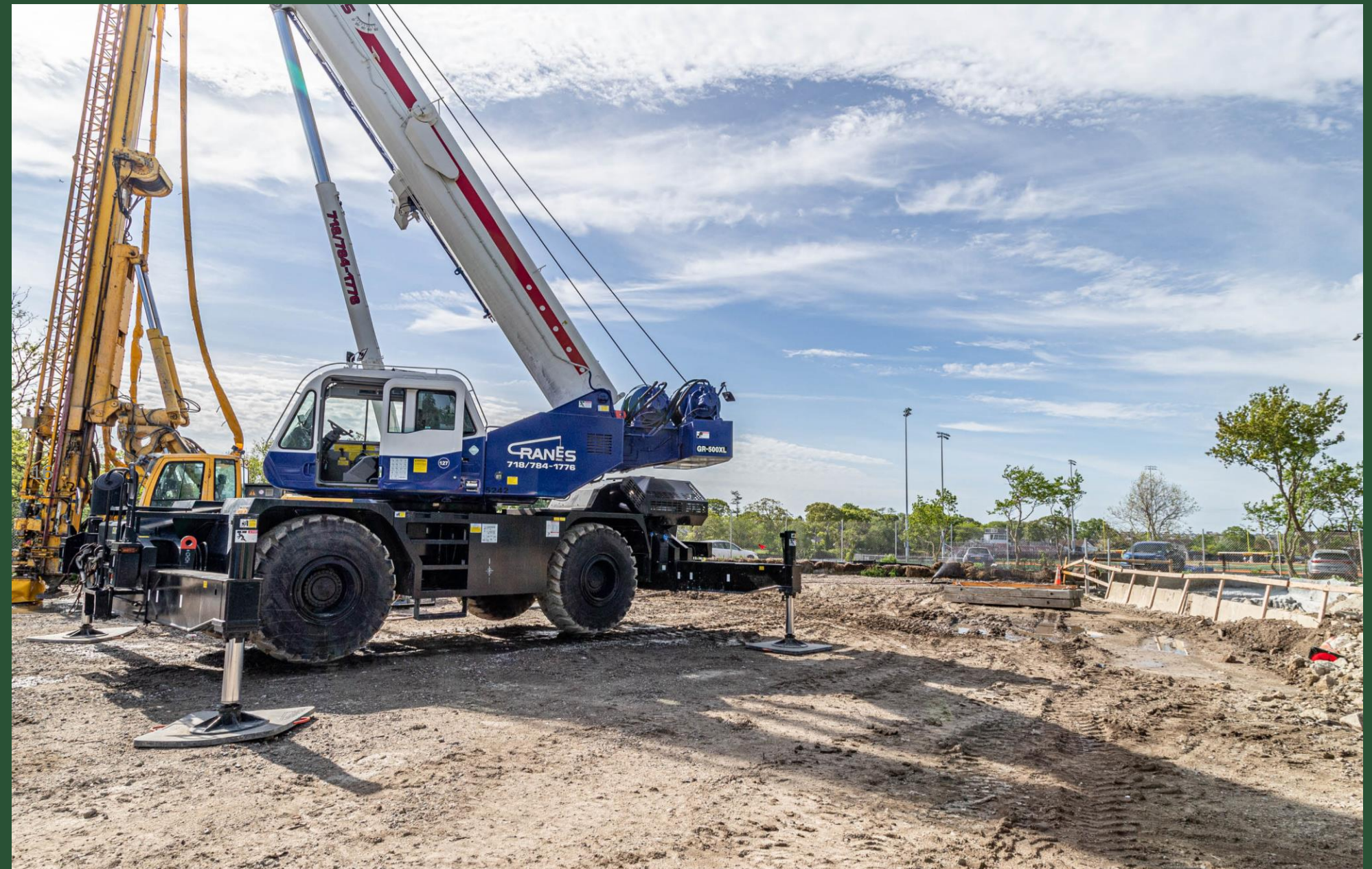
SOE Installation at BP7 (May 2022)
