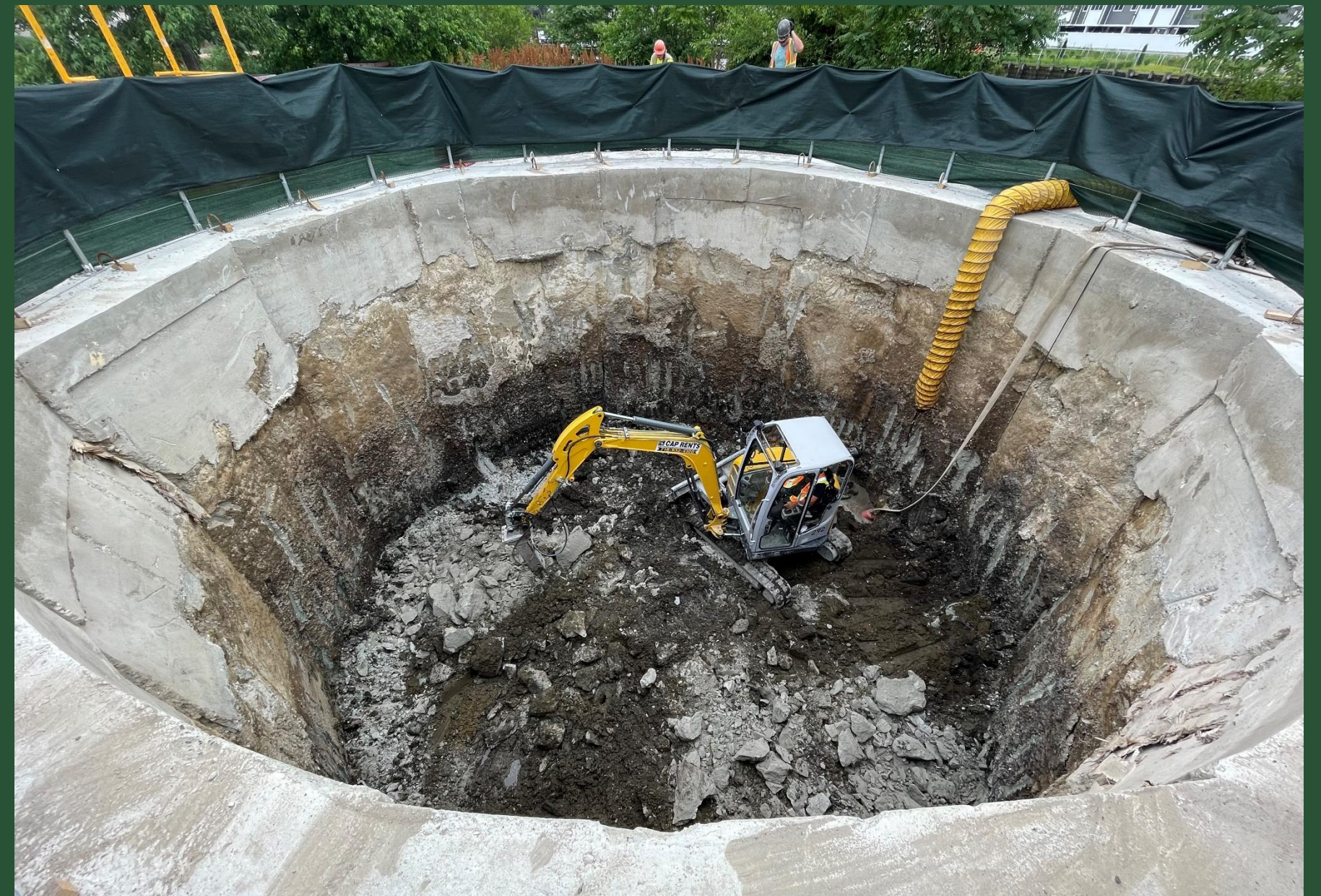
Excavation at BP5 (June 2022)
