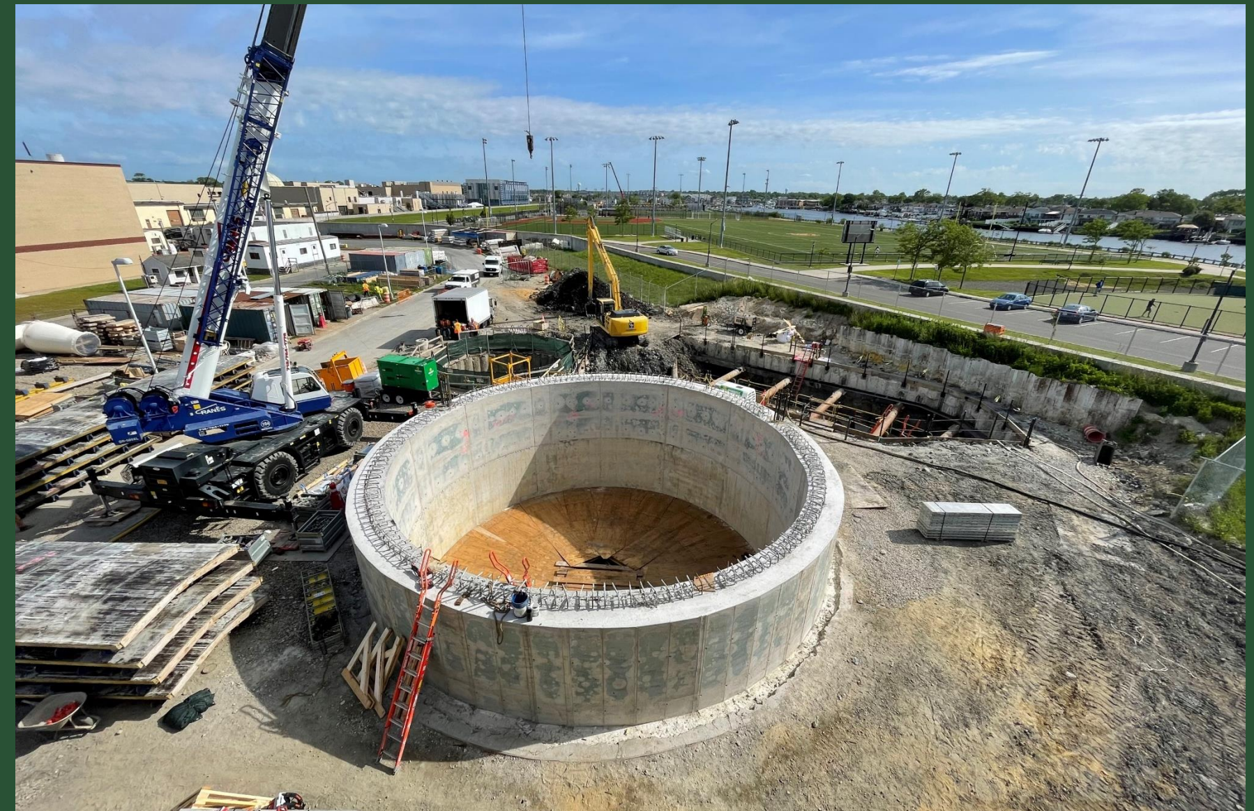
Diversion Structure at BP1 (June 2022)
