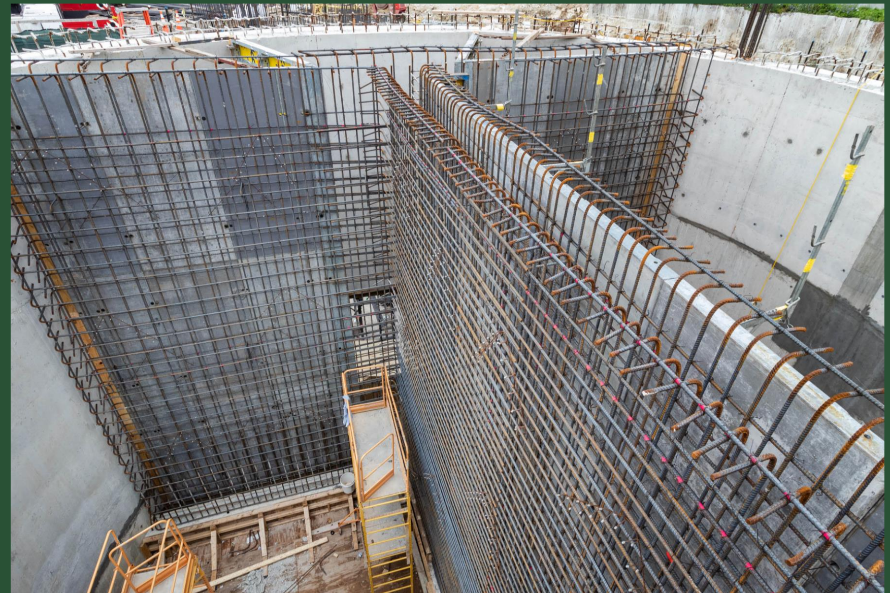
Diversion Structure Wall Construction Near BP1 (July 2022)
