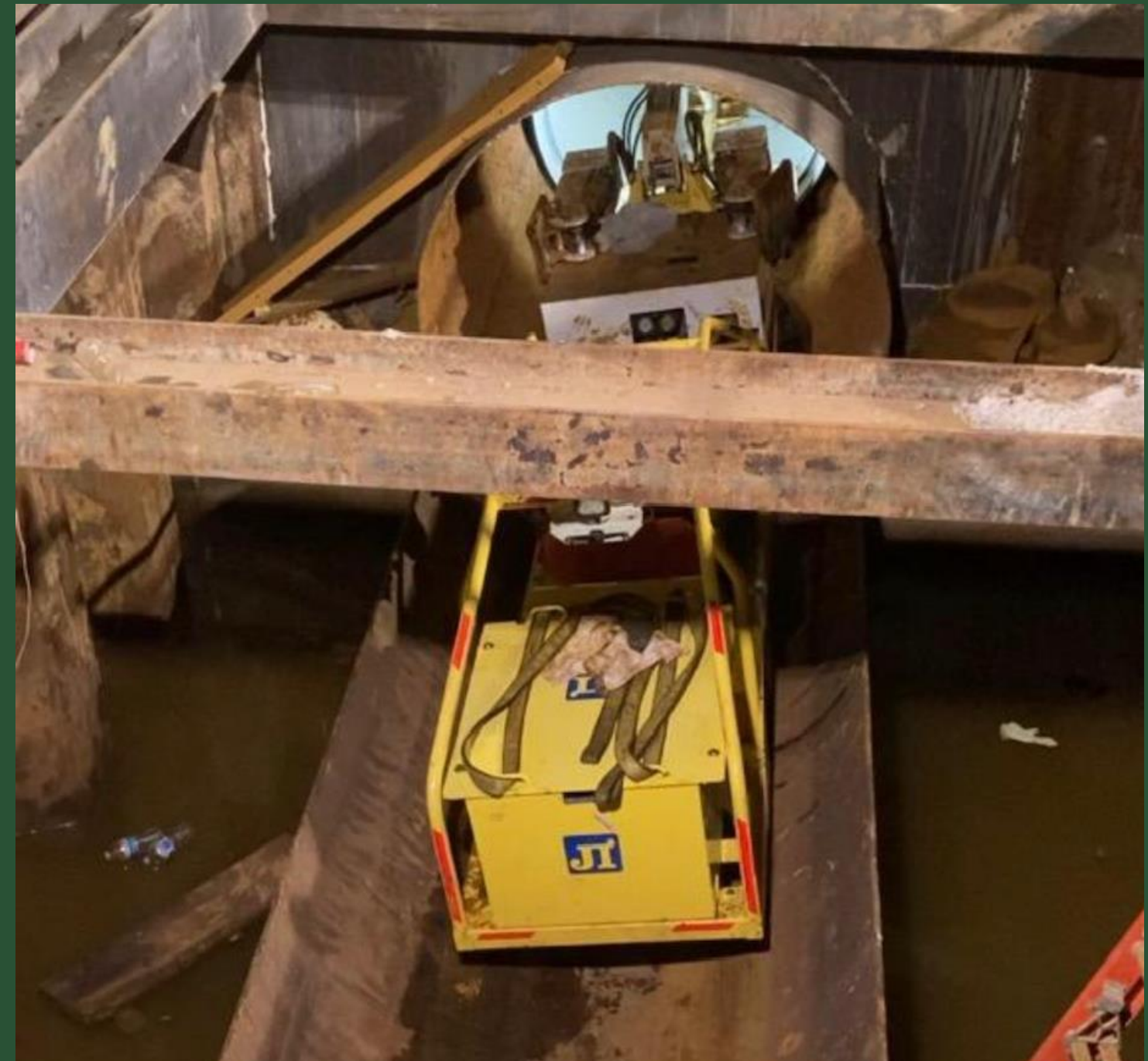
Jacking Equipment at Pit S (August 2022)
