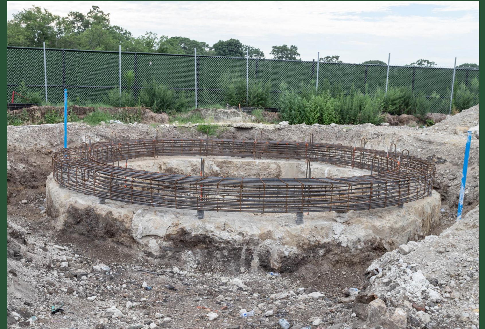
Construction Site at BP7 (July 2022)
