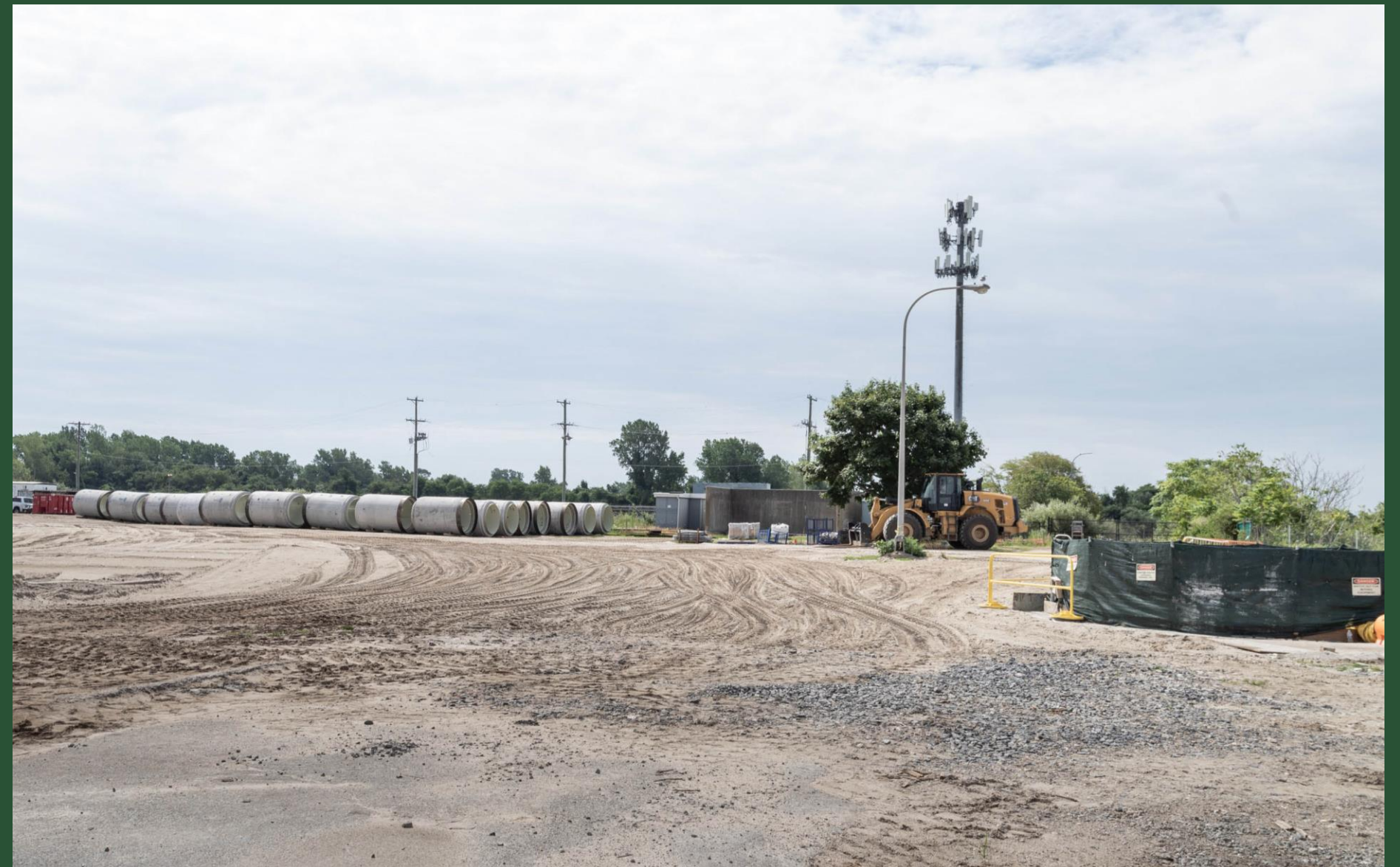
Pipe Delivery at CC1 (July 2022)
