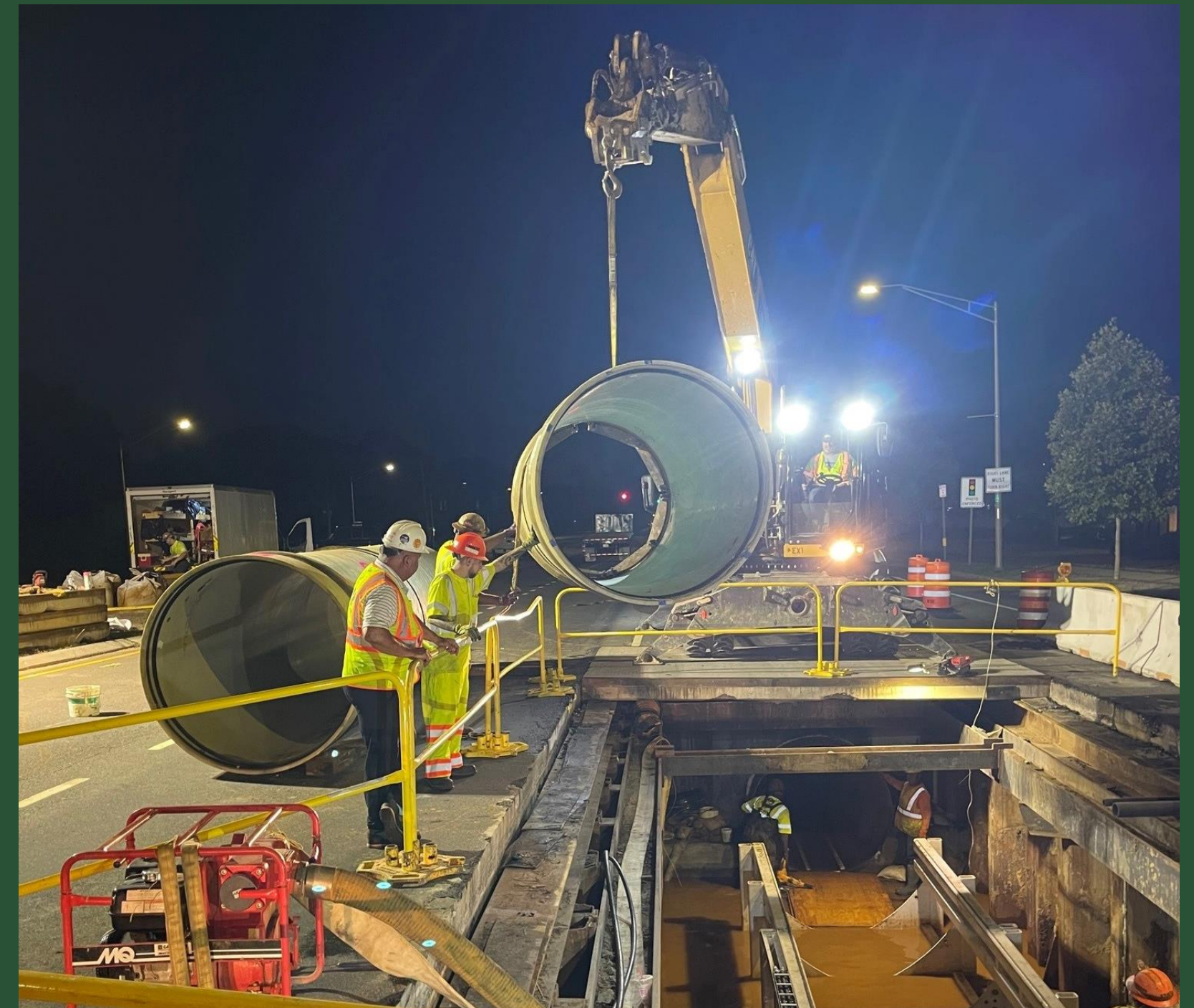
Sliplining Operations at Pit T (July 2022)
