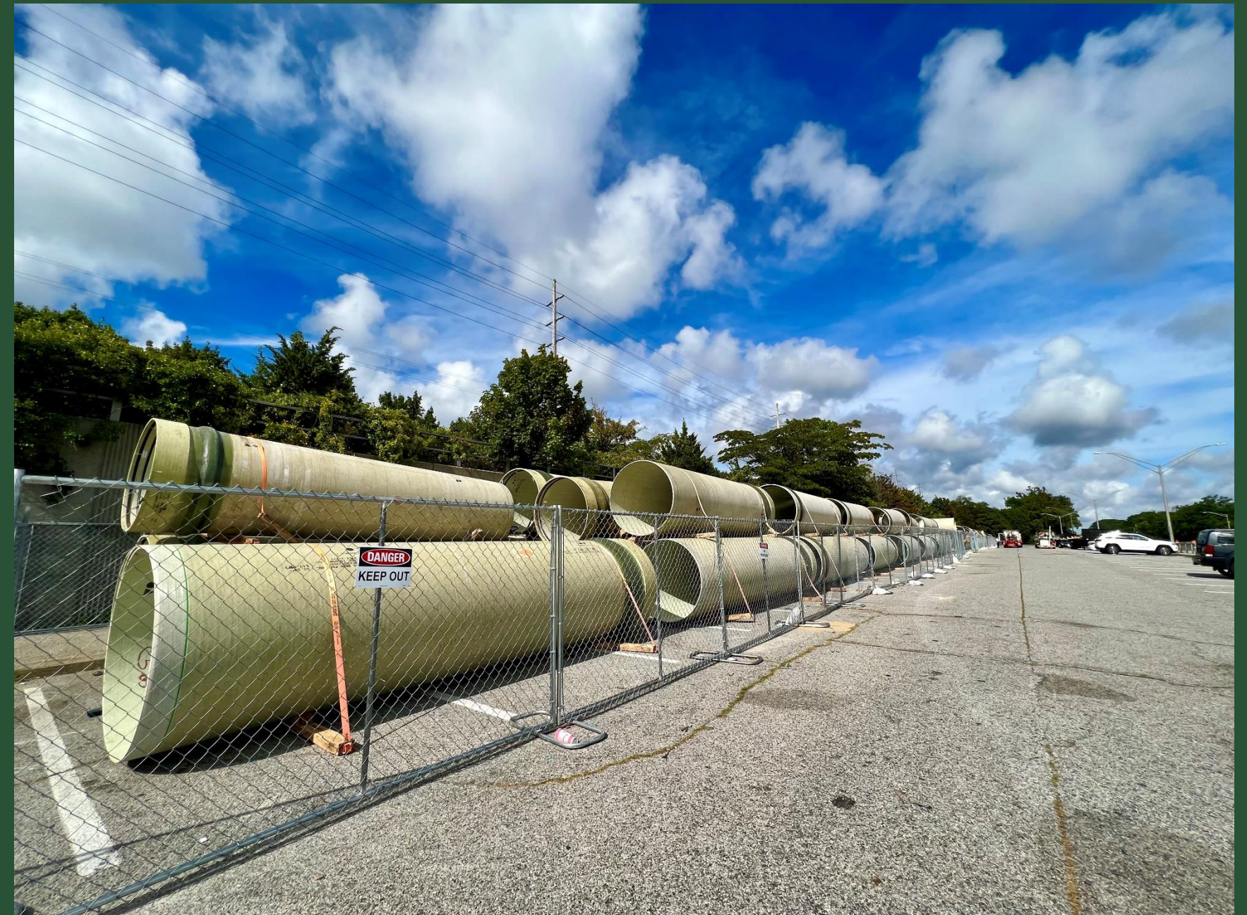
Sliplining Pipe near Sunrise Highway (August 2022)
