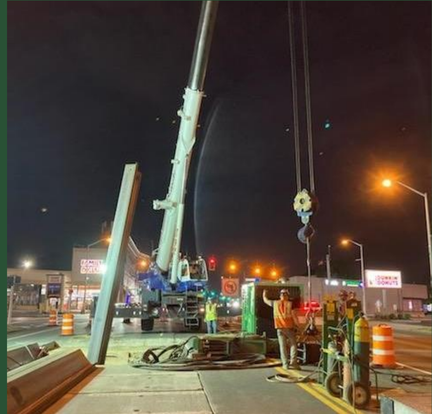
Sheet Pile Installation at Pit N (August 2022)
