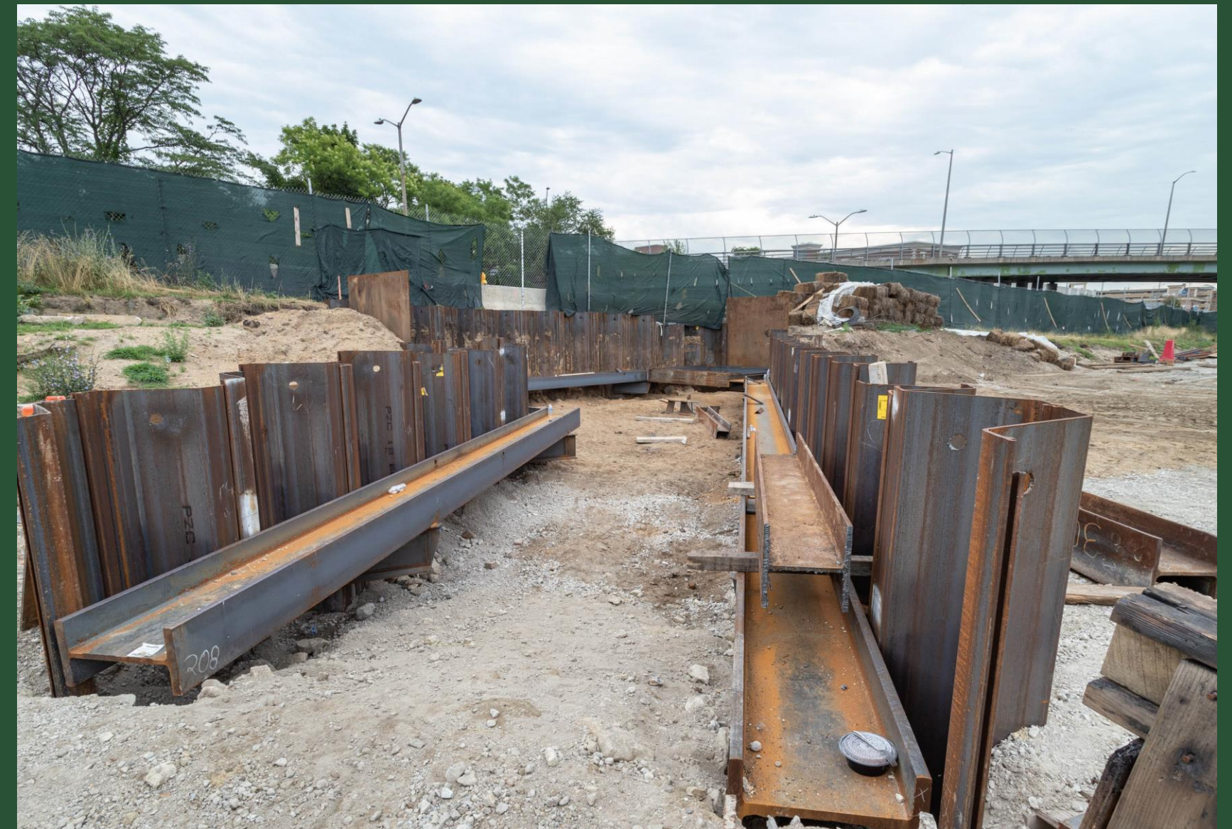
Sheet Pile Installation at BP9 (July 2022)
