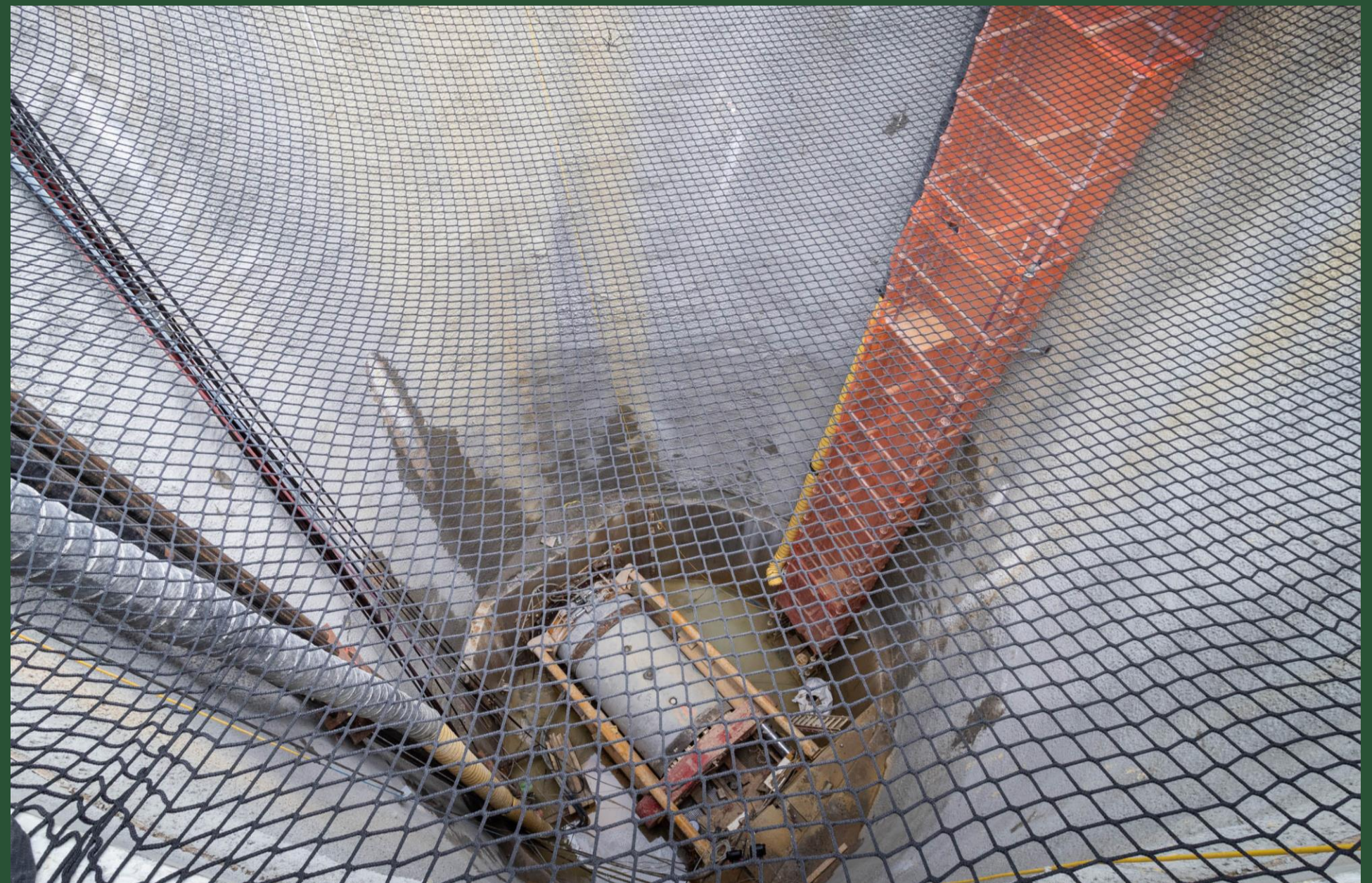
BP2 Microtunnel Operations (July 2022)
