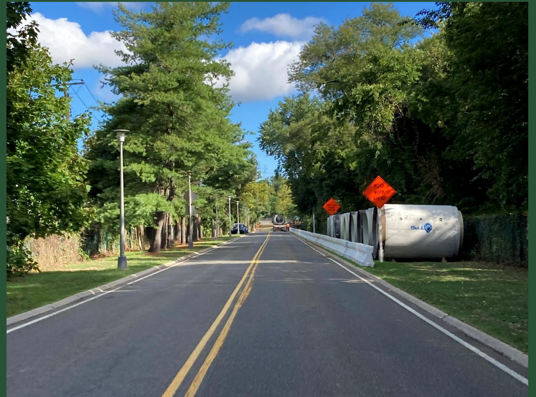
Pipe Delivery at CC4 (August 2022)
