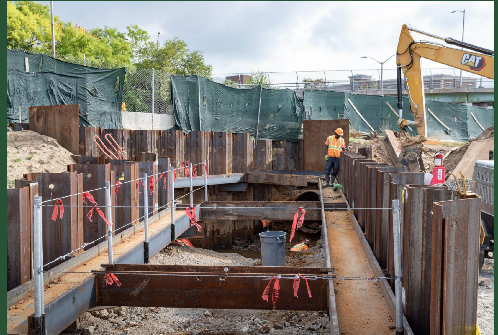
Sheet Pile Installation at BP9 (August 2022)
