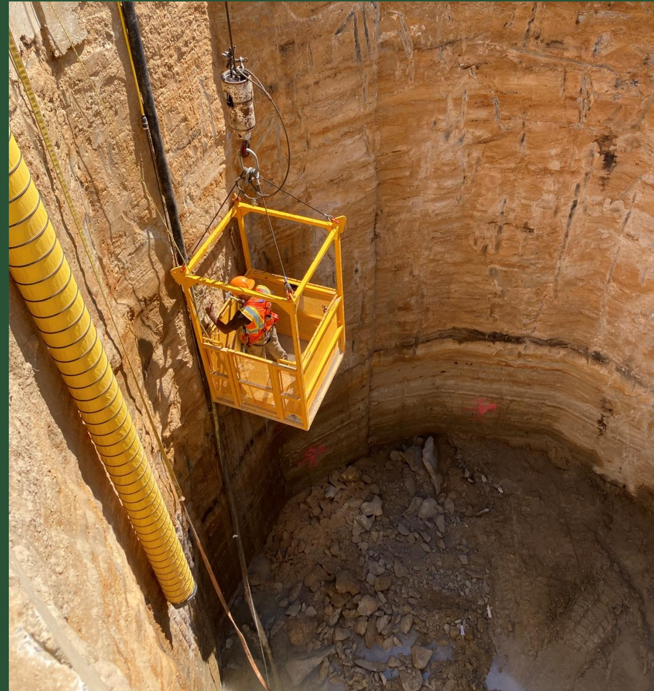
Excavation at CC5 (August 2022)
