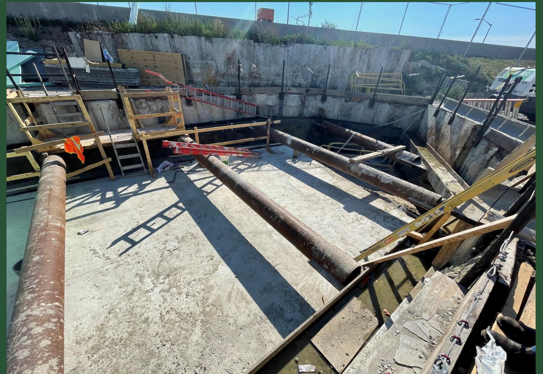
Diversion Structure Construction Near BP1 (August 2022)
