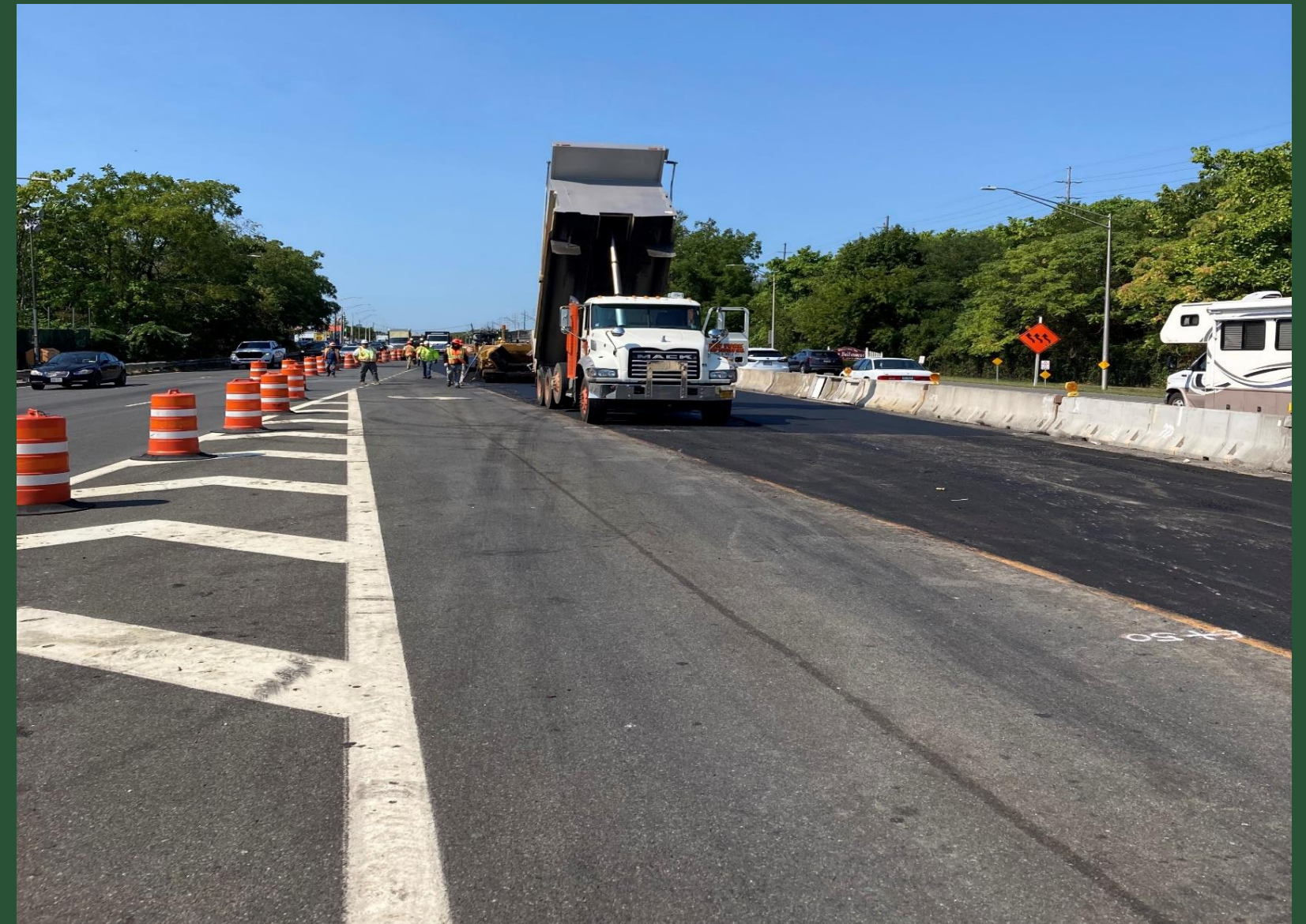
Paving near Pit W (September 2022)
