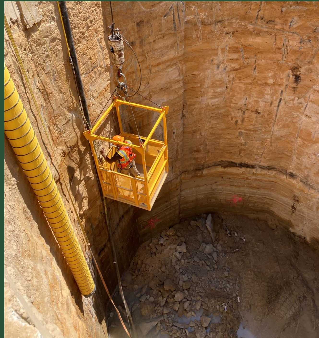
Excavation at CC5 (August 2022)
