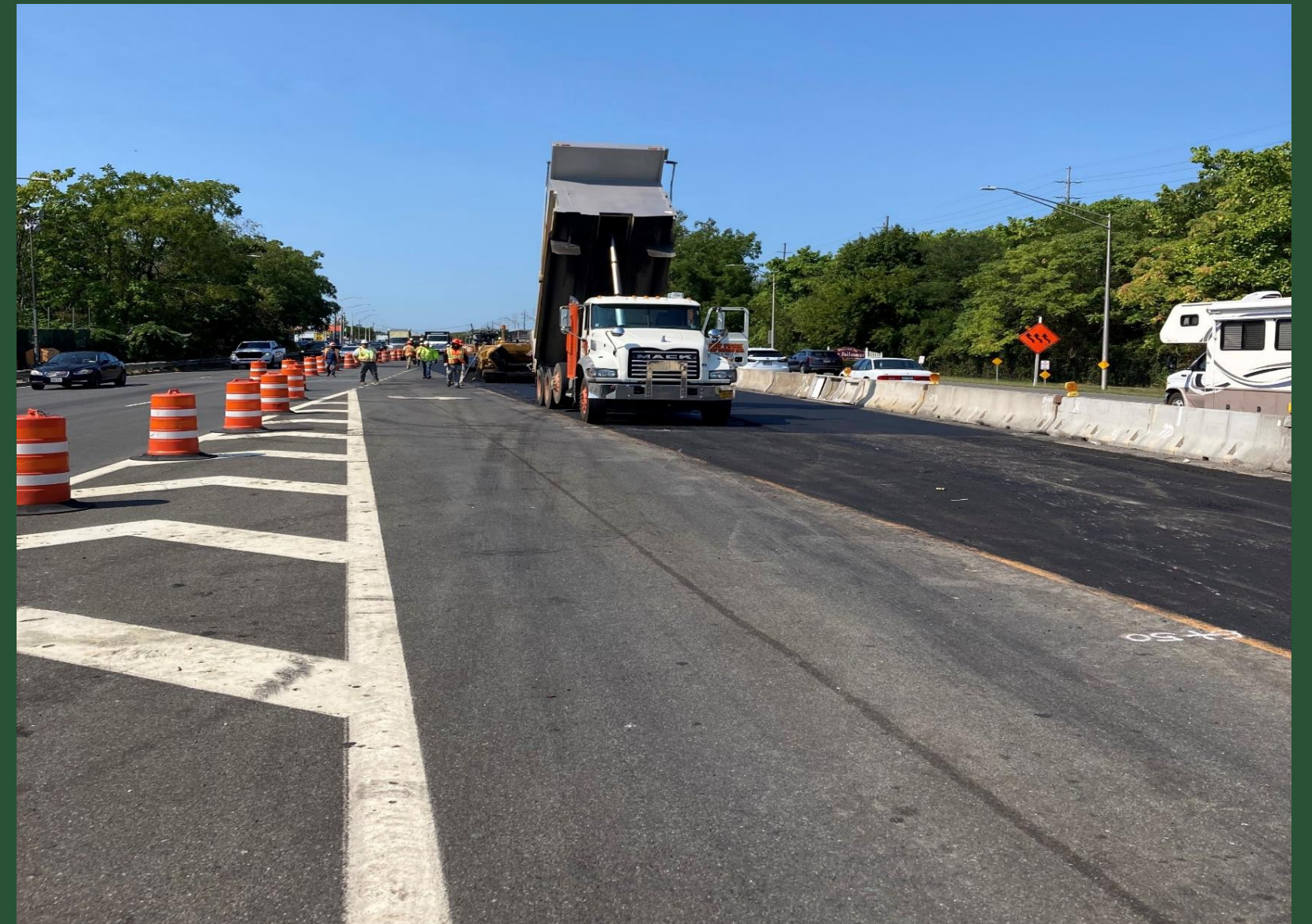
Paving near Pit W (September 2022)
