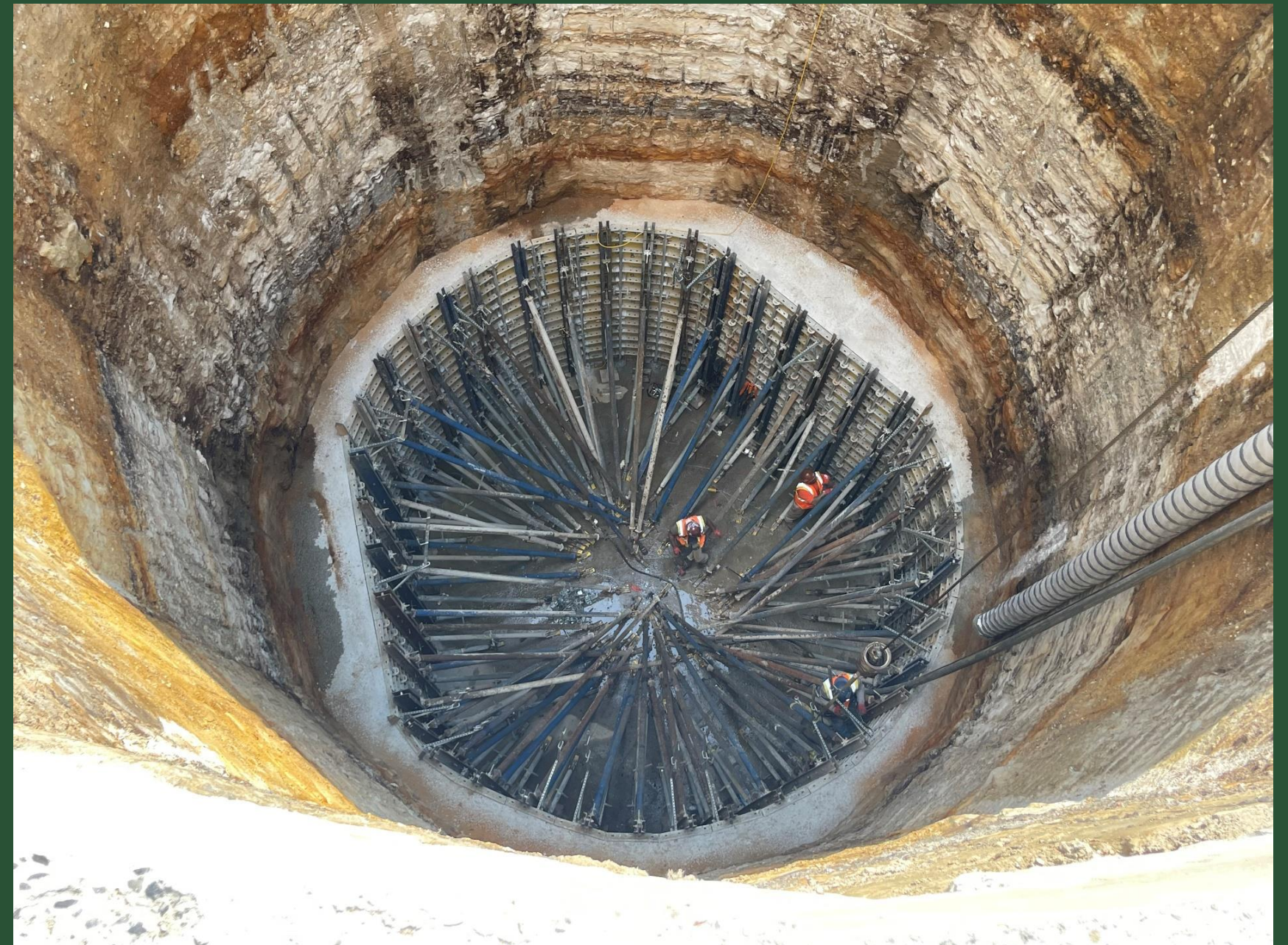
Concrete Liner Wall Construction at BP5 (September 2022)
