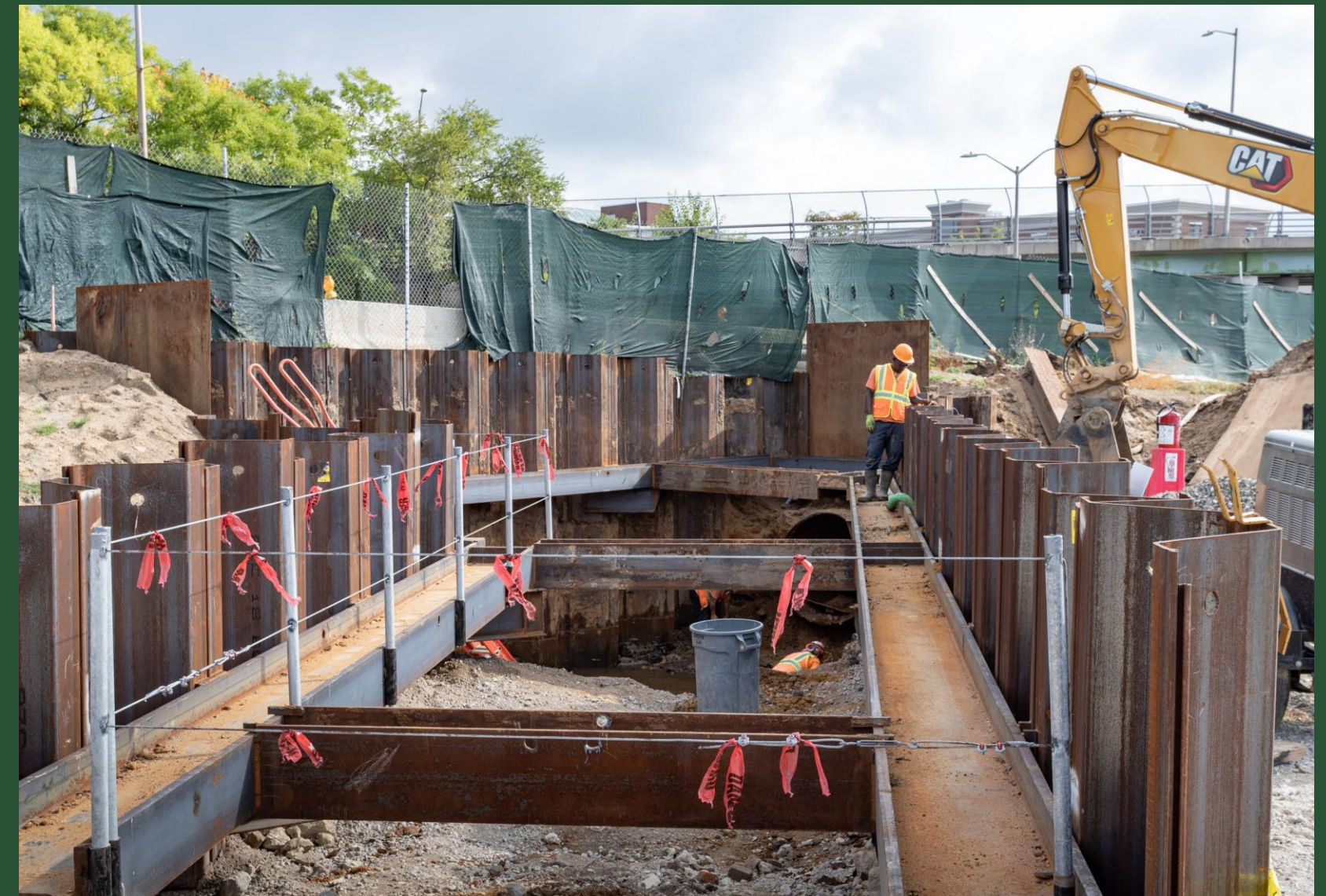
Sheet Pile Installation at BP9 (August 2022)
