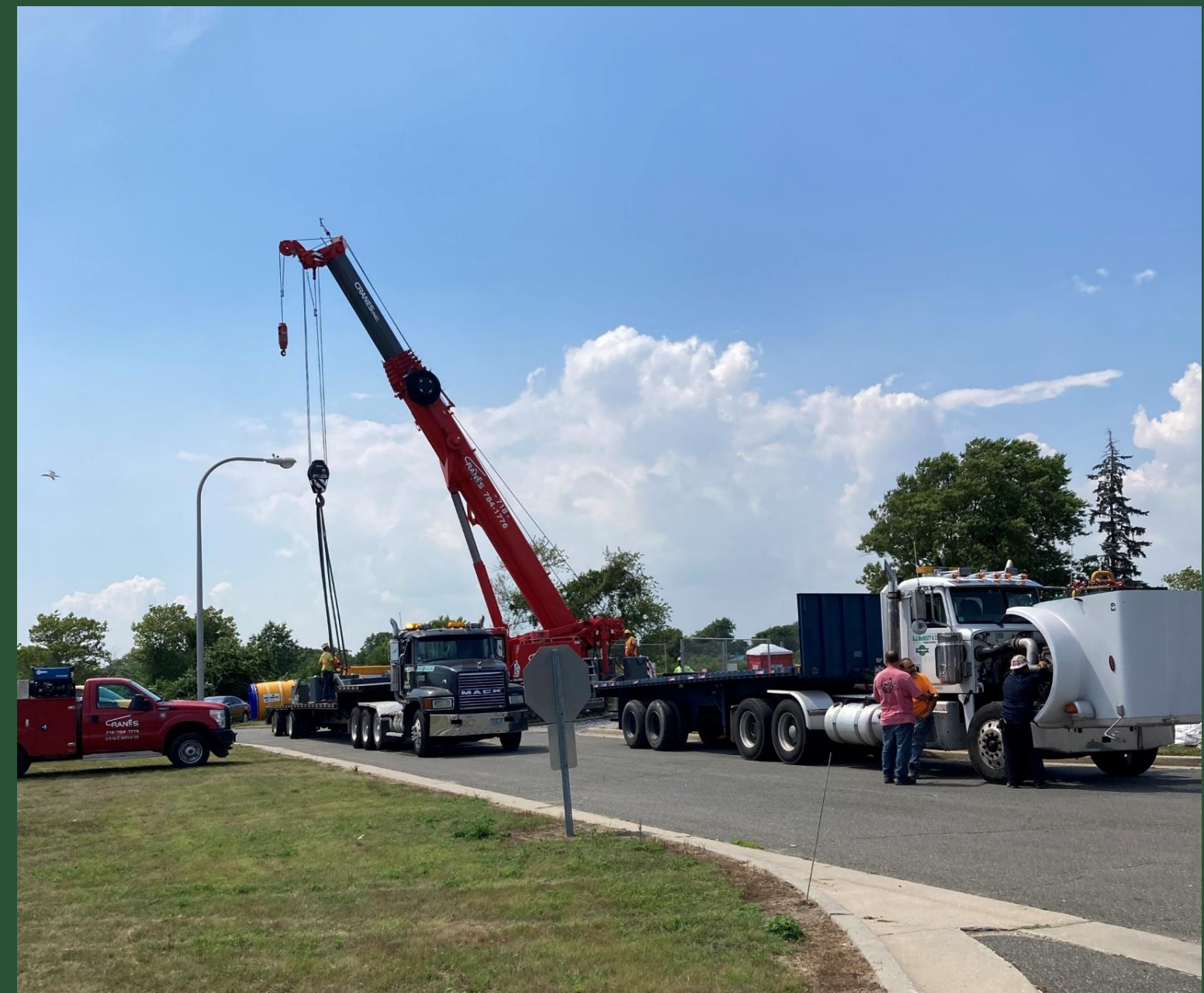
CC2 Mobilization for Microtunneling (August 2022)
