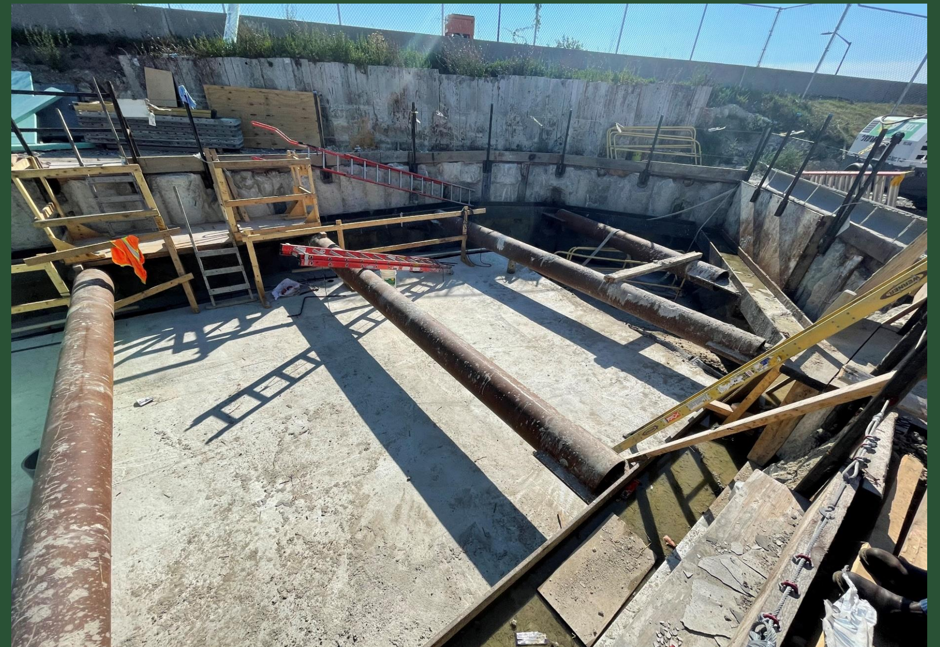
Diversion Structure Construction Near BP1 (August 2022)
