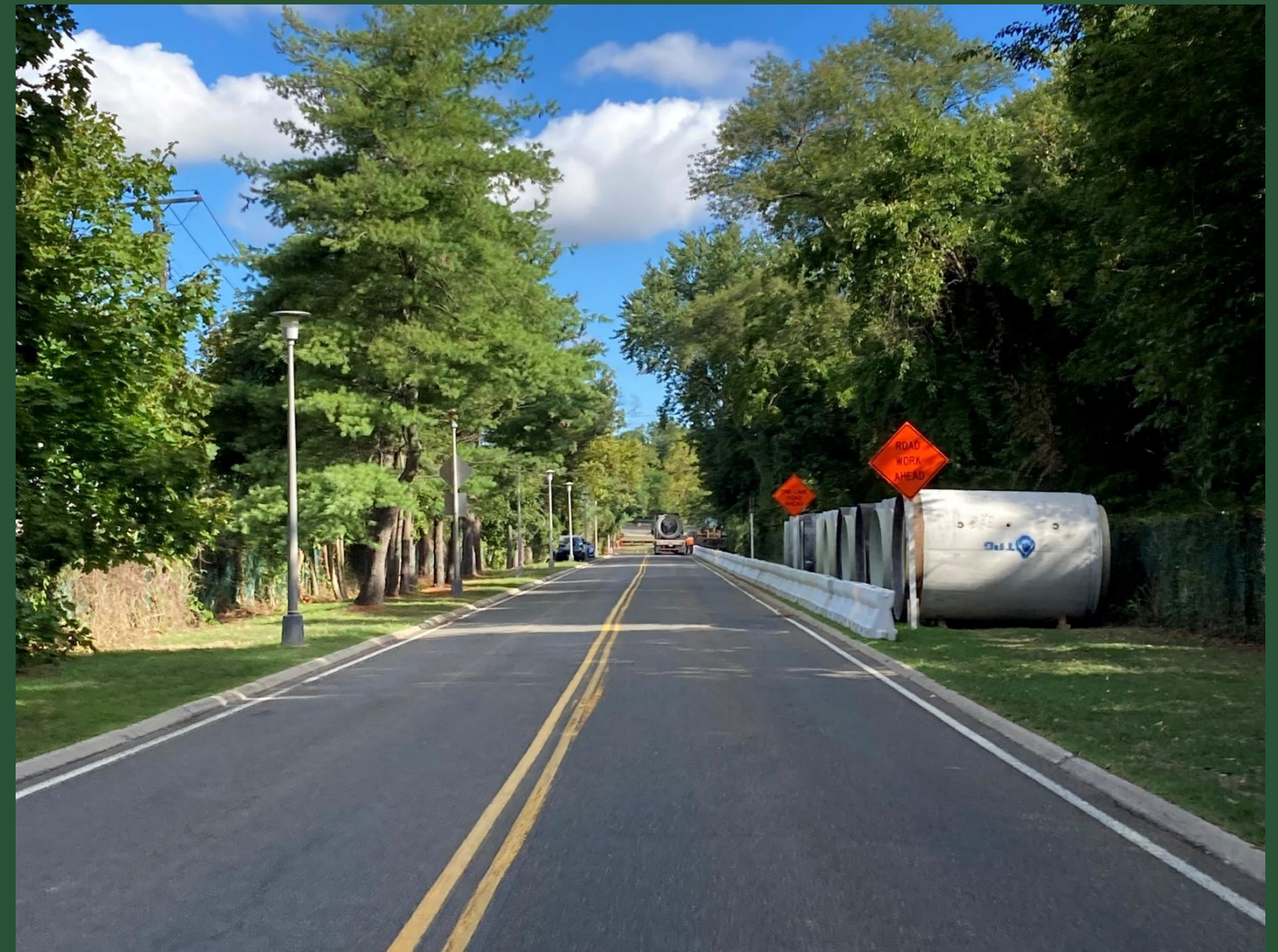
Pipe Delivery at CC4 (August 2022)
