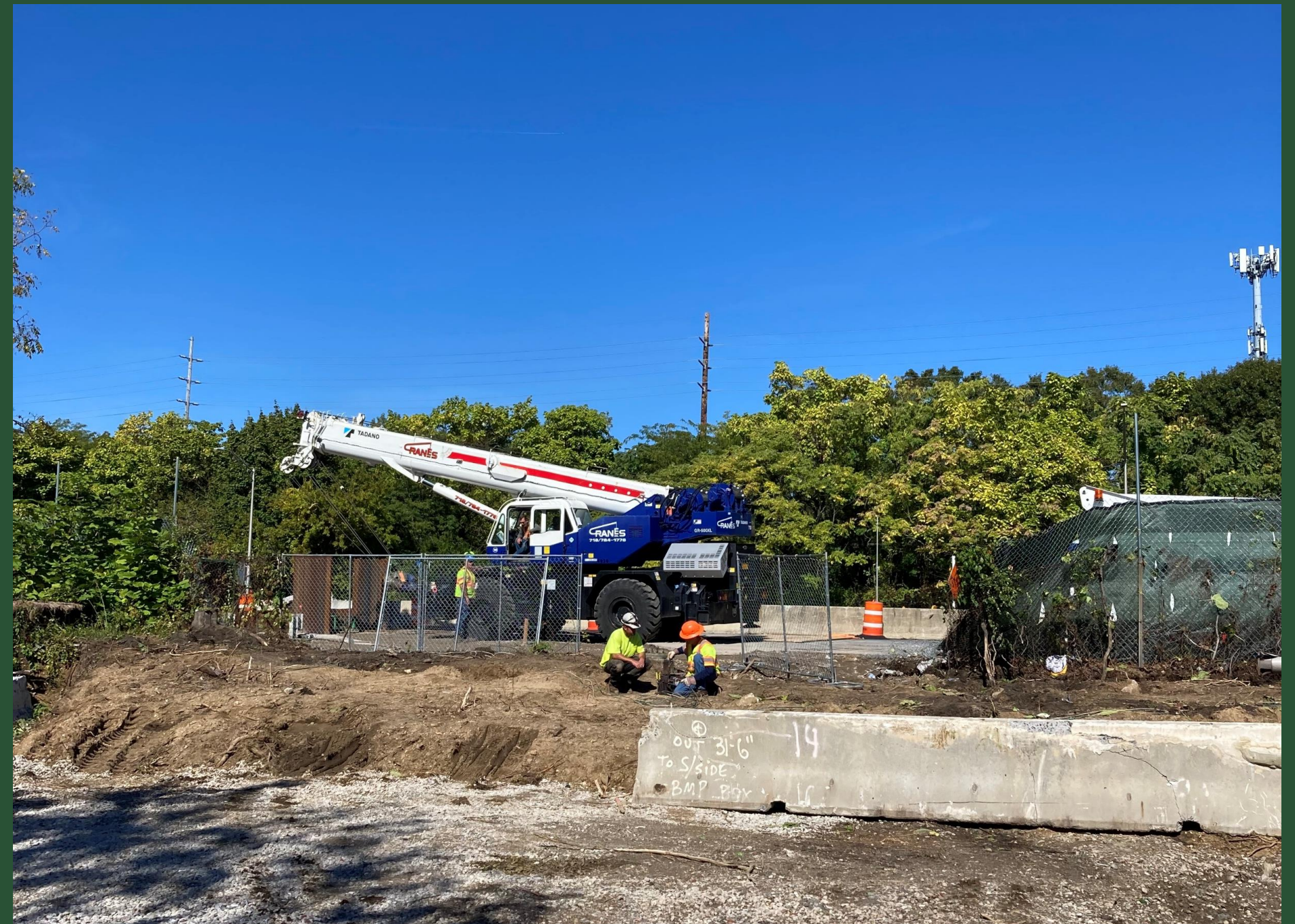
Construction at CC6 (October 2022)
