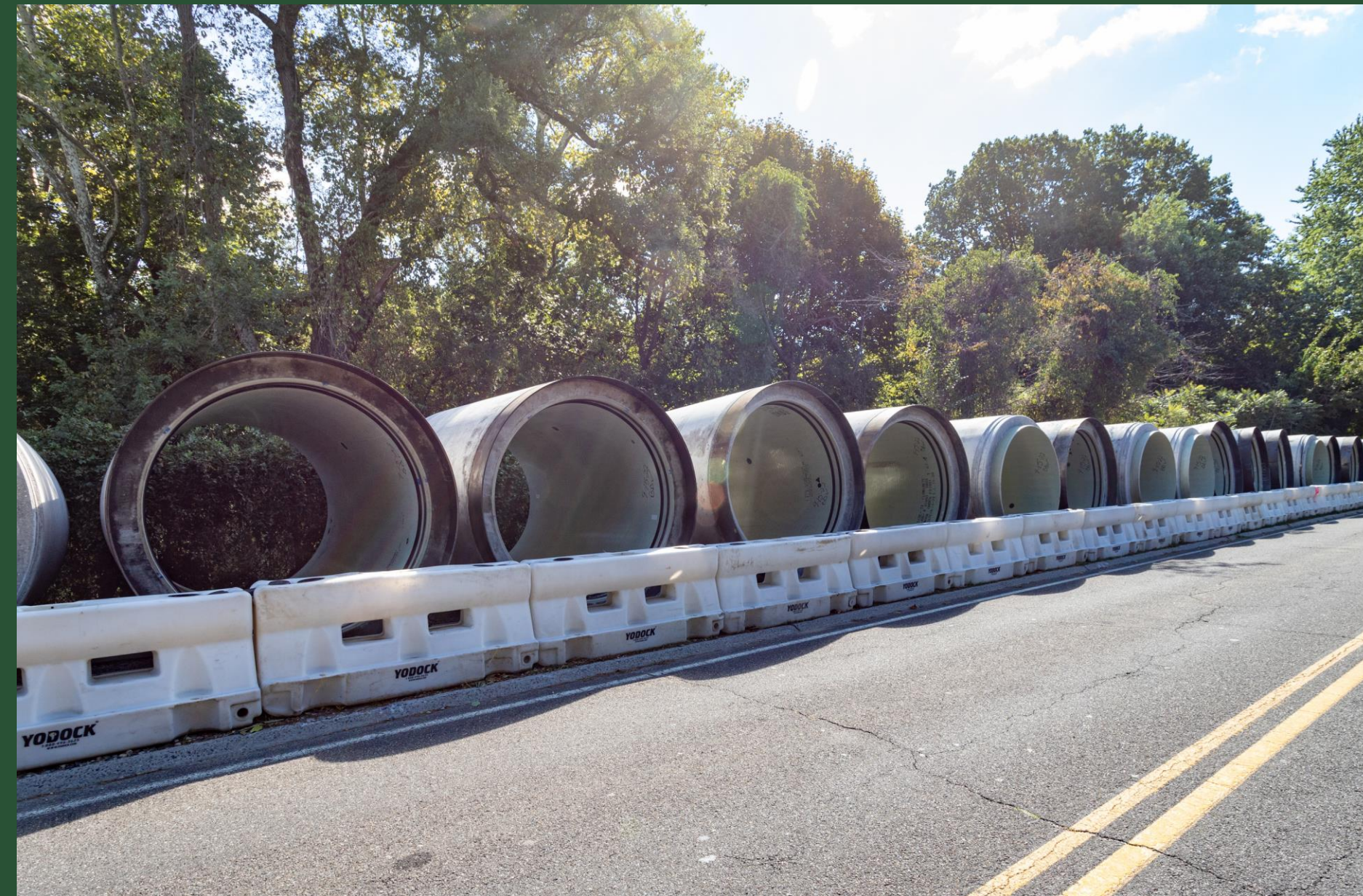
Pipe Delivery at CC4 (September 2022)
