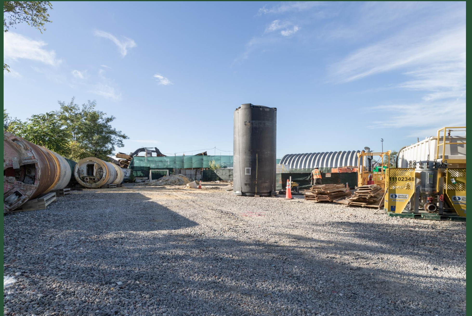
BP3 Construction Site (September 2022)
