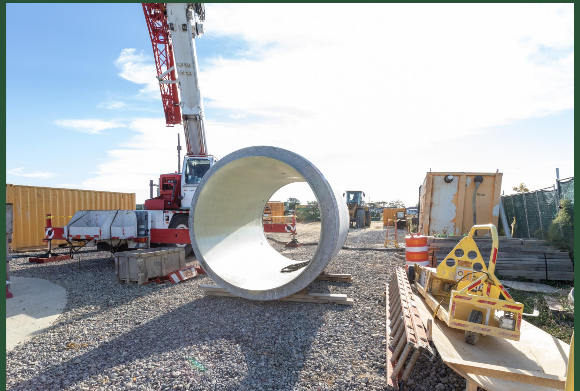
BP2 Construction Site (September 2022)
