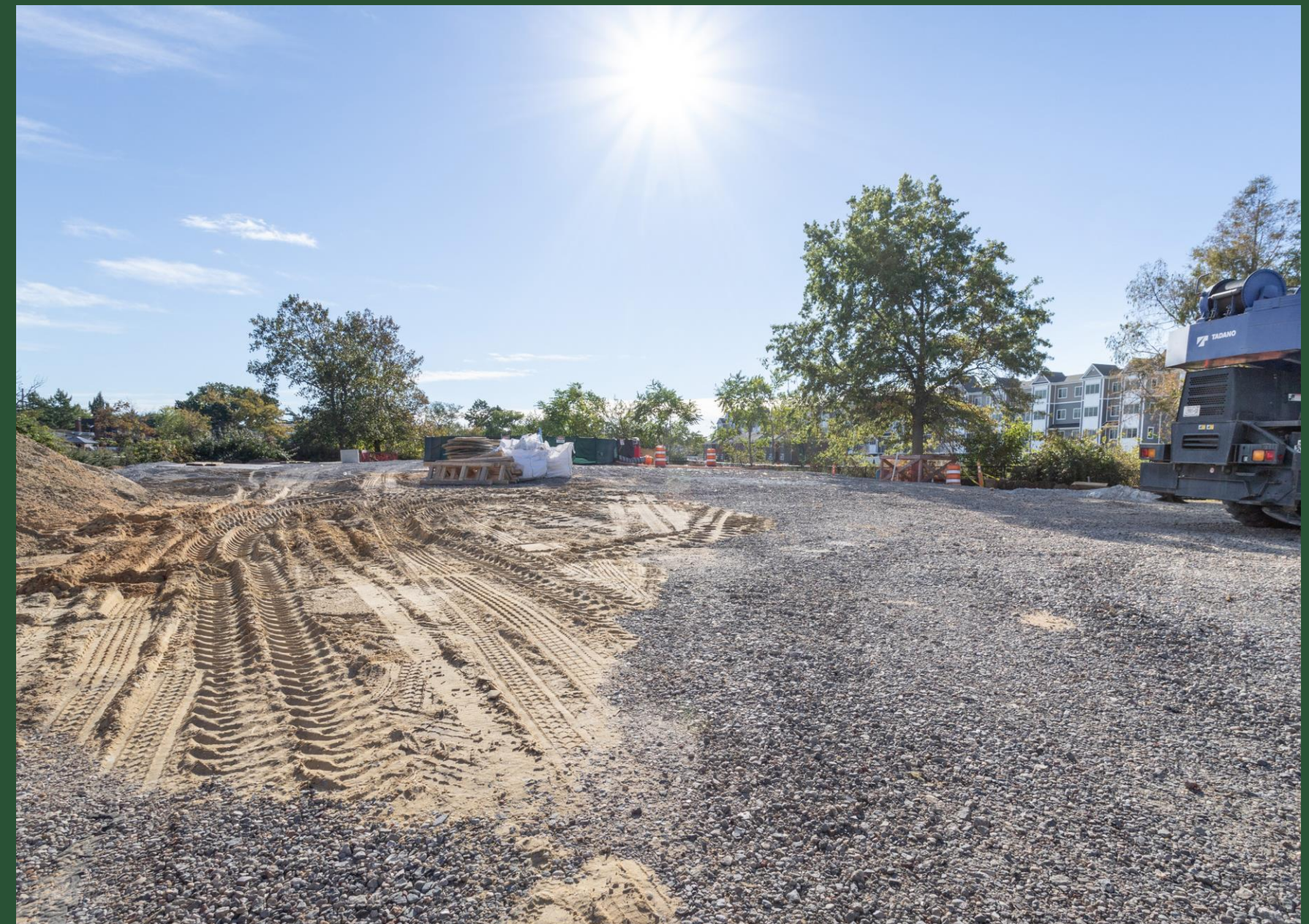
BP5 Construction Site (September 2022)
