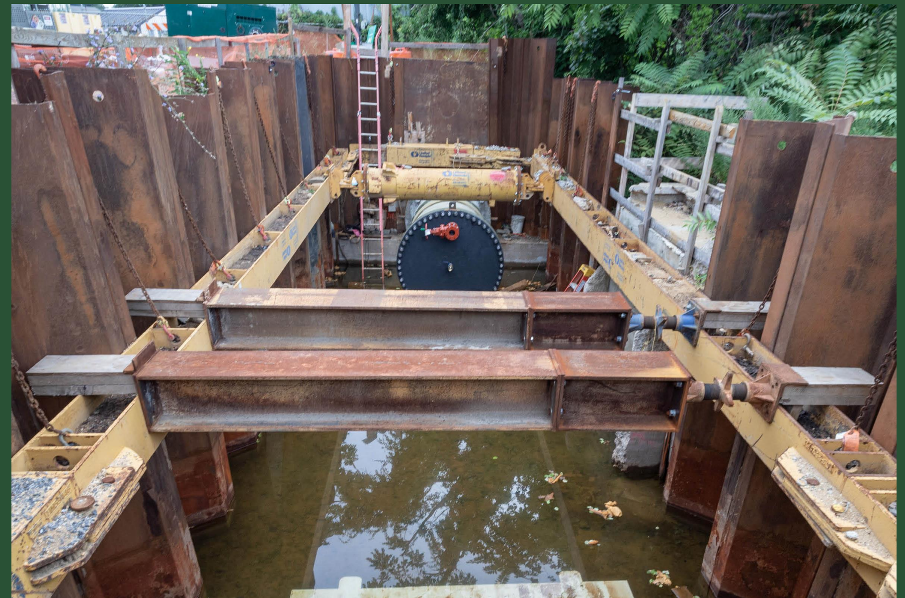
Preparations for Hydrostatic Testing at Pit O (August 2022)
