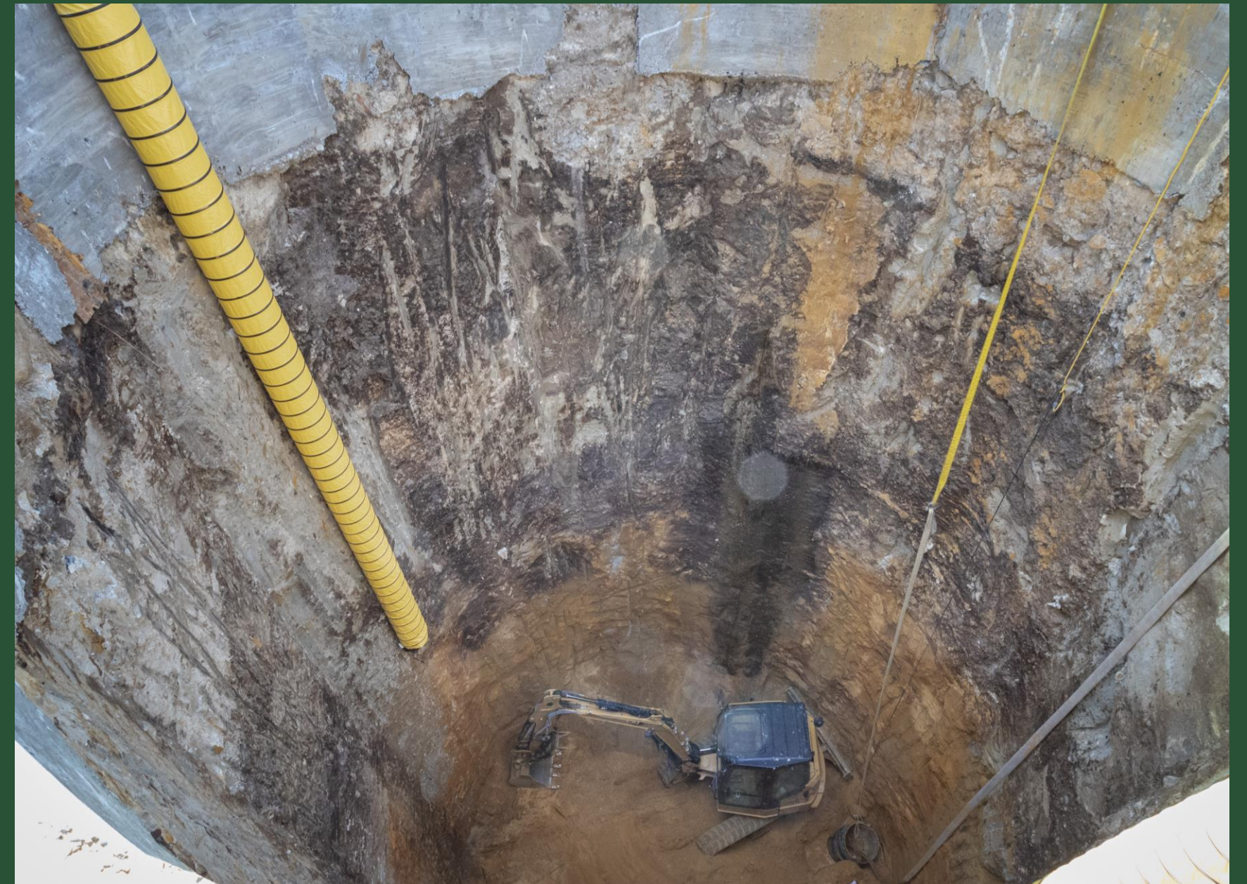
Excavation at BP7 (September 2022)
