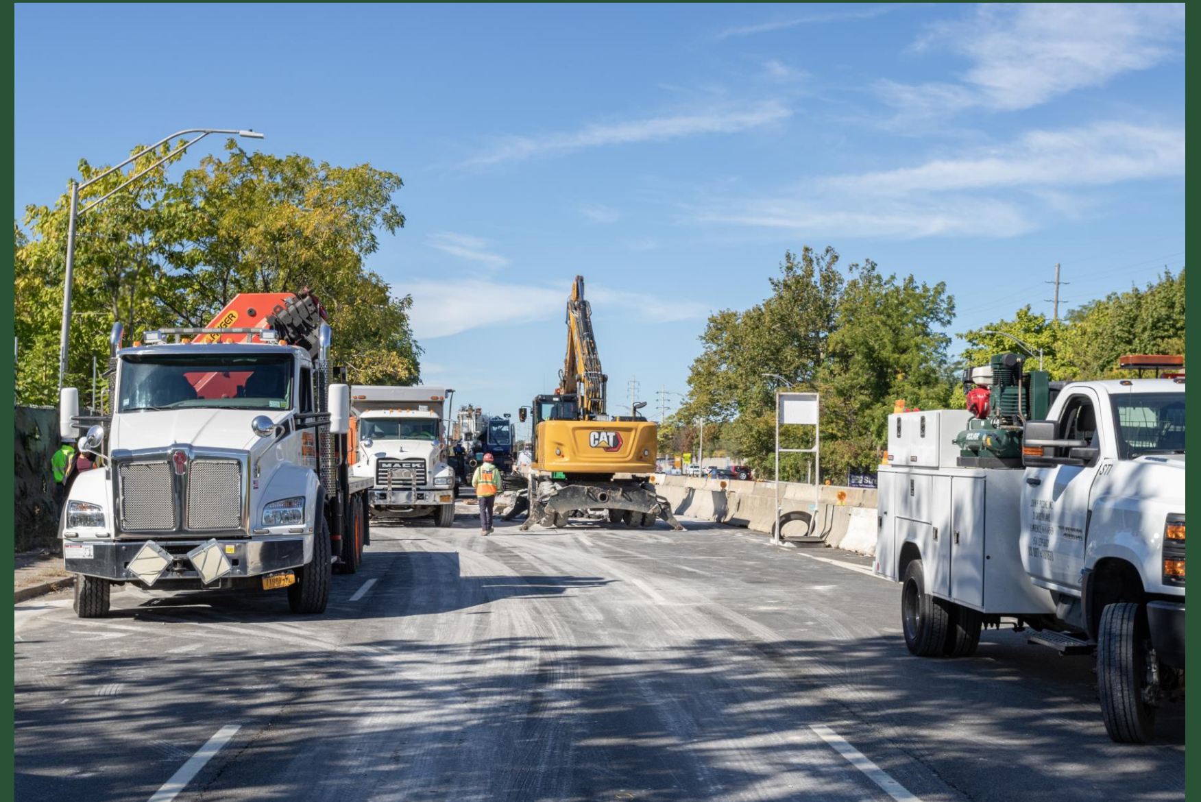
Construction at Pit W (September 2022)
