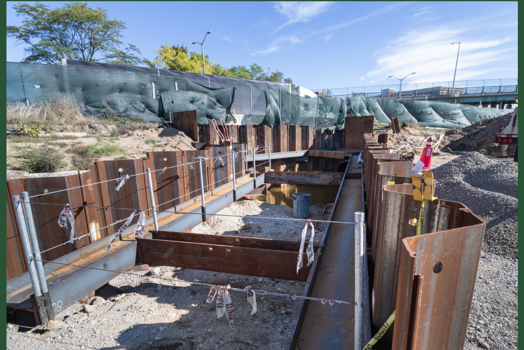
Sheet Pile Installation at BP9 (September 2022)
