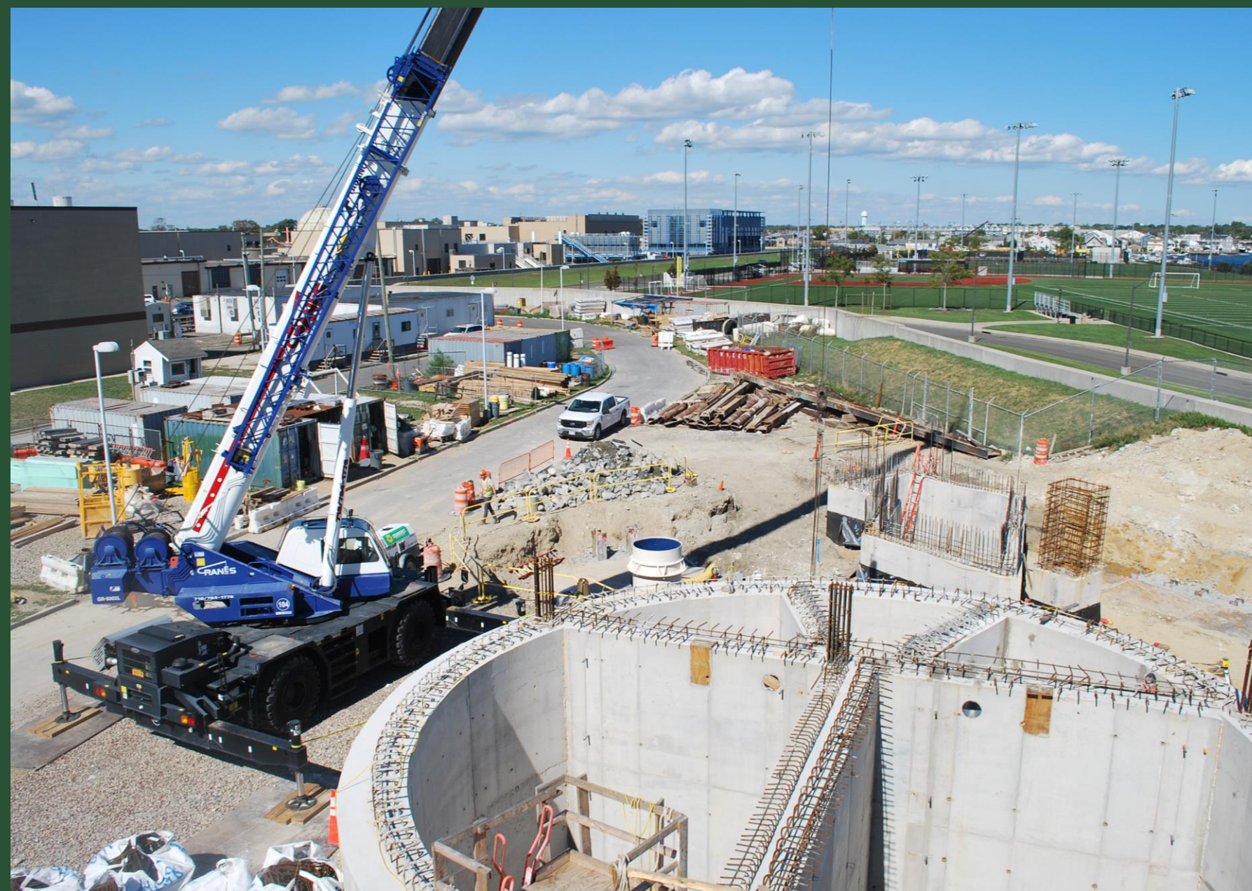
Diversion Structure Construction Near BP1 (September 2022)
