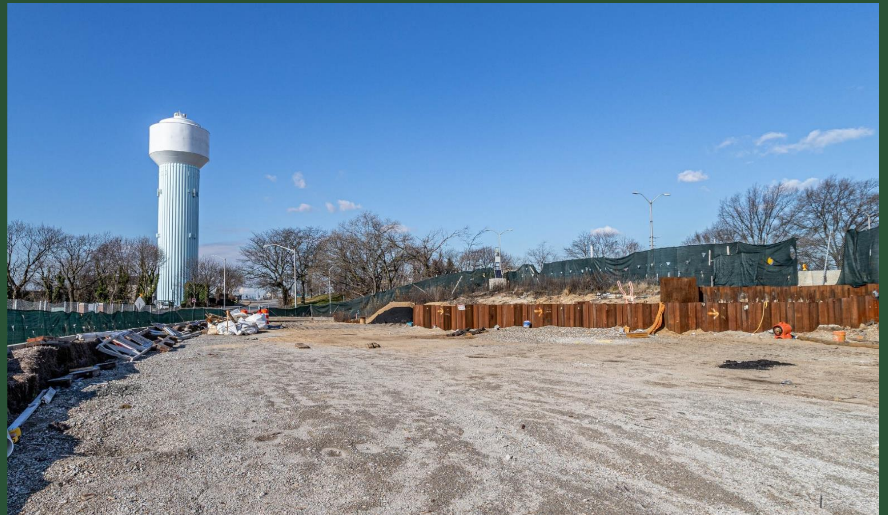
Construction Site at BP9 (January 2023)
