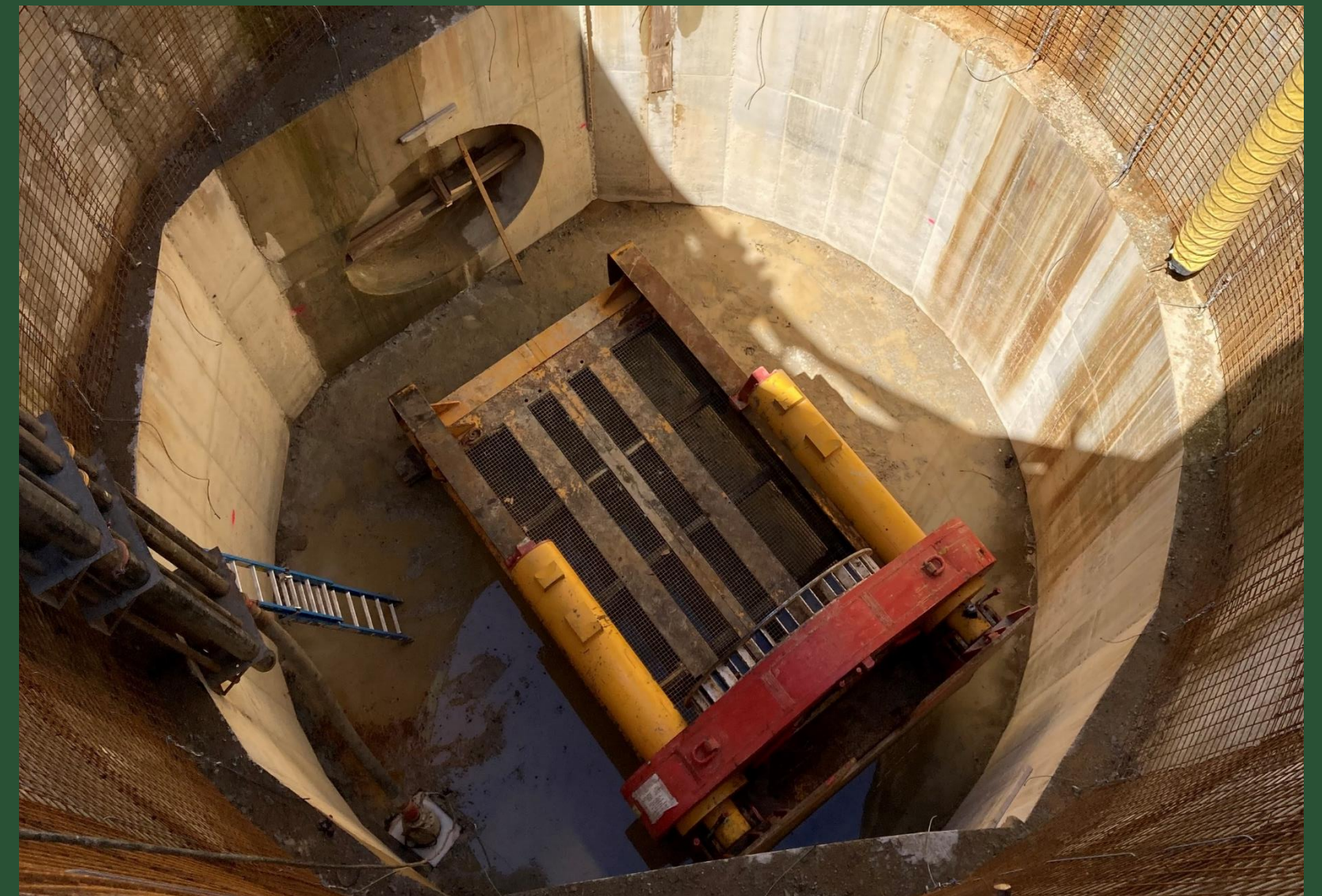
Shaft at CC4 (April 2023)
