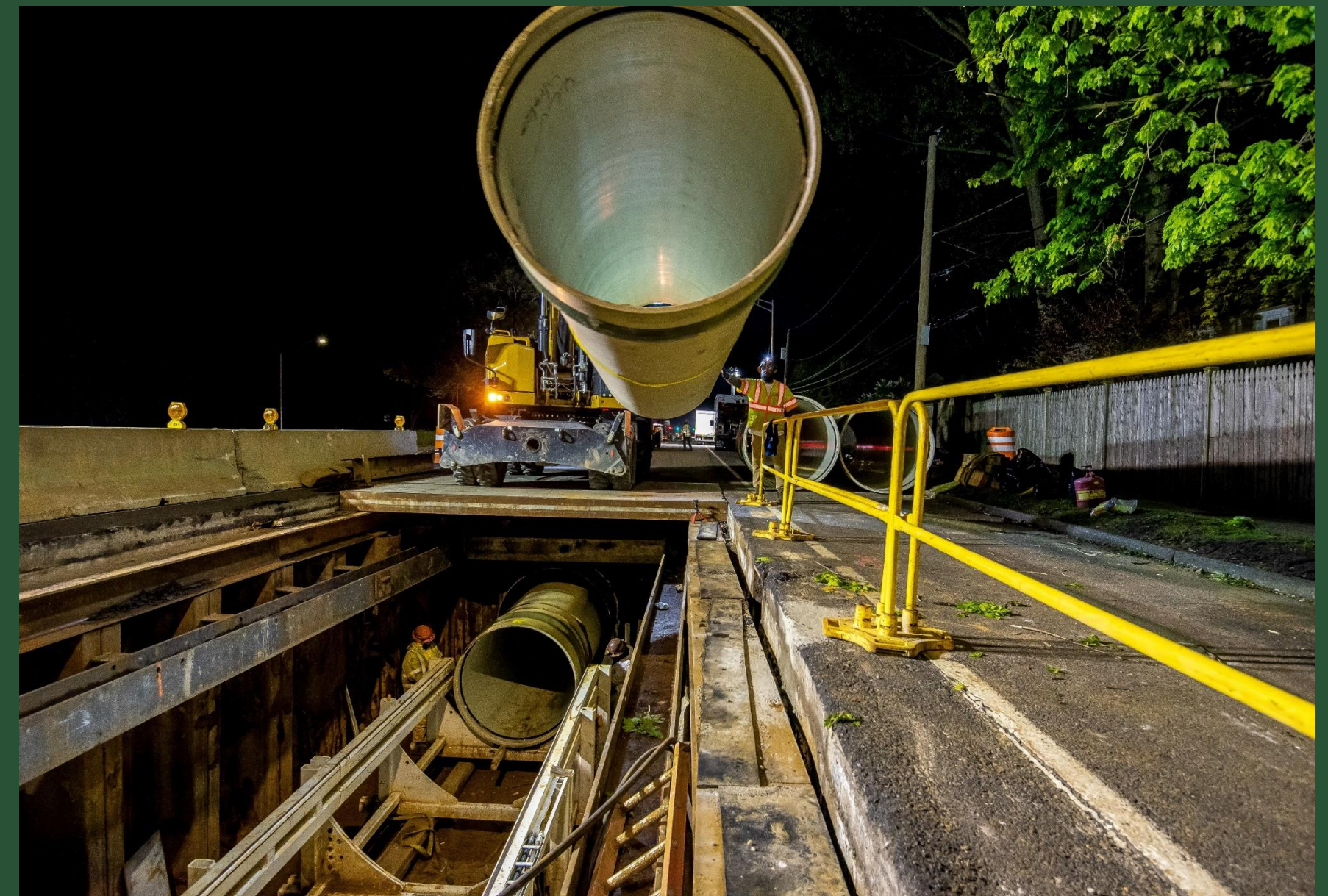
Sliplining at Pit FF (May 2023)
