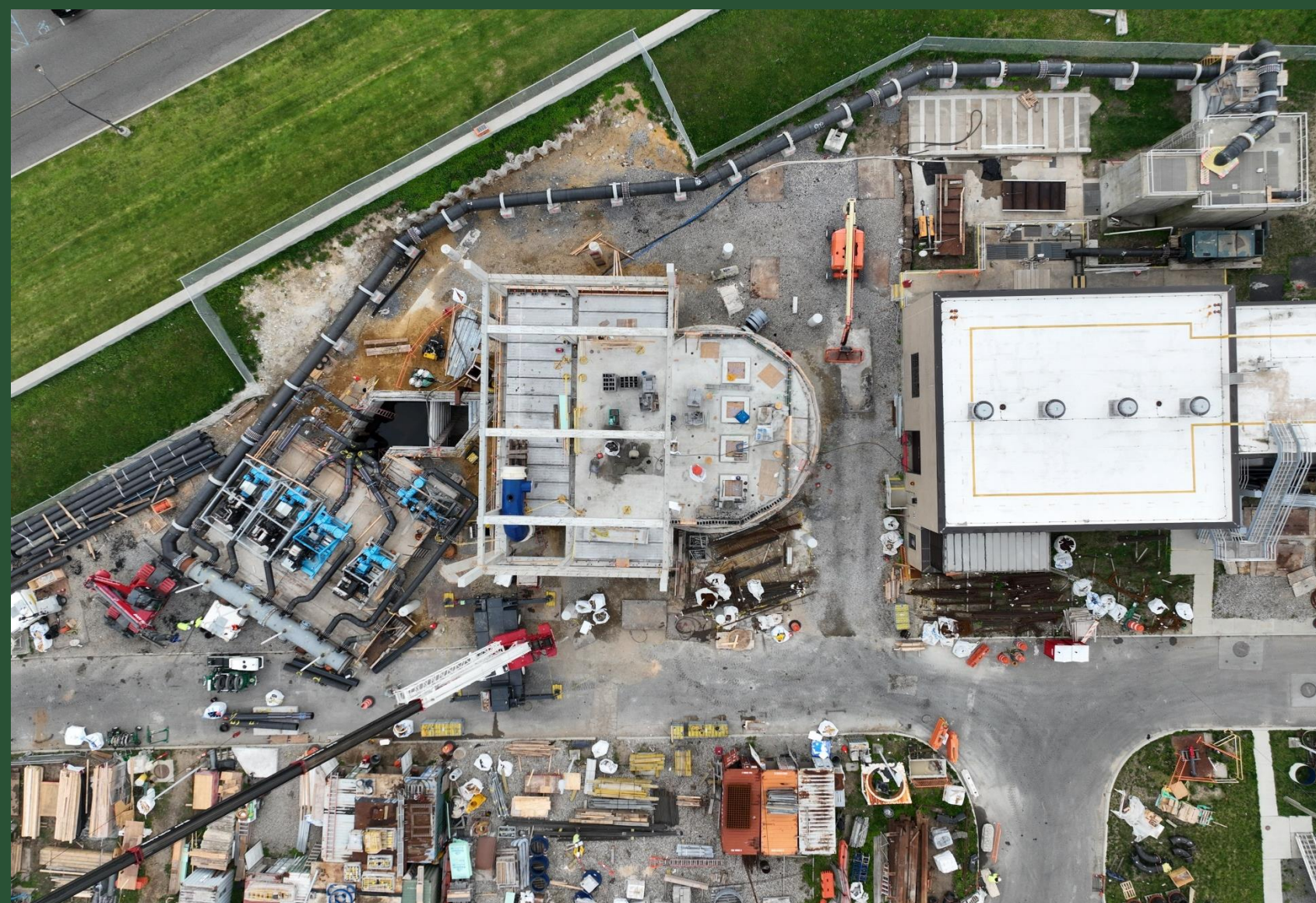
Pump Station Construction Near BP1 (April 2023)
