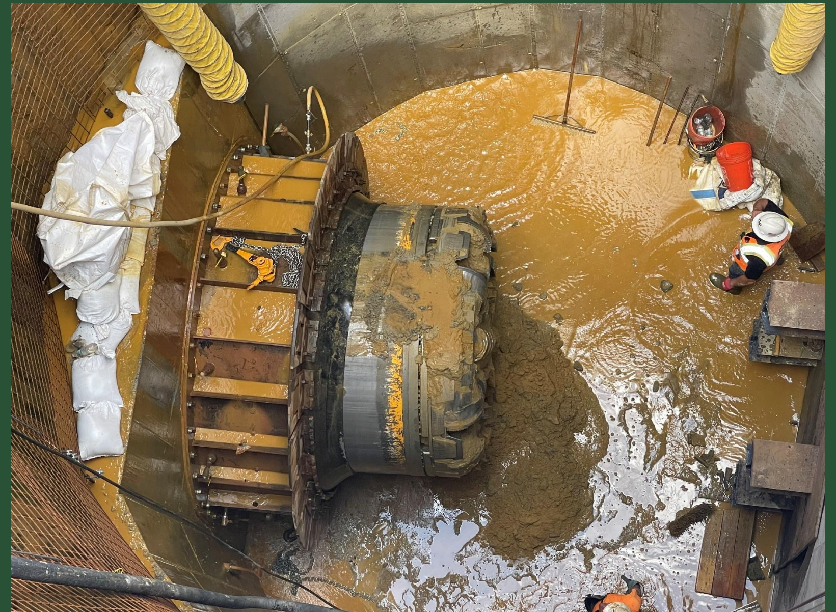
Breakthrough at BP7 (June 2023)
