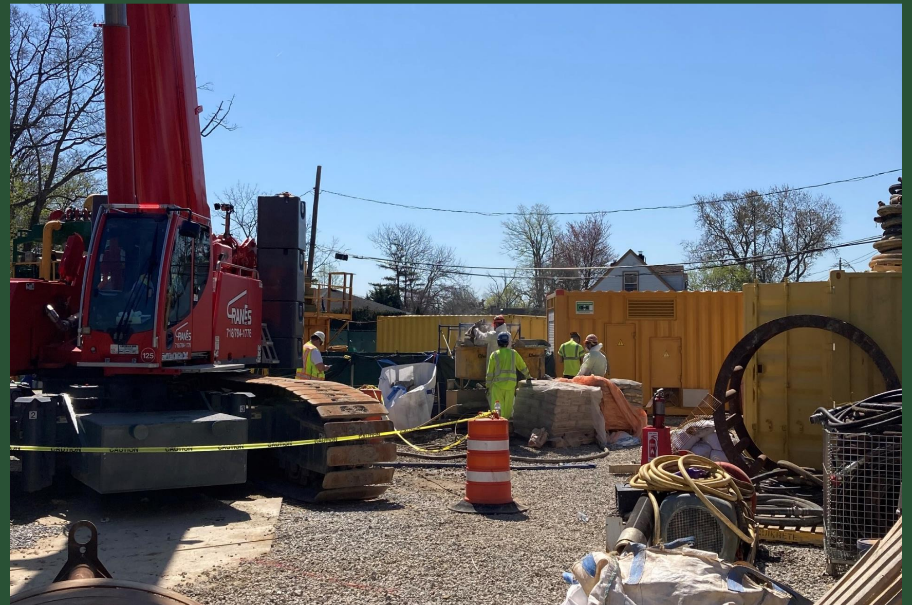
Grouting Activities at CC5 (April 2023)
