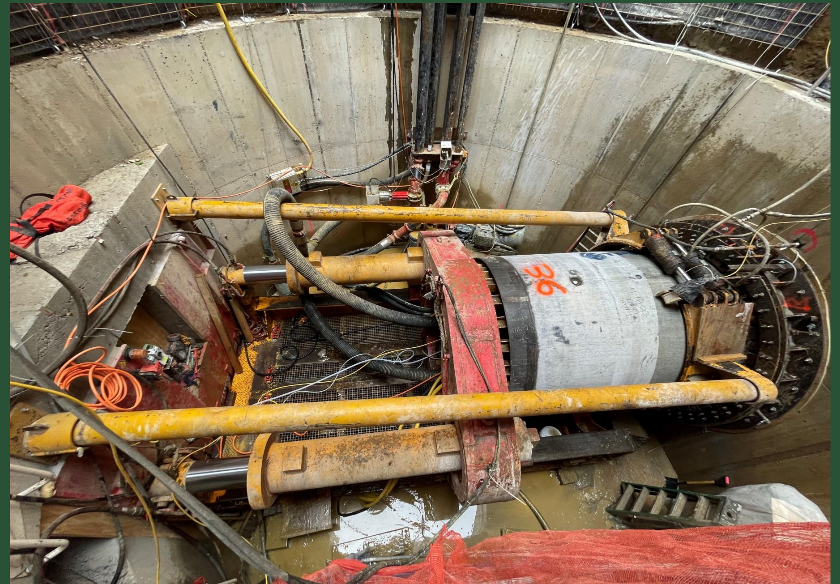
BP5 Microtunneling Activities (May 2023)
