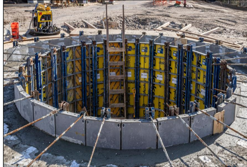
Guide Wall Installation at CC3, January 2022
