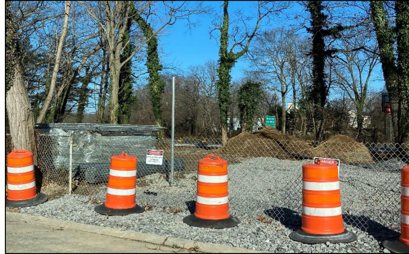
Clearing and Grubbing at CC5, January 2022
