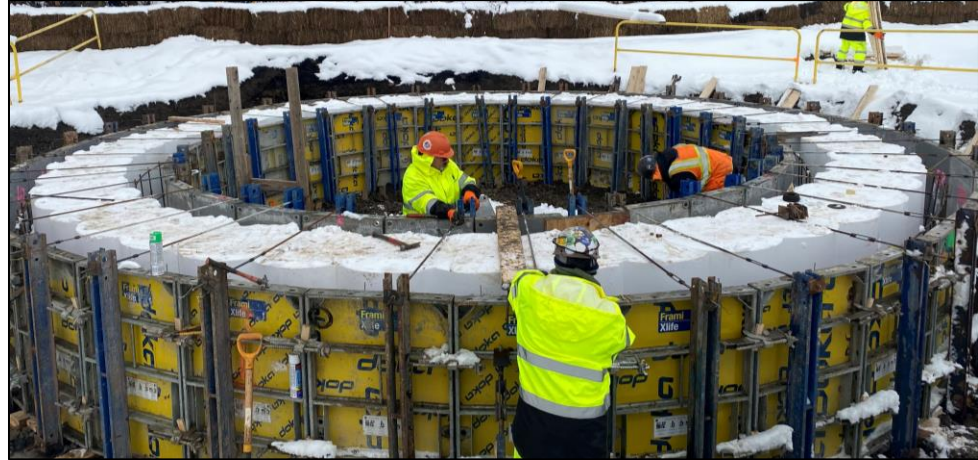
Guide Wall Construction at BP4, January 2022
