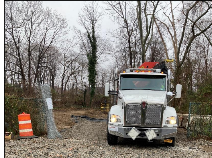
Clearing and Grubbing at CC4, January 2022
