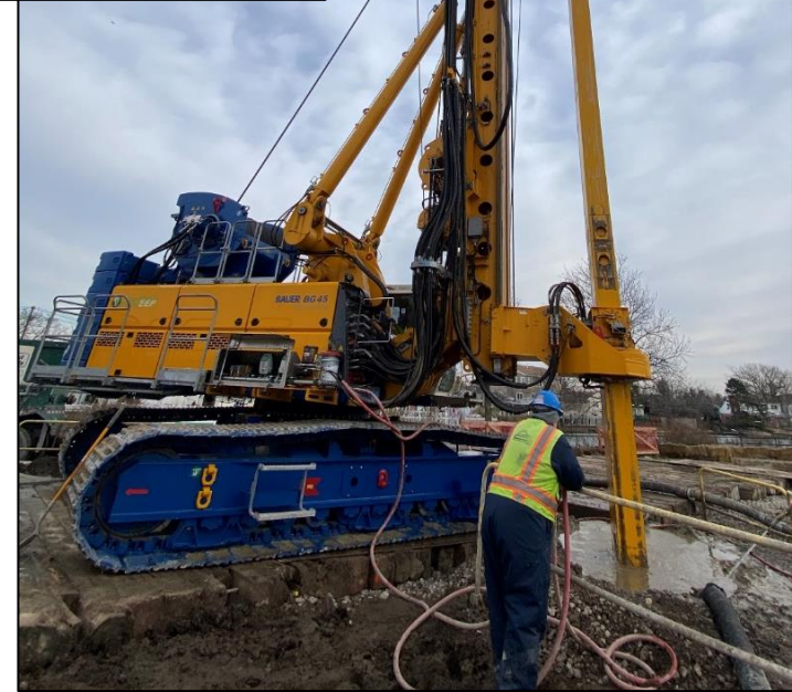
SOE Installation at BP5, December 2021
