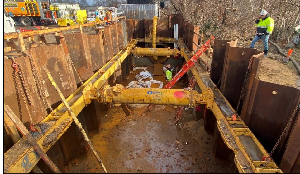
Excavation at Pit O, January 2022
