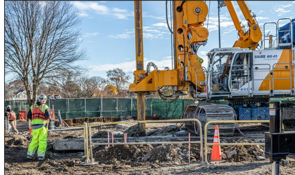
SOE Installation at BP8, December 2021
