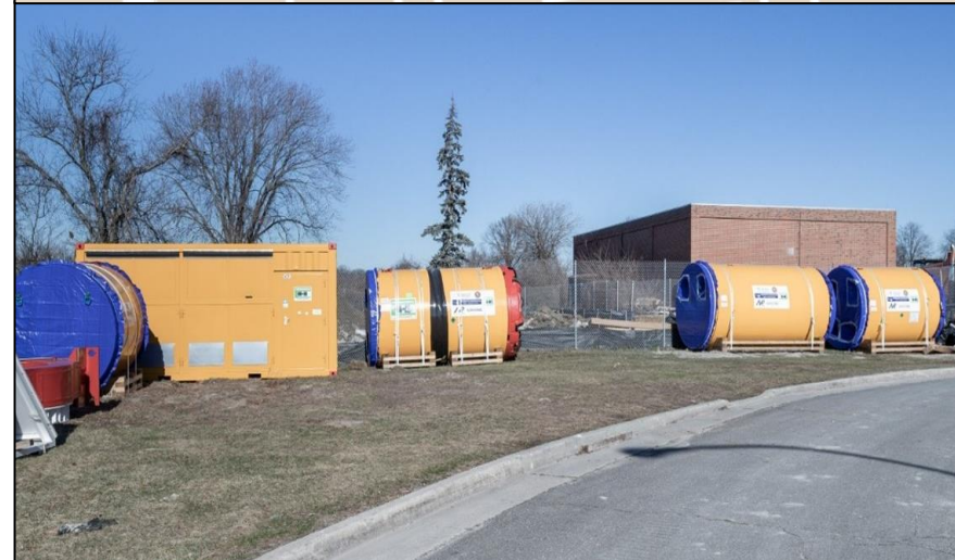
MTBM P.O.S.E.I.D.O.N. Pipe Components at CC2, January 2022
