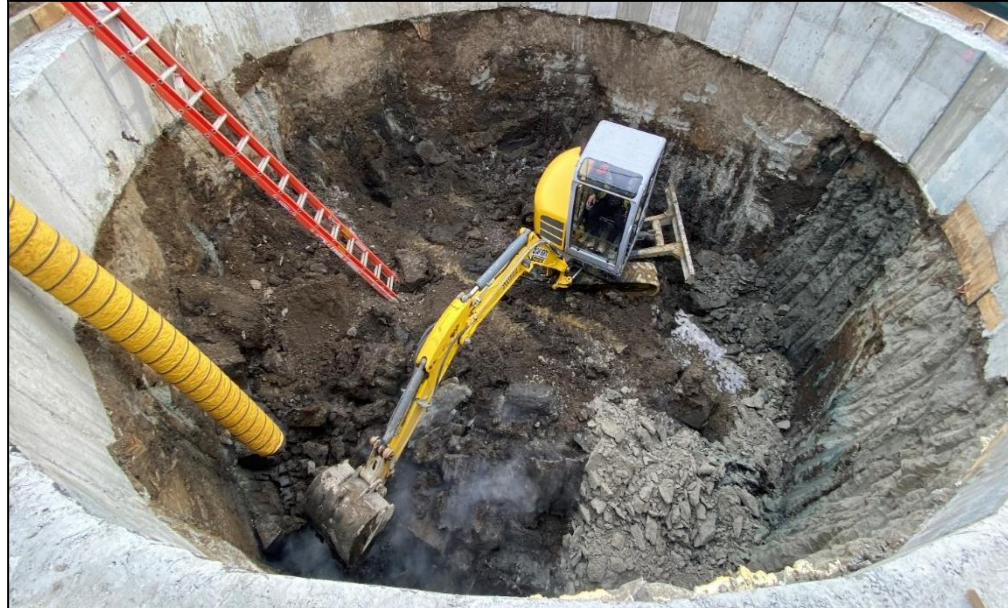
Excavation at BP3, January 2022
