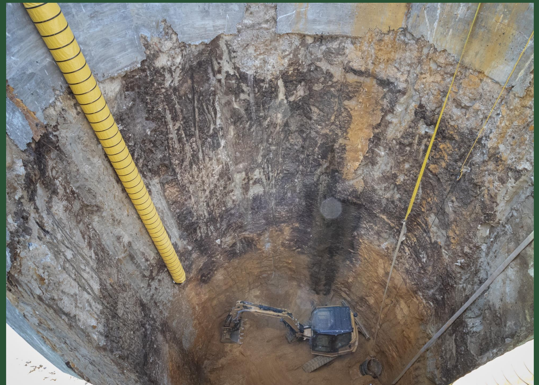
Excavation at BP7 (September 2022)
