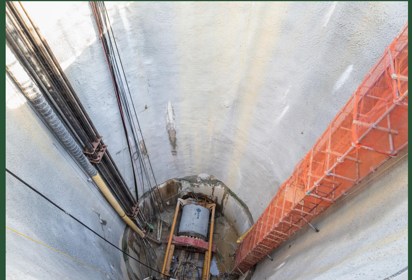
BP2 Microtunnel Operations (September 2022)
