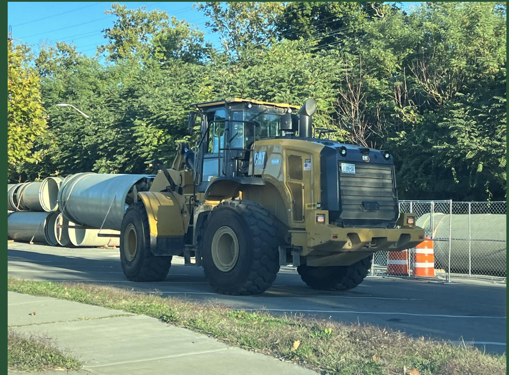
Pipe Storage along Sunrise Highway (September 2022)
