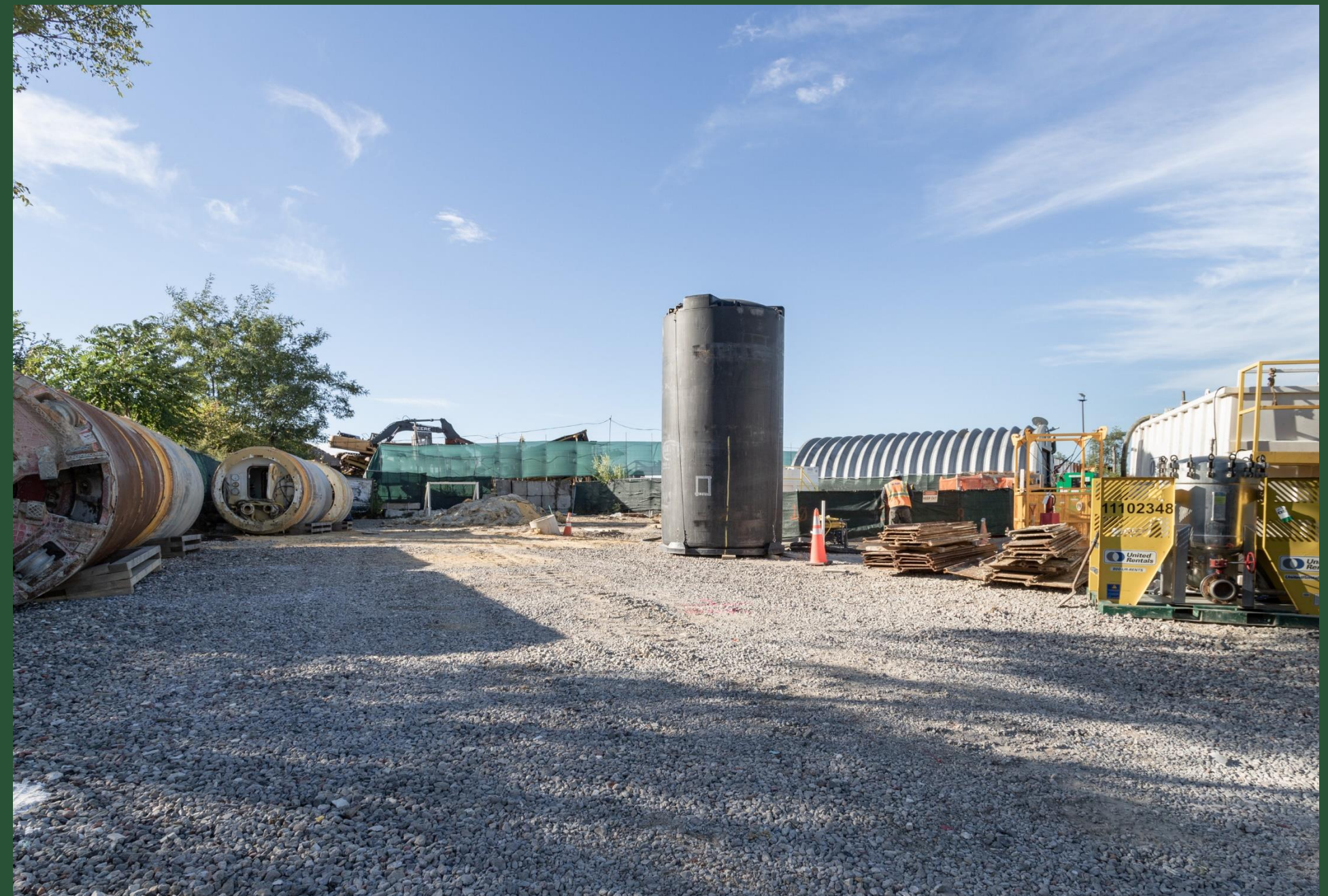
BP3 Construction Site (September 2022)
