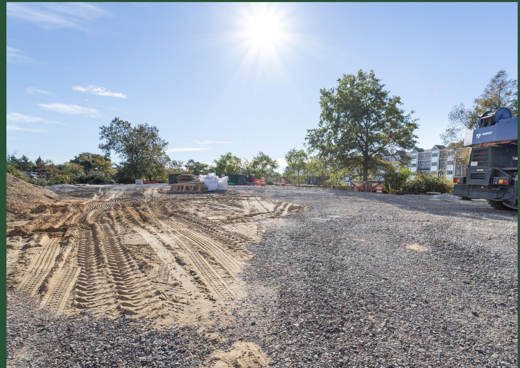
BP5 Construction Site (September 2022)
