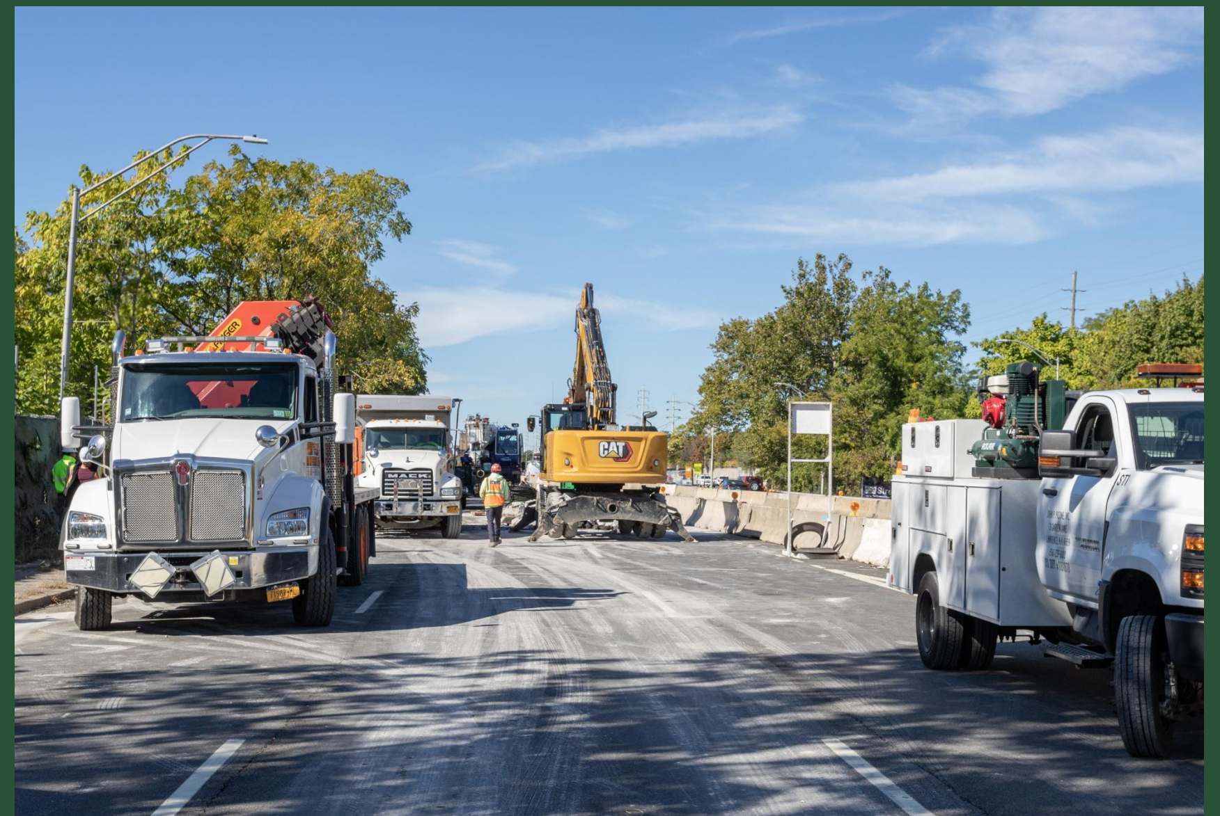
Construction at Pit W (September 2022)
