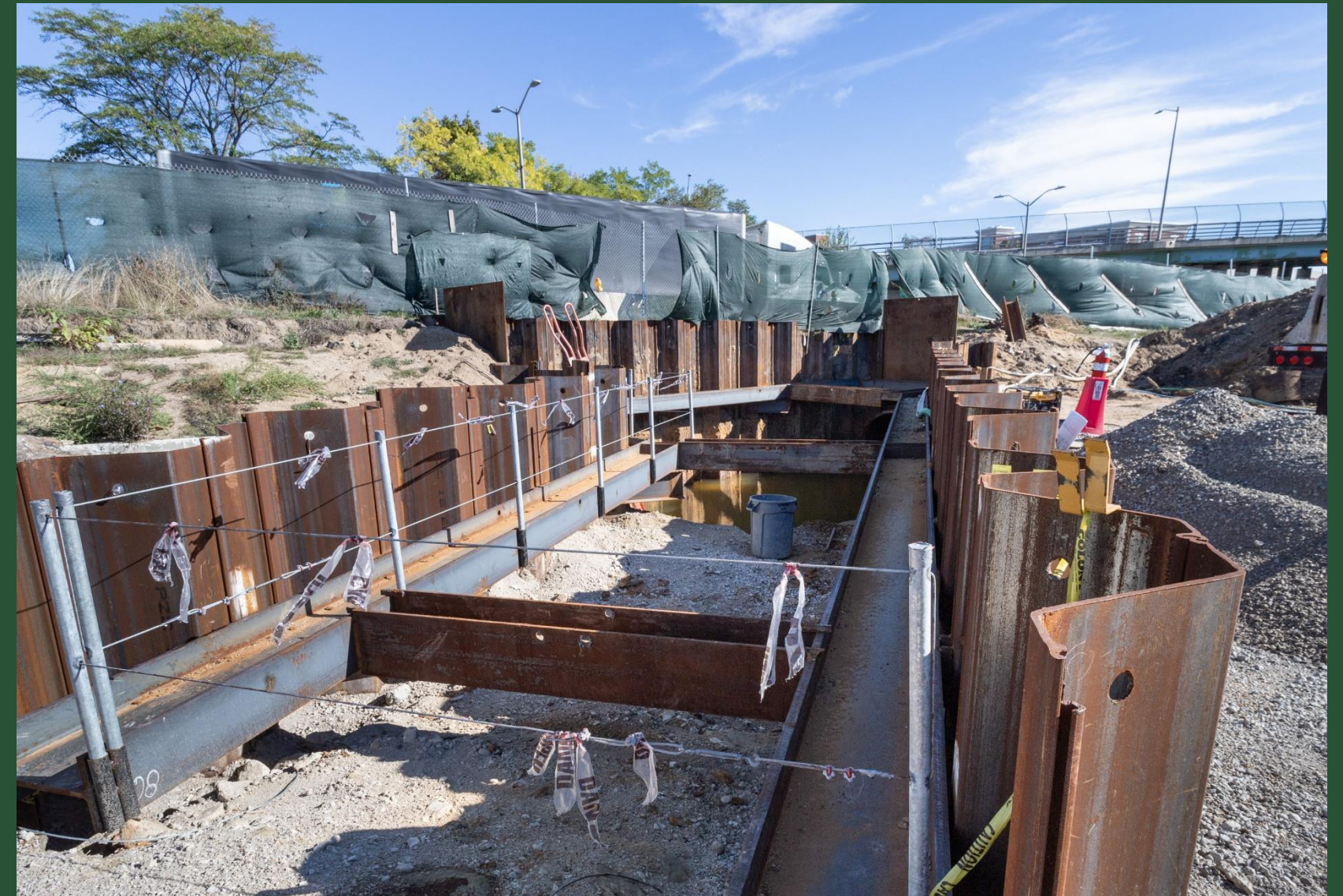
Sheet Pile Installation near BP9 (September 2022)
