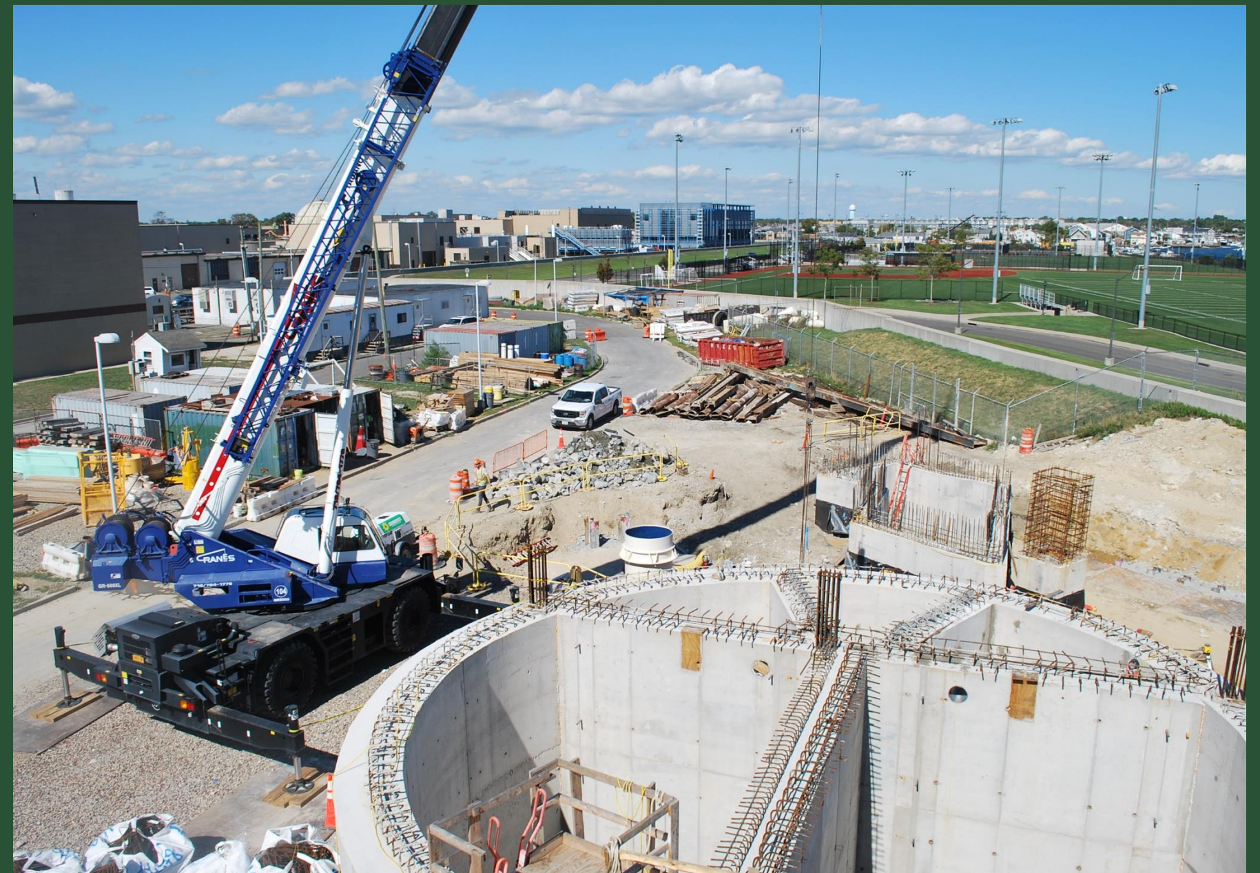
Diversion Structure Construction Near BP1 (September 2022)
