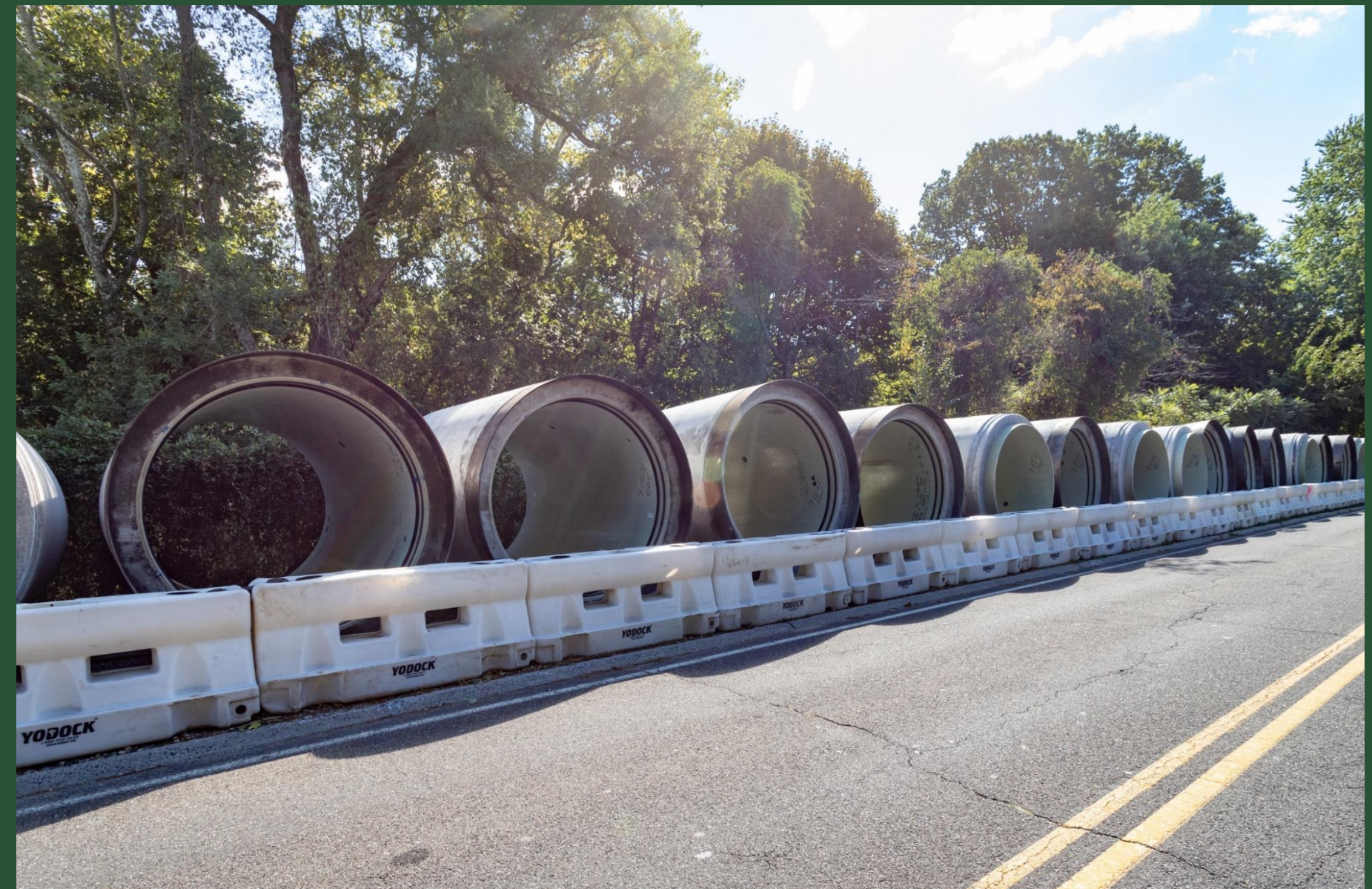
Pipe Storage at CC4 (September 2022)
