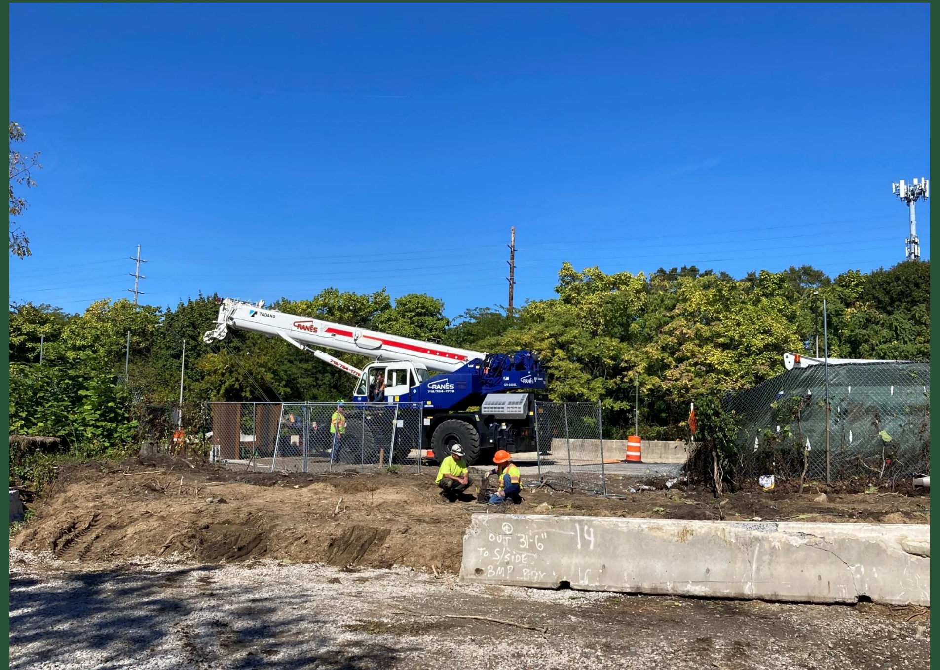
Construction at CC6 (October 2022)
