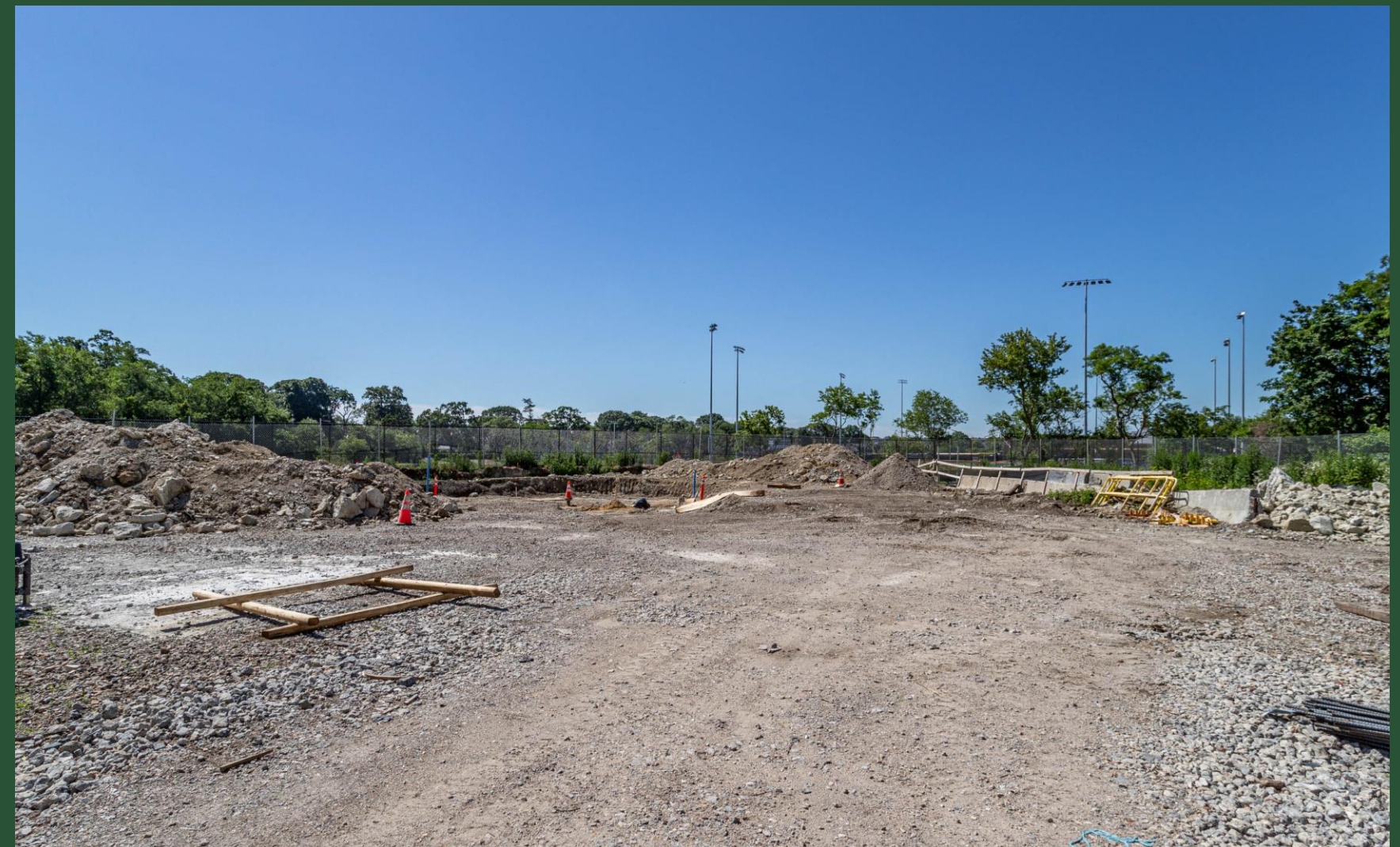
Construction Site at BP7 (May 2022)
