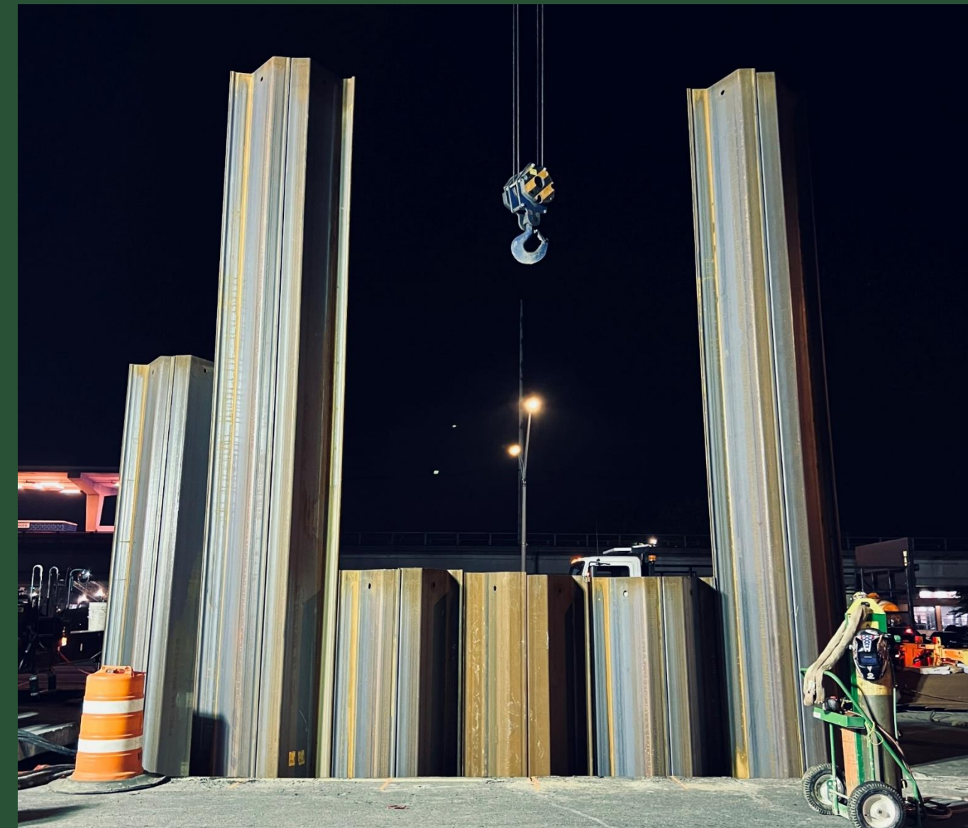
SOE installation at Pit V (June 2022)
