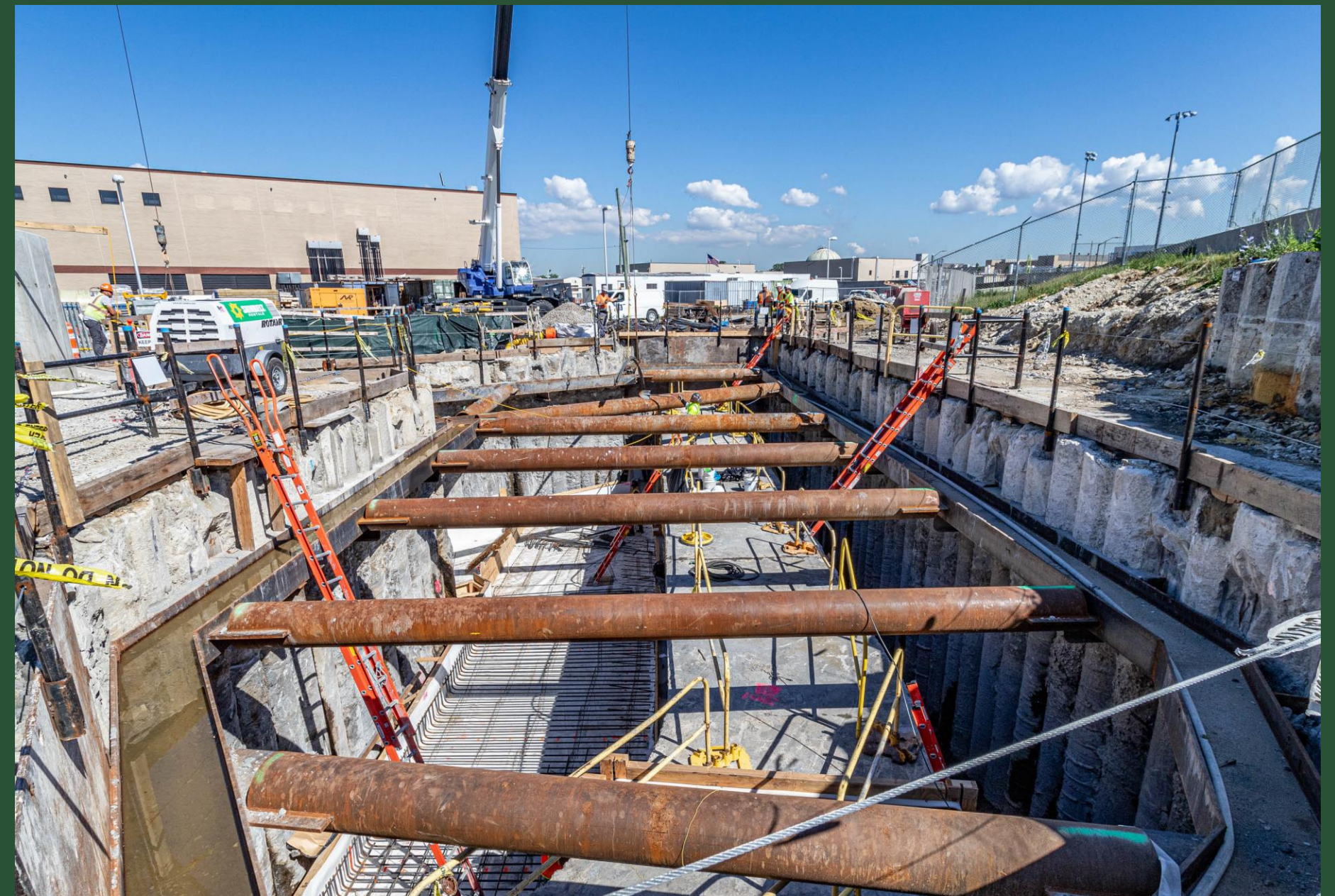
Diversion Structure at BP1 (June 2022)
