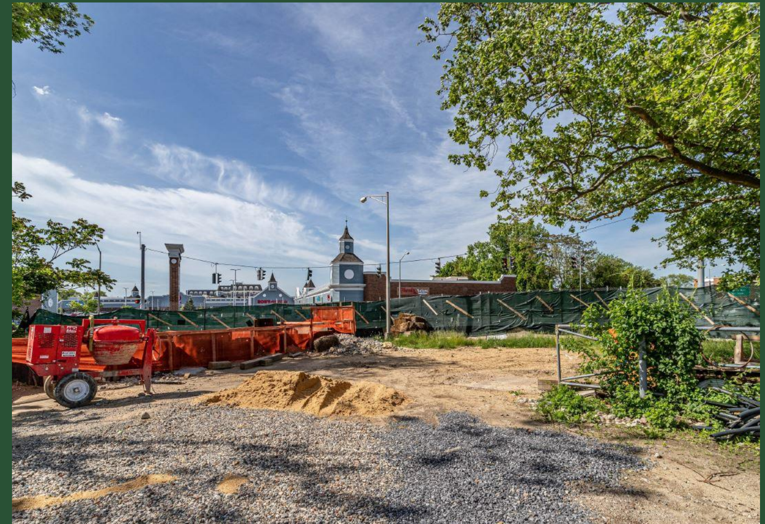
Pit O Construction Site (May 2022)
