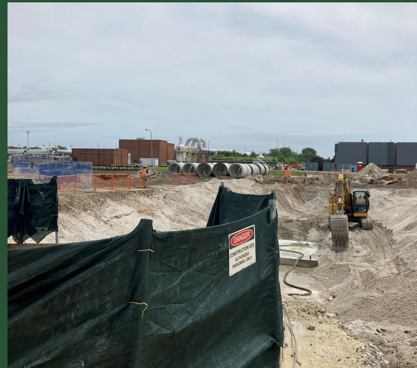
Excavation at CC2 (June 2022)
