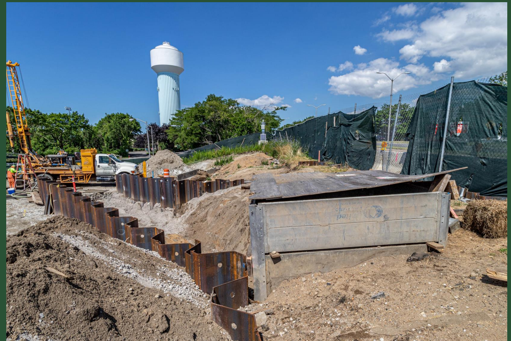
Sheet Installation at Pit A (June 2022)
