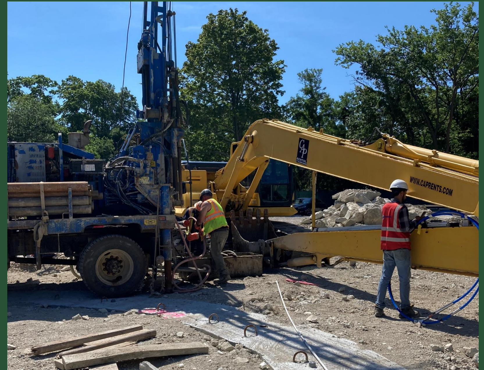
Core Drilling at CC4 (June 2022)
