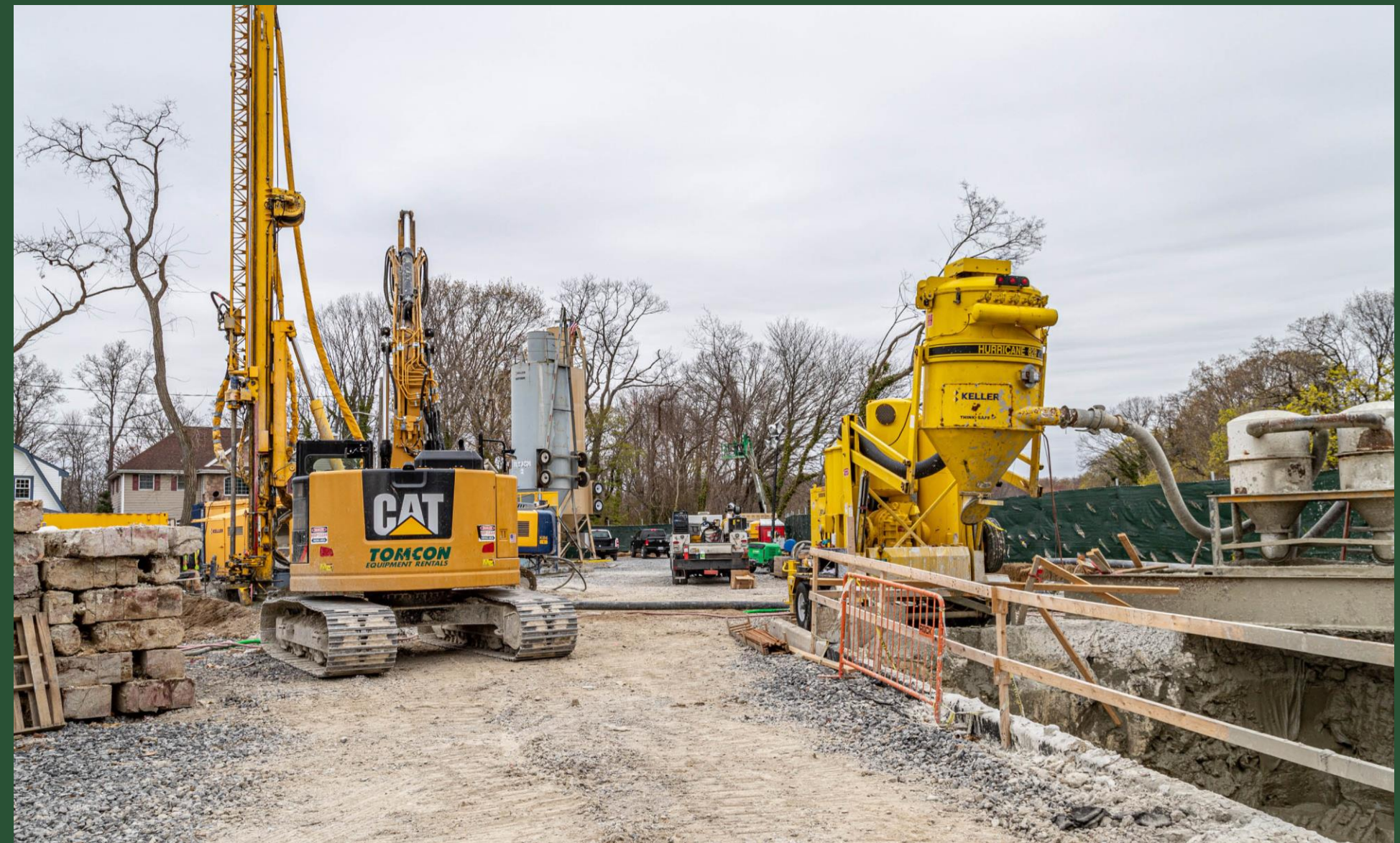
Construction Site at CC5 (April 2022)
