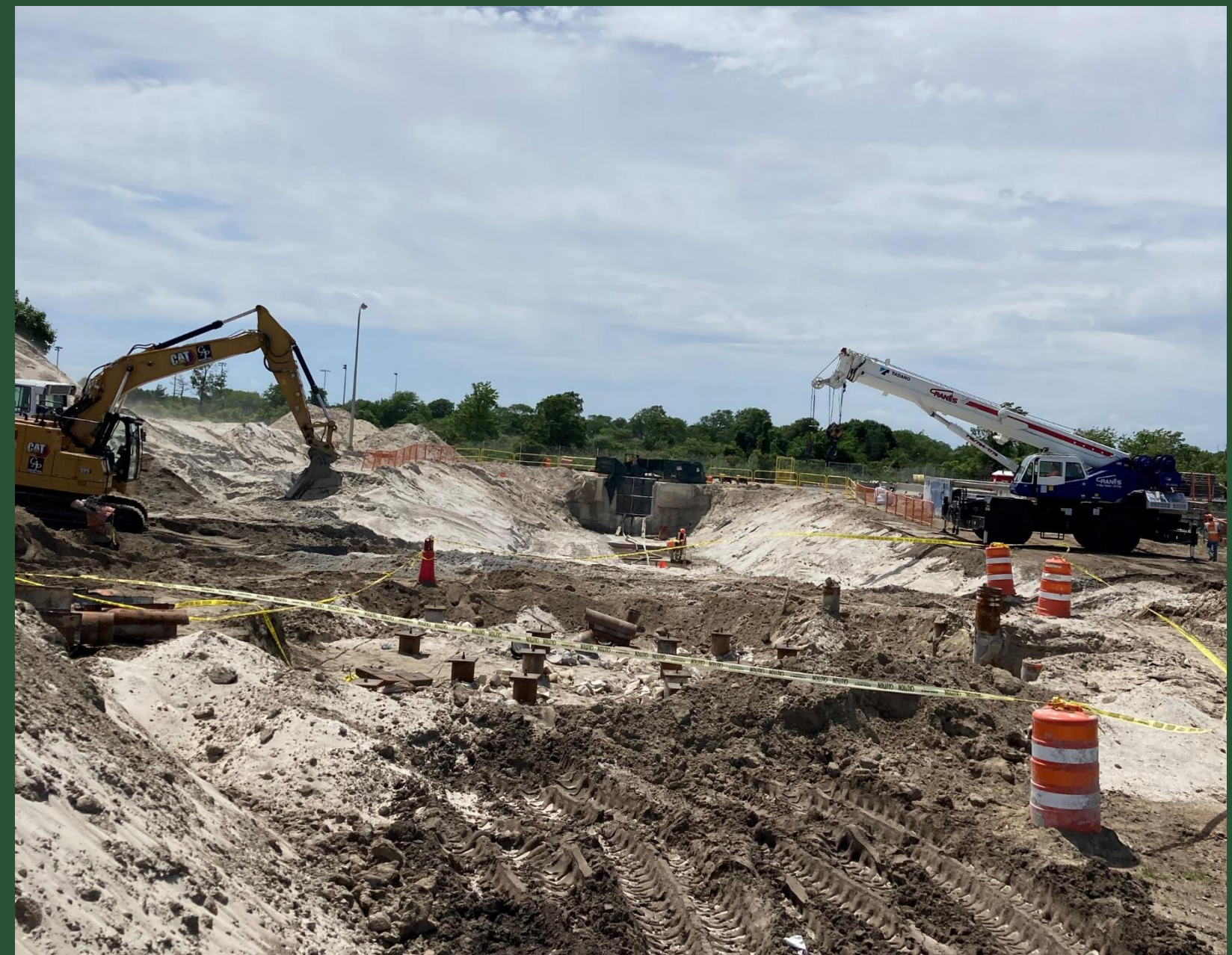
Construction Near CC1 (June 2022)
