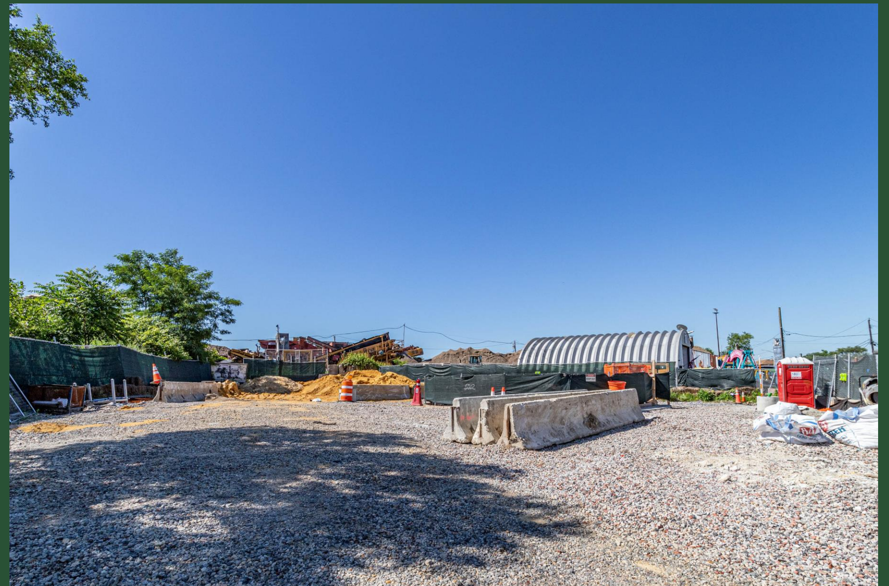
Construction Site at BP3 (June 2022)
