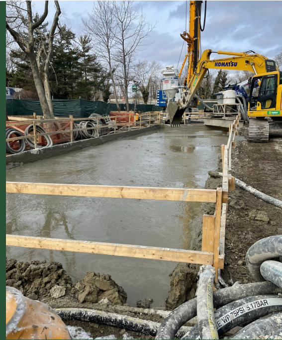
Jet Grout Installation CC4 (February 2022)
