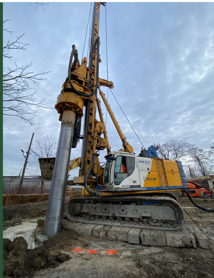
Secant Pile Installation at BP4 (February 2022)
