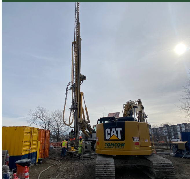
Jet Grout Installation at BP5 (February 2022)
