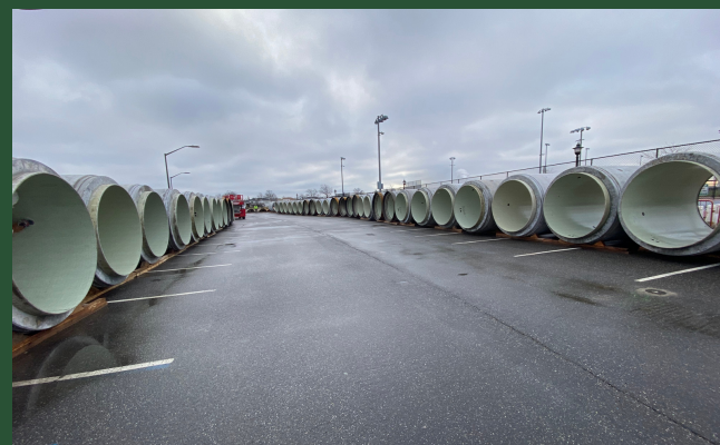
Pipe Laydown at BP2 (February 2022)
