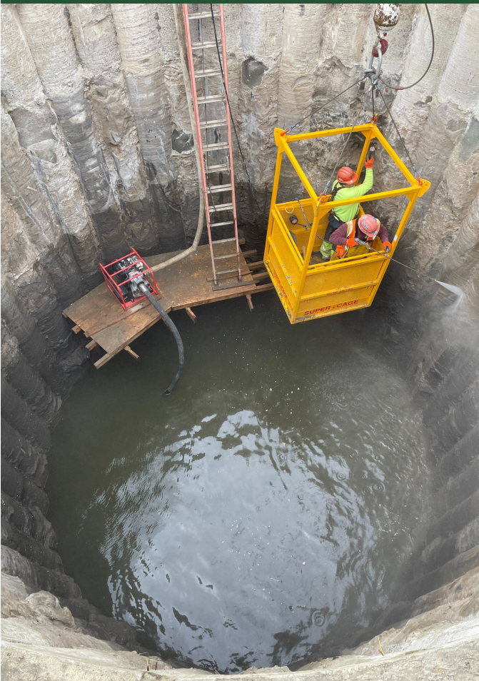
Shaft Excavation at CC1 (February 2022)
