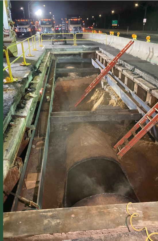
Pit Q on Sunrise Highway Night Work (February 2022)
