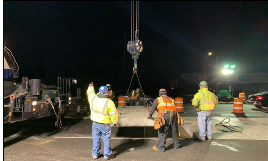
Pit Construction at Pit Q, January 2022
