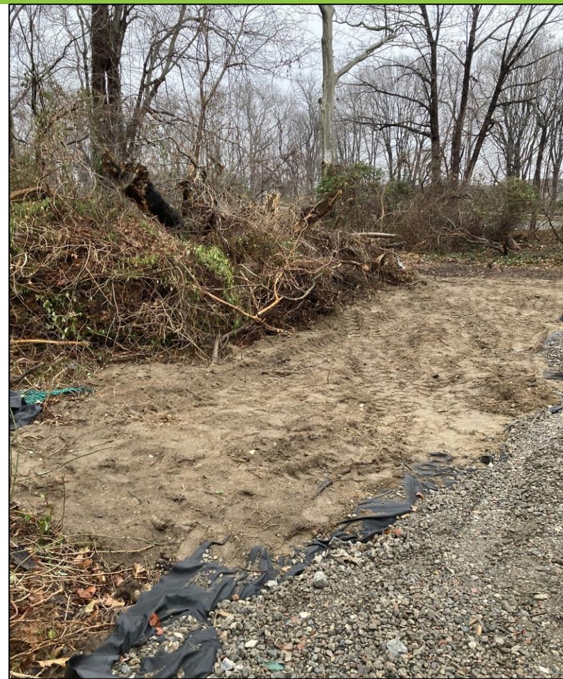
Clearing and Grubbing at CC4, January 2022
