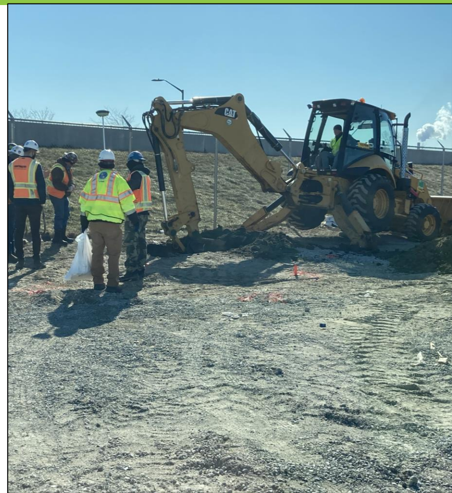
Site Preparation at BP1, March 2021
