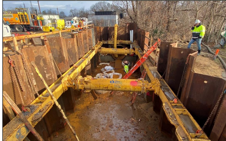
Excavation at Pit O, January 2022
