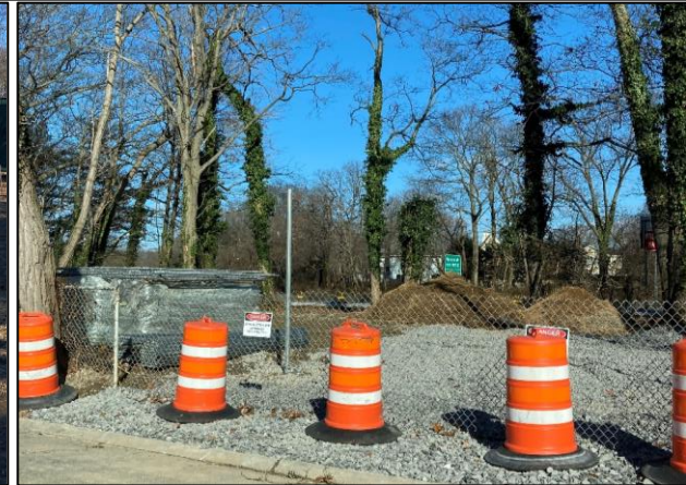
Clearing / Grubbing at CC5, Jan 2022
