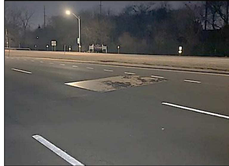
Road Plate Placed at Pit W, February 2022
