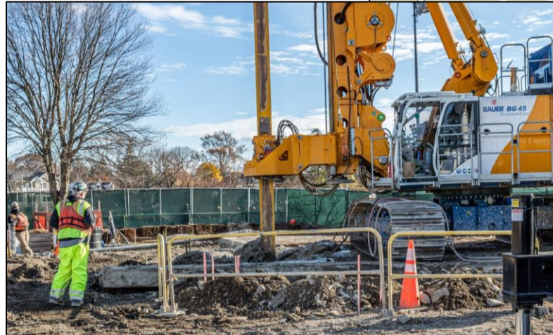
SOE Installation at BP8, December 2021
