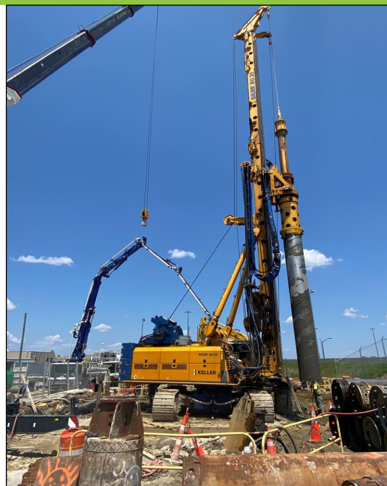
CSM Panel Installation at BP1, November 2021
