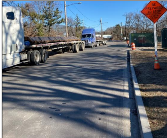
Construction Entrance at CC6, Feb 2022
