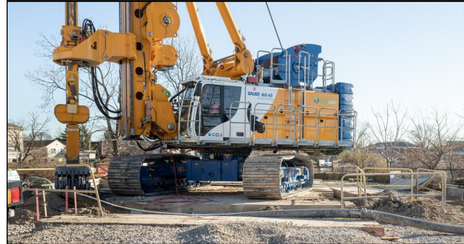
BP5 Jet Grout Installation, January 2022
