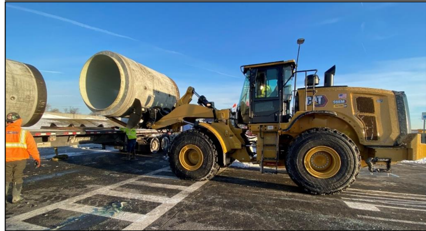
Microtunnel Pipe Delivery at BP2, January 2022
