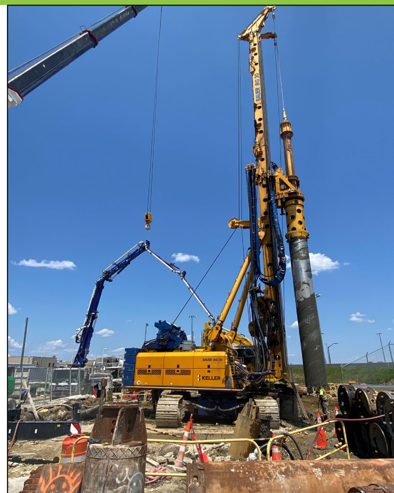
CSM Panel Installation at BP1, November 2021
