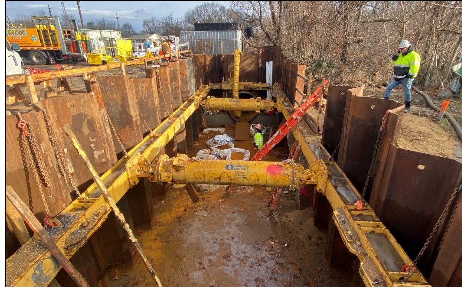
Excavation at Pit O, January 2022
