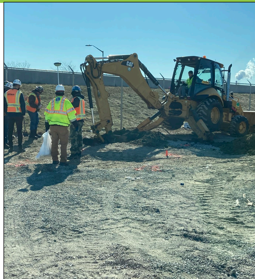
Site Preparation at BP1, March 2021
