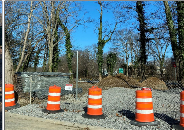
Clearing / Grubbing at CC5, Jan 2022
