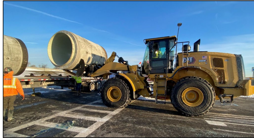
Microtunnel Pipe Delivery at BP2, January 2022
