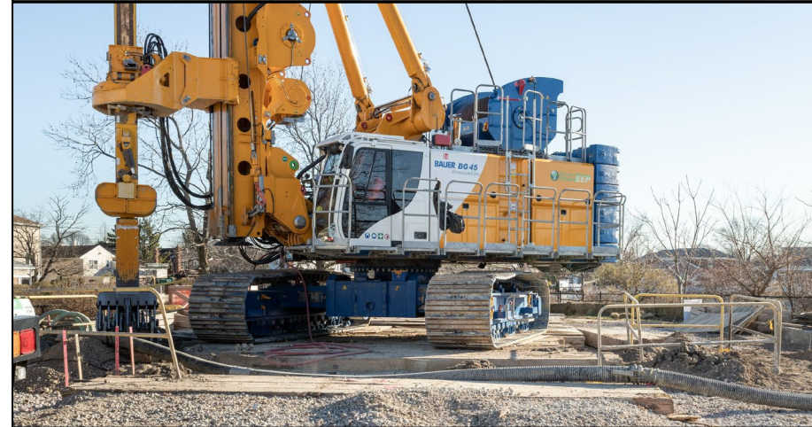
BP5 Jet Grout Installation, January 2022
