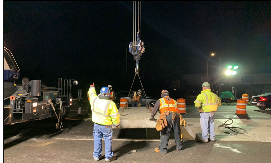
Pit Construction at Pit Q, January 2022
