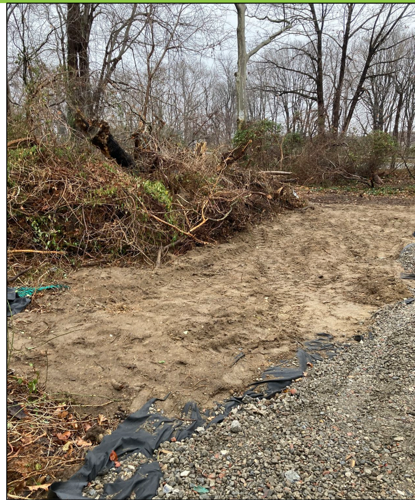
Clearing and Grubbing at CC4, January 2022
