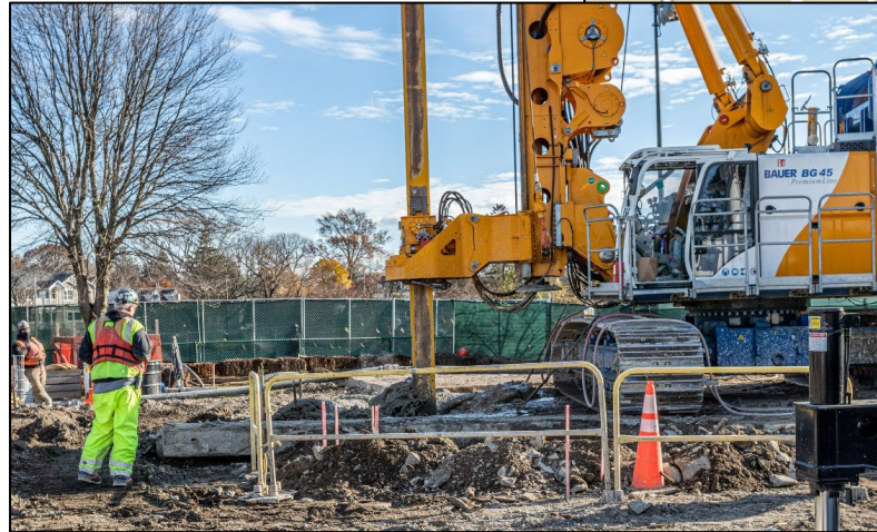
SOE Installation at BP8, December 2021
