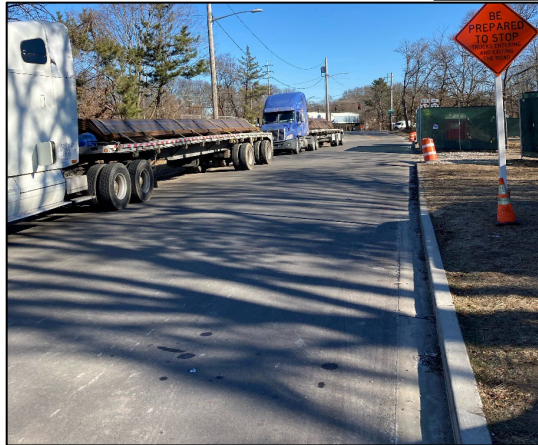
Construction Entrance at CC6, Feb 2022
