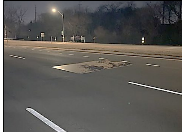
Road Plate Placed at Pit W, February 2022
