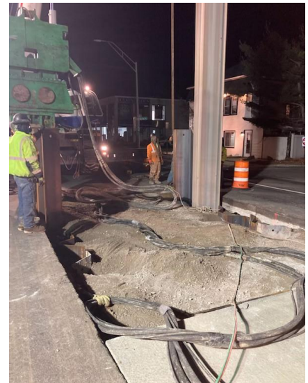
Sheet Pile Installation at Pit R on Sunrise Highway
