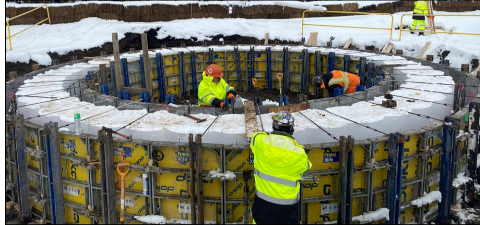
Guide Wall Construction at BP4, January 2022
