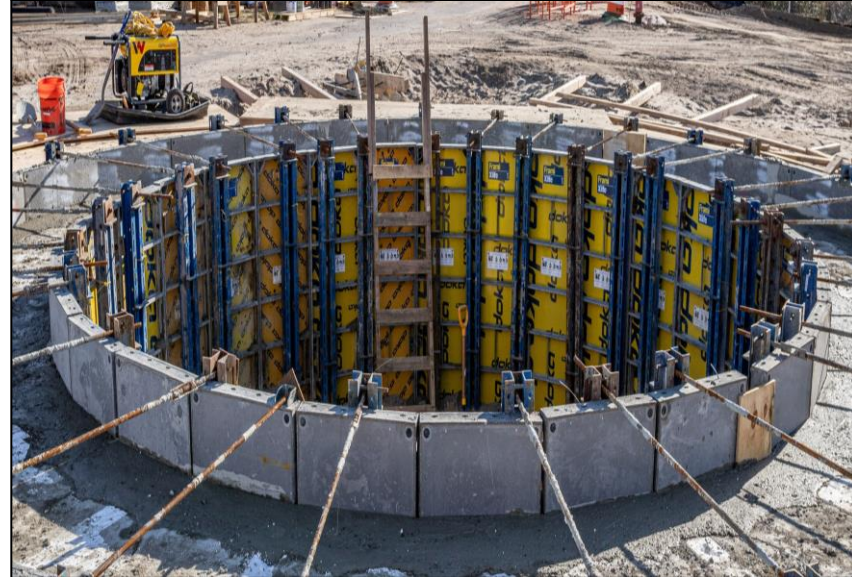
Guide Wall Installation at CC3, January 2022
