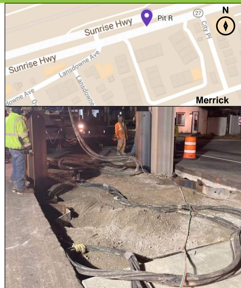
Installation of Sheet Piles at Pit R, February 2022
