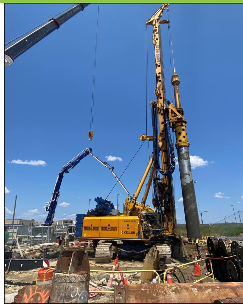
SOE Installation at BP1, November 2021
