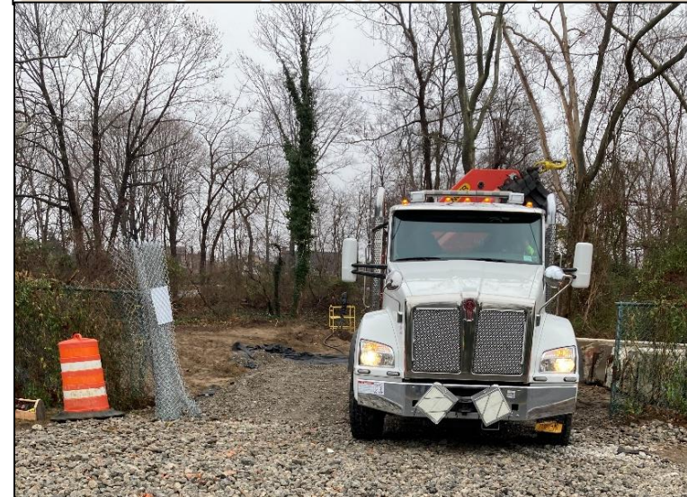
Clearing and Grubbing at CC4, January 2022
