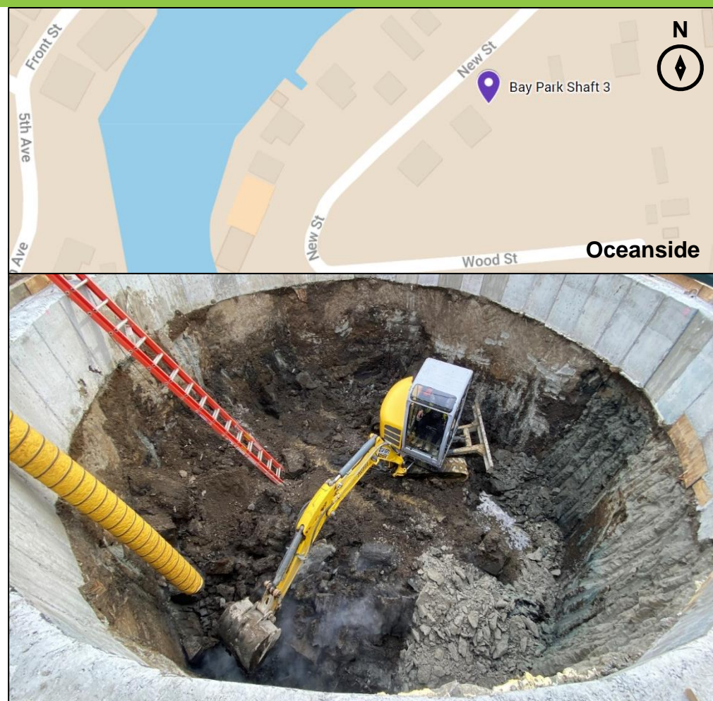
Excavation at BP3, January 2022
