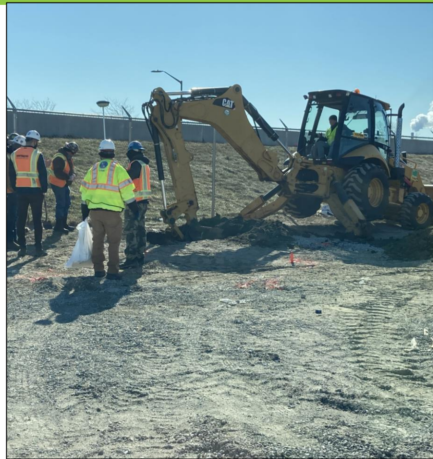
Site Preparation at BP1, March 2021
