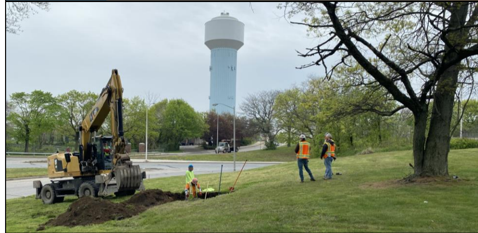
Site Prep at BP9, April 2021
