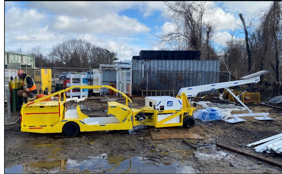
Sliplining Equipment at Pit O, January 2022
