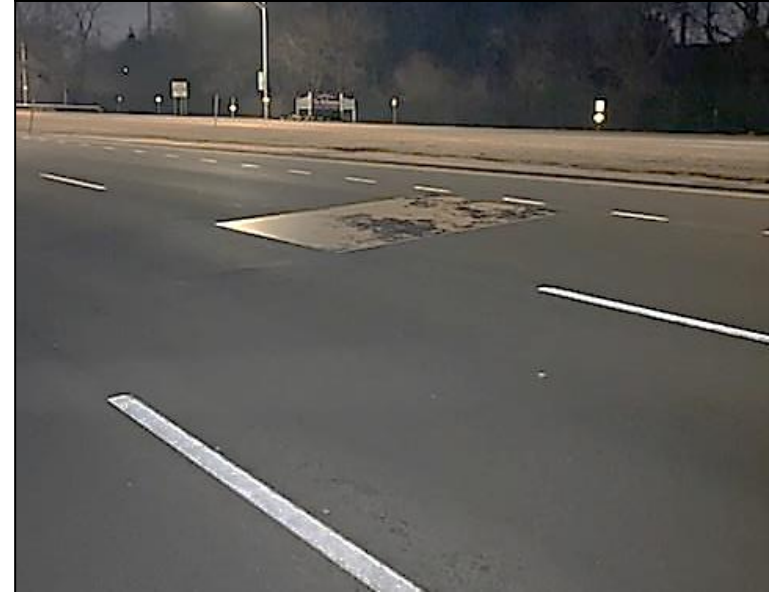
Road Plate Placed at Pit W, February 2022
