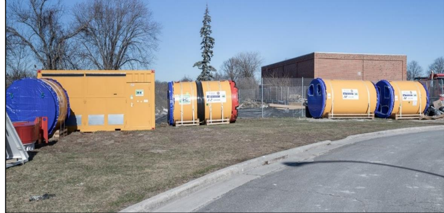
MTBM P.O.S.E.I.D.O.N. Pipe Components at CC2, January 2022
