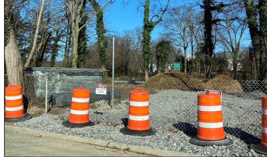
Clearing and Grubbing at CC5, January 2022
