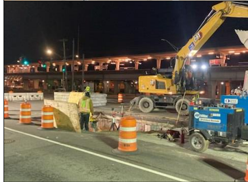
Ongoing Construction at Pit S, February 2022
