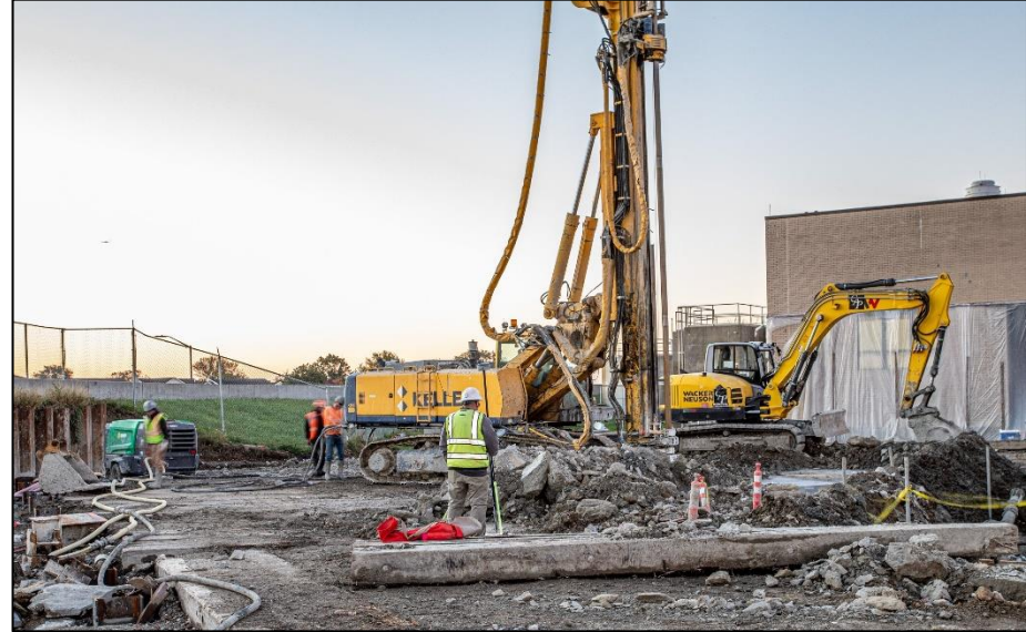
Jet Grout Installation at BP1, November 2021
