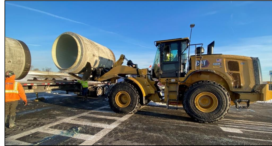
Microtunnel Pipe Delivery at BP2, January 2022
