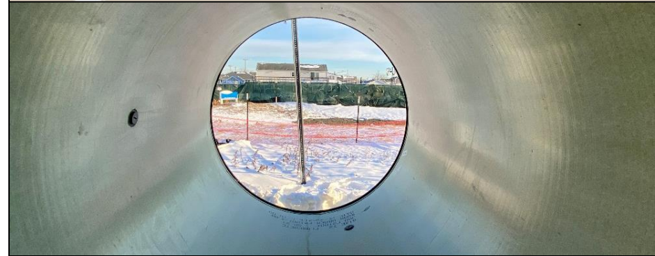
A Look Inside Microtunneling Pipe, January 2022
