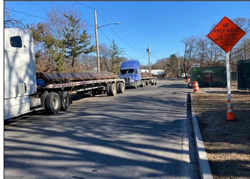
Construction Entrance at CC6, February 2022
