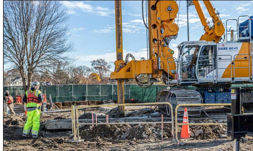
SOE Installation at BP8, December 2021
