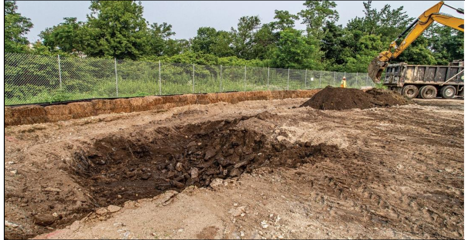
Spoils Pit and Erosion Control at BP7, July 2021
