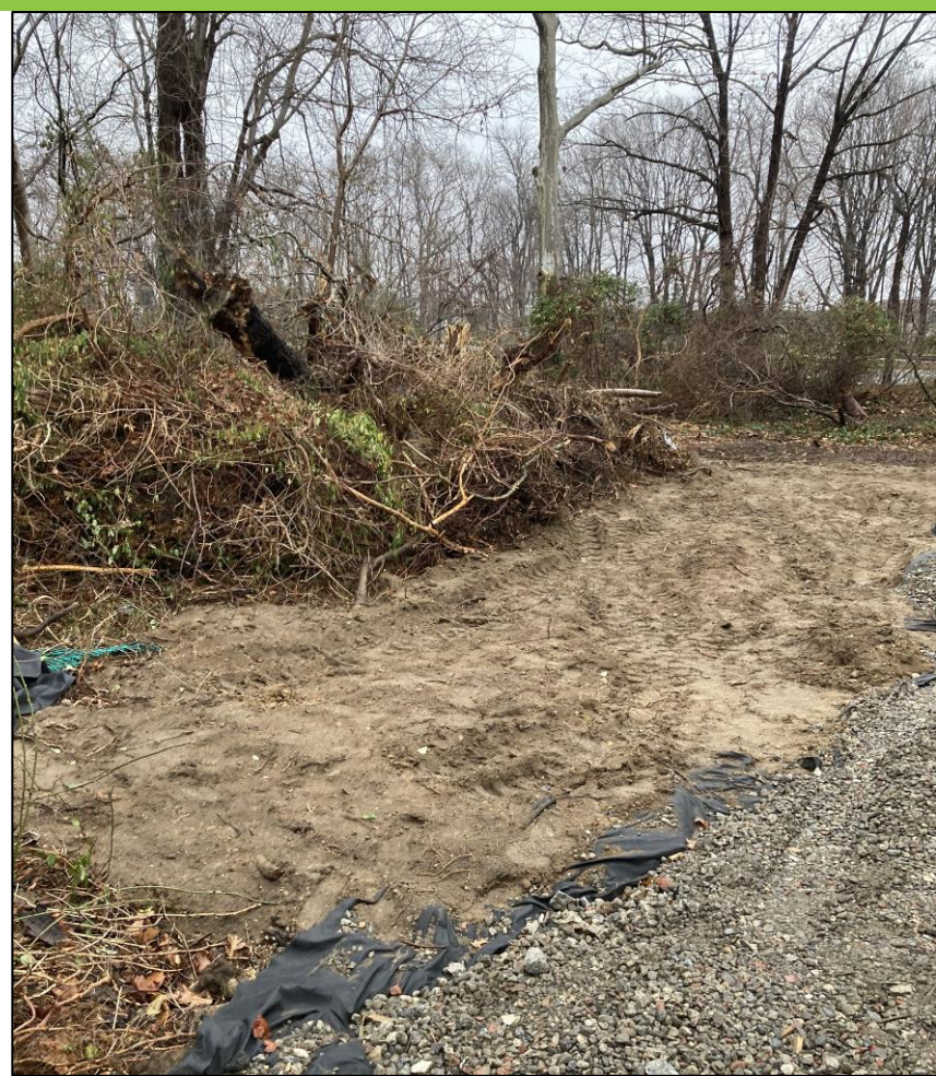
Clearing and Grubbing at CC4, January 2022
