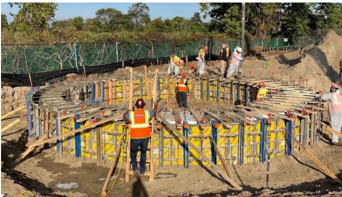
Guidewall installation at Cedar Creek Shaft 2
