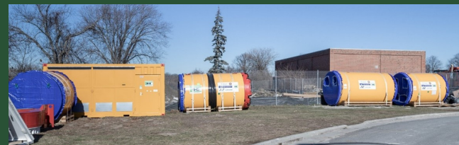
Cedar Creek Shaft 2 MTBM P.O.S.E.I.D.O.N. (January 2022)
