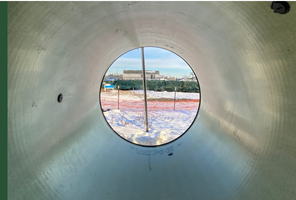
An Inside Look at a Microtunnel Pipe (January 2022)
