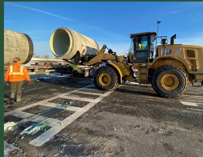
Bay Park Shaft 2 Microtunnel Pipe Delivery (January 2022)
