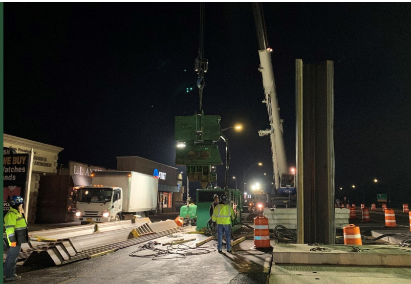
Sunrise Highway Pit Q Night Work (January 2022)
