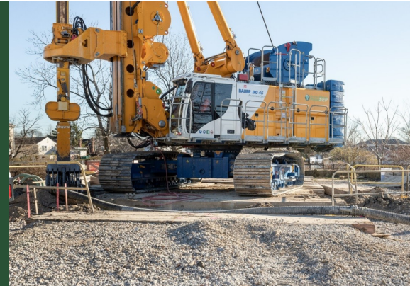
Bay Park Shaft 5 Jet Grout Installation (January 2022)
