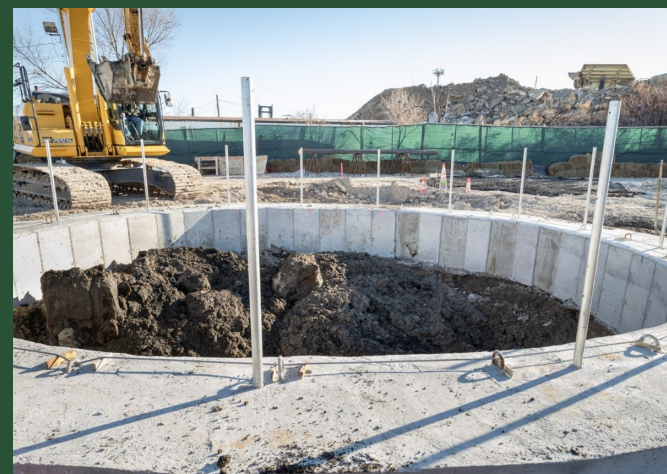
Bay Park Shaft 3 Site Work (January 2022)
