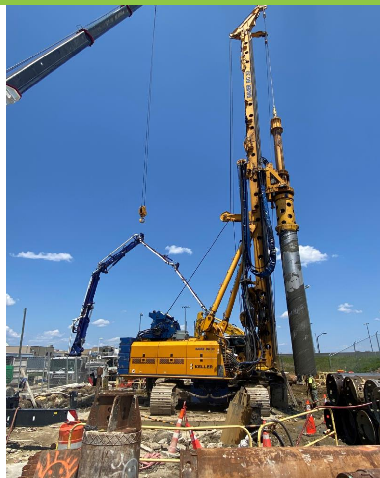
CSM Panel Installation at BP1, November 2021
