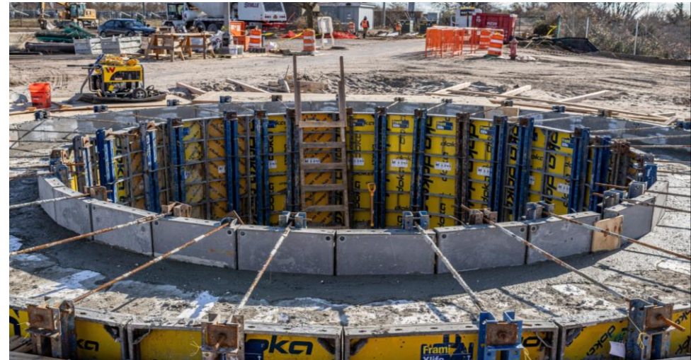
Guide Wall Installation at CC3, December 2021
