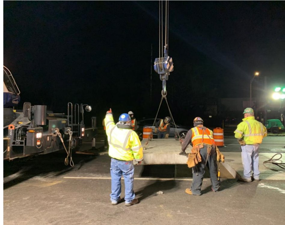
Pit Construction at Pit Q, January 2022
