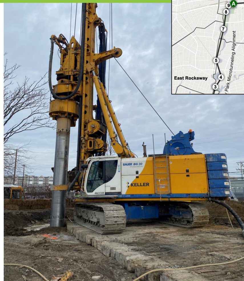
Secant Pile Installation at BP4, January 2022
