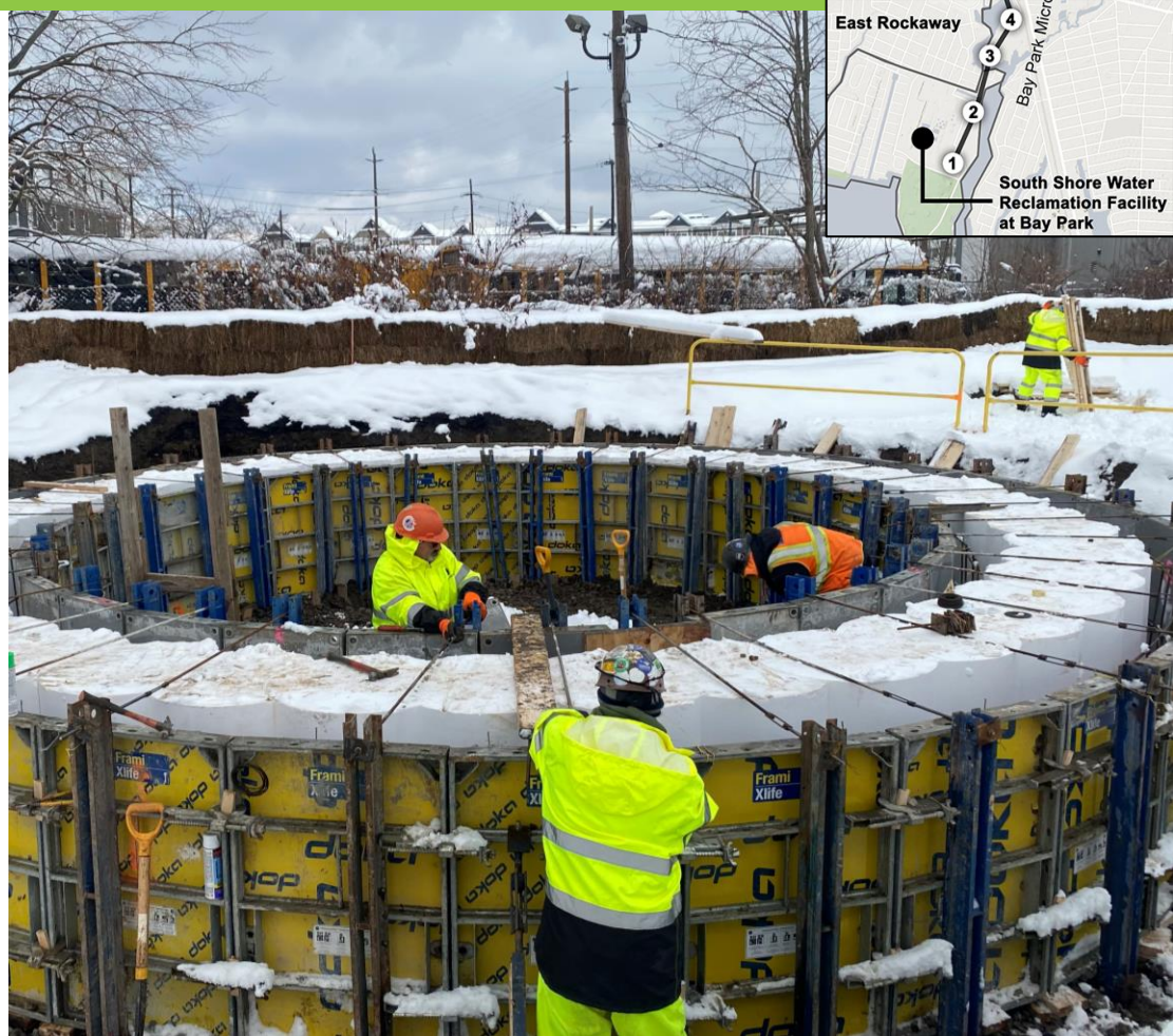
Guide Wall Construction at BP4, January 2022
