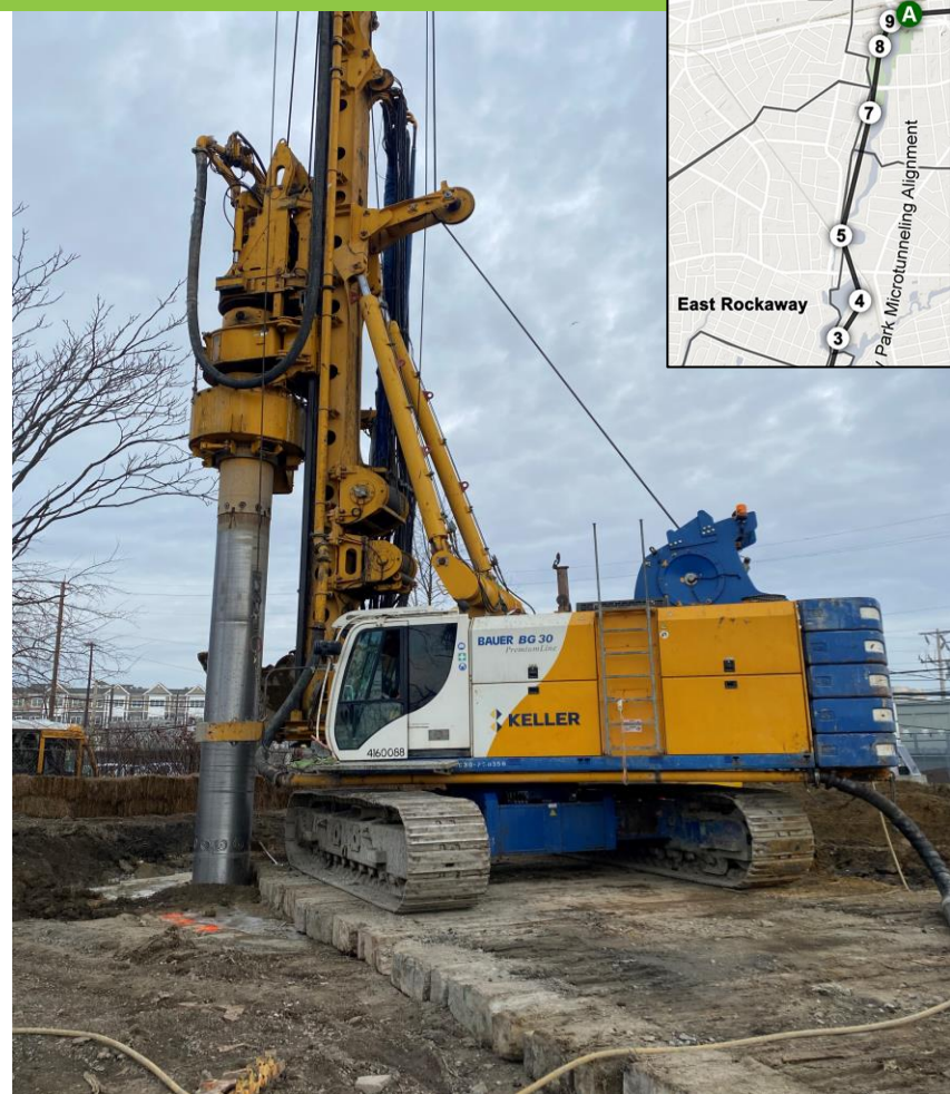
Secant Pile Installation at BP4, January 2022
