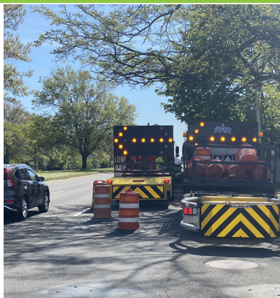
MPT deployed at Pit F on Sunrise Highway, May 2021
