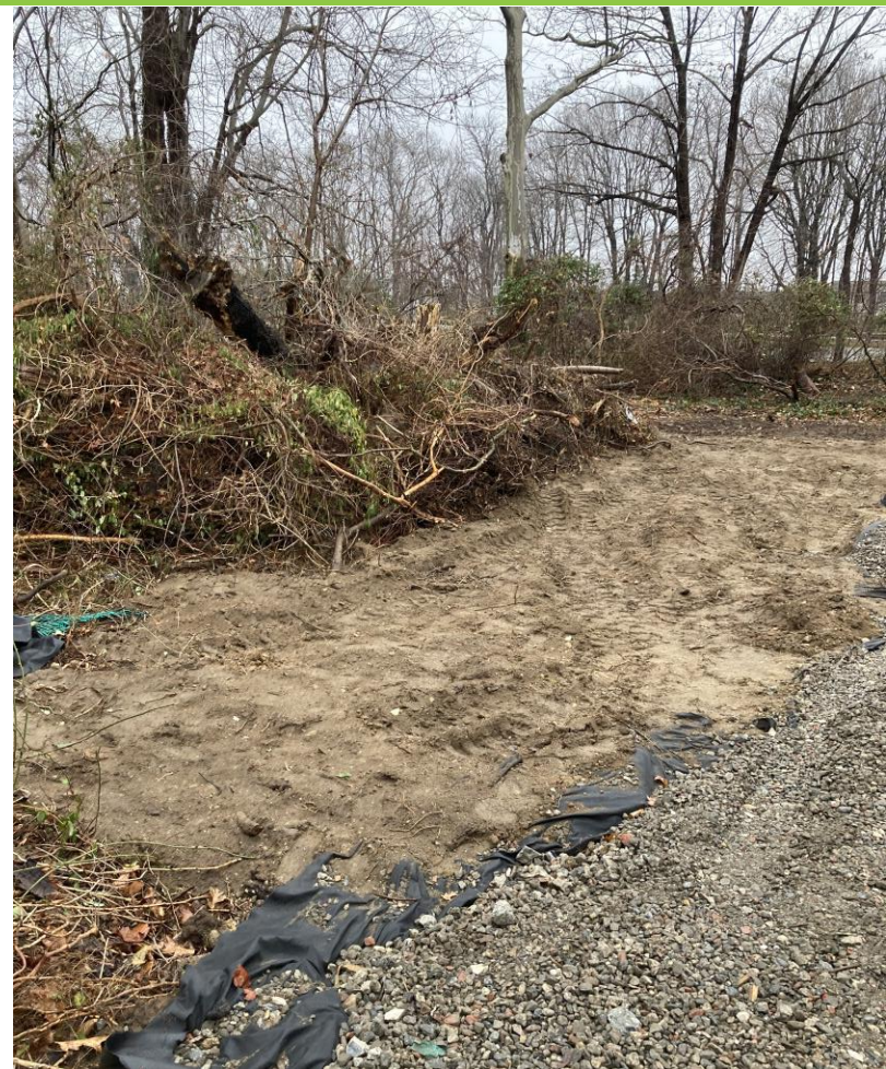
Clearing and Grubbing at CC4, January 2022
