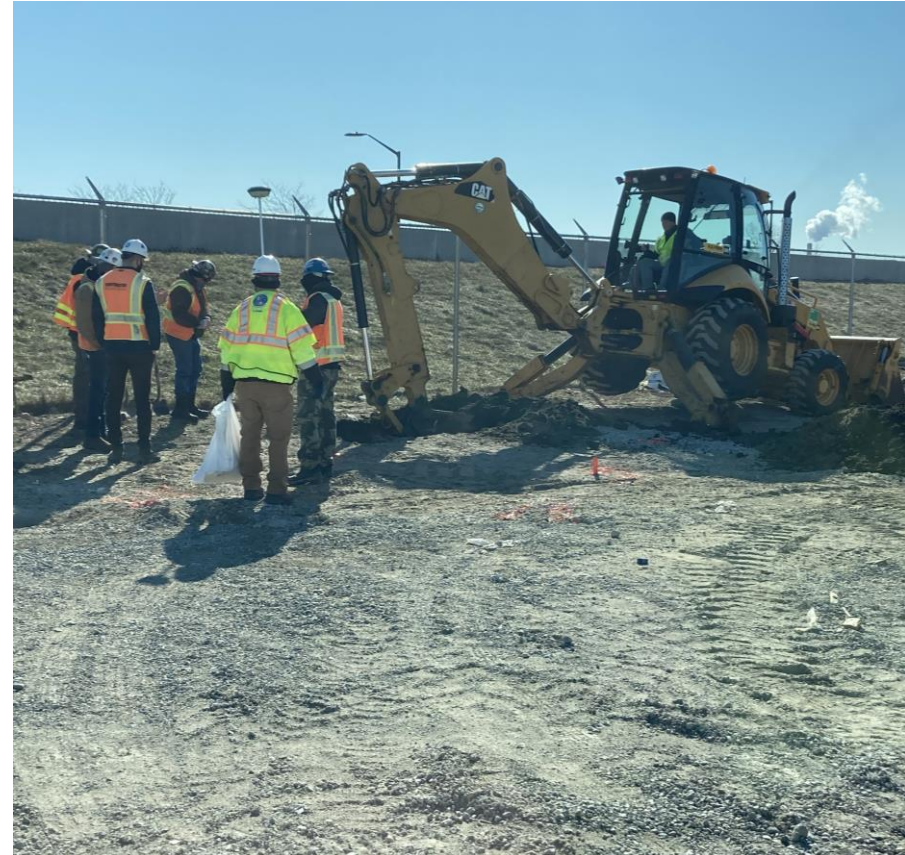
Site Preparation at BP1, March 2021
