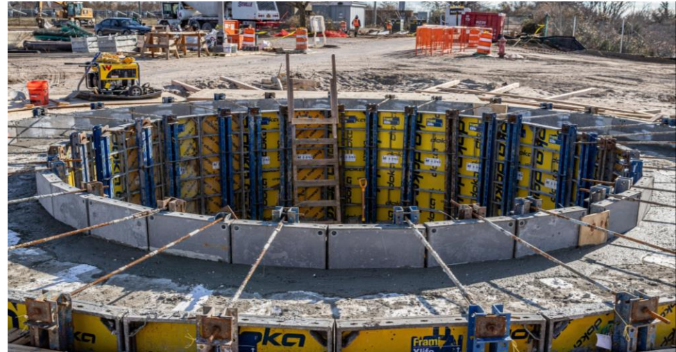
Guide Wall Installation at CC3, December 2021
