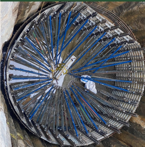
Bay Park Shaft 1: 15 Feet High Concrete Liner (December 2021)
