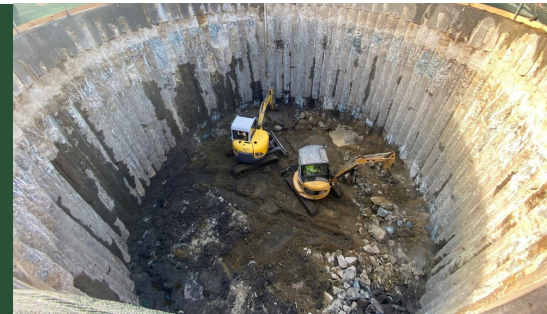
Bay Park Shaft 1: Excavating Wet Well for New Pump Station (December 2021)
