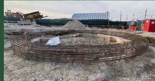
Bay Park Shaft 3: Rebar Ring Beam (December 2021)
