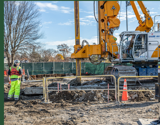
Bay Park Shaft 8: SOE Installation (December 2021)
