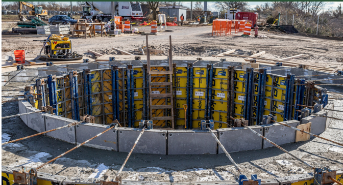
Cedar Creek Shaft 3: Guide Wall Construction (December 2021)
