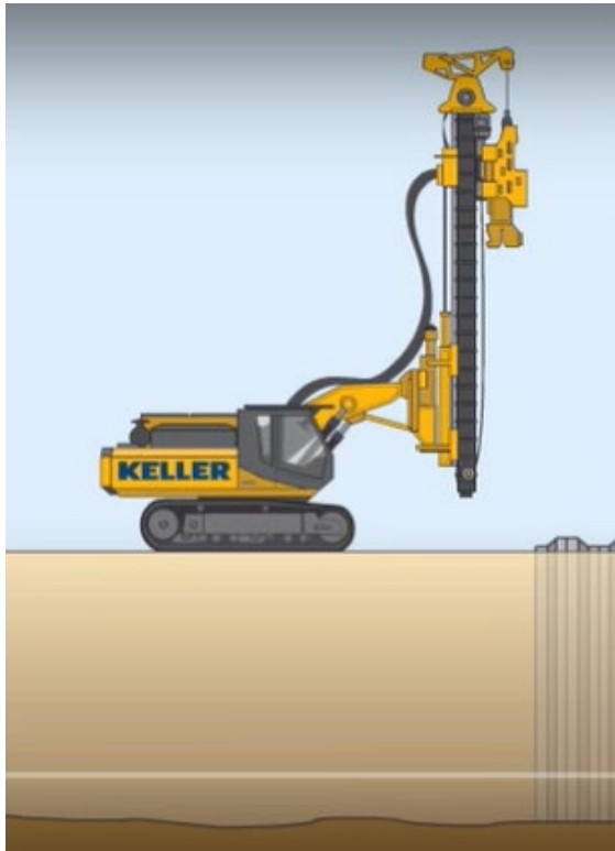
Animation of Sheet Pile Installation Credit: Keller North America
