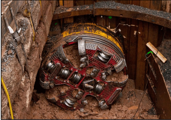
Microtunnel Boring Machine
