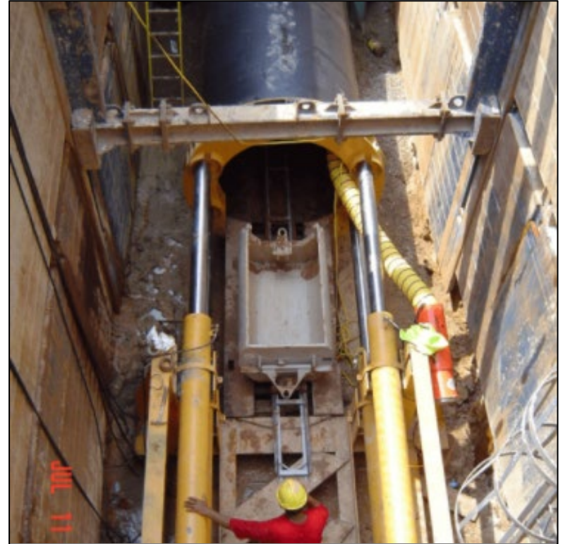
Sliplining Pipe and Pit
