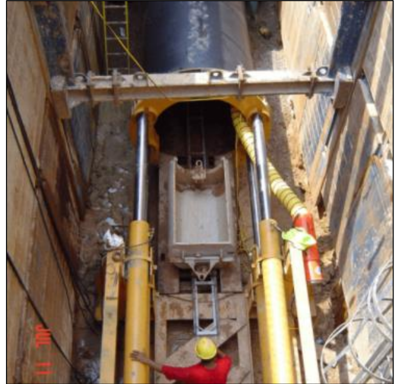
Sliplining Pipe and Pit
