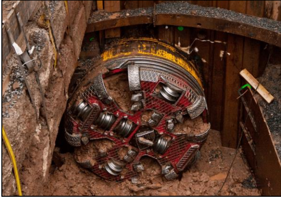
Microtunnel Boring Machine
