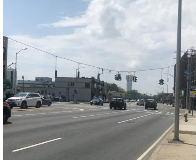
Work Pits constructed along Sunrise Highway
