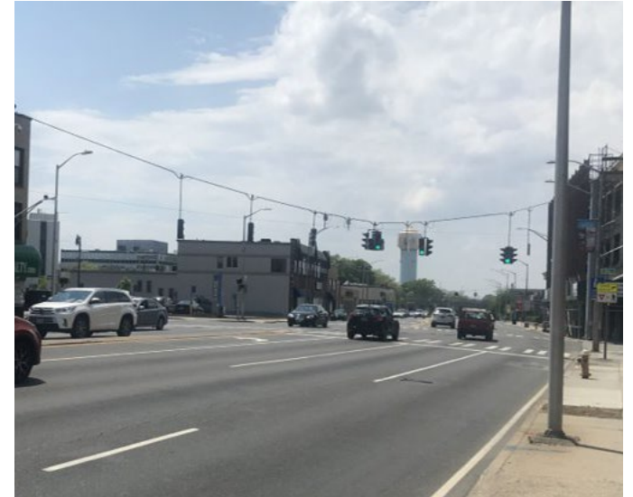
Work Pits constructed along Sunrise Highway
