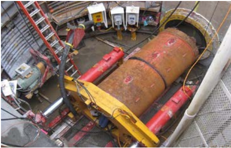
Example of tunneling in progress
