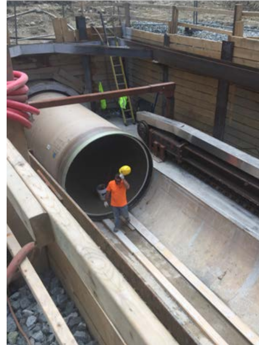
Example of sliplining in progress
