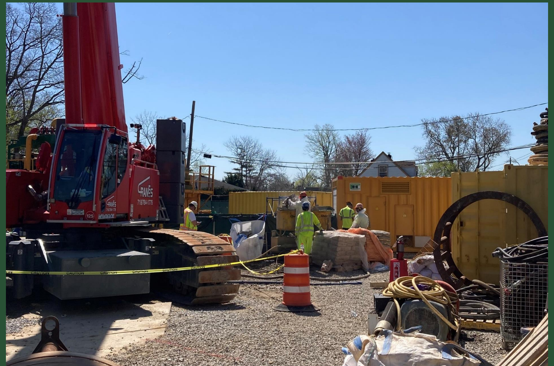
Grouting Activities at CC5 (April 2023)
