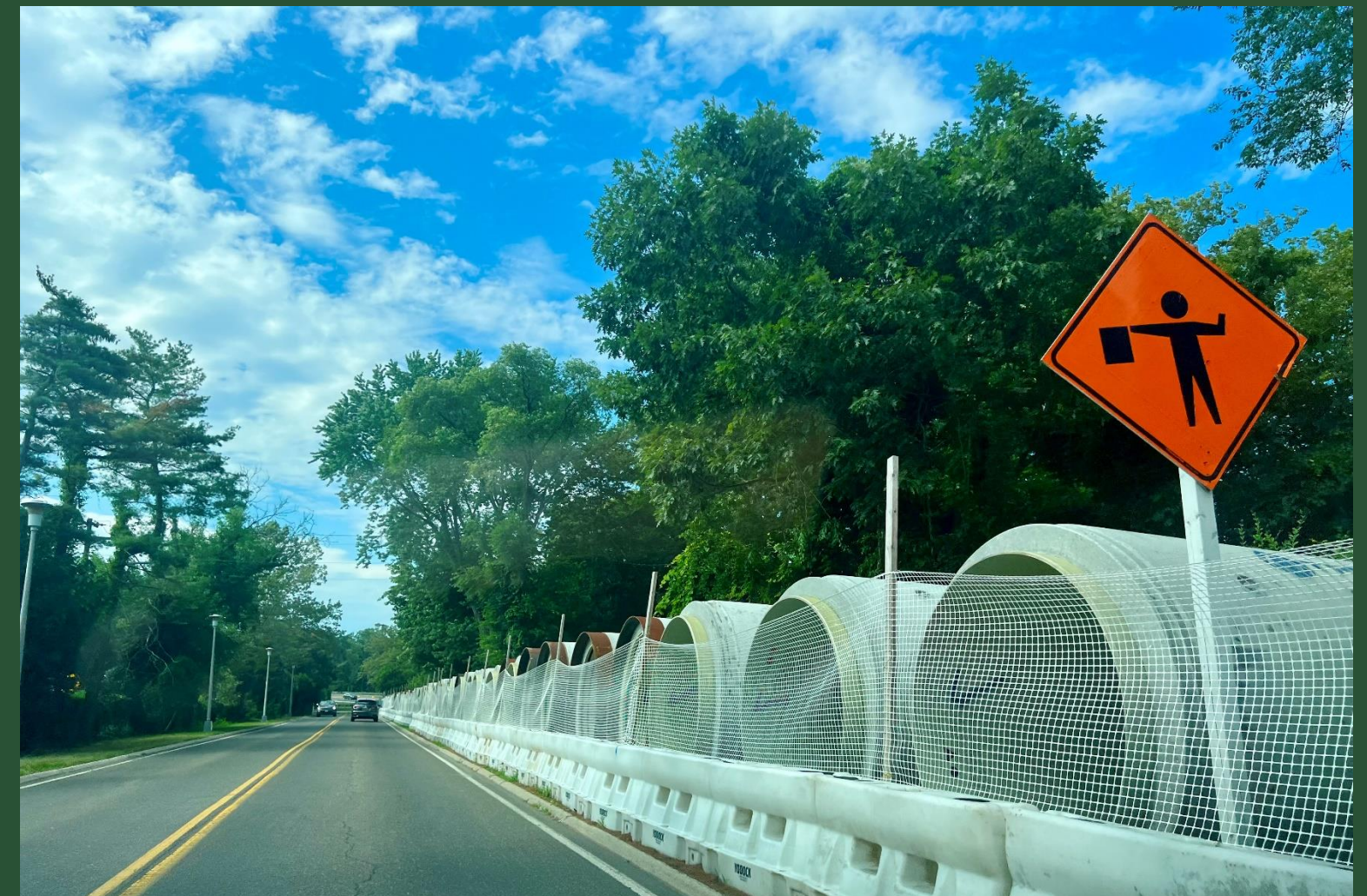
Pipe Storage near CC4 (July 2023)
