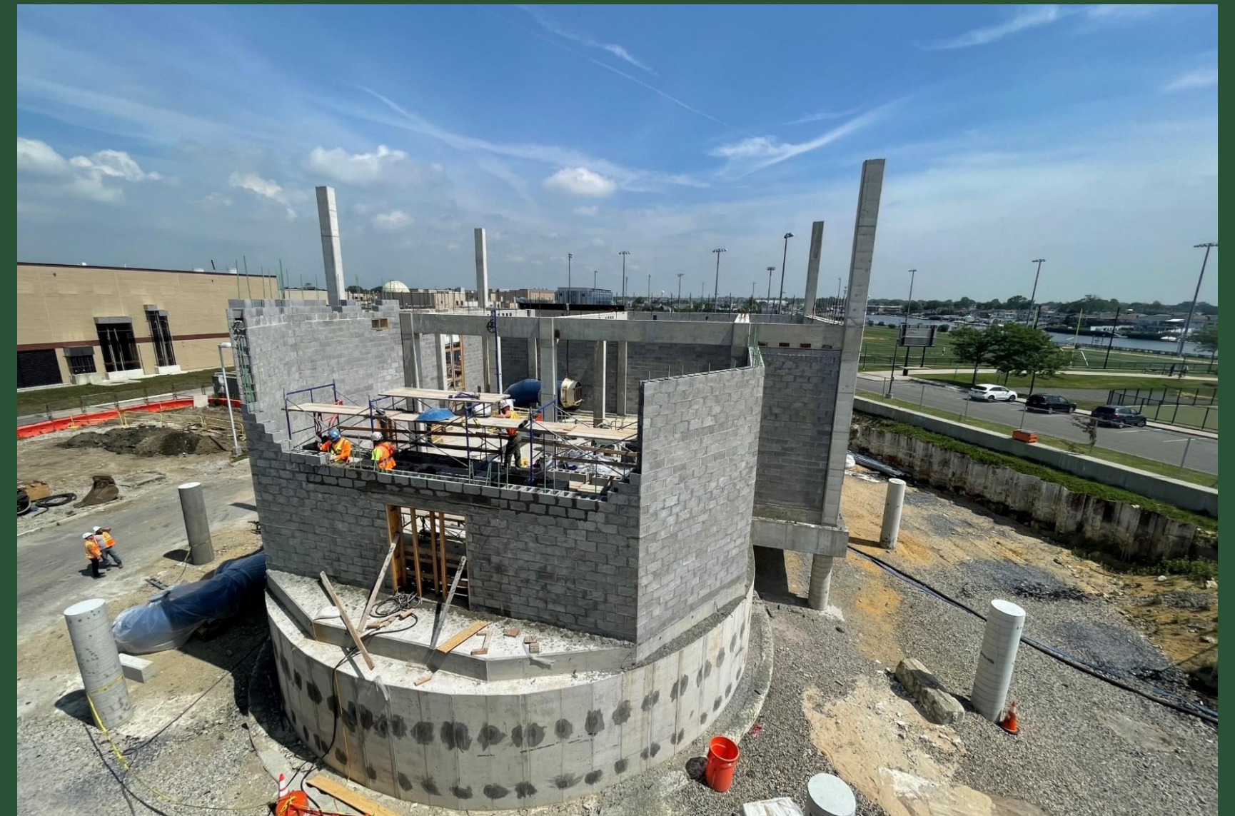
Pump Station Construction Near BP1 (July 2023)
