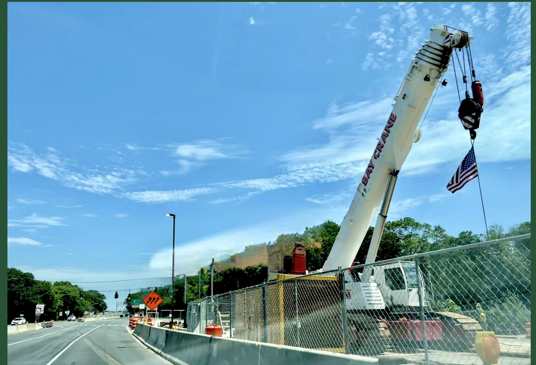
Construction at Pit W (July 2023)
