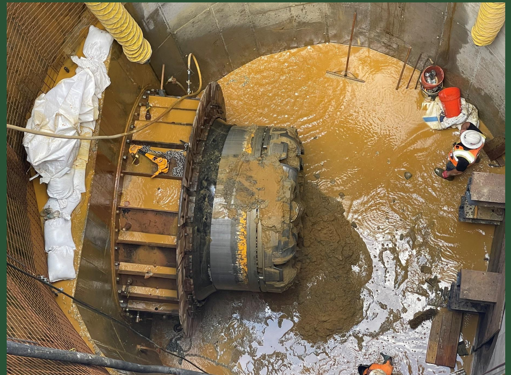
MTBM Breakthrough at BP7 (June 2023)
