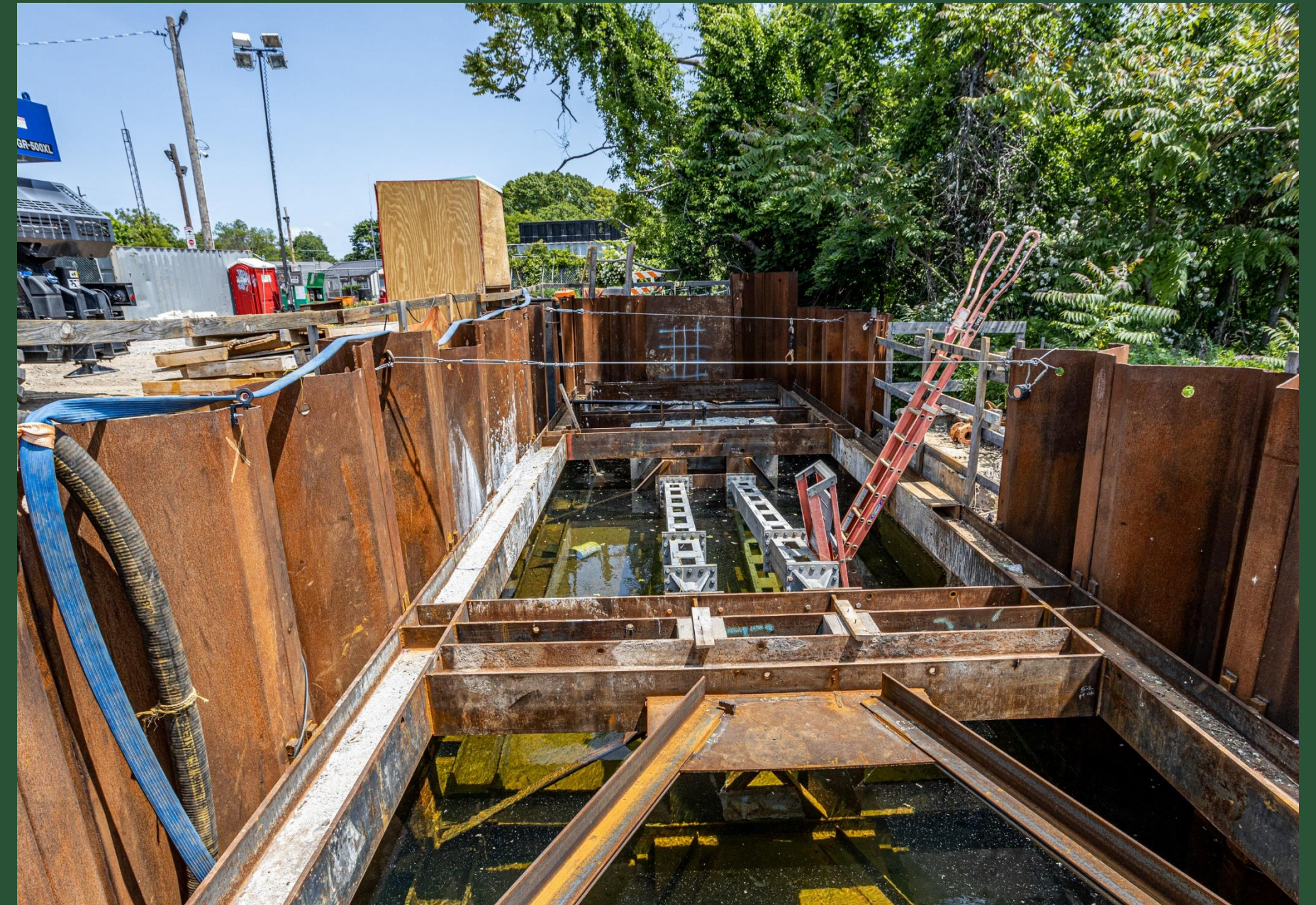
Work at Pit O (May 2023)
