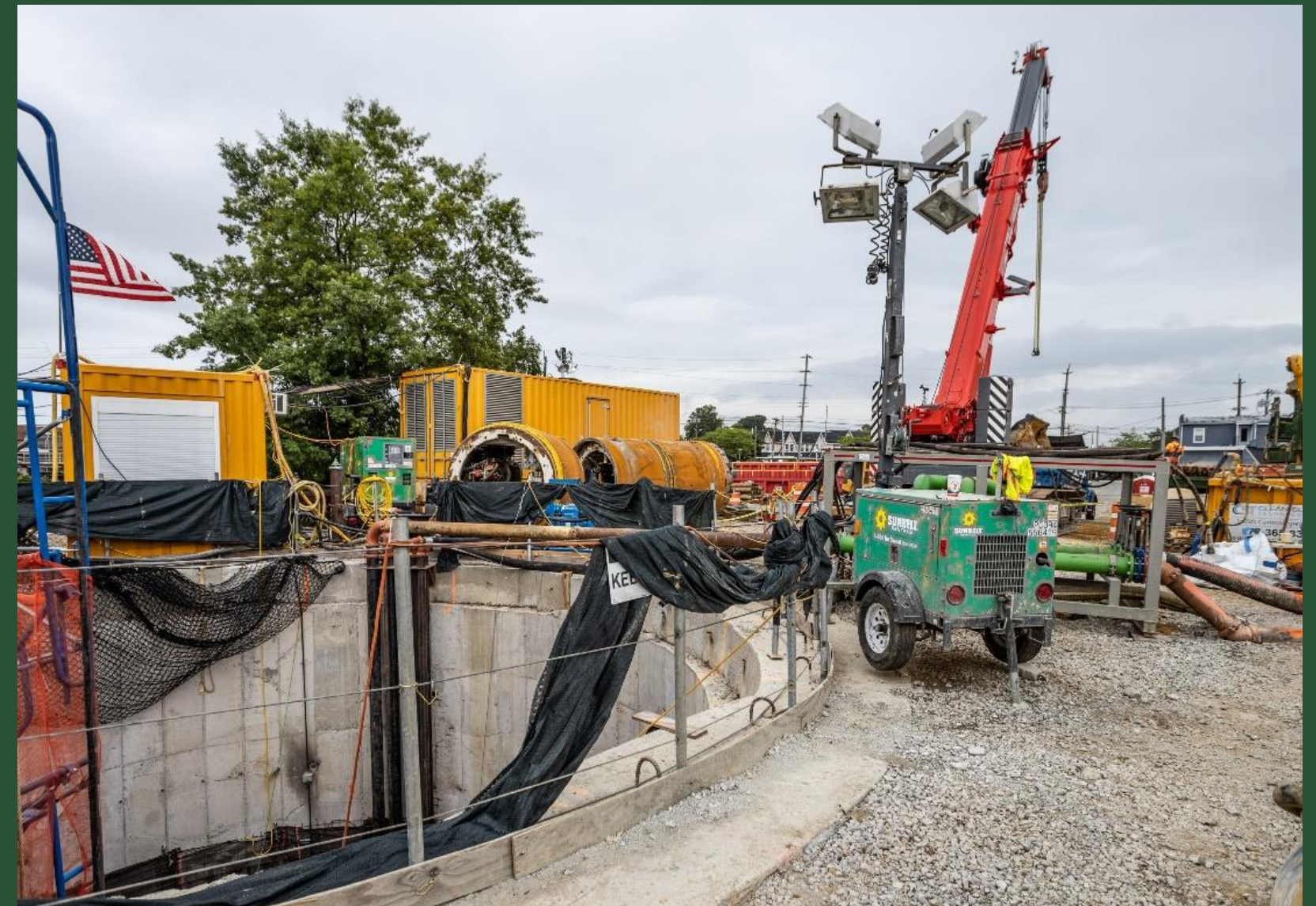
Microtunneling Activities at BP5 (July 2023)
