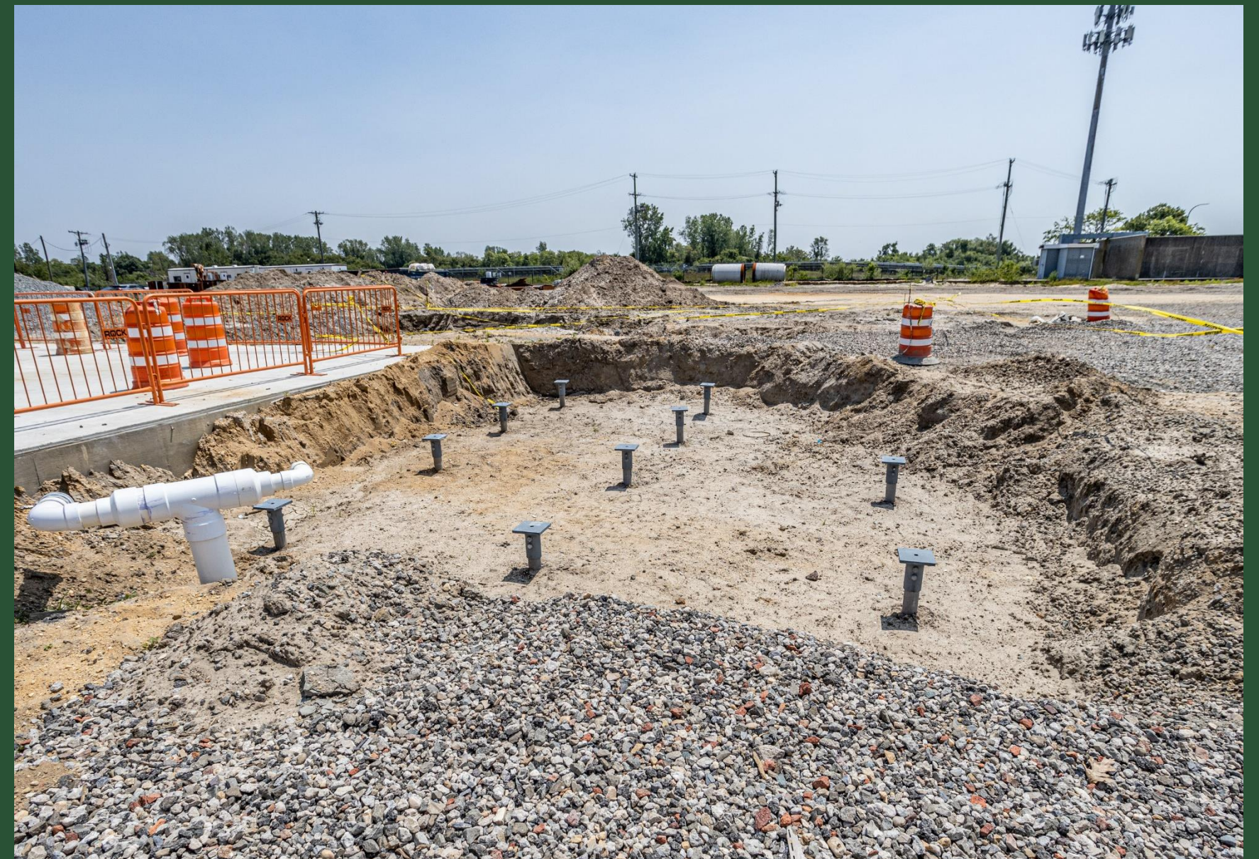
Helical Pile Installation near CC1 (May 2023)
