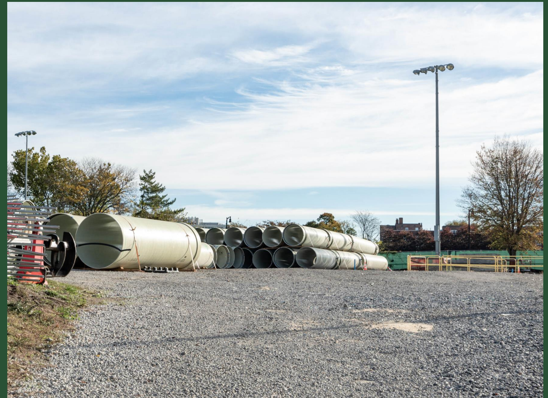
Pipe Storage at BP8 (October 2022)
