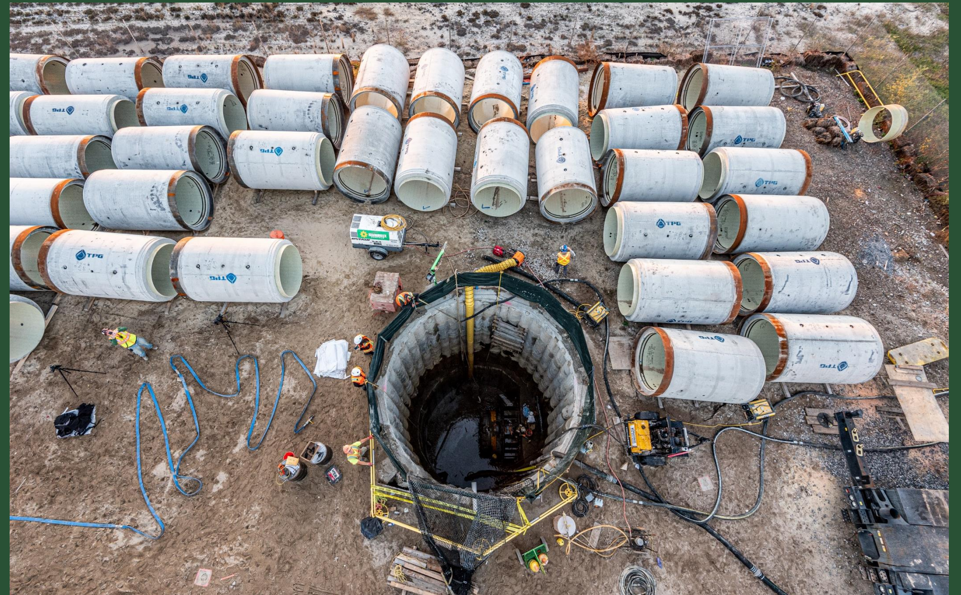
MTBM Breakthrough at CC1 (November 2022)
