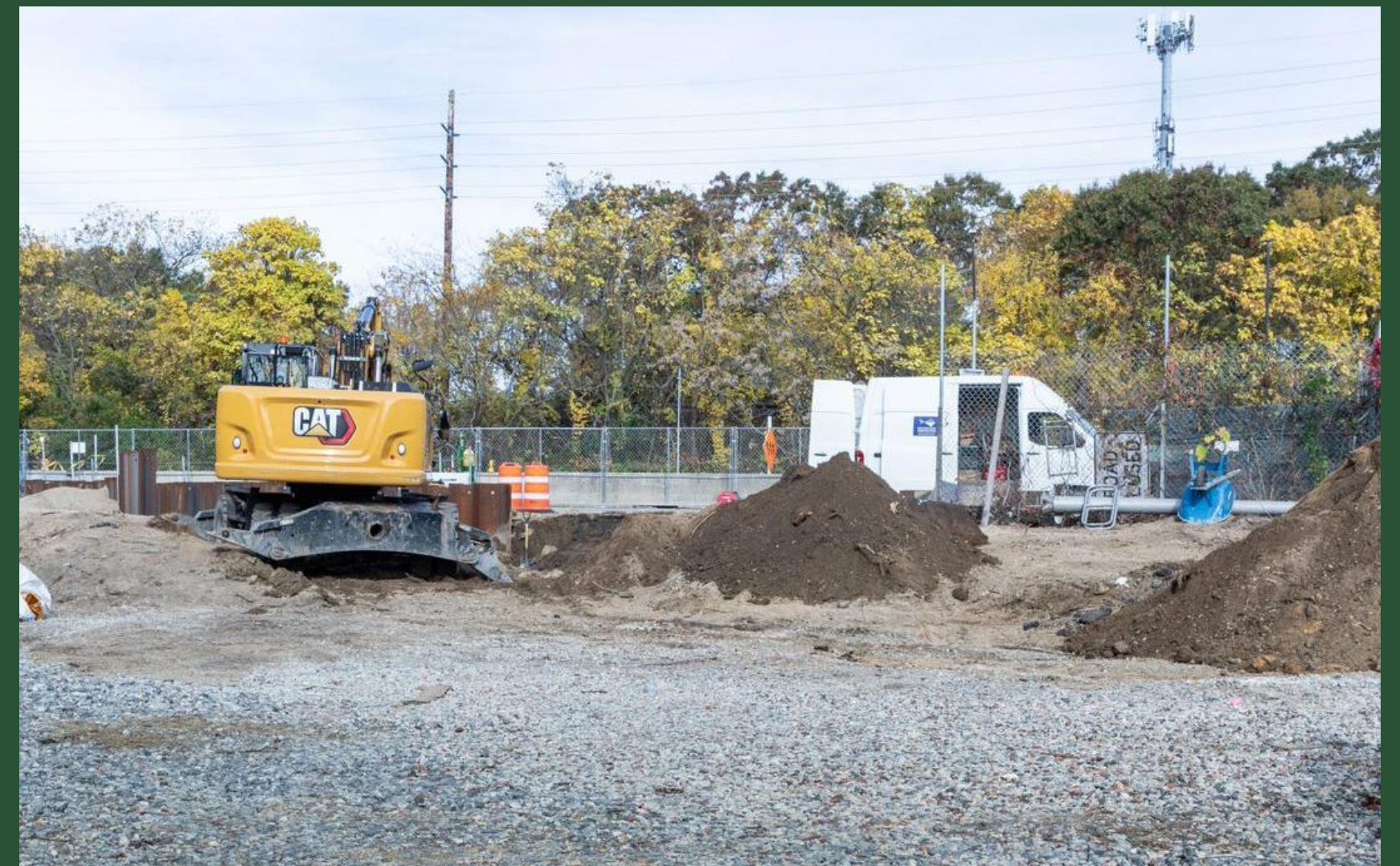
SOE Installation at Pit W (November 2022)
