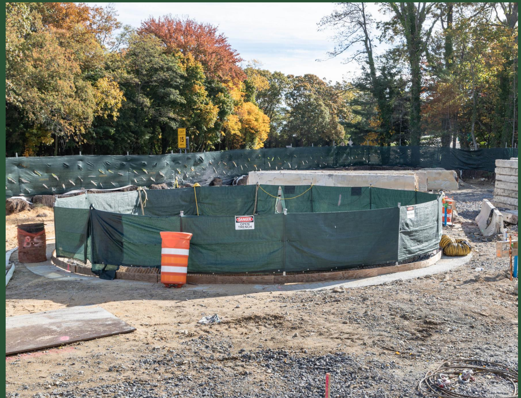
Construction Site at CC5 (July 2022)
