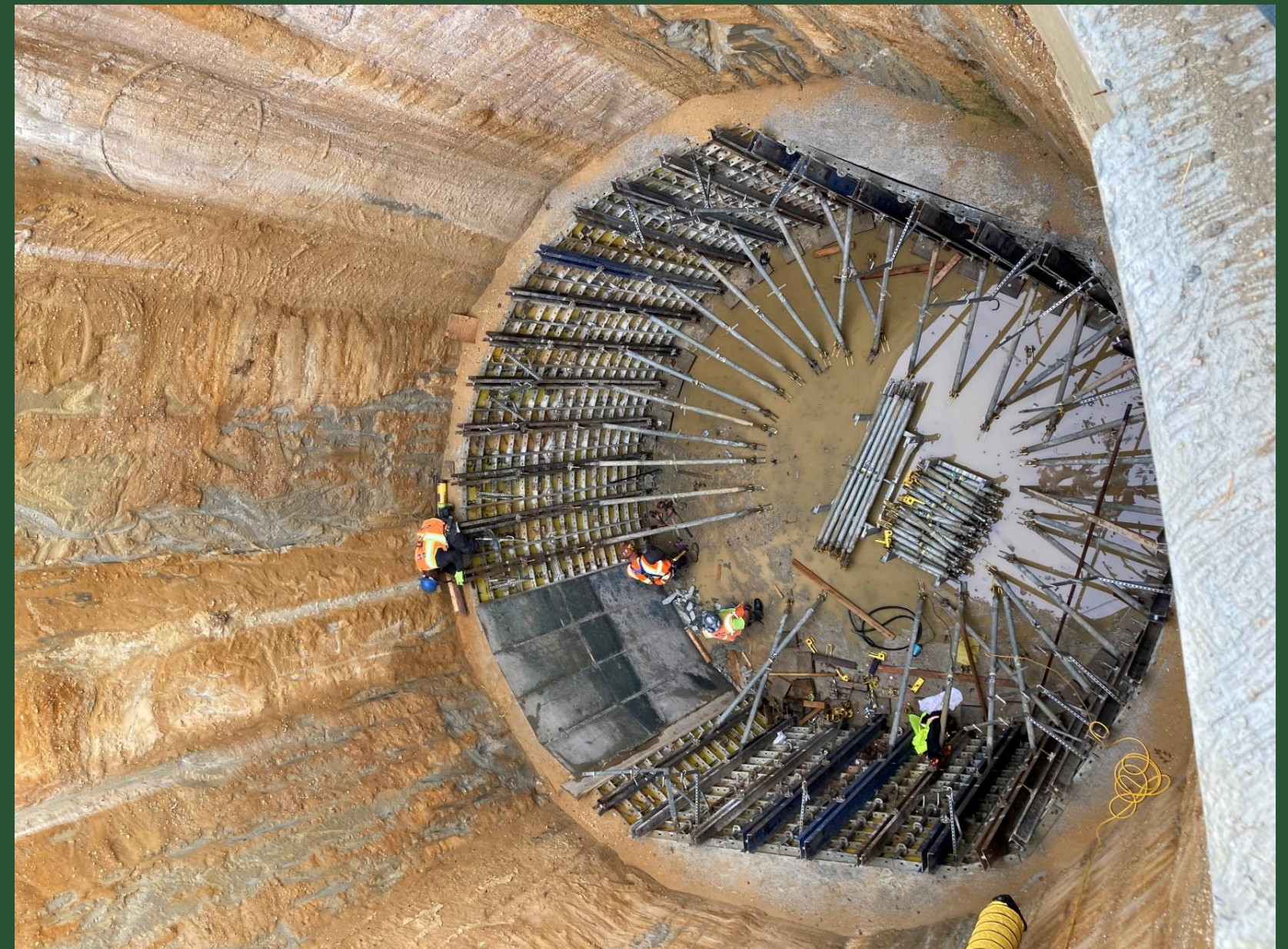
Reinforced Concrete Liner Wall Construction at CC4 (October 2022)
