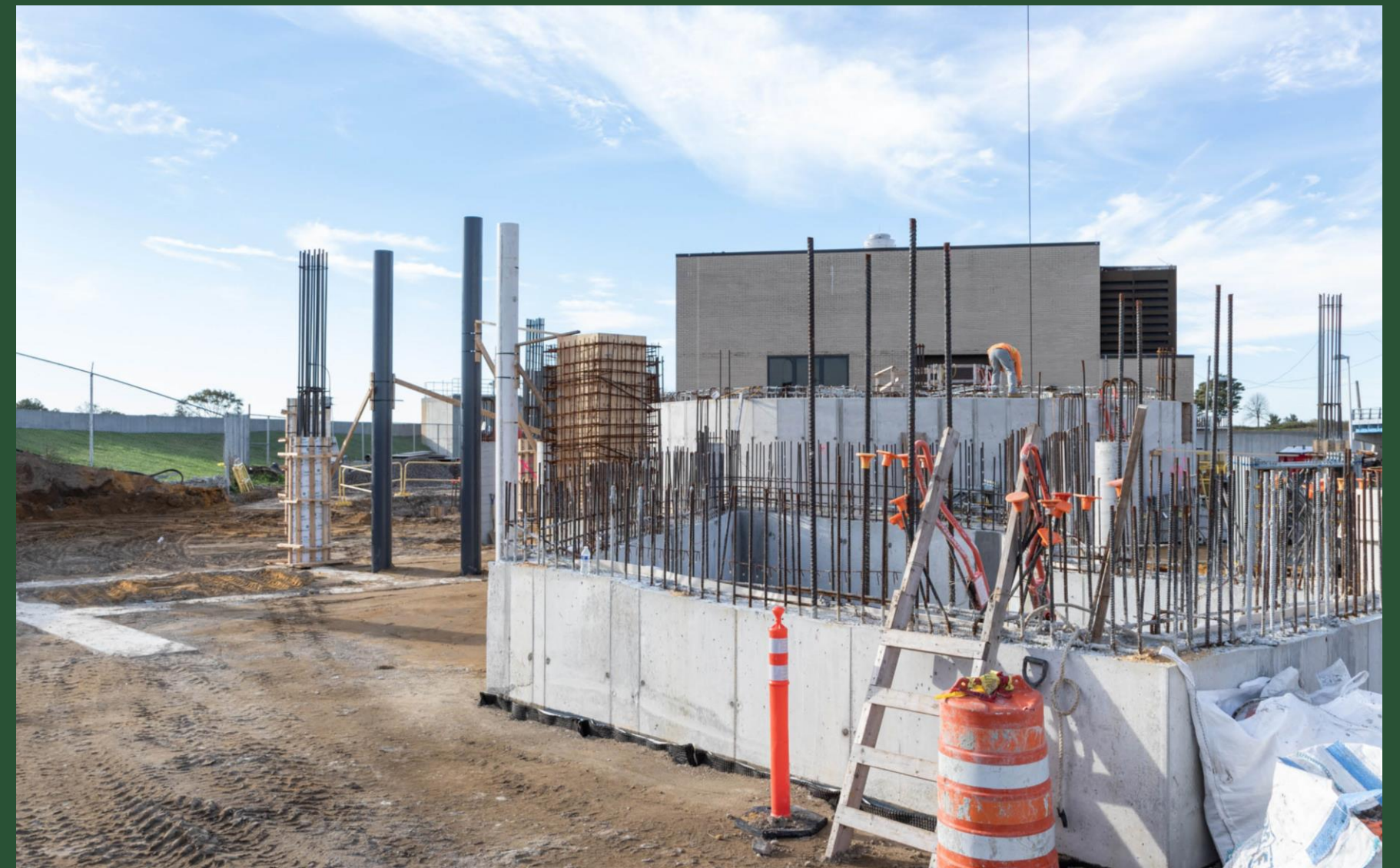
Diversion Structure Construction Near BP1 (October 2022)
