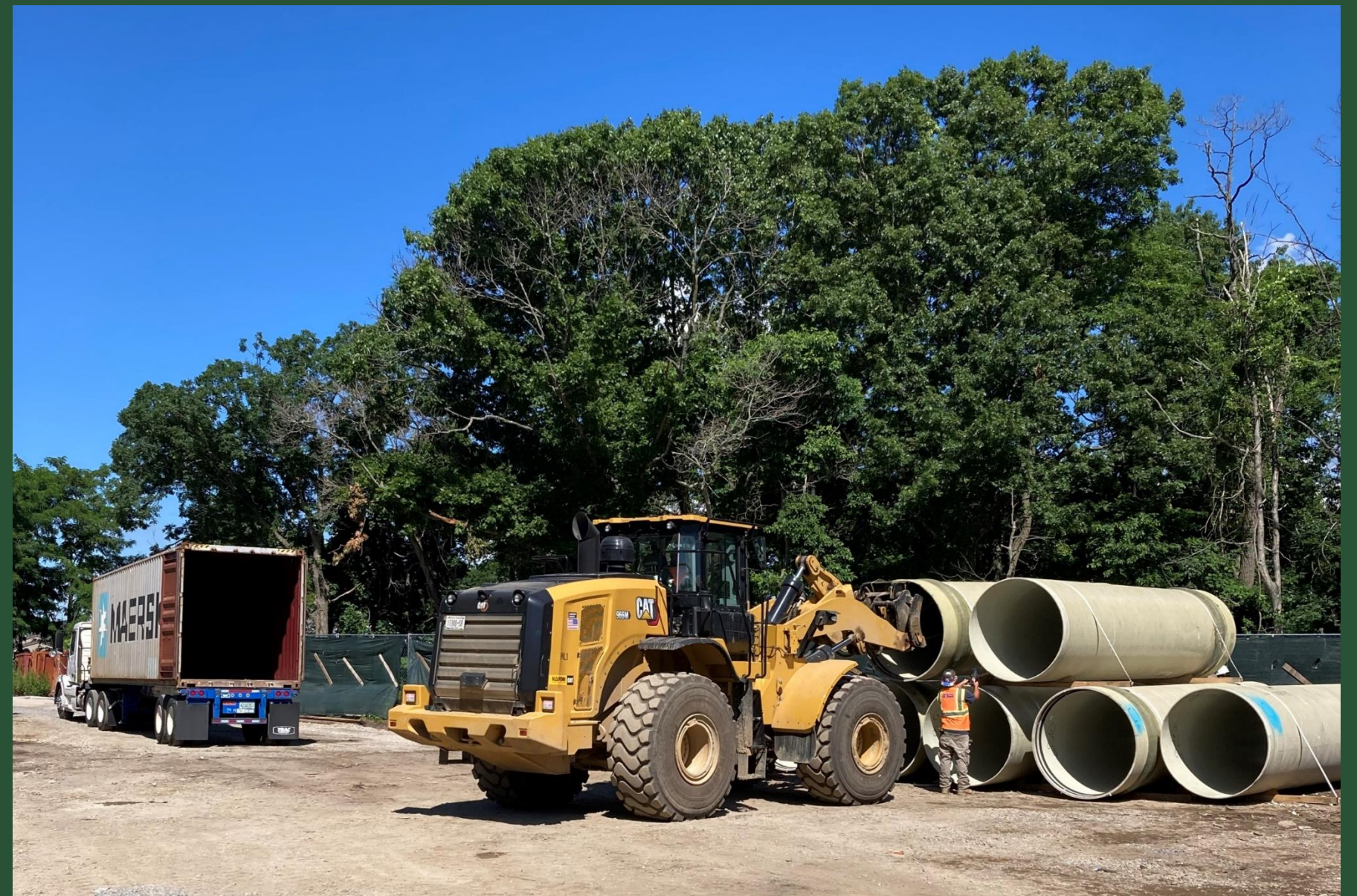
Pipe Delivery at Pit P (July 2022)
