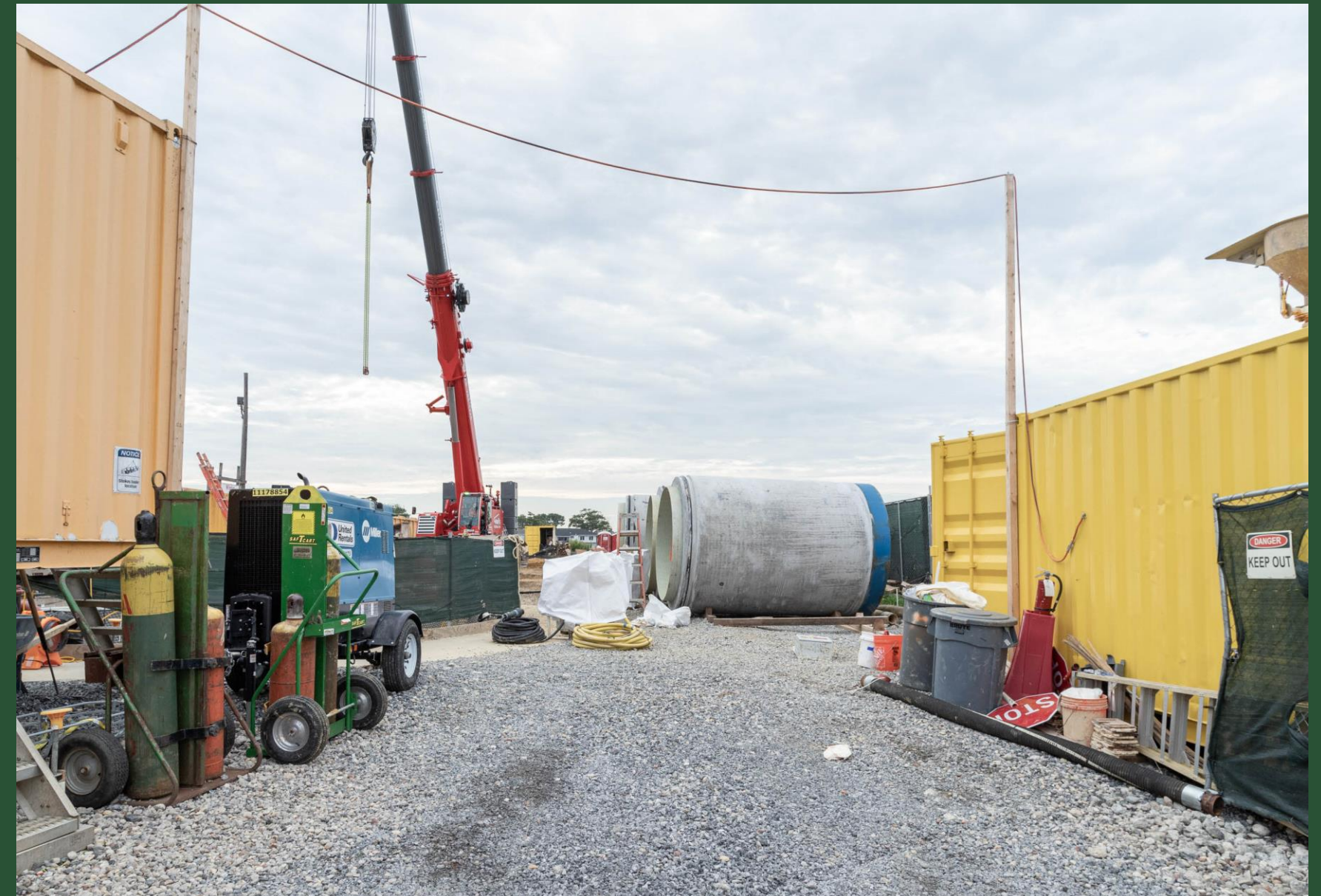
Construction Site at BP2 (July 2022)
