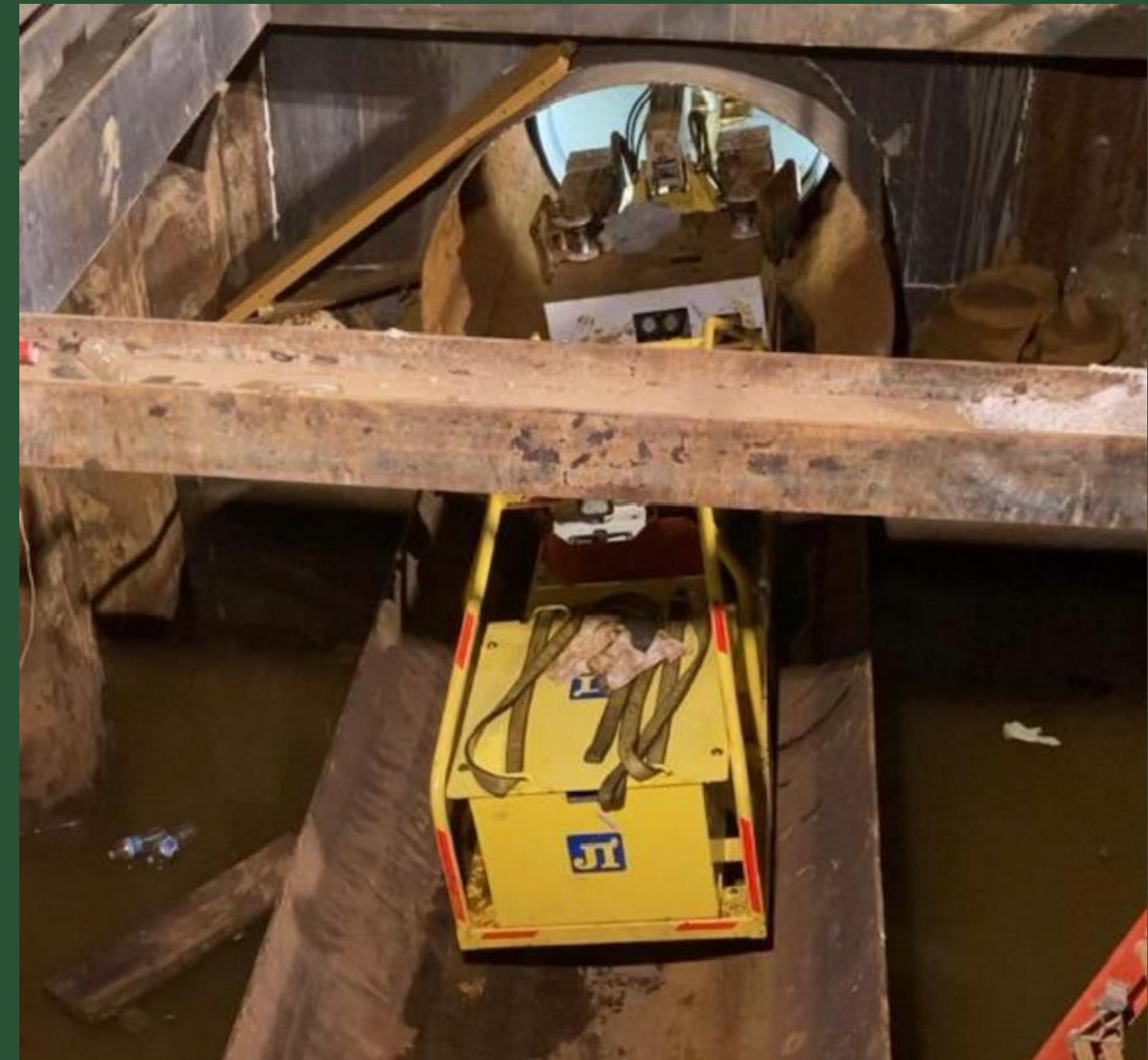
Jacking Equipment at Pit S (August 2022)
