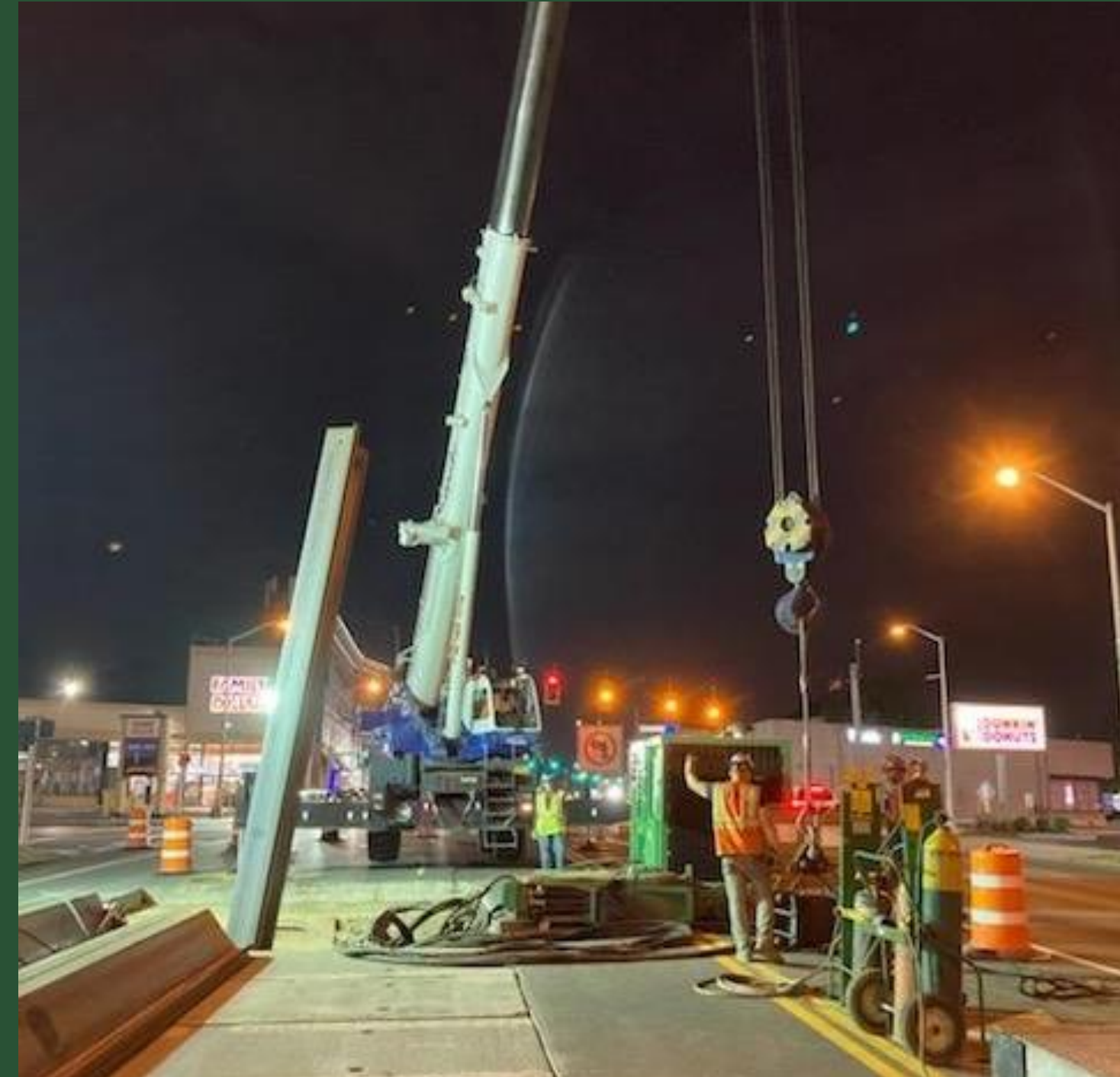
Sheet Pile Installation at Pit N (August 2022)
