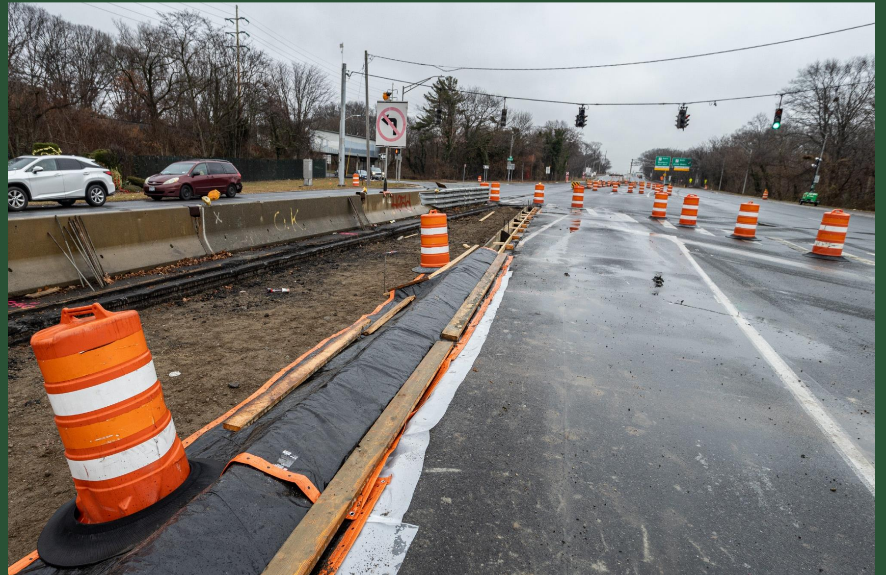
Construction at Pit W (September 2023)
