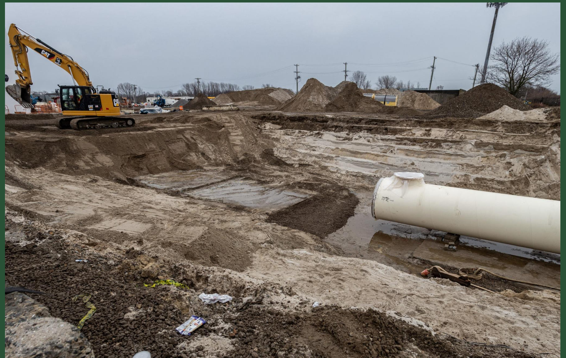
Installing Pipe toward CC1 (September 2023)
