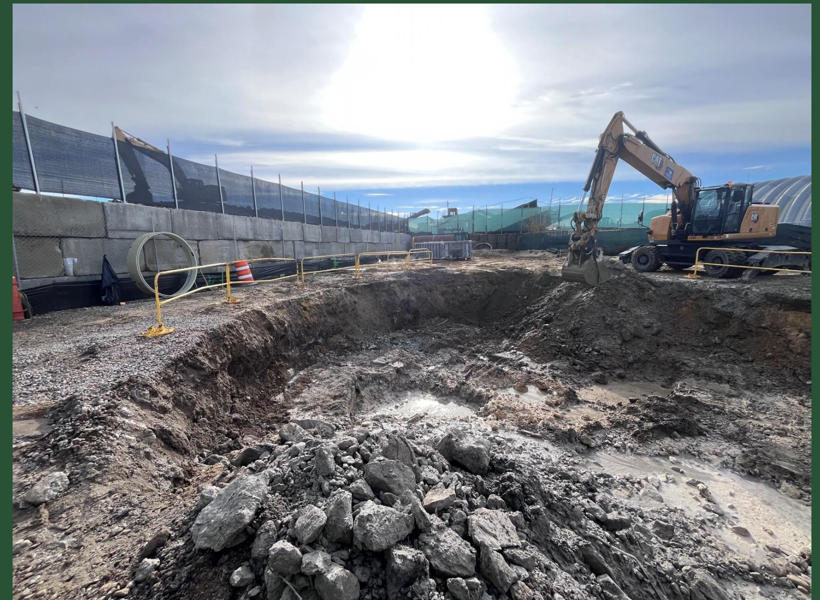
BP3 Restoration Activities (December 2023)
