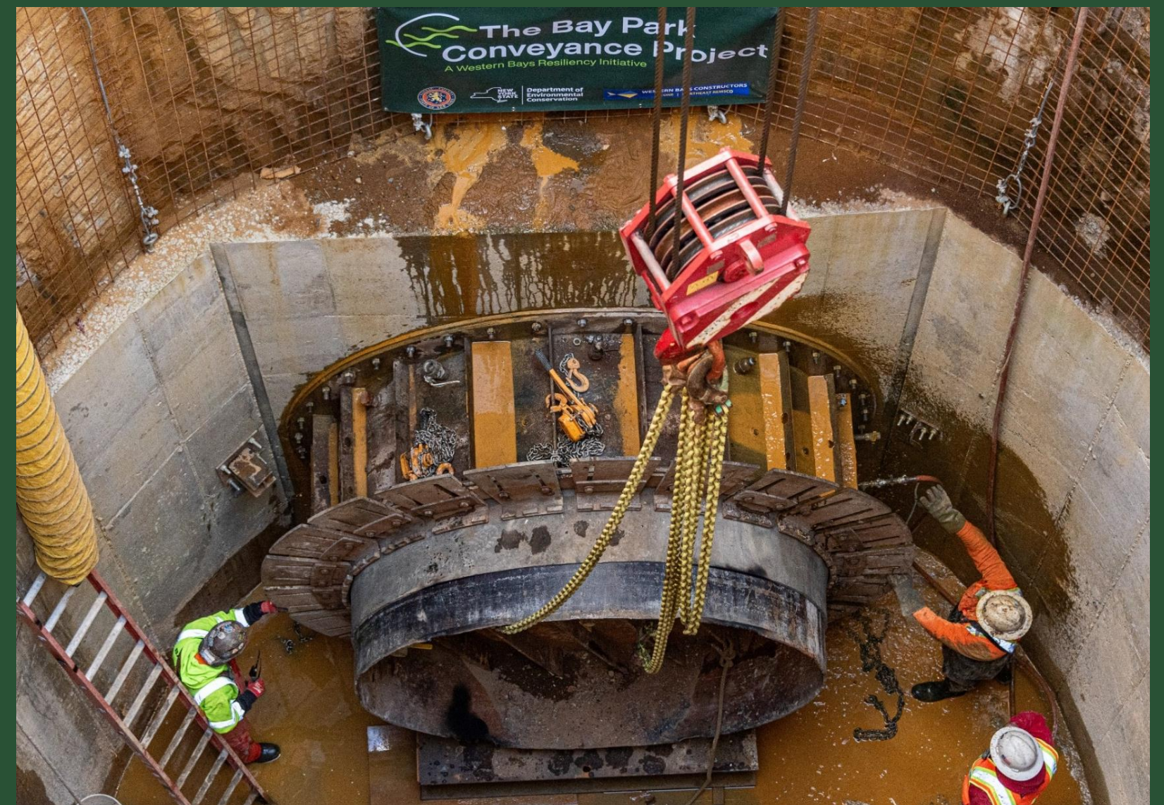
Breakthrough at BP7 (November 2023)
