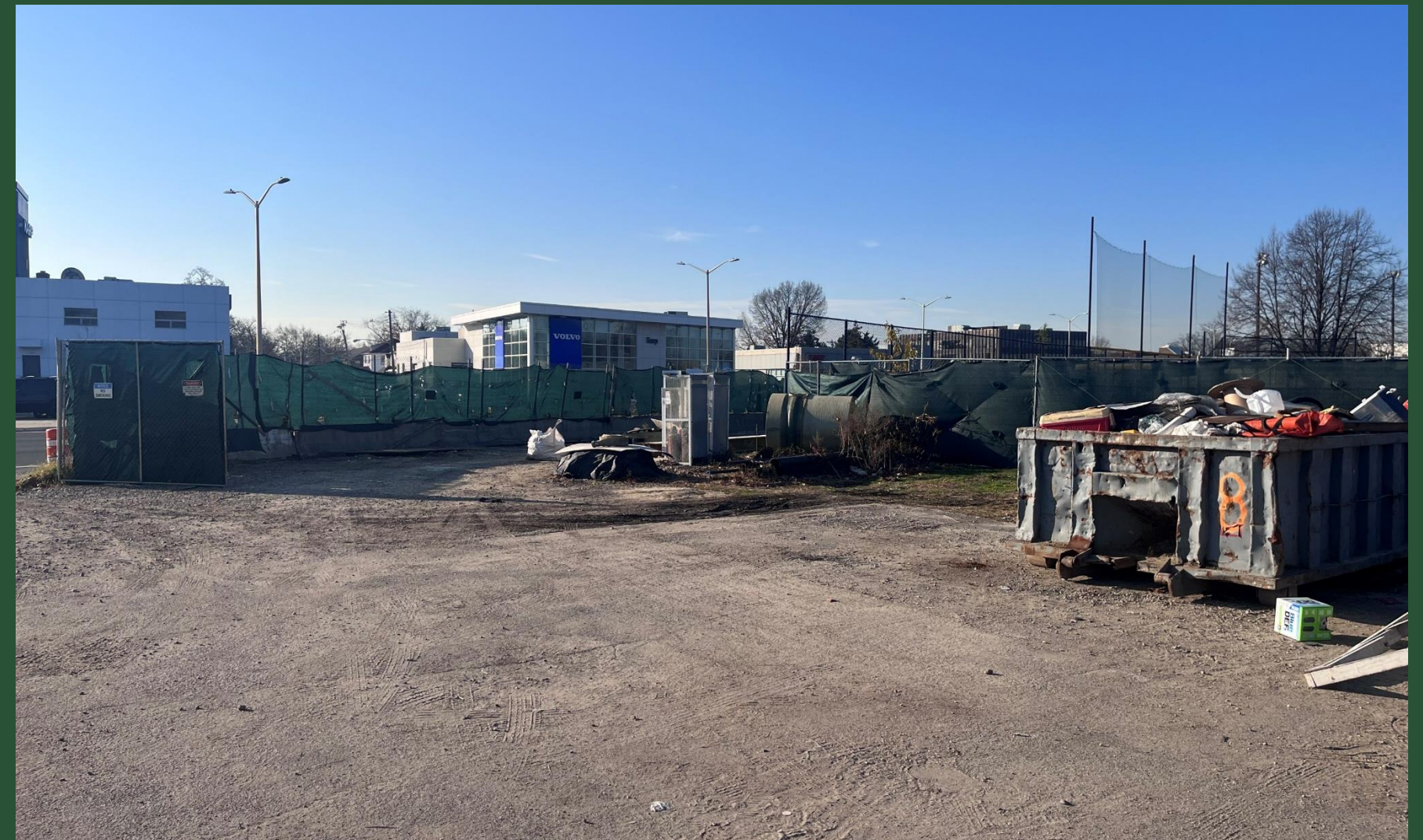
Pit A Site (December 2023)
