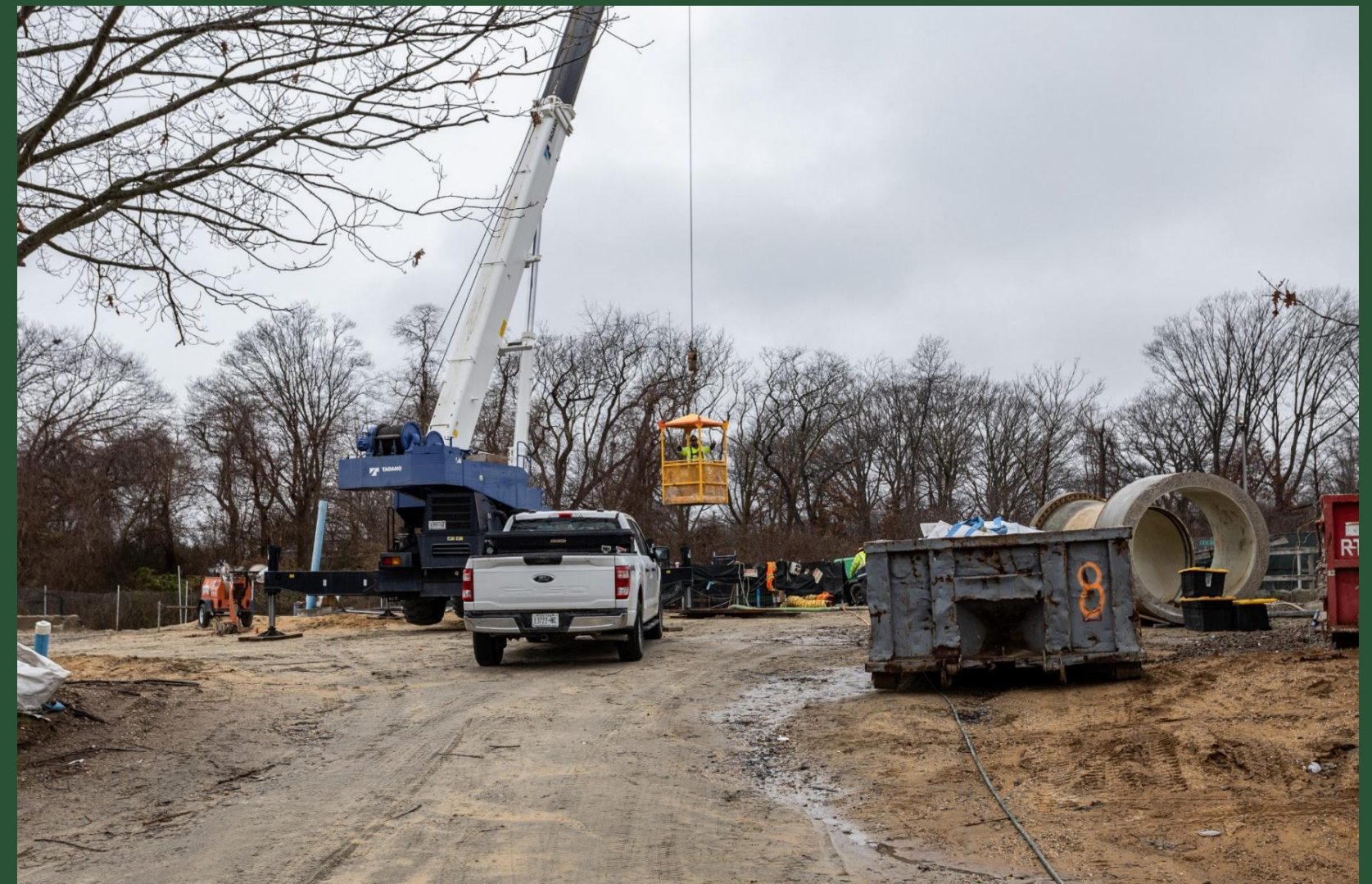
CC3 Construction Site (December 2023)
