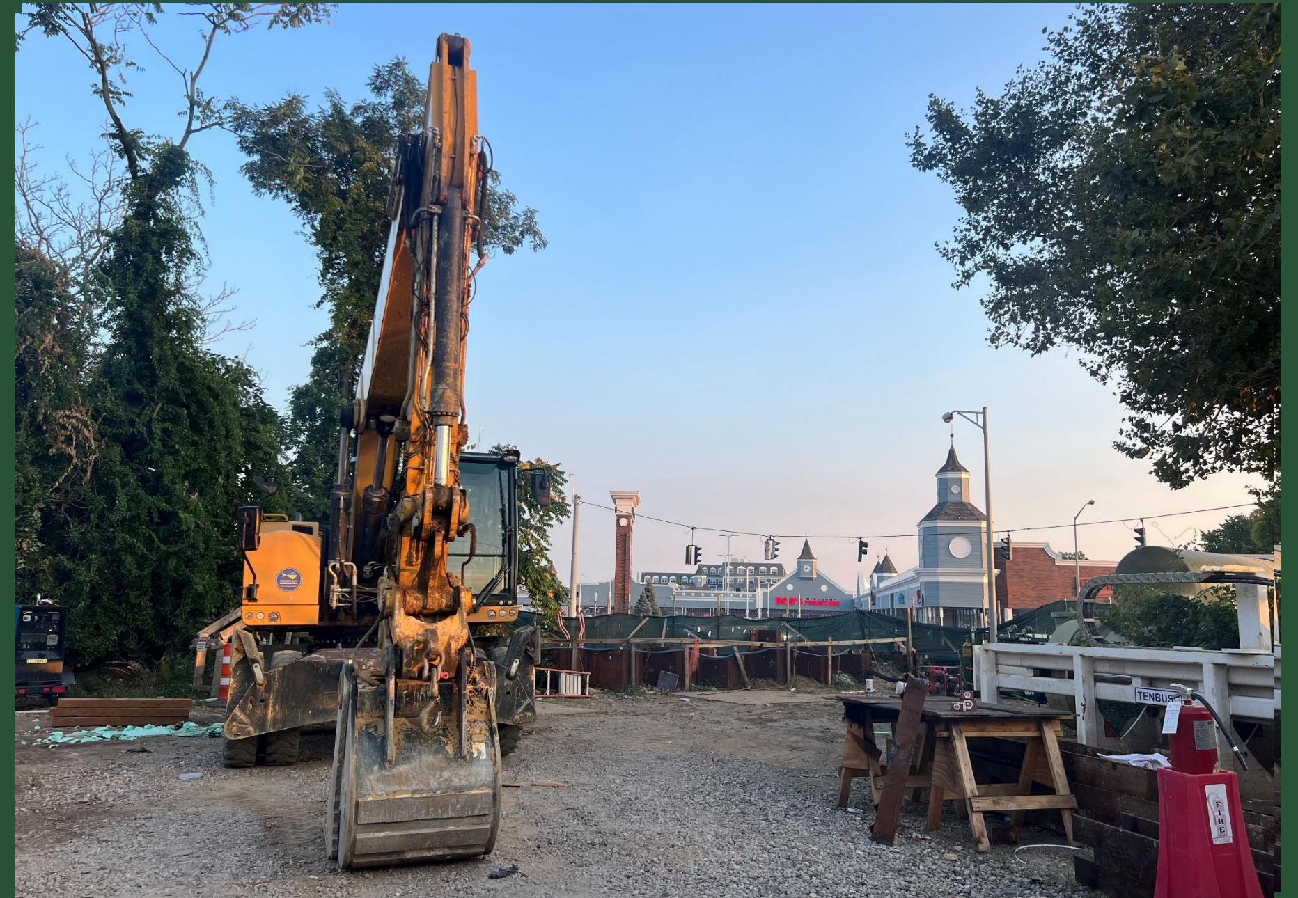
Site at Pit O (September 2023)
