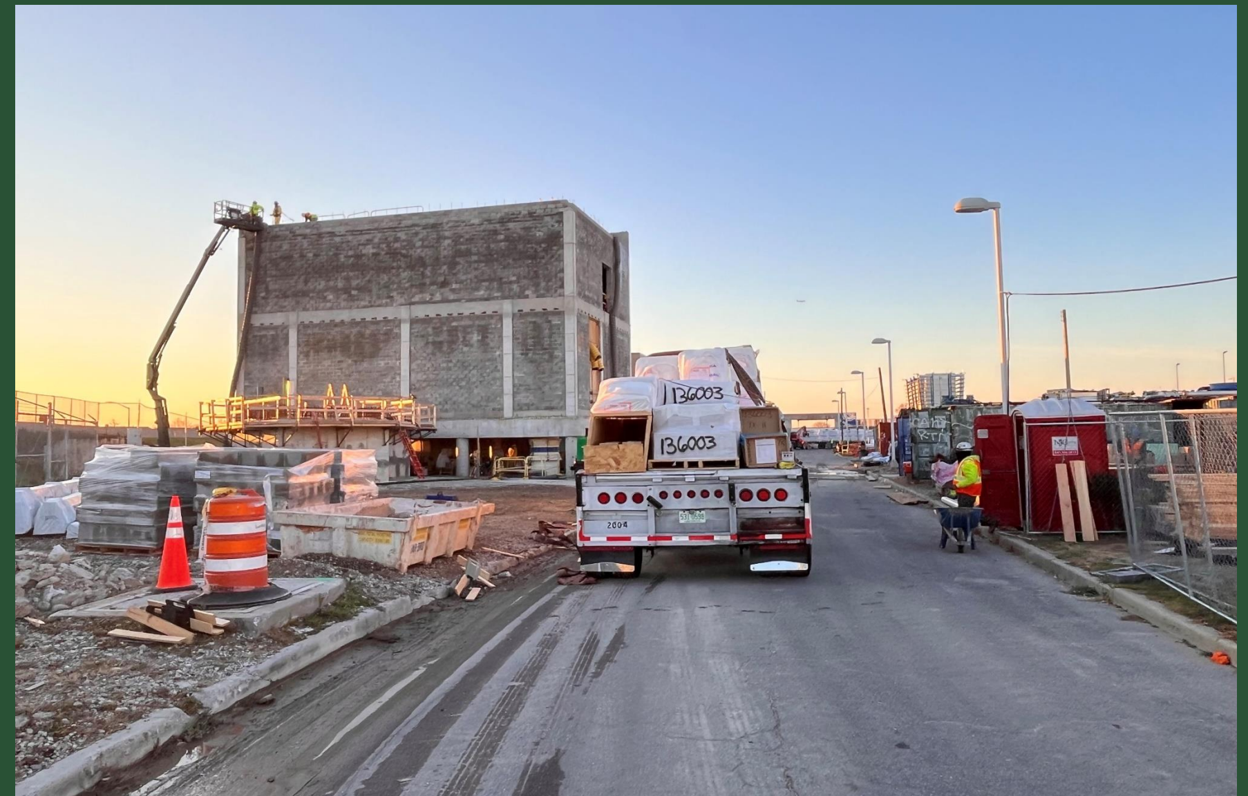
Pump Station Construction (November 2023)
