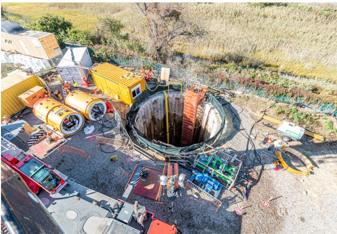
CC2 Construction Site
