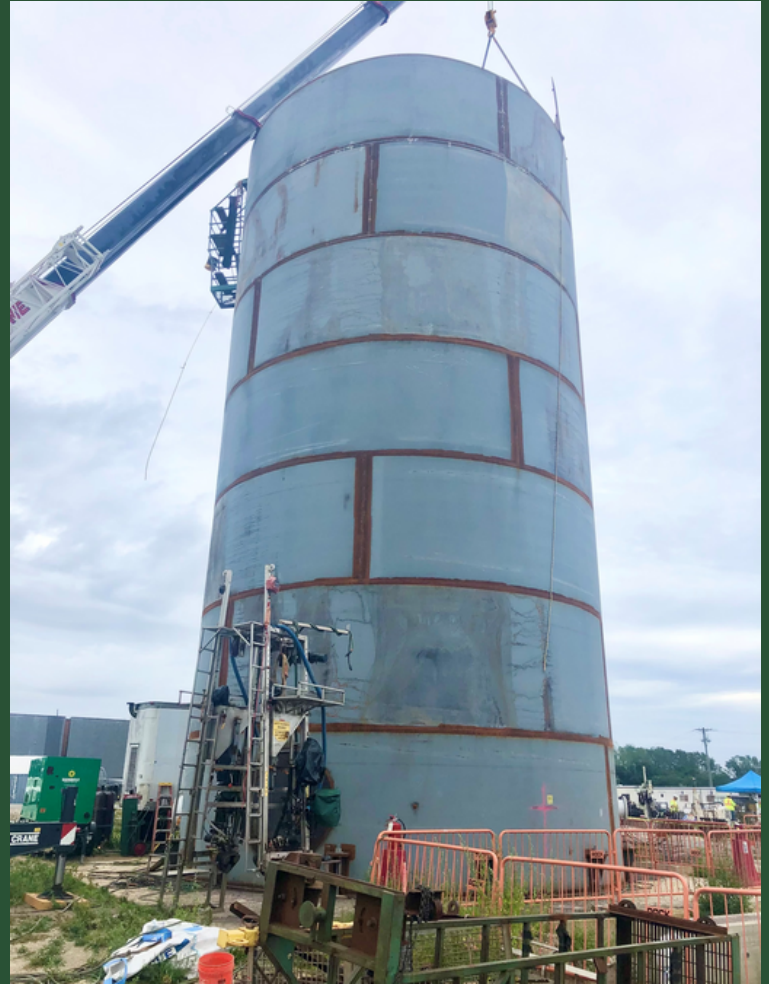
Construction of the Receiving Tank Structure (August 2023)
