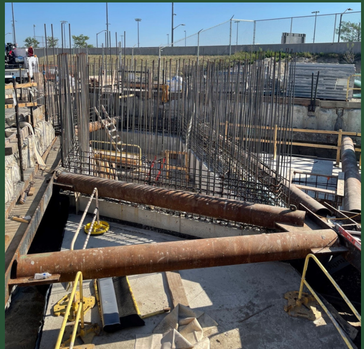
Diversion Structure Construction at BP1 (August 2022)
