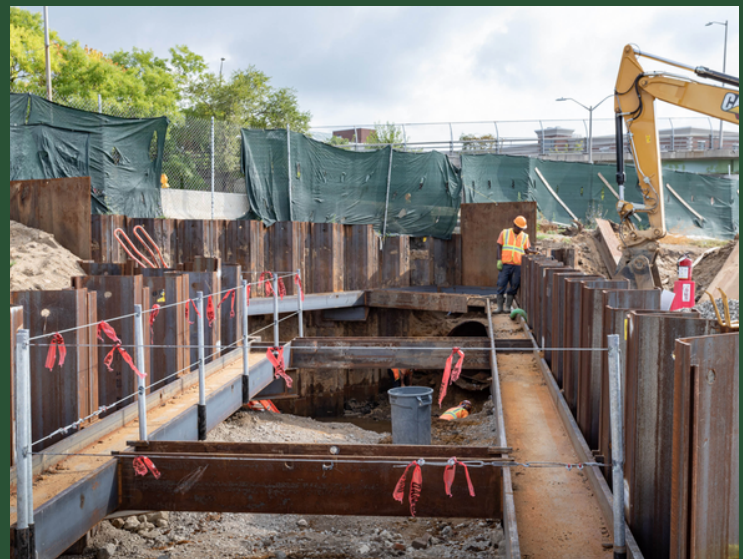
Sheet Pile Installation near Bay Park Shaft 9 (BP9) (August 2022)
