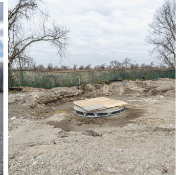
Backfilling at Cedar Creek Shaft 2
