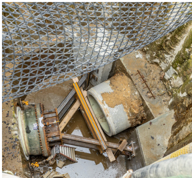
Cedar Creek Shaft 3
