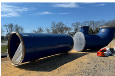
Bay Park Shaft 9 Pipe Delivery
