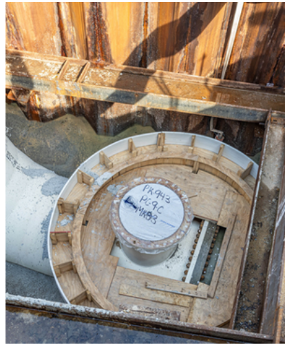
Riser Pipe at Cedar Creek Shaft 6
