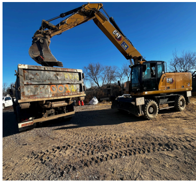
Regrading Activities at Bay Park Shaft 7
