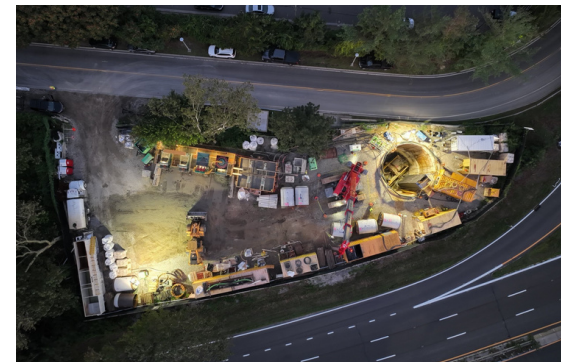
CC4 Construction Site
