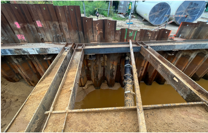
Construction at Pit W
