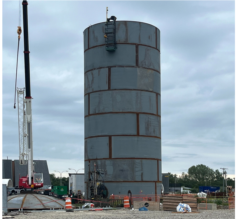
Receiving Tank Structure
