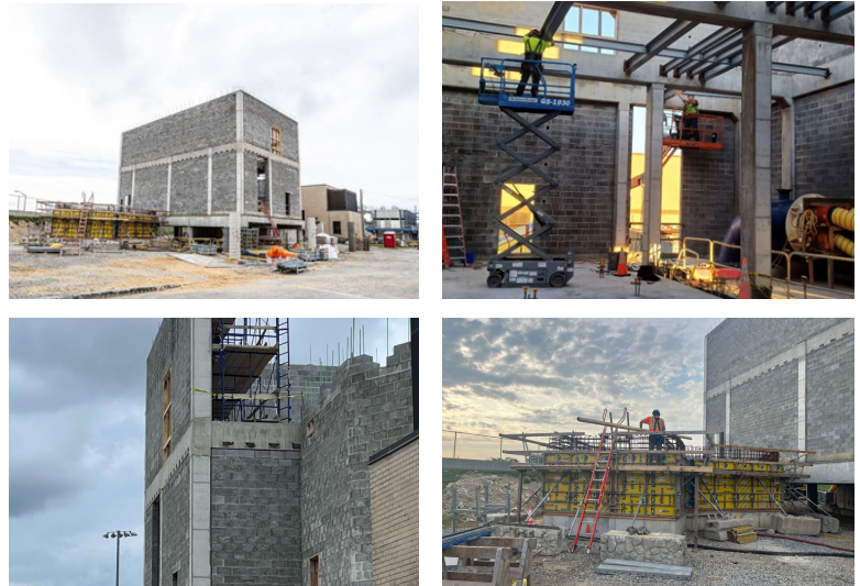
Pump Station Progress
