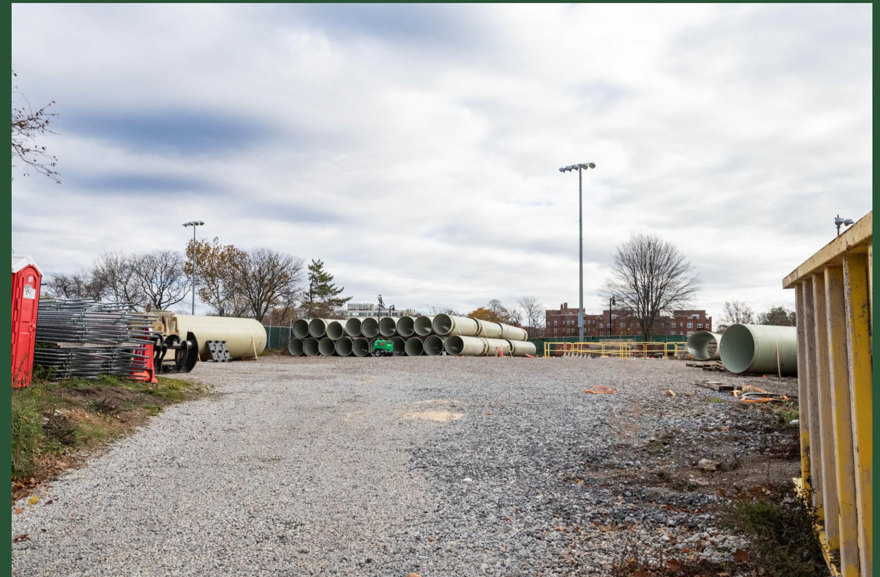
Pipe Storage at BP8 (November 2022)
