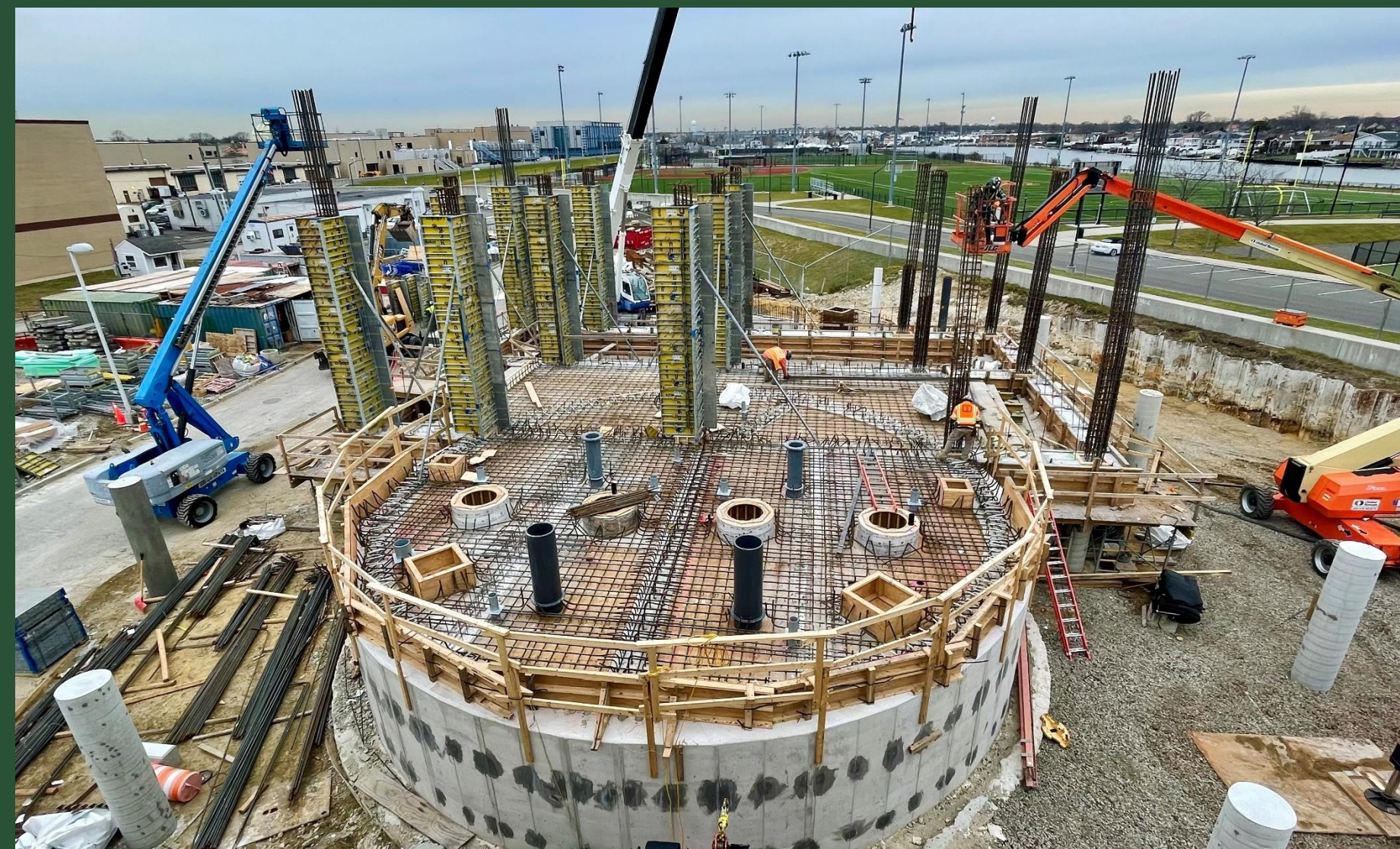
Pump Station Construction Near BP1 (January 2023)
