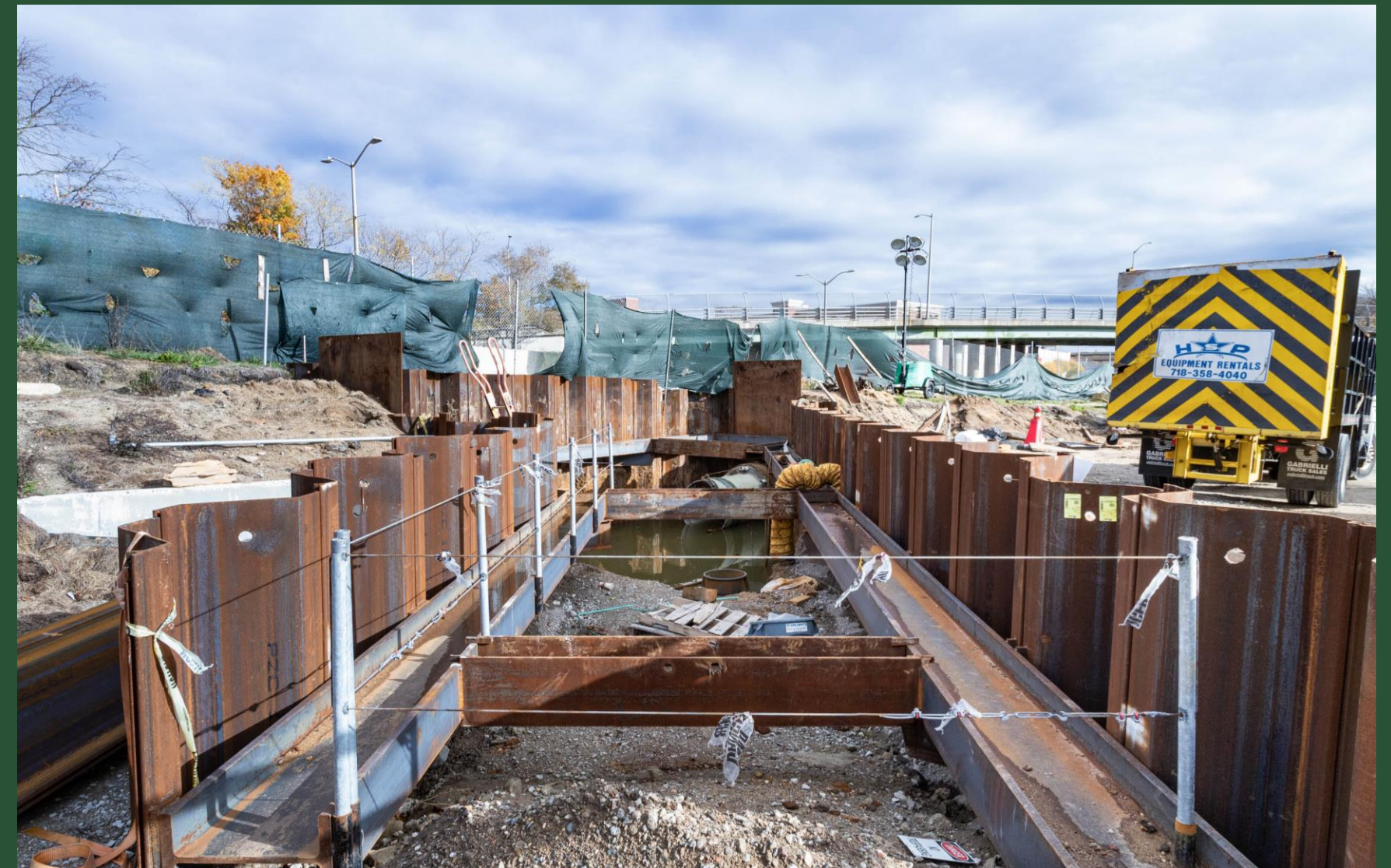
Sheet Pile Installation at BP9 (November 2022)
