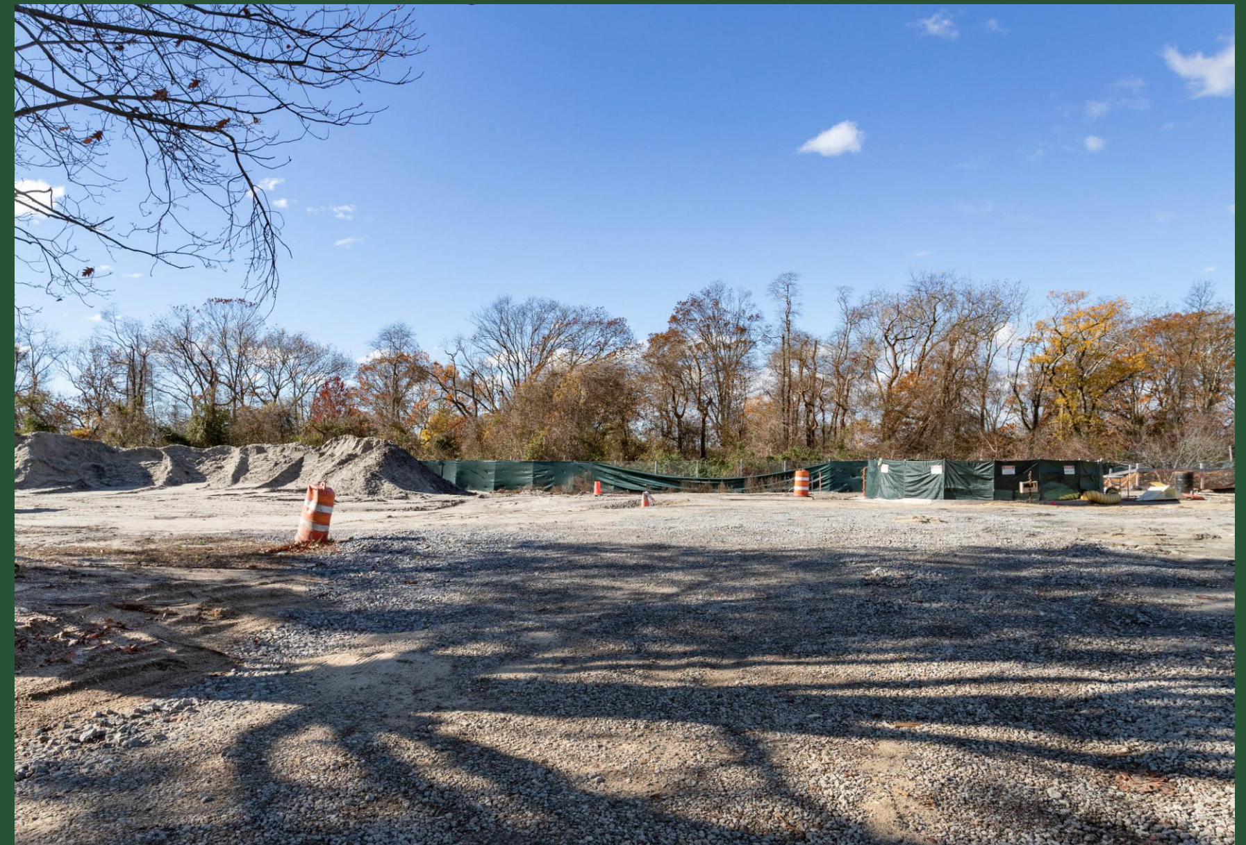
Construction Site at CC4 (November 2022)
