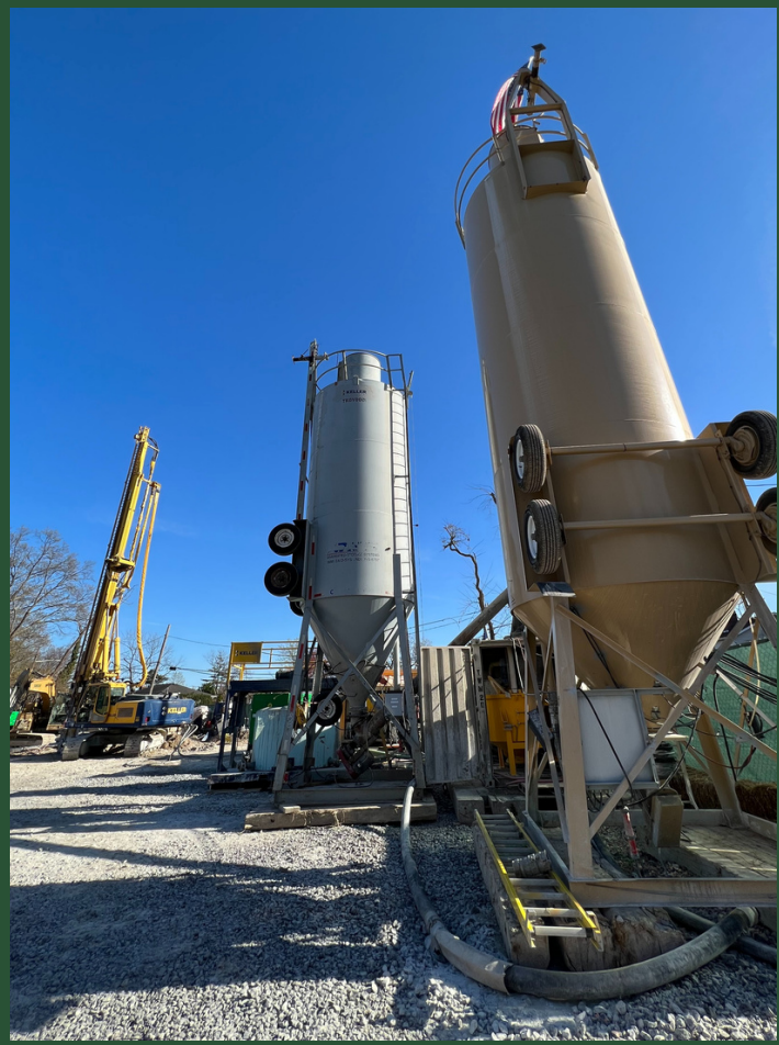
CC5 Jet Grout Operation, April 2022
