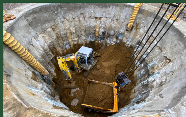
Excavation at BP4, April 2022
