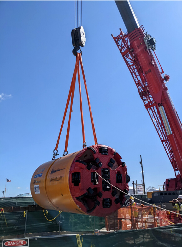
MTBM installation at BP2, April 2022
