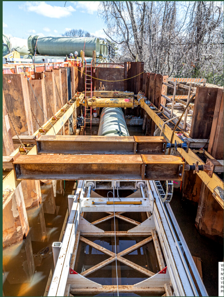
Pipe Jacking from Pit P to Pit O, March 2022
