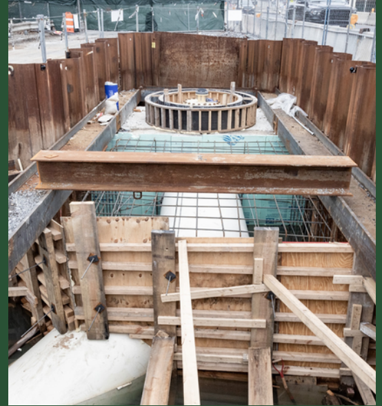
SOE at Pit W (March 2023)
