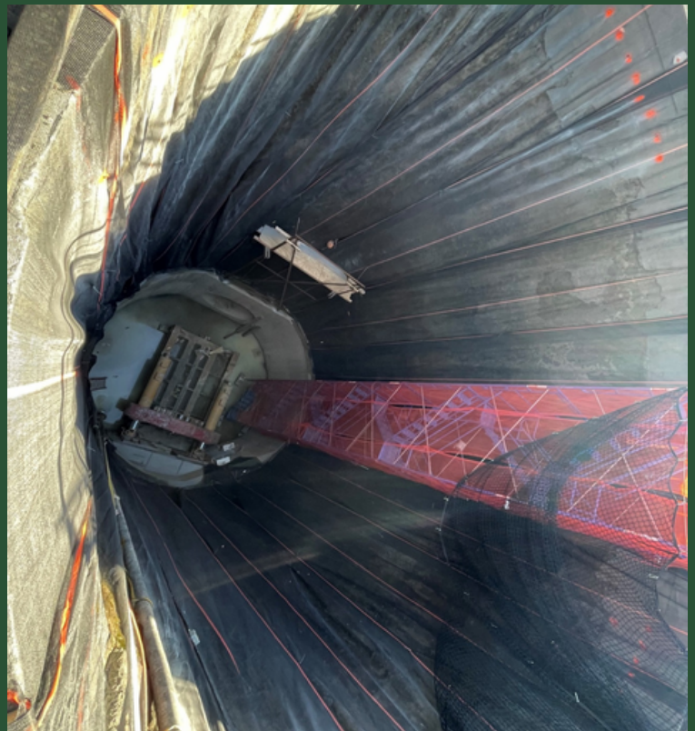
BP5 Microtunneling Preparations (April 2023)
