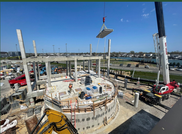
Pump Station Construction near BP1 (April 2023)
