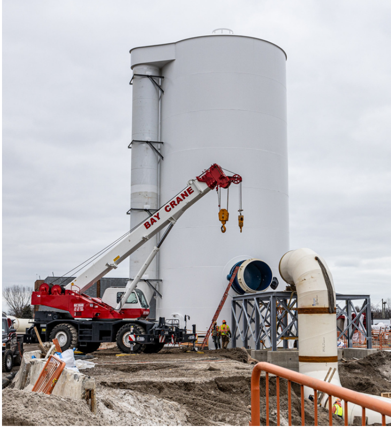
Receiving Tank Structure Progress (January 2024)
