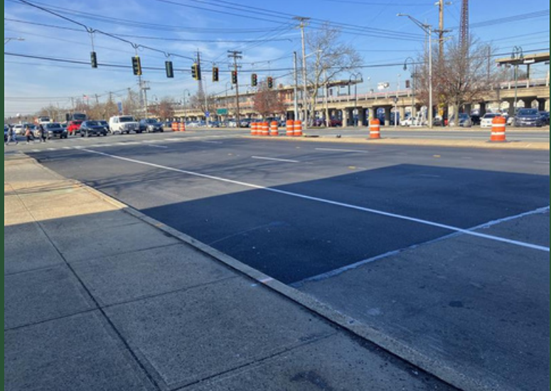
Final Roadway Restoration at Pit GG in Baldwin
