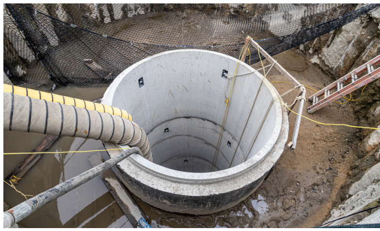
Cedar Creek Shaft 2 Manhole Installation (February 2024)
