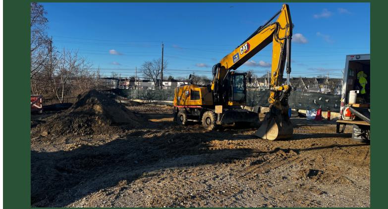
Regrading at Bay Park Shaft 5 (January 2024)
