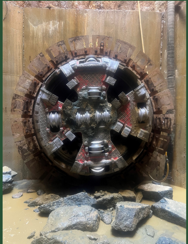
Breakthrough at BP4 (February 2023)
