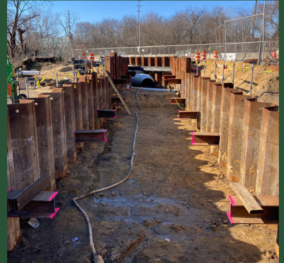
SOE Installation Between Pit W and CC6 (February 2023)
