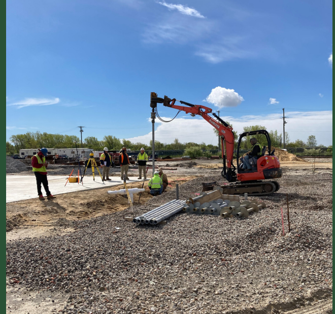
Helical Pile Installation near CC1 (April 2023)
