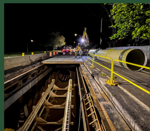
Sliplining at Pit F (May 2023)
