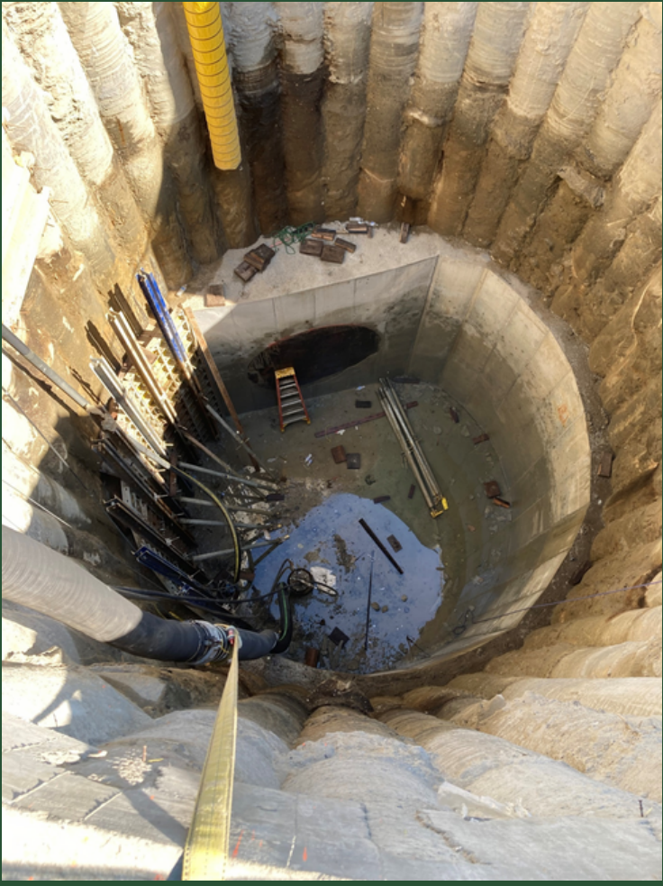
Liner Wall Installation at CC1 (May 2022)
