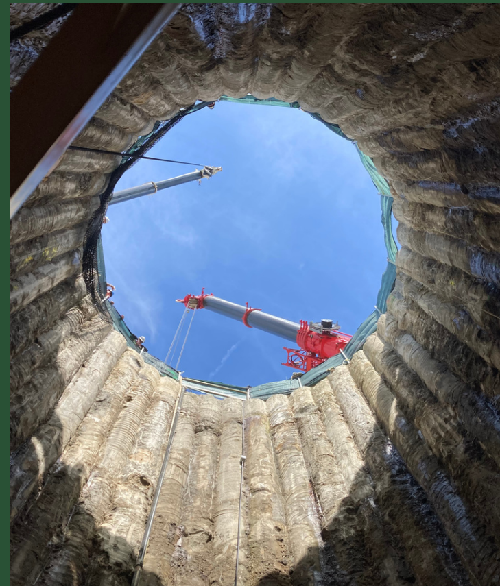
Inside the Shaft at BP1 (May 2022)
