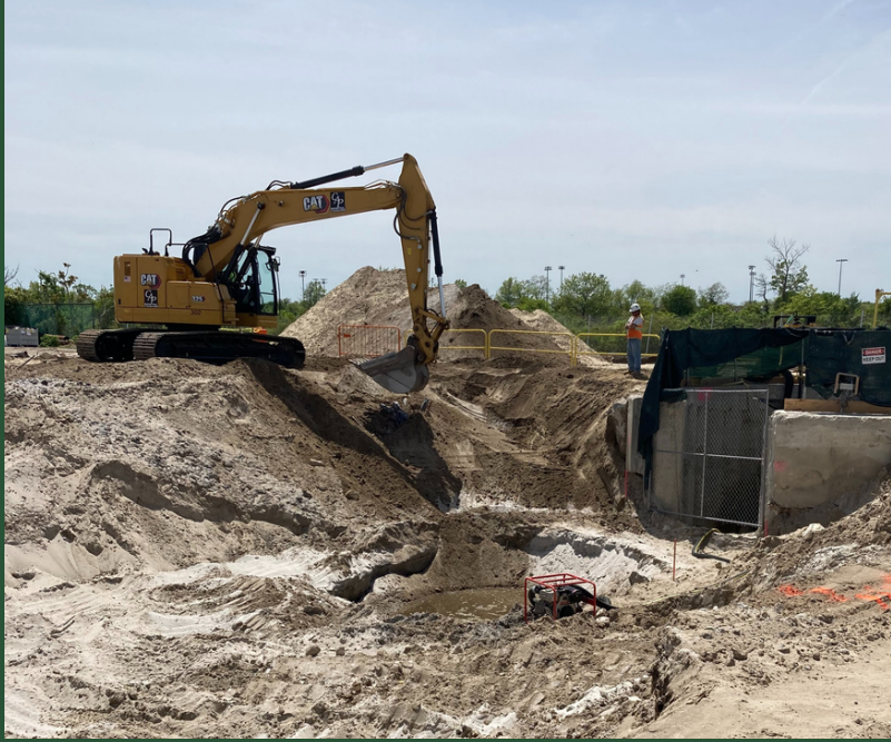
Construction Site at CC1 (May 2022)
