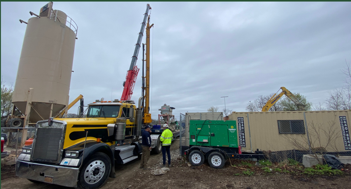
Jet Grout Operations at BP7 (May 2022)
