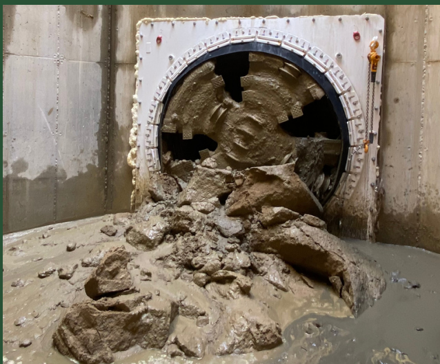
MTBM Arrival at BP1 (May 2022)
