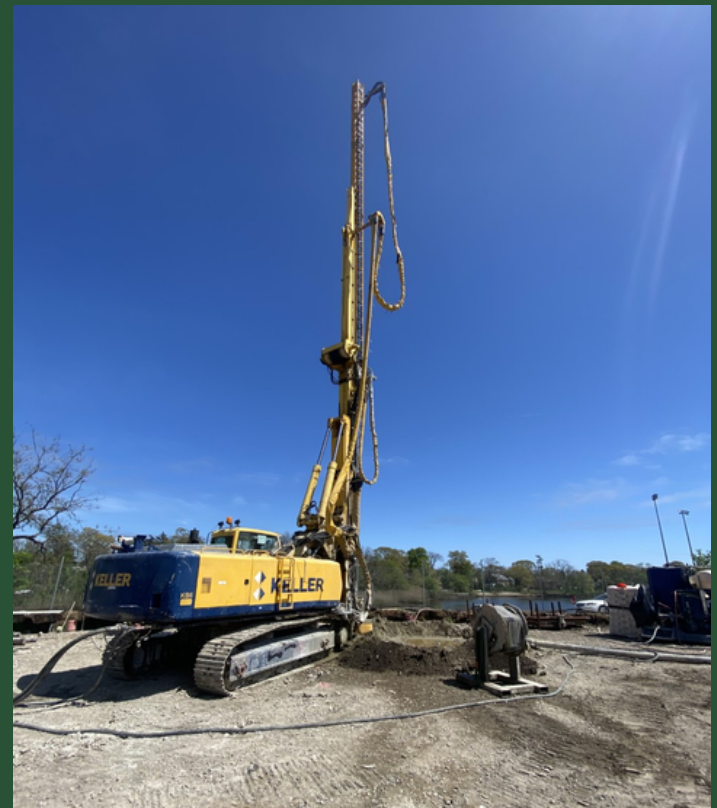
Jet Grout Operations at BP7 (May 2022)
