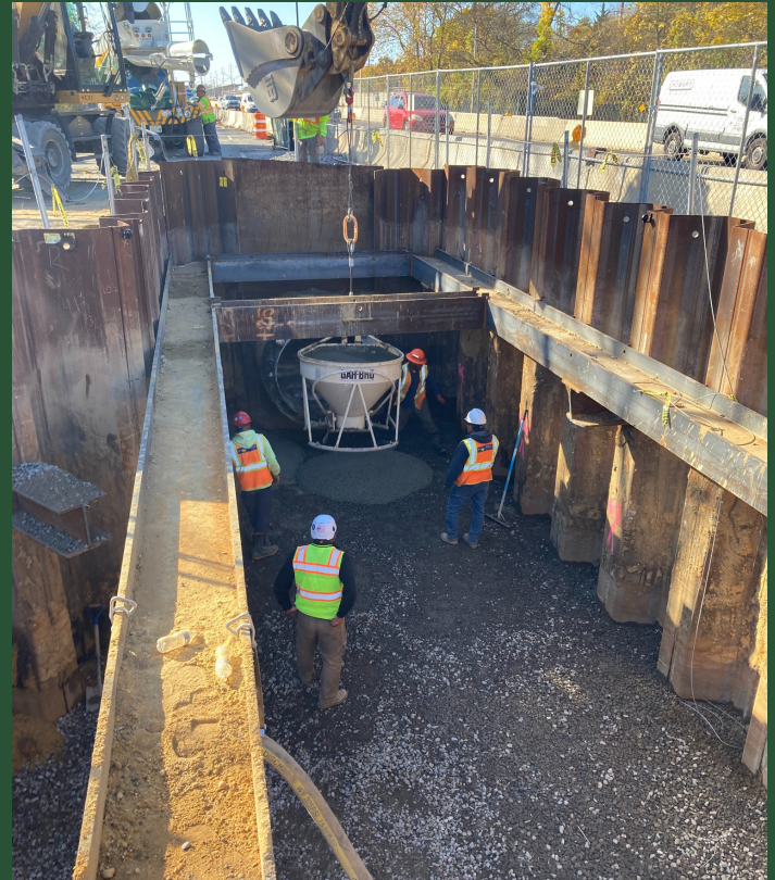
SOE installation at Pit W (November 2022)
