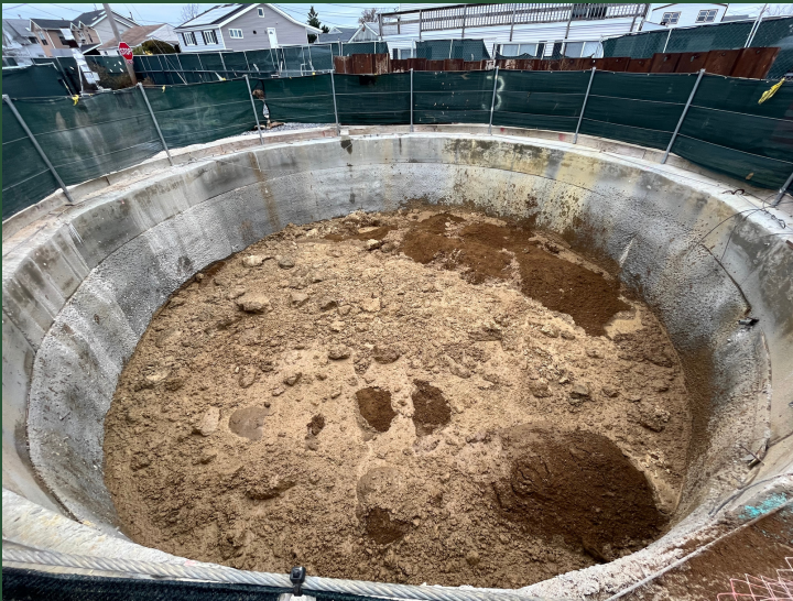
BP2 Backfilling Efforts (December 2022)
