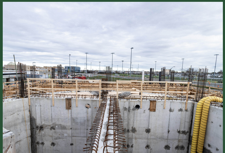
Construction near BP1 (October 2022)
