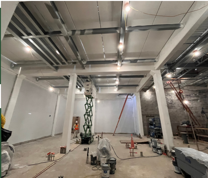
Interior of the new Effluent Diversion Pump Station at SSWRF (November 2023)
