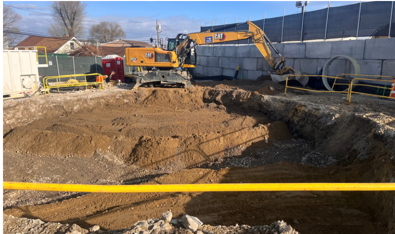
Regrading Activities at BP3 (November 2023)
