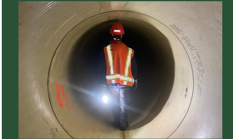
Inspecting the Microtunneling Pipeline (November 2023)
