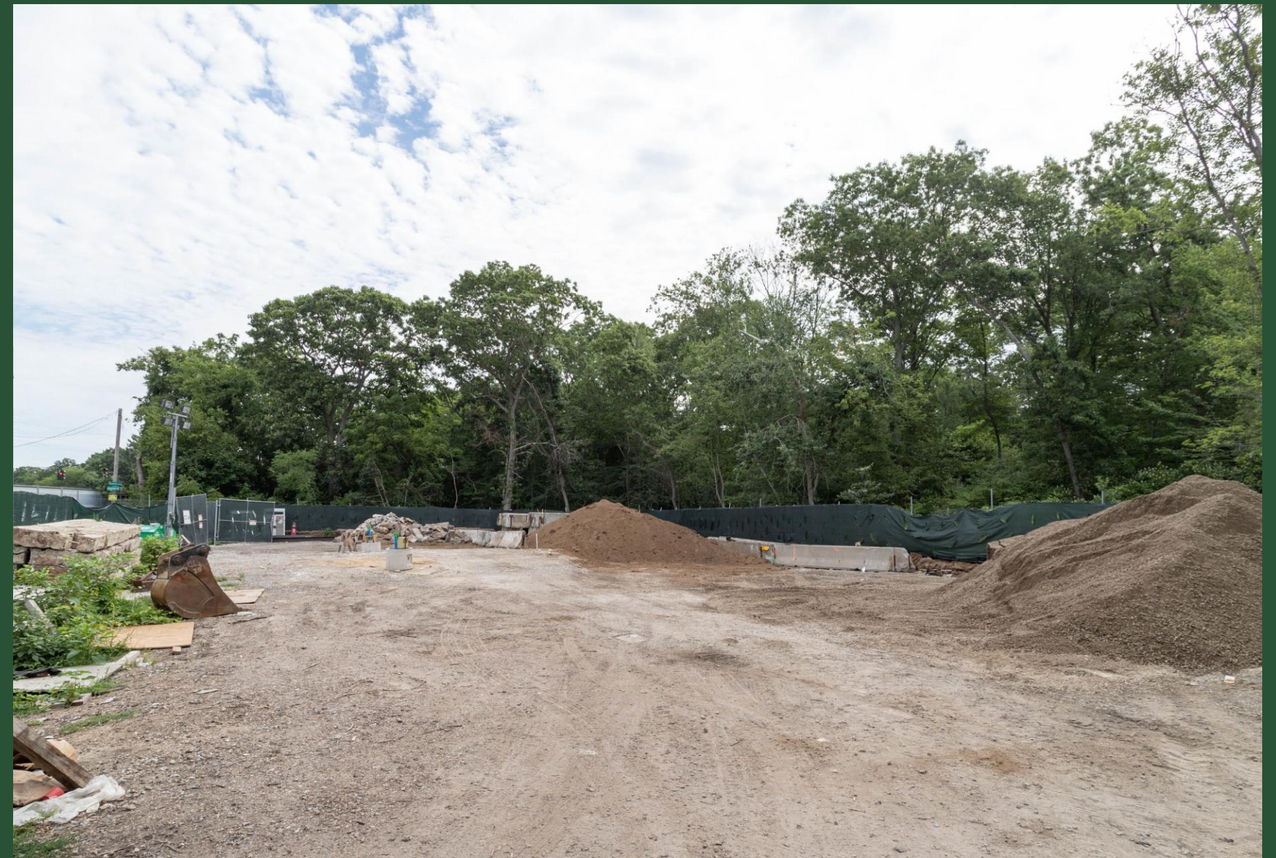
Construction Site at CC6 (July 2022)
