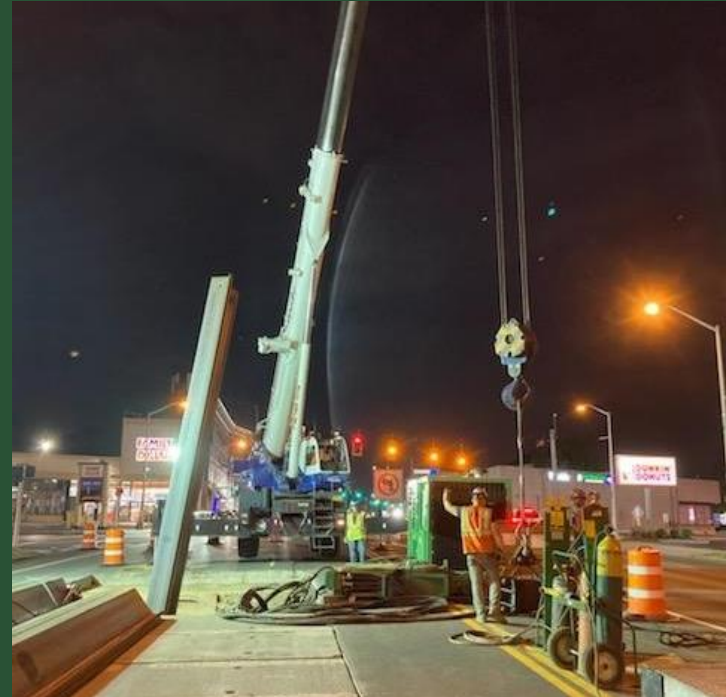
Sheet Pile Installation at Pit N (August 2022)
