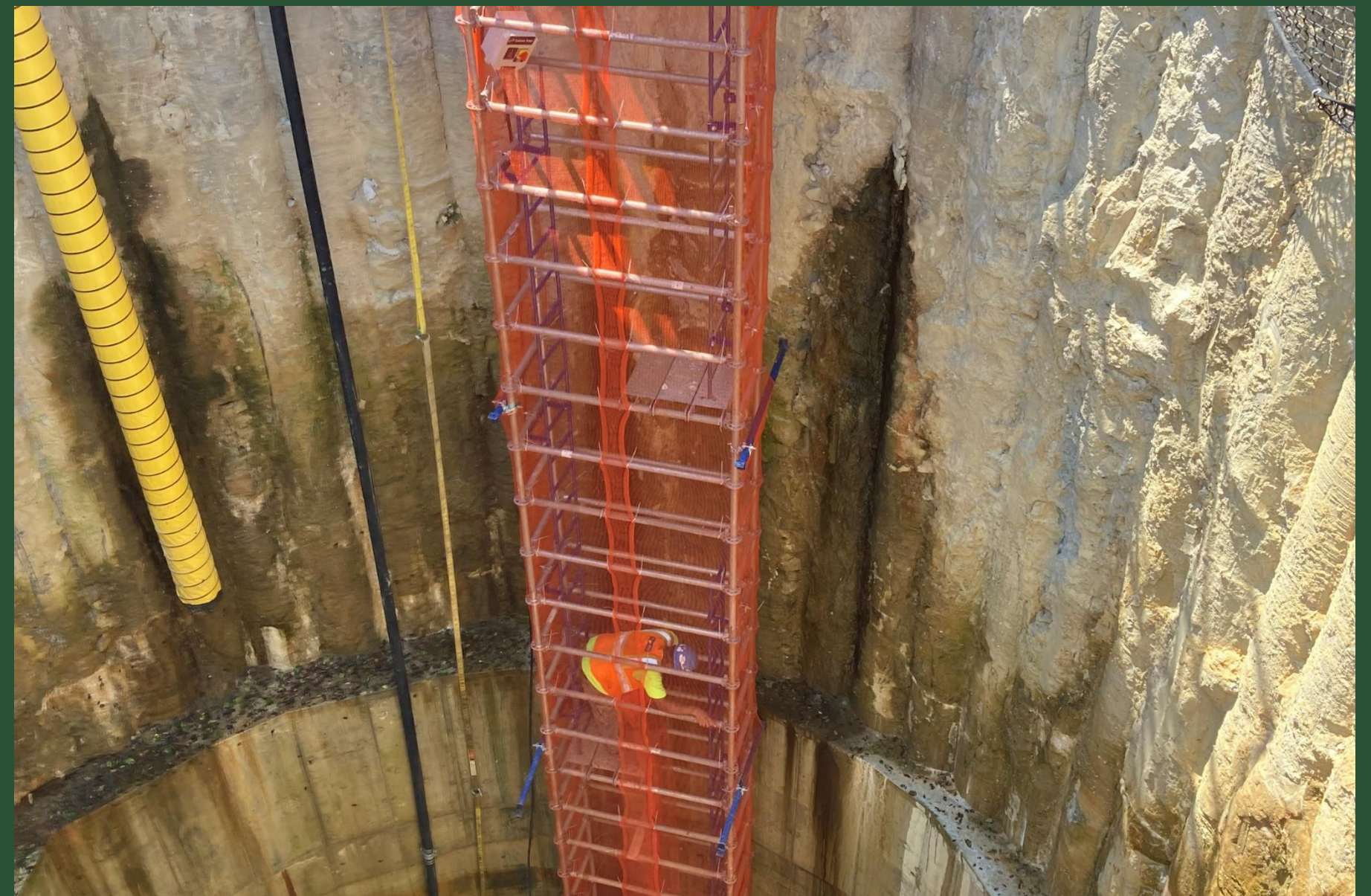
Stair Tower Installation at CC2 (July 2022)
