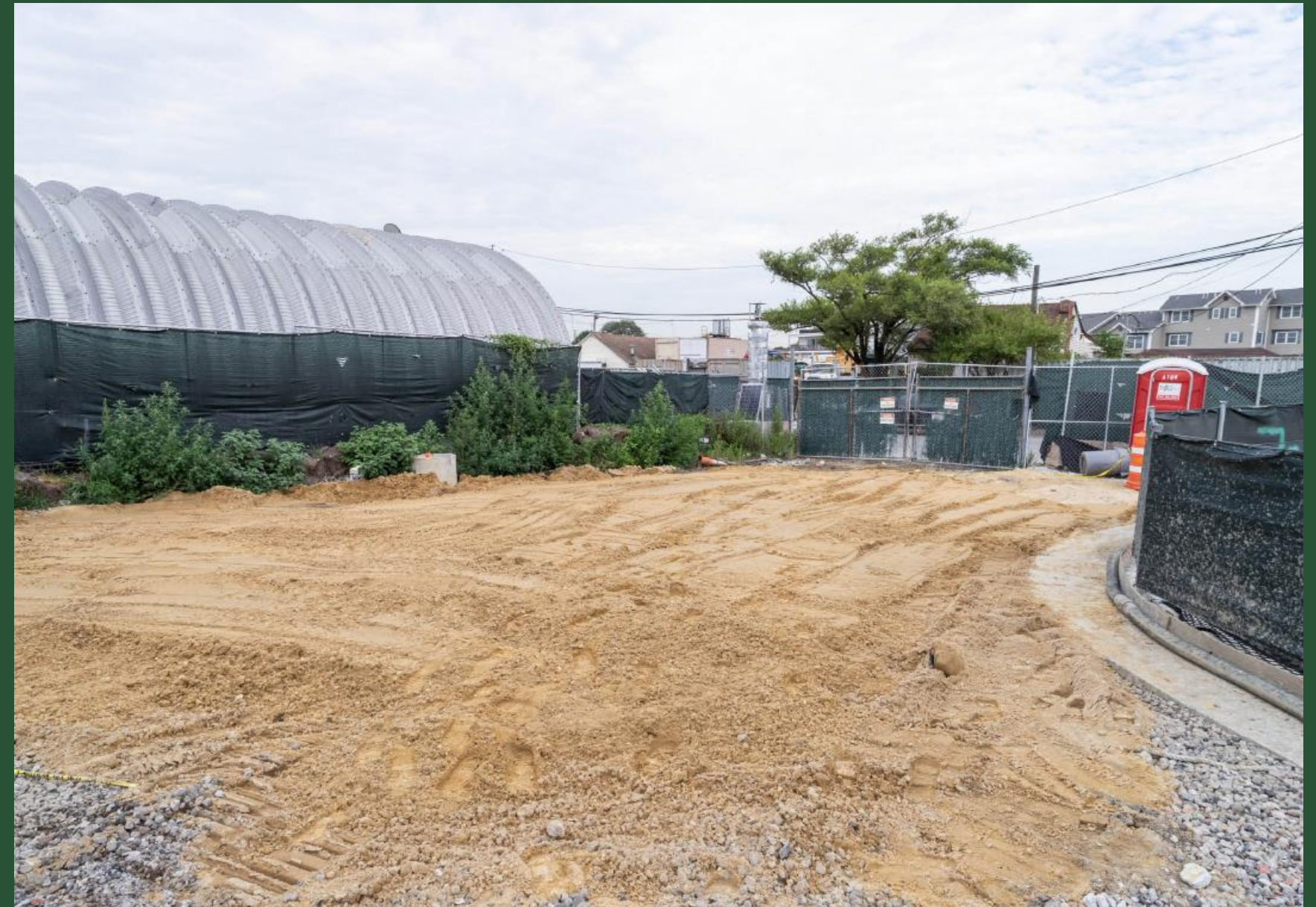
Construction Site at BP3 (July 2022)
