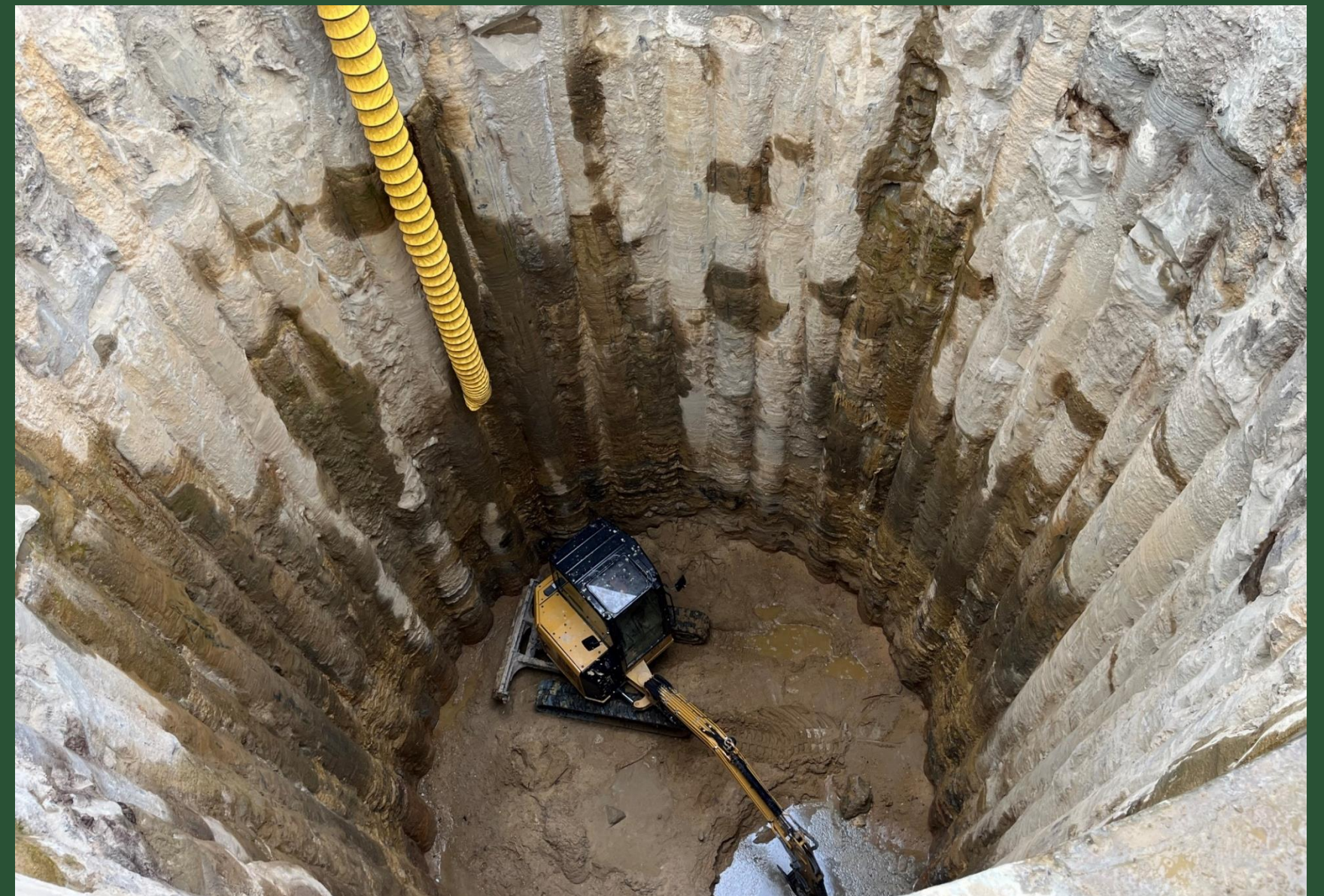
Excavation at BP4 (July 2022)
