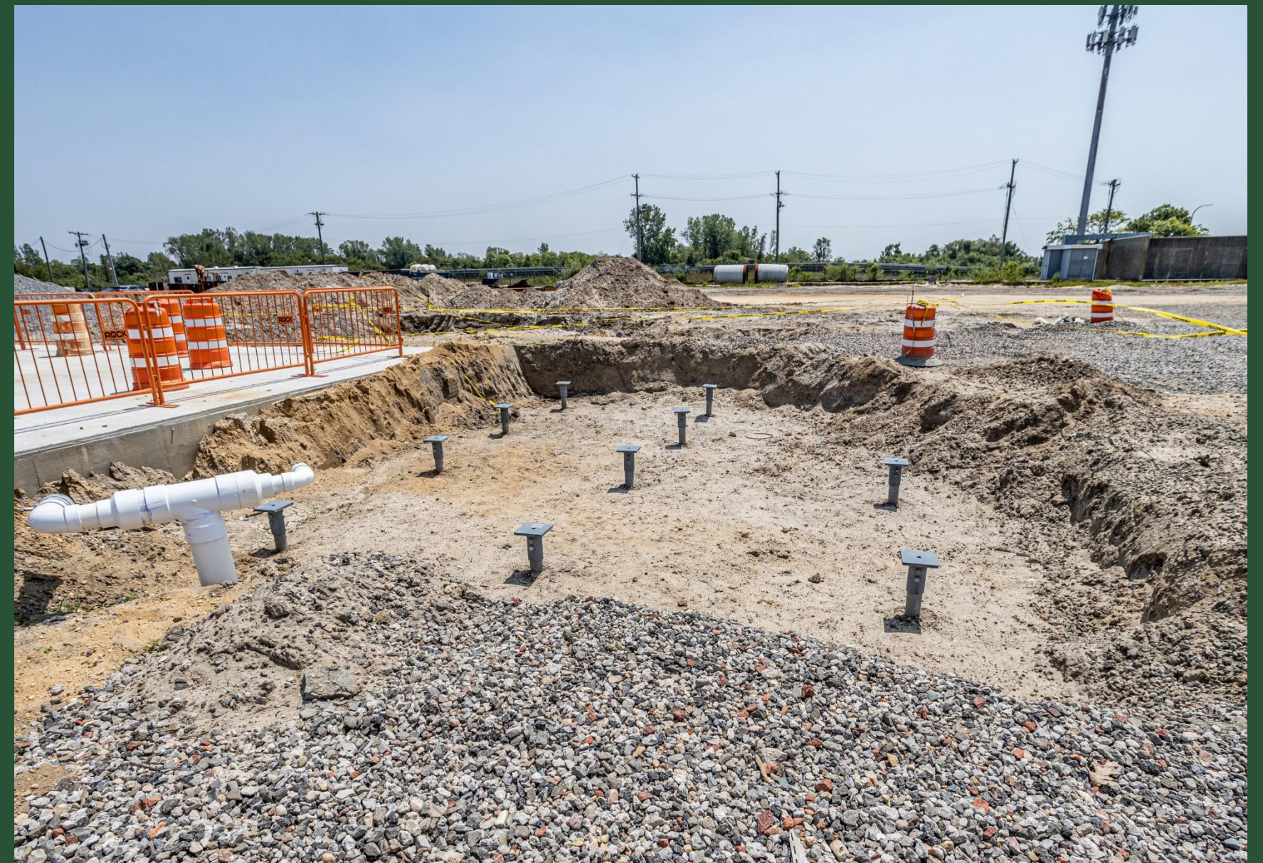
Helical Pile Installation near CC1 (May 2023)
