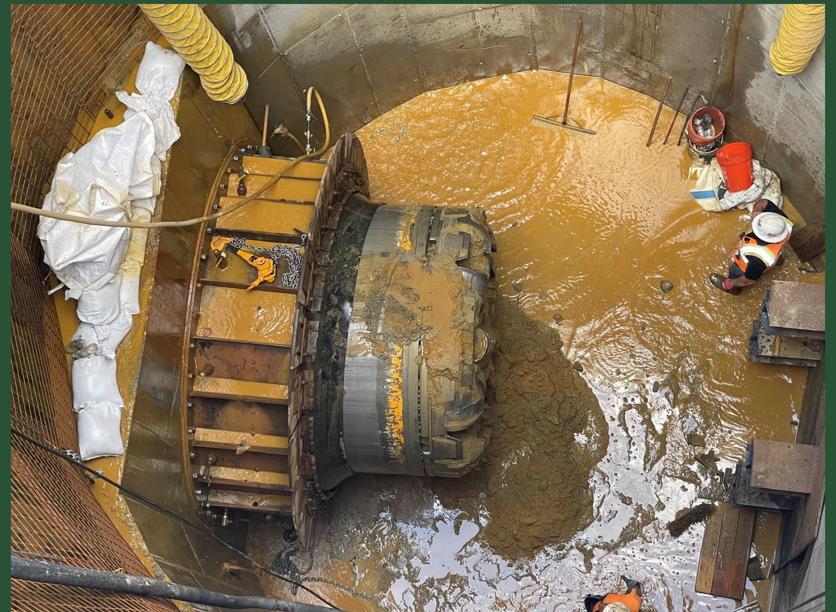
MTBM Breakthrough at BP7 (June 2023)
