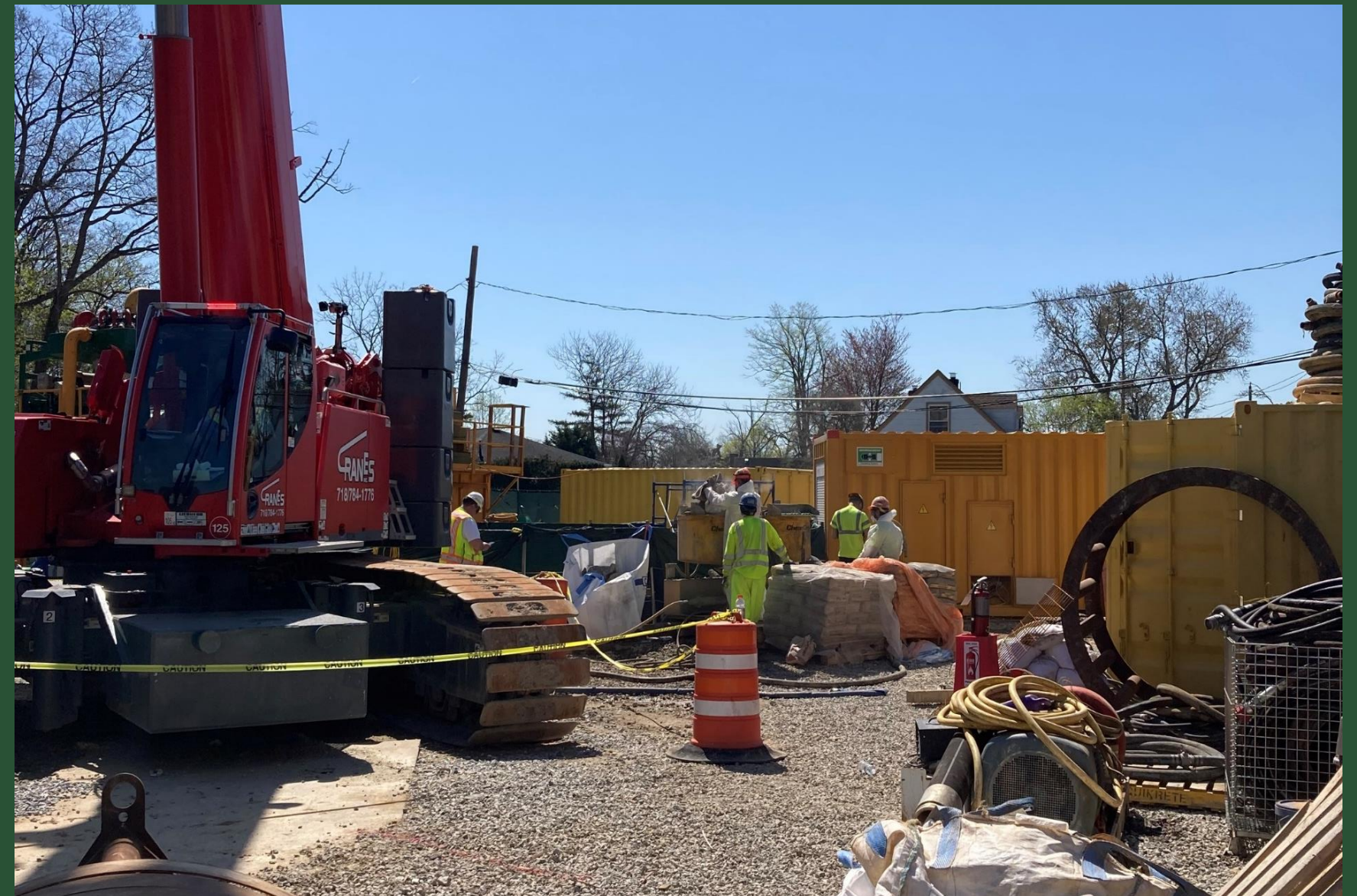
Grouting Activities at CC5 (April 2023)
