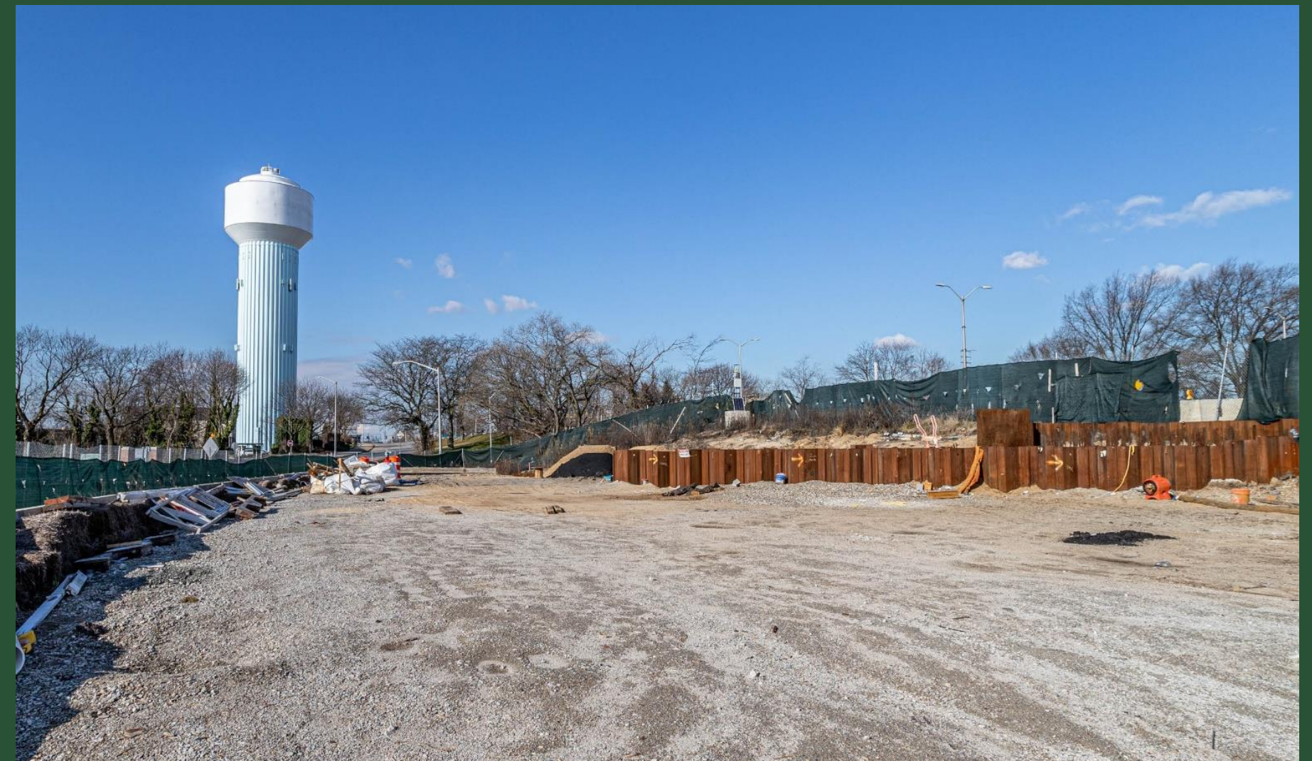
Construction Site at BP9 (January 2023)
