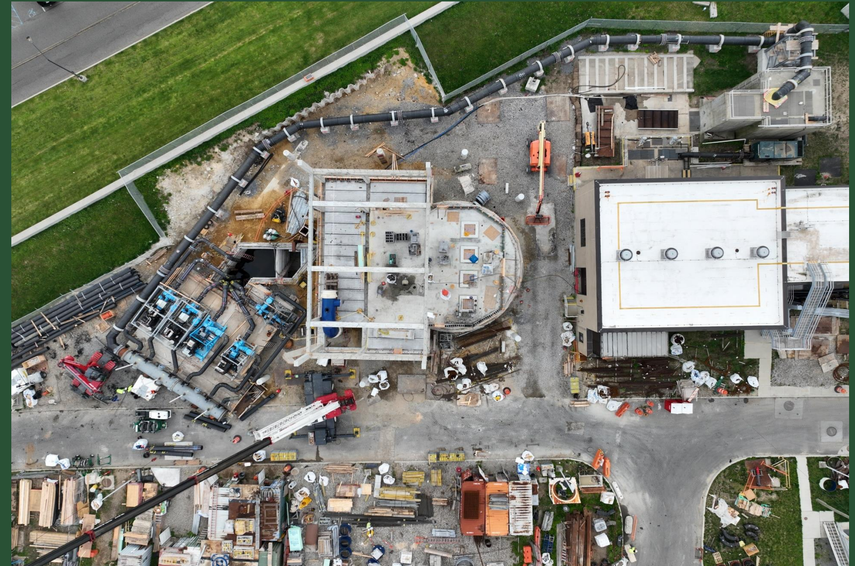
Pump Station Construction Near BP1 (April 2023)
