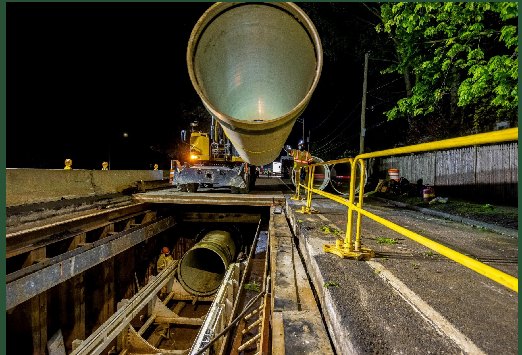
Sliplining at Pit FF (May 2023)
