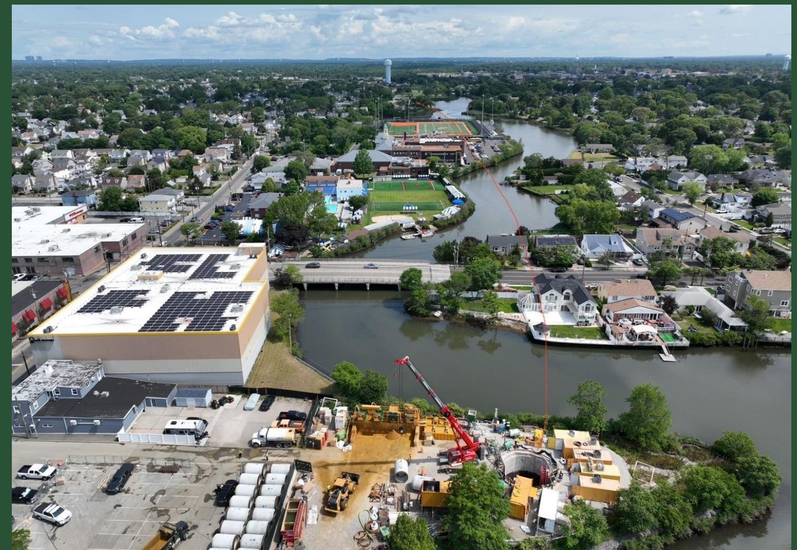
View of Microtunneling Activities at BP5 (June 2023)
