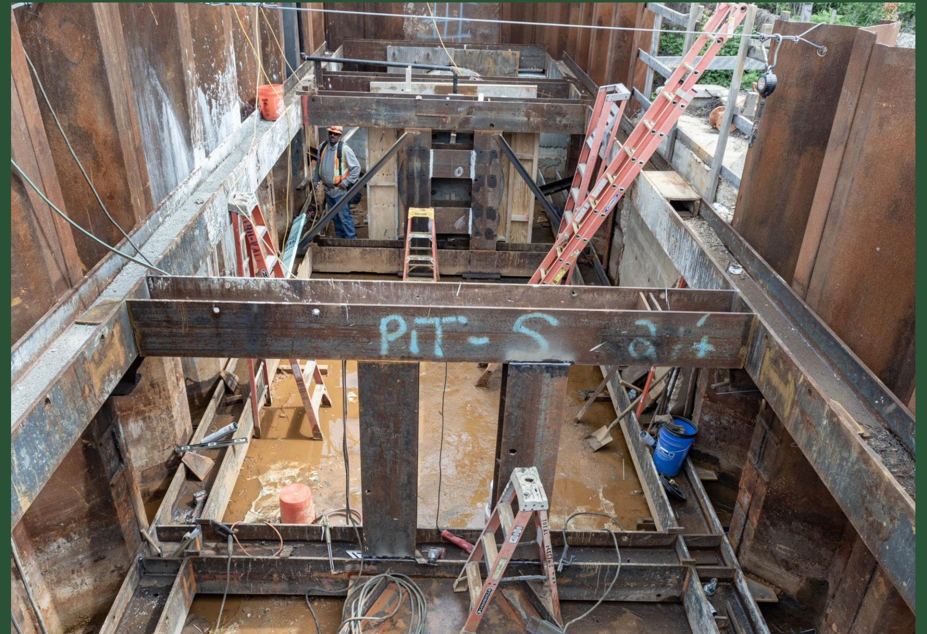
Work at Pit O (April 2023)
