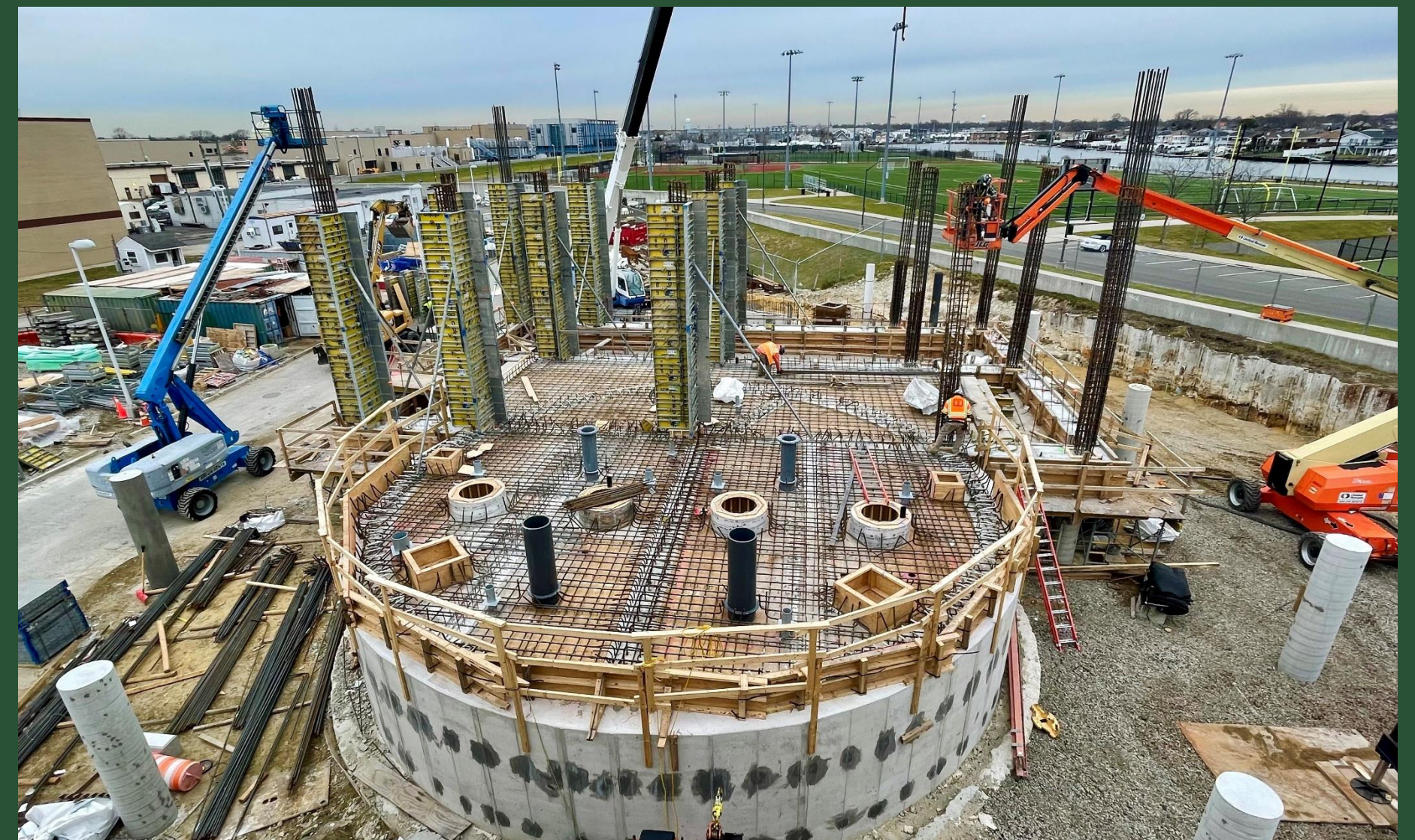
Pump Station Construction Near BP1 (January 2023)
