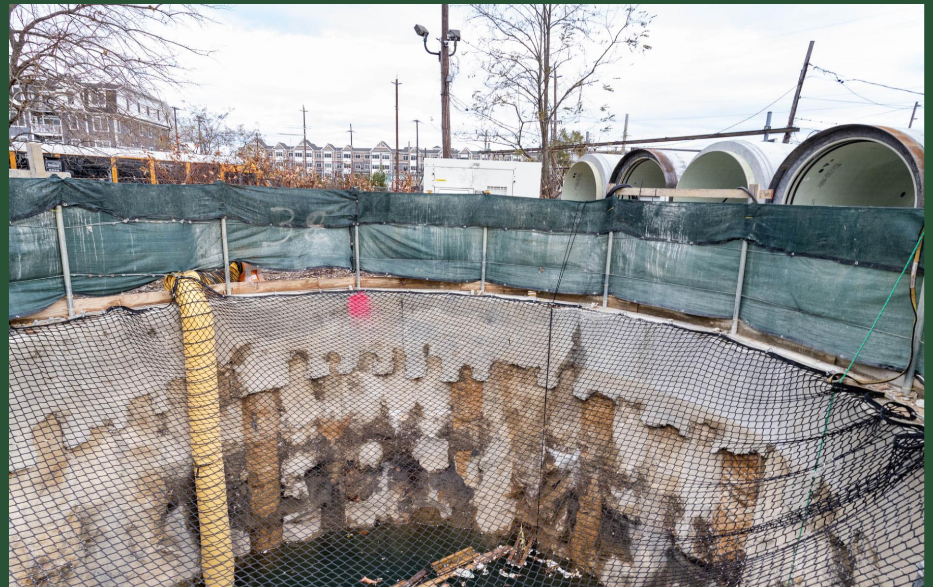
BP4 and Construction Site (November 2022)
