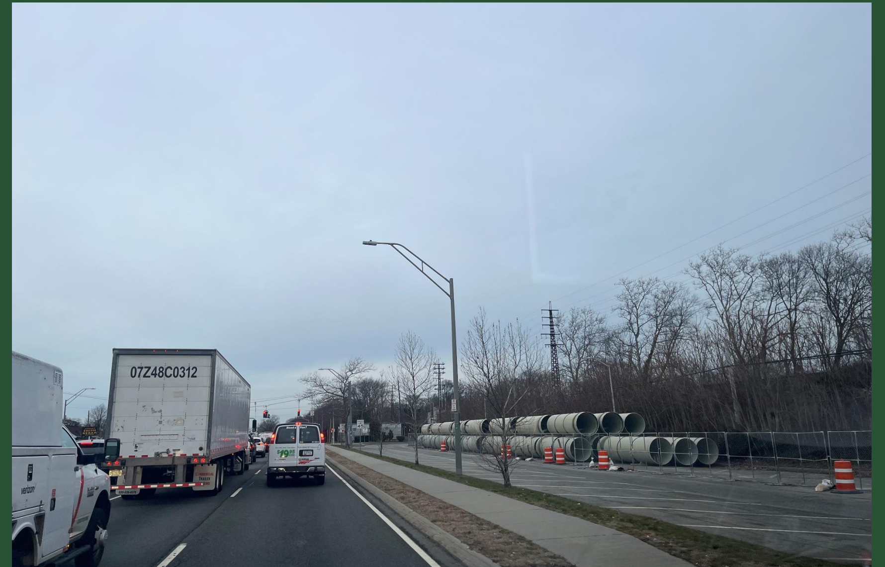
Pipe Storage on Sunrise Highway (January 2023)
