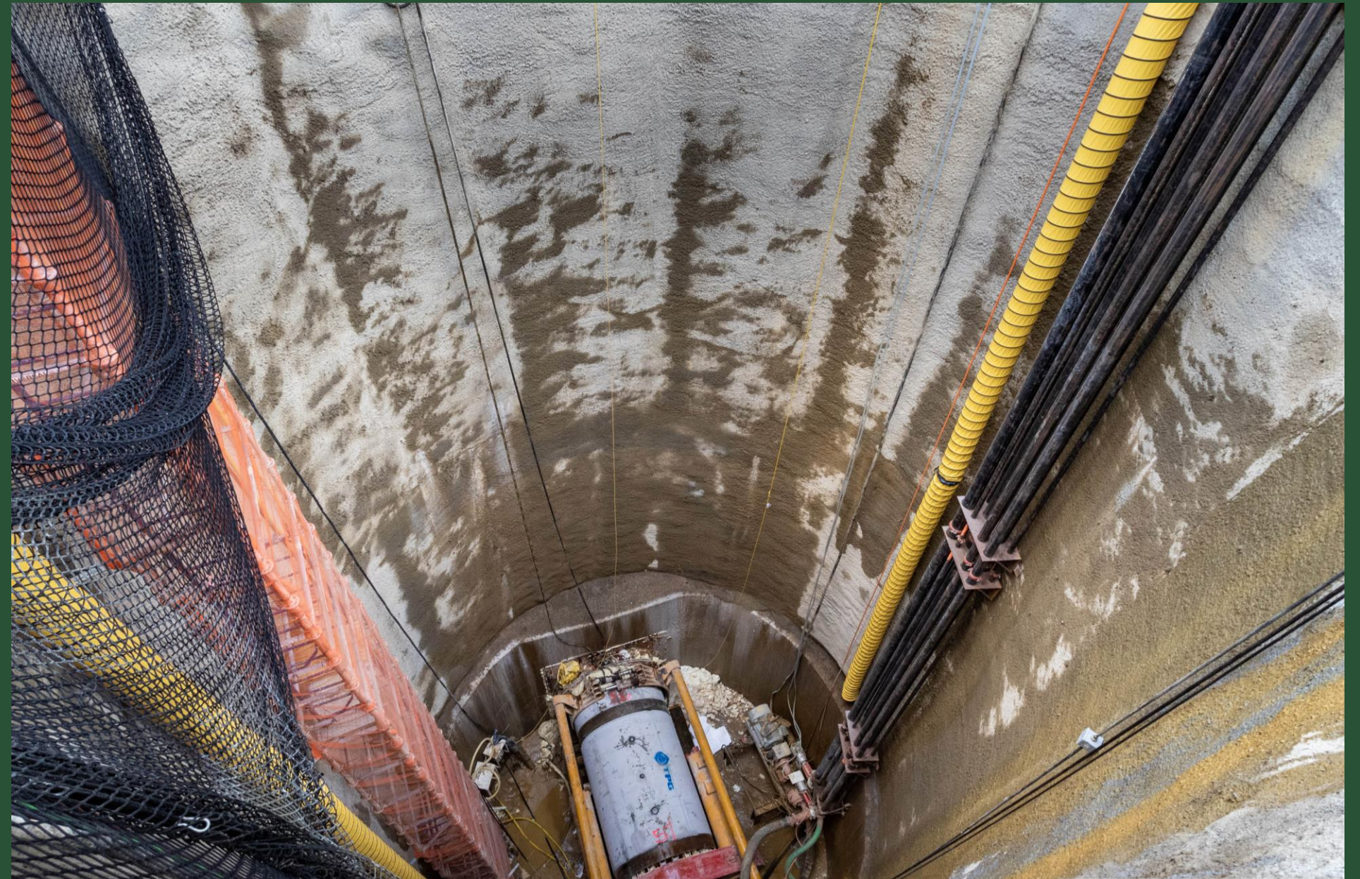
BP3 Microtunnel Activities (November 2022)
