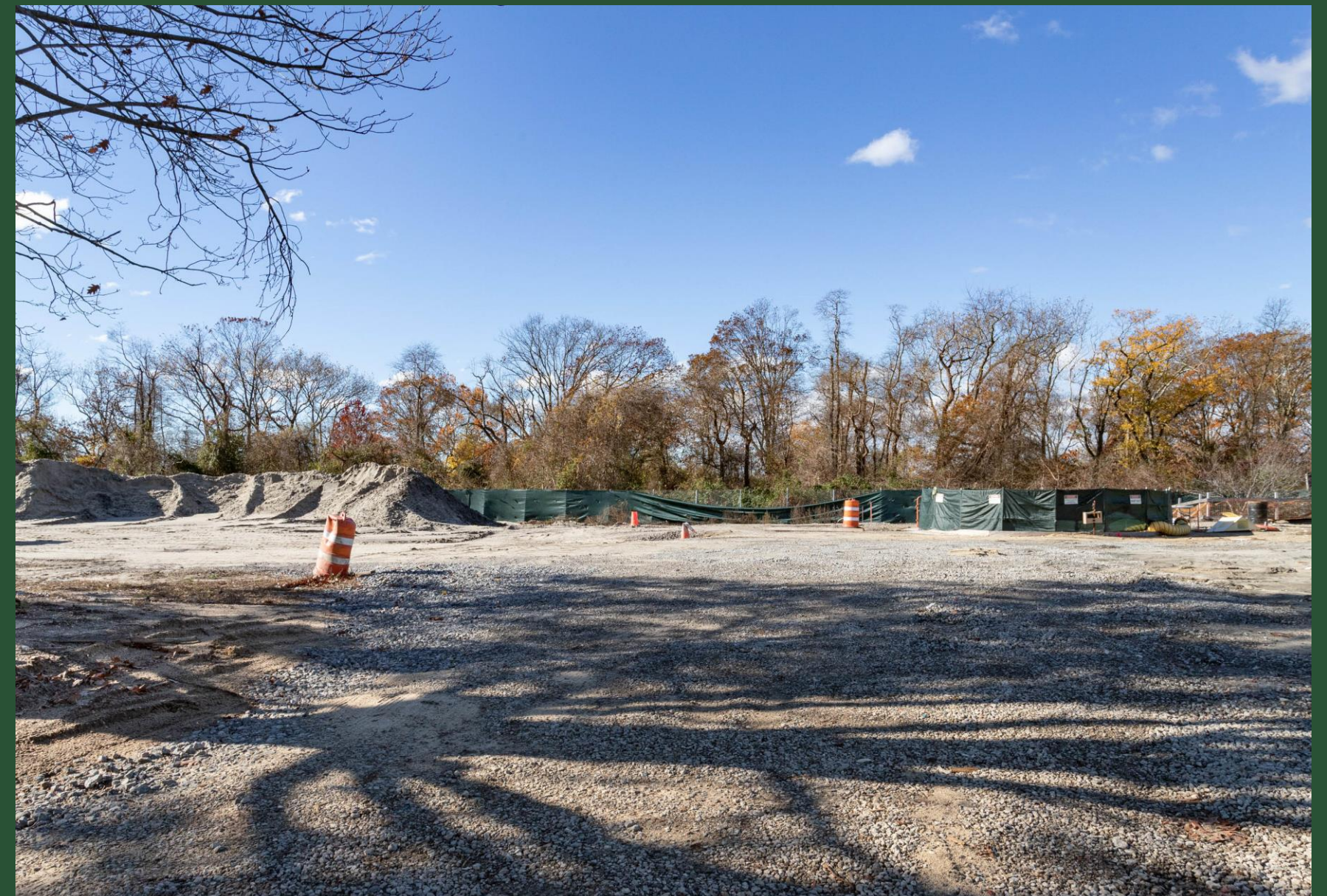
Construction Site at CC4 (November 2022)
