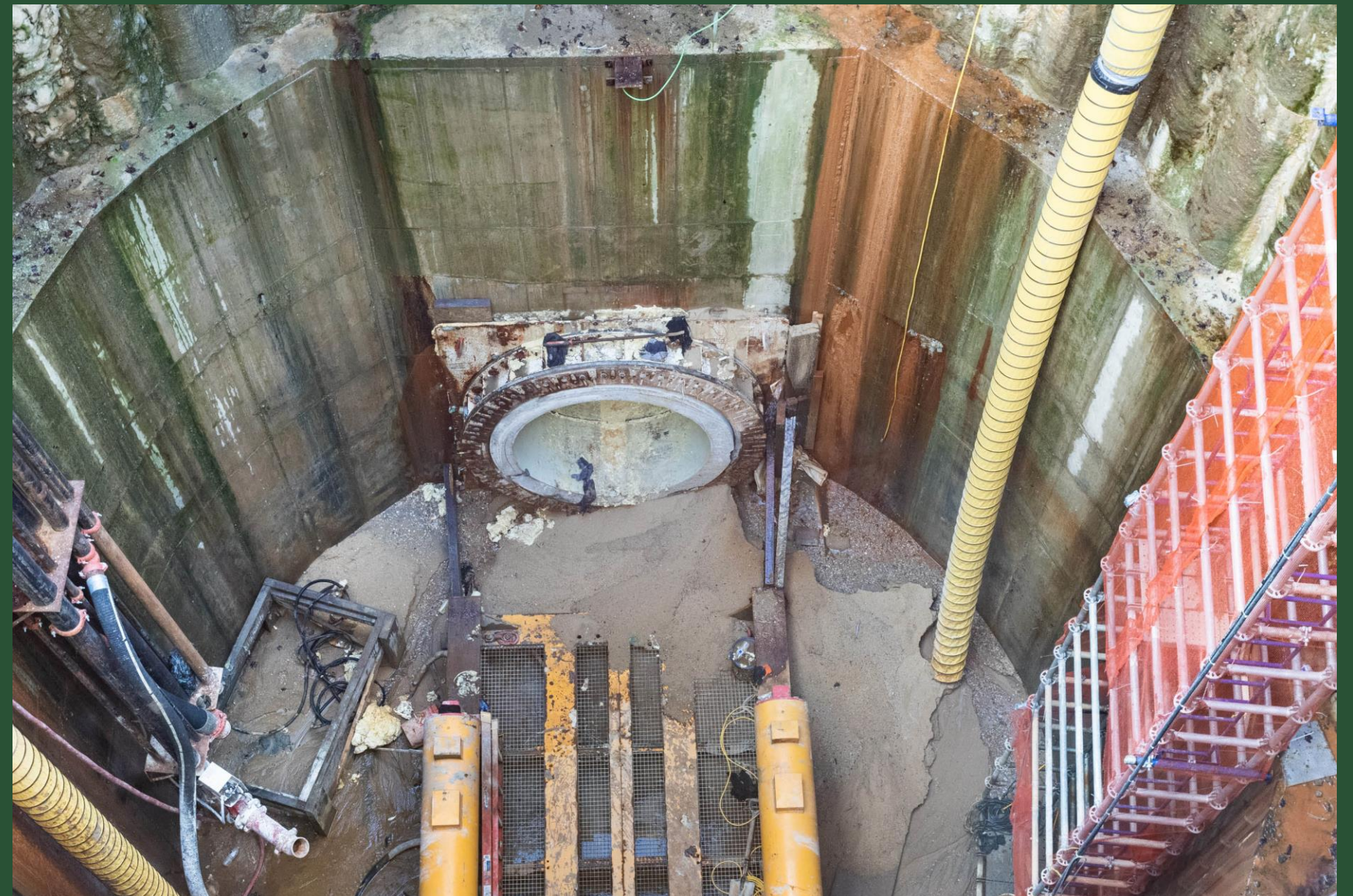
Post Microtunneling Activities at CC2 (November 2022)
