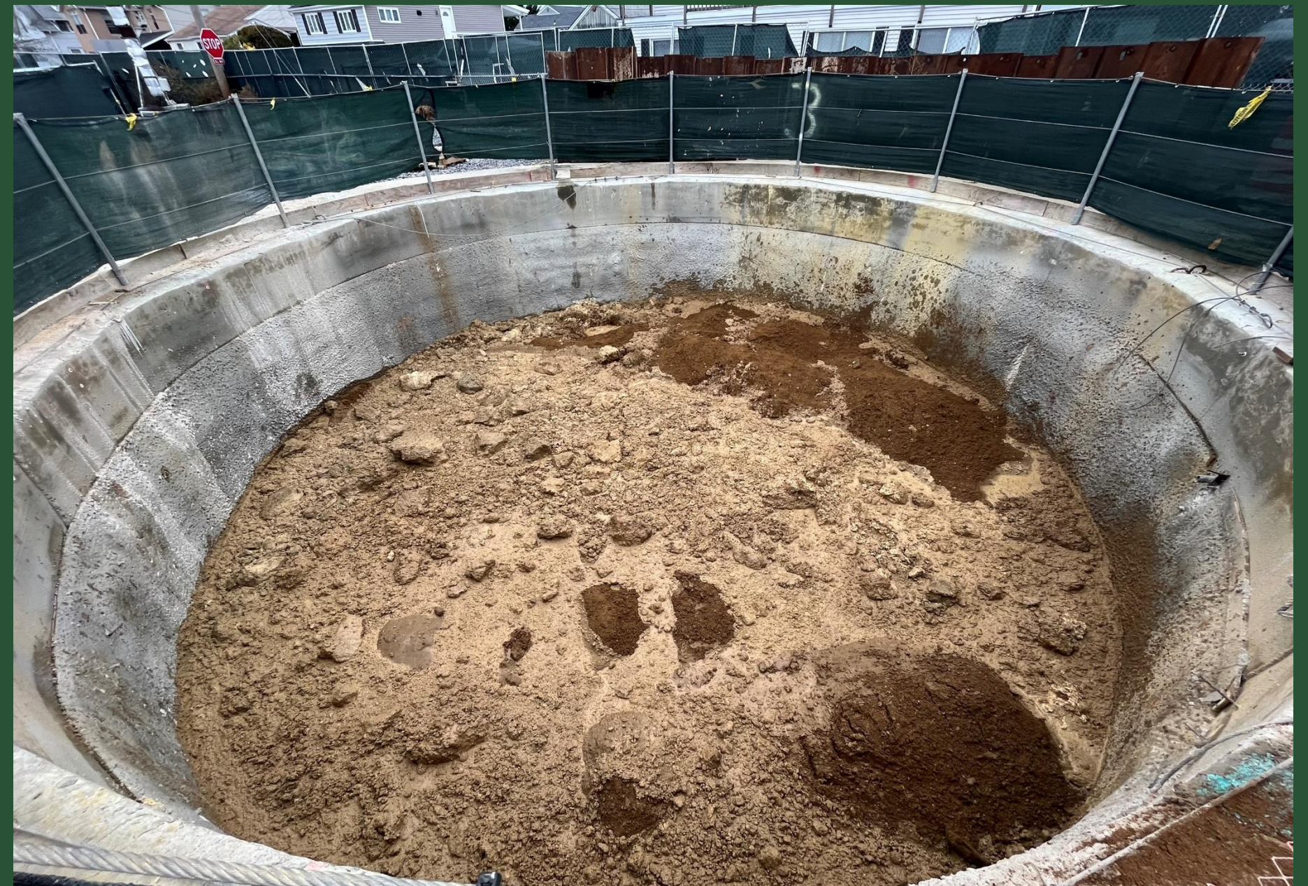
Backfilling at BP2 (December 2022)
