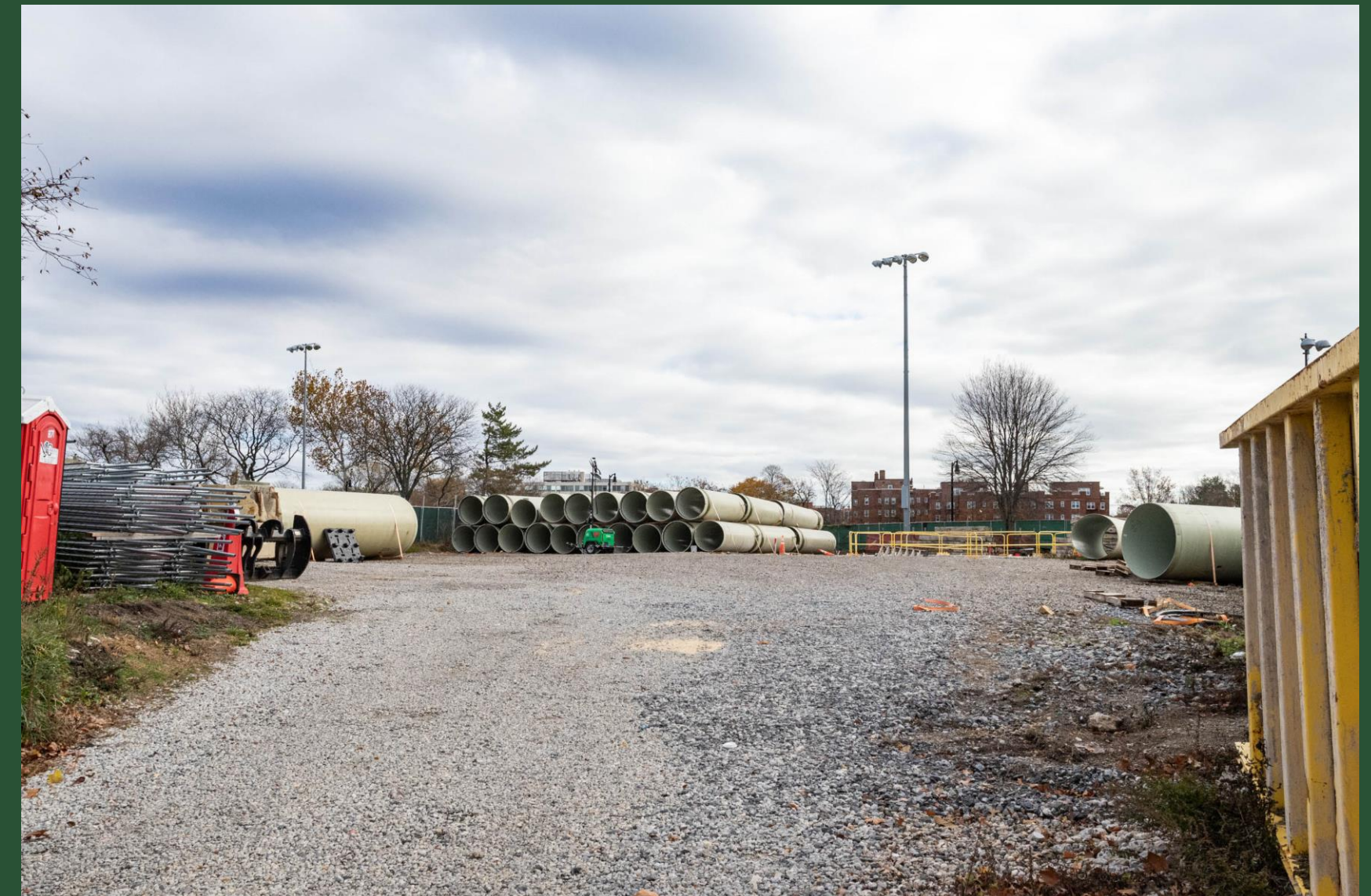
Pipe Storage at BP8 (November 2022)
